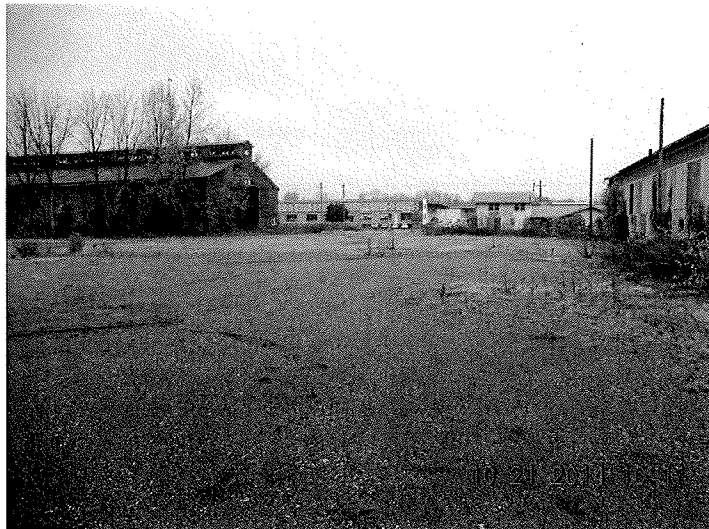
5. Excavation area of Site, facing northeast.
