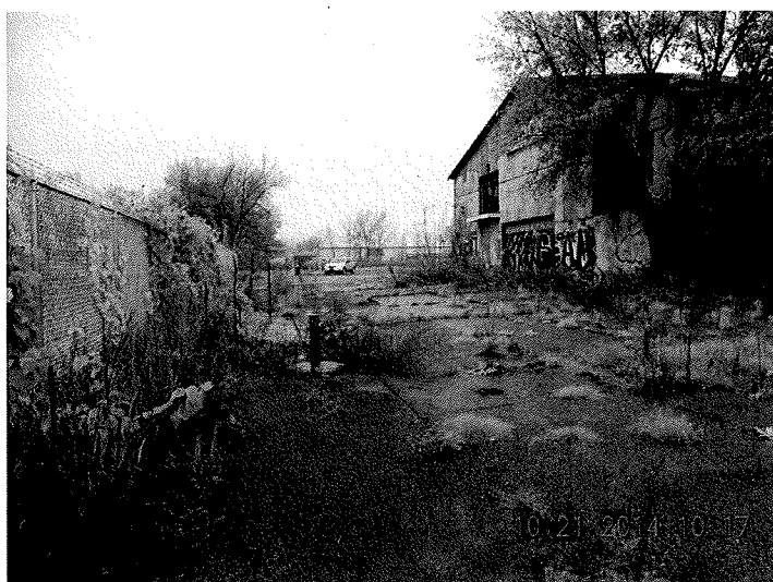
3. Southwestern portion of Site, facing northwest.
