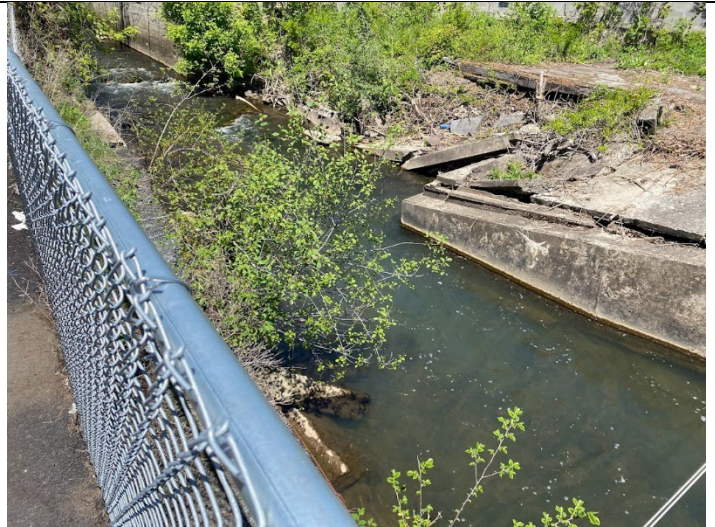
Photo 10: View of woody vegetation protruding from the retaining wall, looking west.
