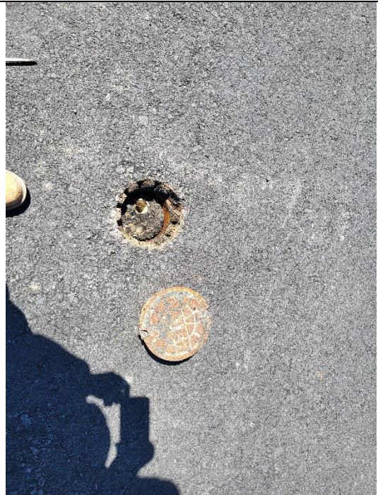
Photo 12: View of HRP-MW-7 with municipal water supply manhole. TRC was unable to sample due to the riser being clogged with debris,
