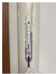
Delaware, access to document the manometer was not provided during the 2020 time period. When observed in February, 2021 the manometer read 2.6" WC, demonstrating sub-slab de-pressurization.
