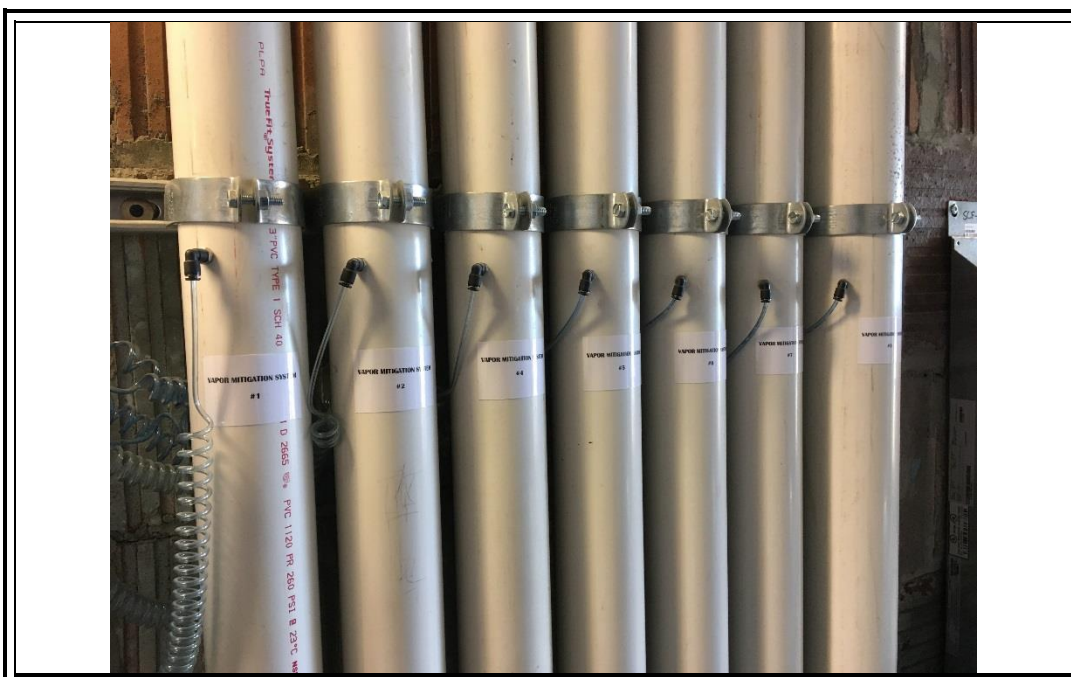
Photo 14: Vertical riser pipes for the seven sub-systems comprising the vapor mitigation system at 144 State Street.
