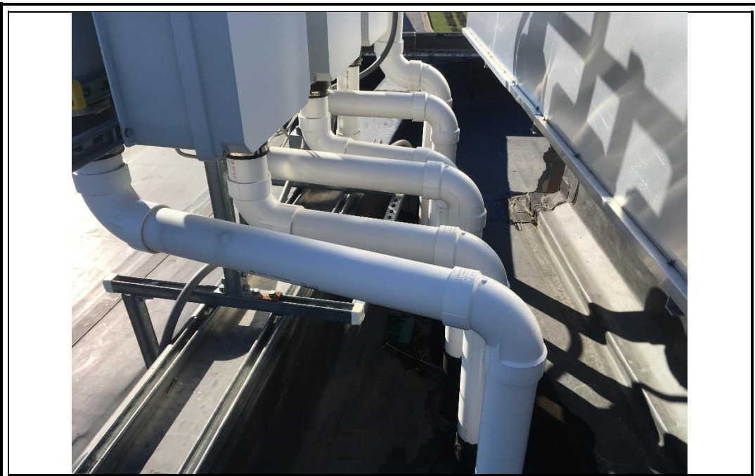
Photo 16: Vapor mitigation system piping connecting the vertical riser pipes with the fans at 144 State Street.
