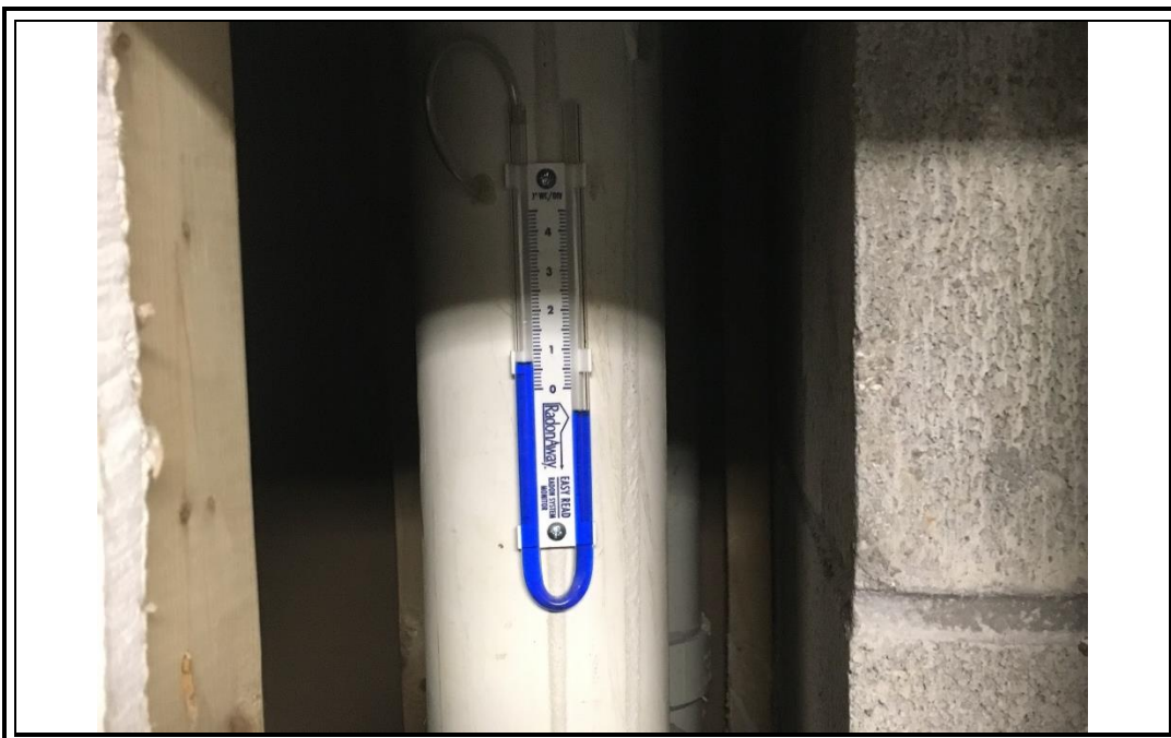
Photo 10: Vacuum gauge on vertical riser pipe for vapor mitigation system at 140 State Street (gauge accessed via a wall hatch in the basement).
