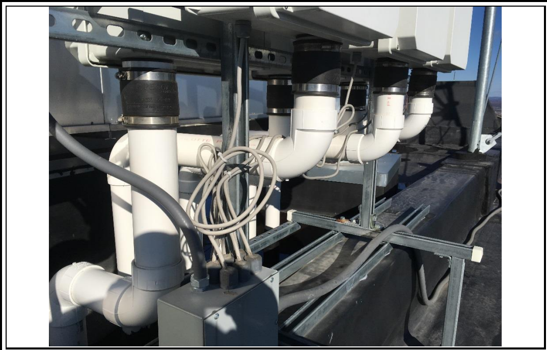
Photo 17: Vapor mitigation system piping connecting the vertical riser pipes with the fans at 144 State Street.
