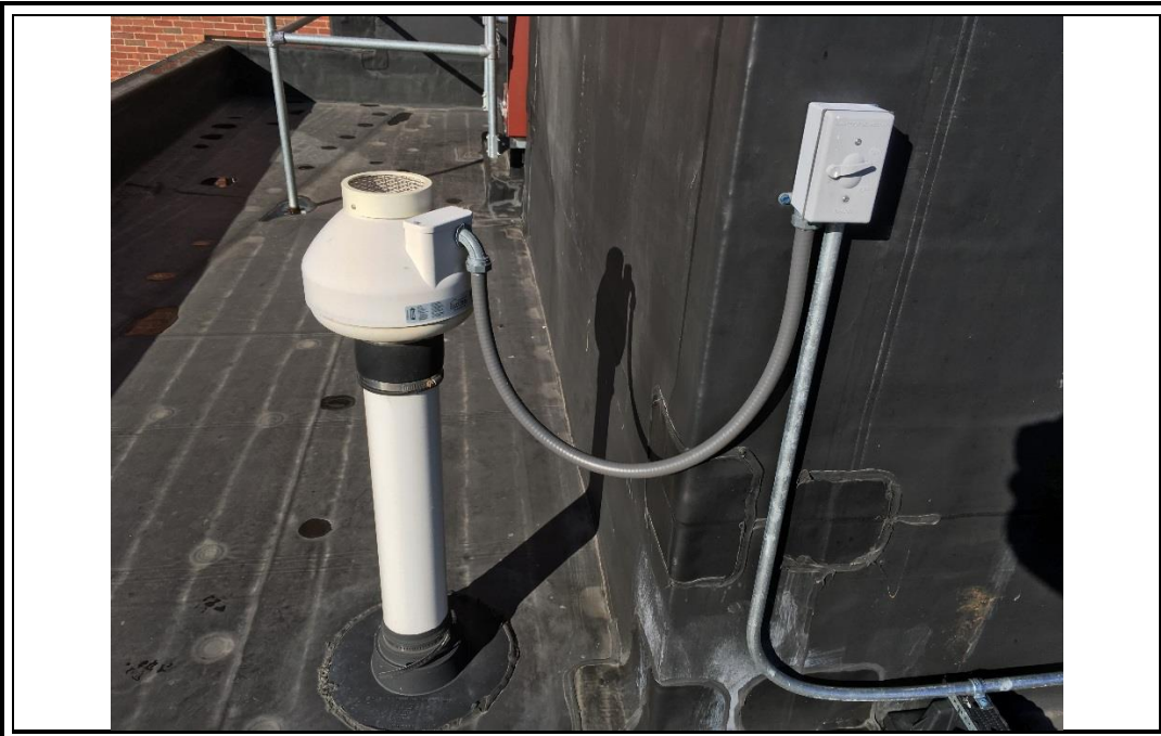
Photo 11: Fan and vapor mitigation system exhaust point on the roof of 140 State Street.
