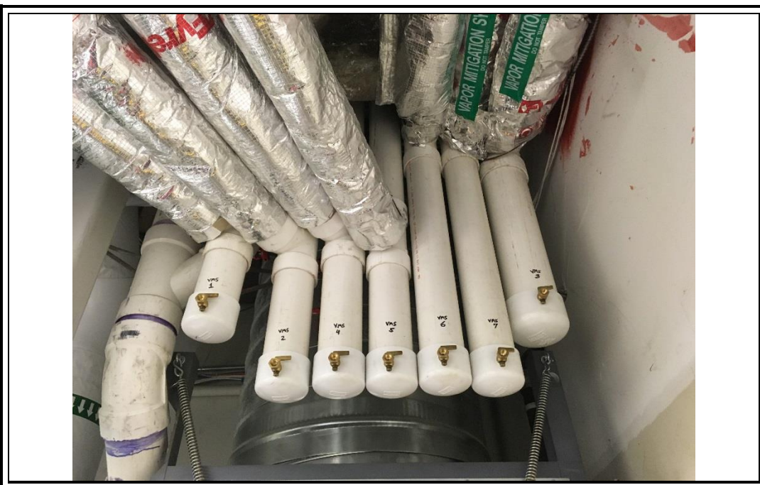
Photo 12: Bottoms of vertical riser pipes for the vapor mitigation system at 144 State Street (pipes are accessed via a closet in the basement of the building).
