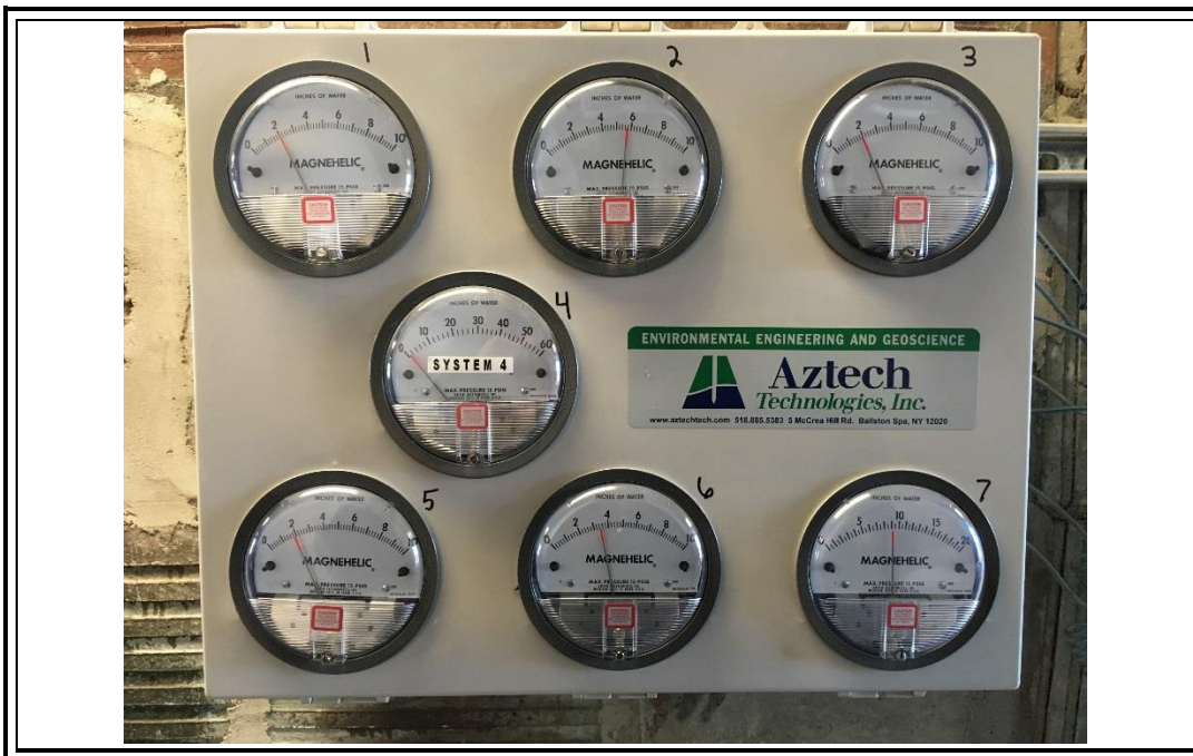
Photo 13: Vacuum gauge panel for vapor mitigation system at 144 State Street.
