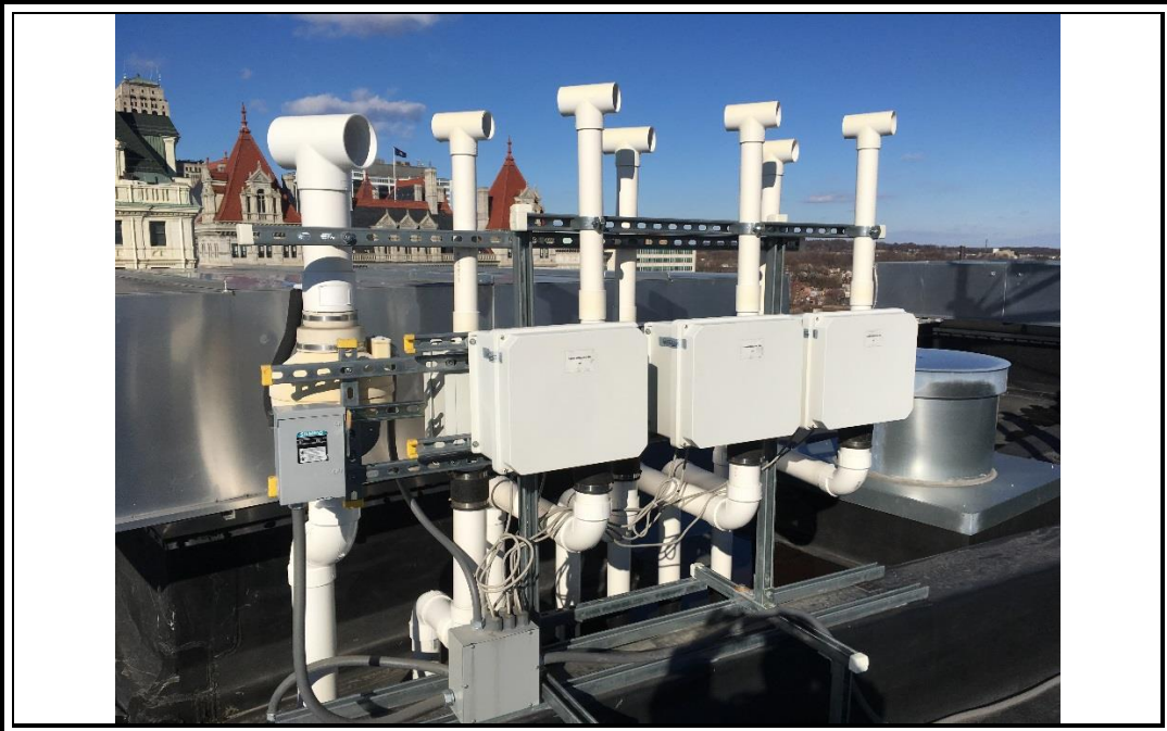
Photo 15: Vapor mitigation system fans and exhaust piping on the roof of 144 State Street.
