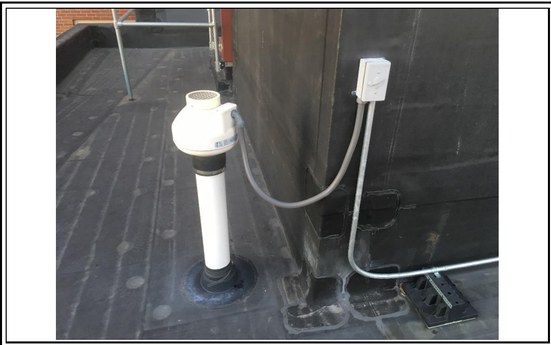
Photo 18: Roof of 140 State Street building; exhaust stack, fan and switch for the sub-slab depressurization system (12/10/18).
