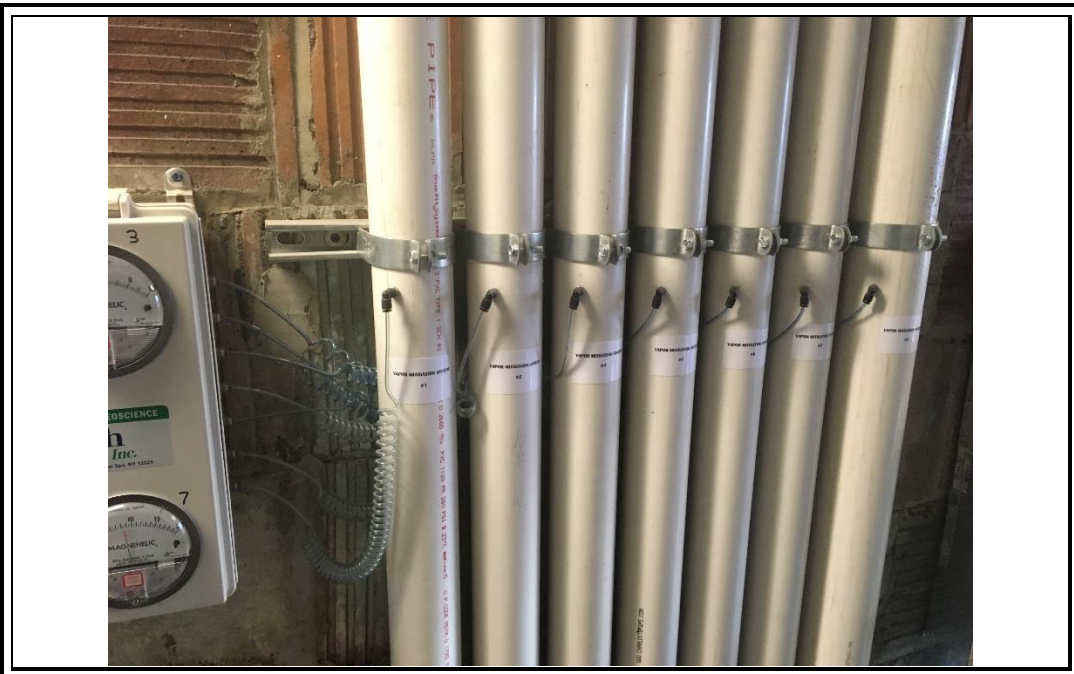
Photo 2: Close-up view of riser pipes for individual subsystems and tubing associated with the magnehelic manometers (12/05/18).
