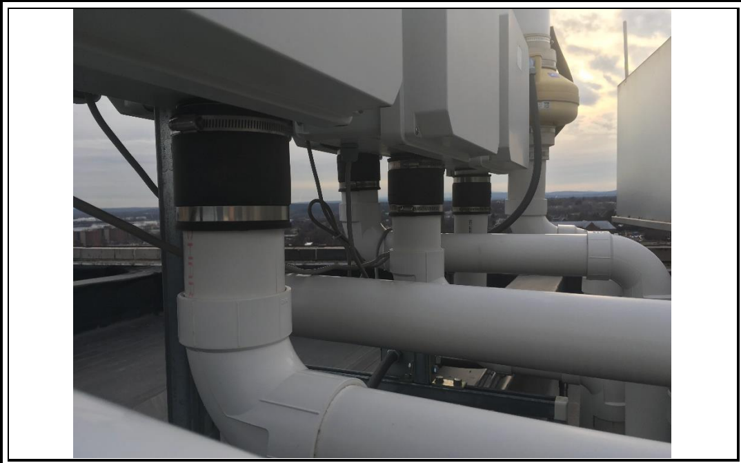
Photo 7: Piping connections to fans for individual subsystems at 144 State Street (12/05/18).
