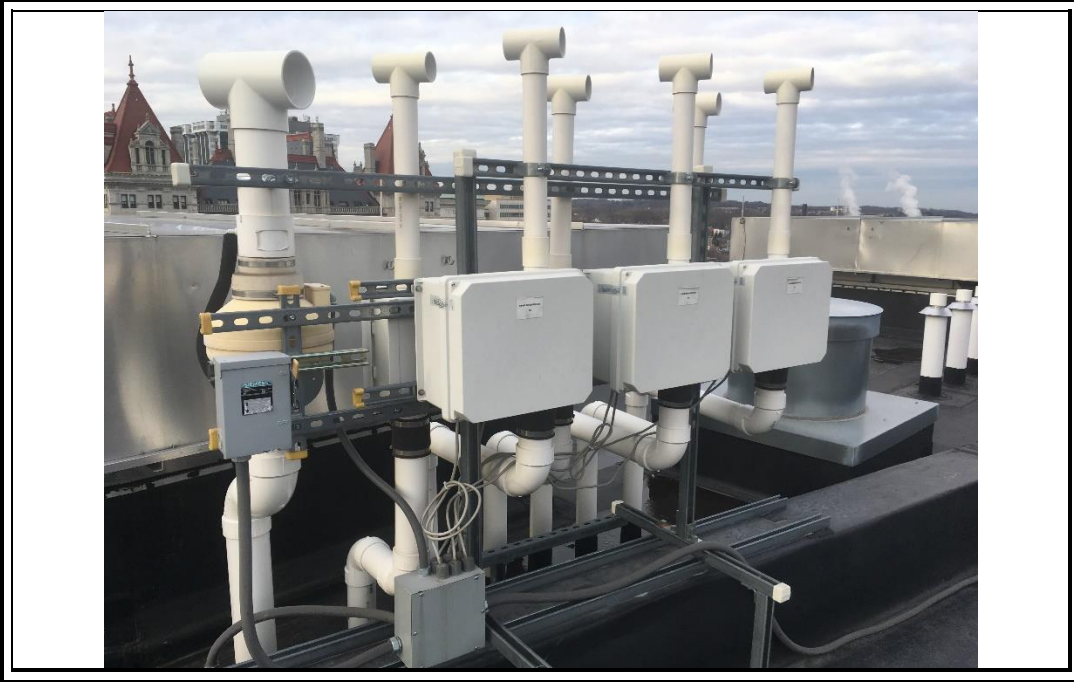
Photo 5: Roof-mounted fan units and exhaust points for individual subsystems at 144 State Street (12/05/18)
