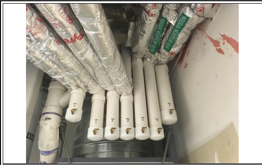
Photo 9: Inside laundry chute room in basement of 144 State Street; horizontal piping for individual subsystems connected to vertical riser pipes; condensation collection sumps comprise bottom portion of each vertical riser pipe (12/05/18) .
