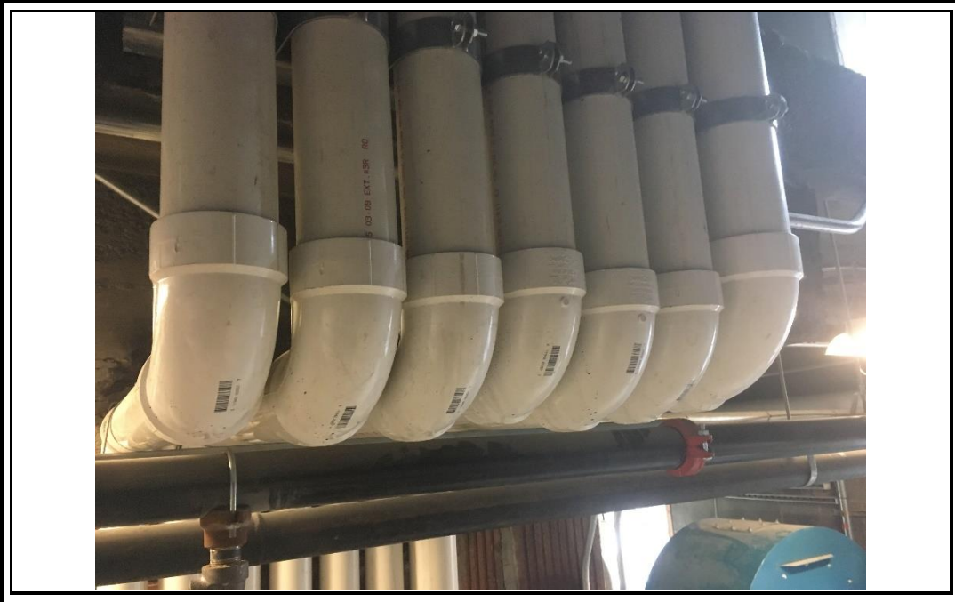
Photo 3: Riser pipes for individual subsystems (12/05/18).
