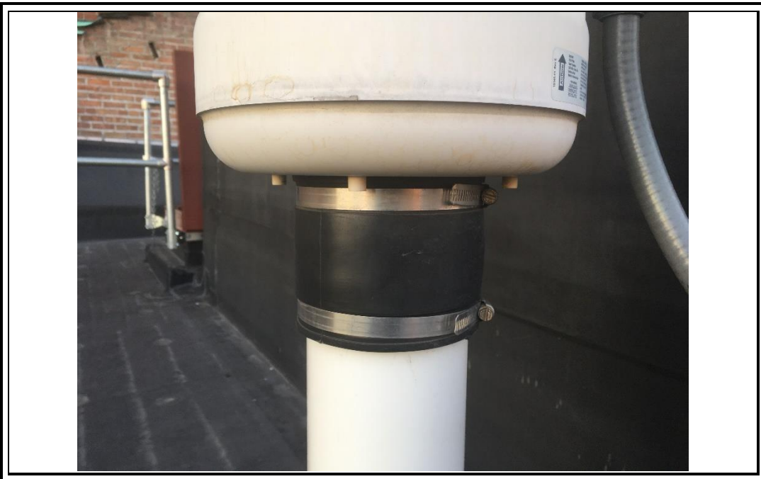
Photo 20: Close-up view of connection between SSDS exhaust stack and fan at 140 State Street (12/10/18).
