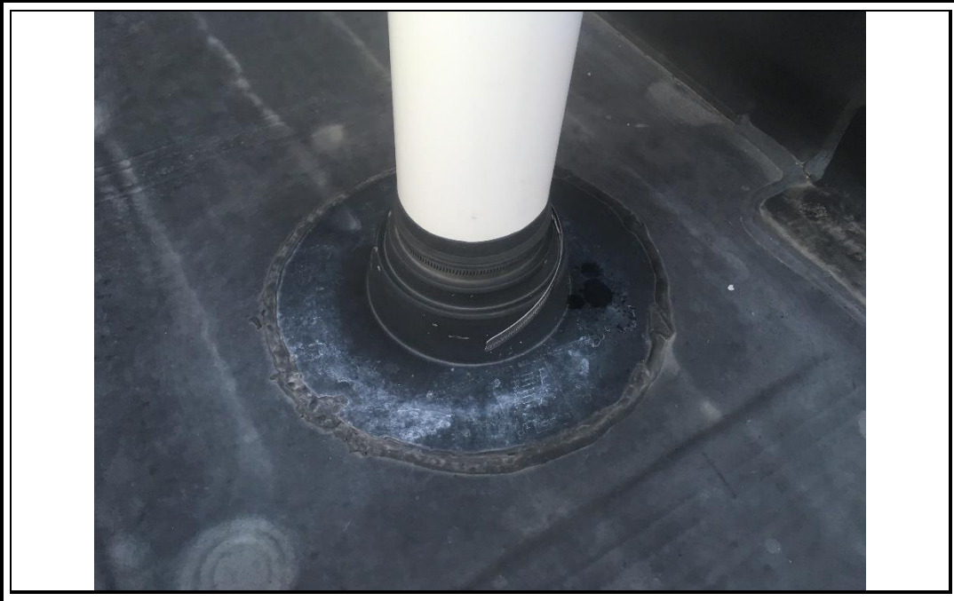
Photo 19: Close-up view of roof penetration point for SSDS exhaust stack at 140 State Street (12/10/18).
