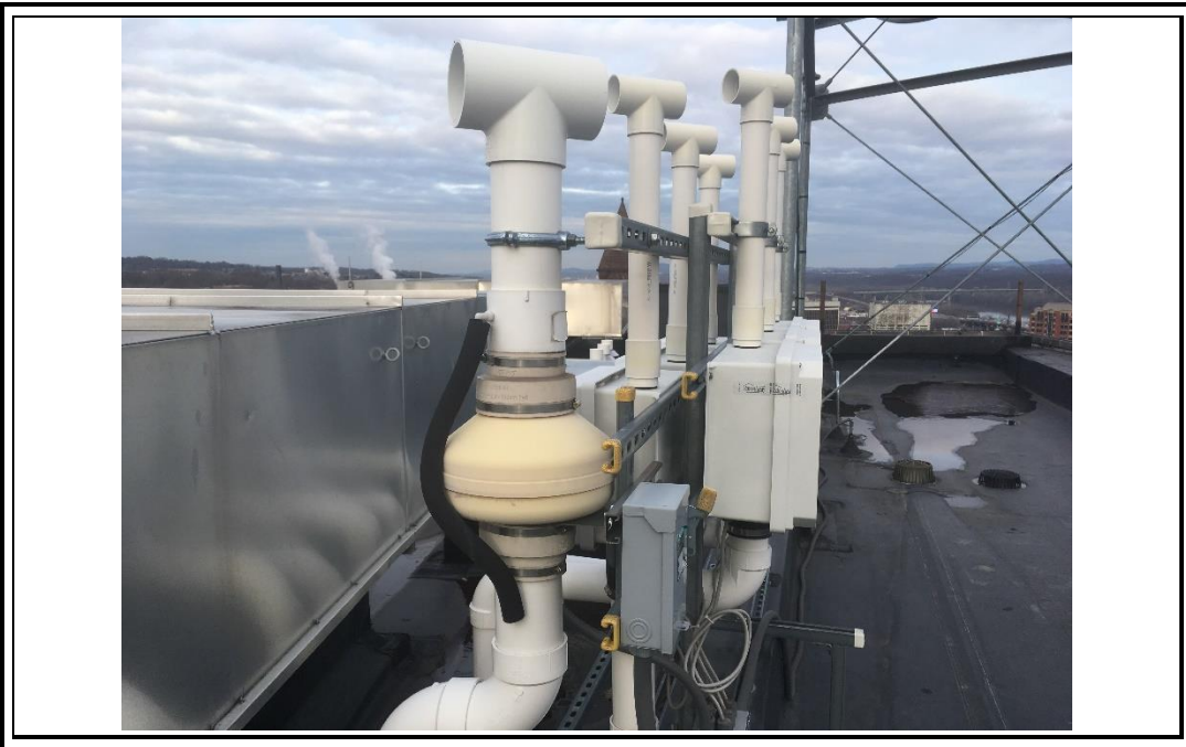
Photo 6: Roof-mounted fan units and exhaust points for individual subsystems at 144 State Street (12/05/18)
