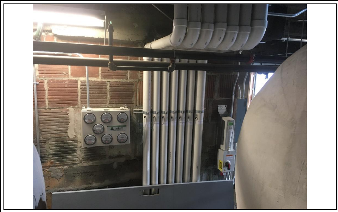
Photo 1: Magnehelic manometer panel and riser pipes for the seven individual subsystems comprising the sub-slab depressurization system at 144 State Street (12/05/18).
