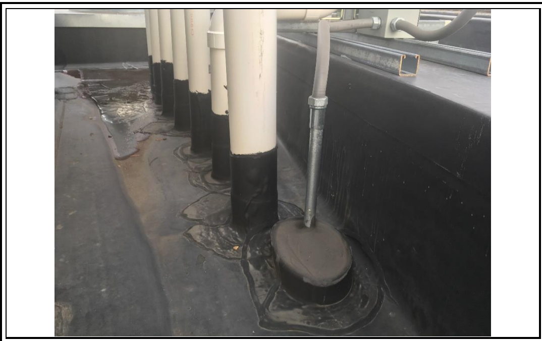
Photo 8: Riser pipes for individual subsystems extending through the roof at 144 State Street (12/05/18)
