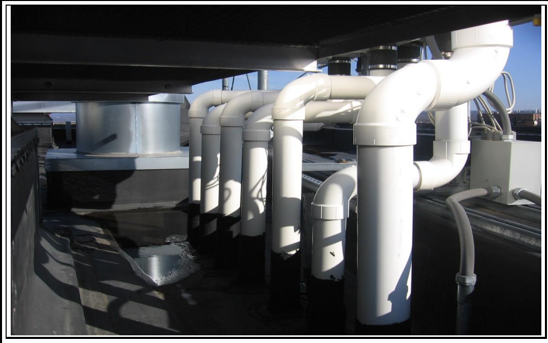
Photo 9: Riser pipes extending through roof and into fan units (12/3/20).
