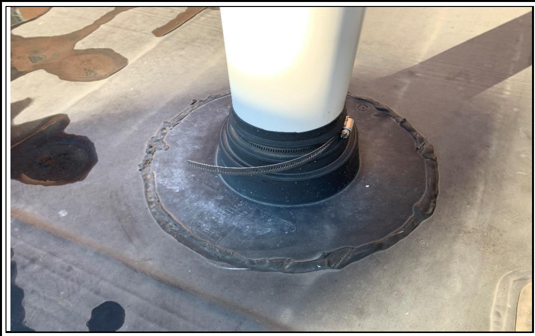
Photo 22: Close-up view of roof penetration/seal for SSDS exhaust stack at 140 State Street (12/3/20).
