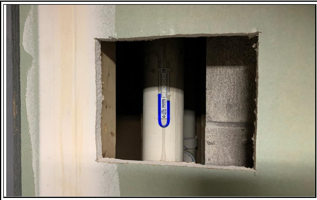
Photo 24: View of manometer and vertical riser pipe for SSDS at 140 State Street (access via basement level) (12/3/20).
