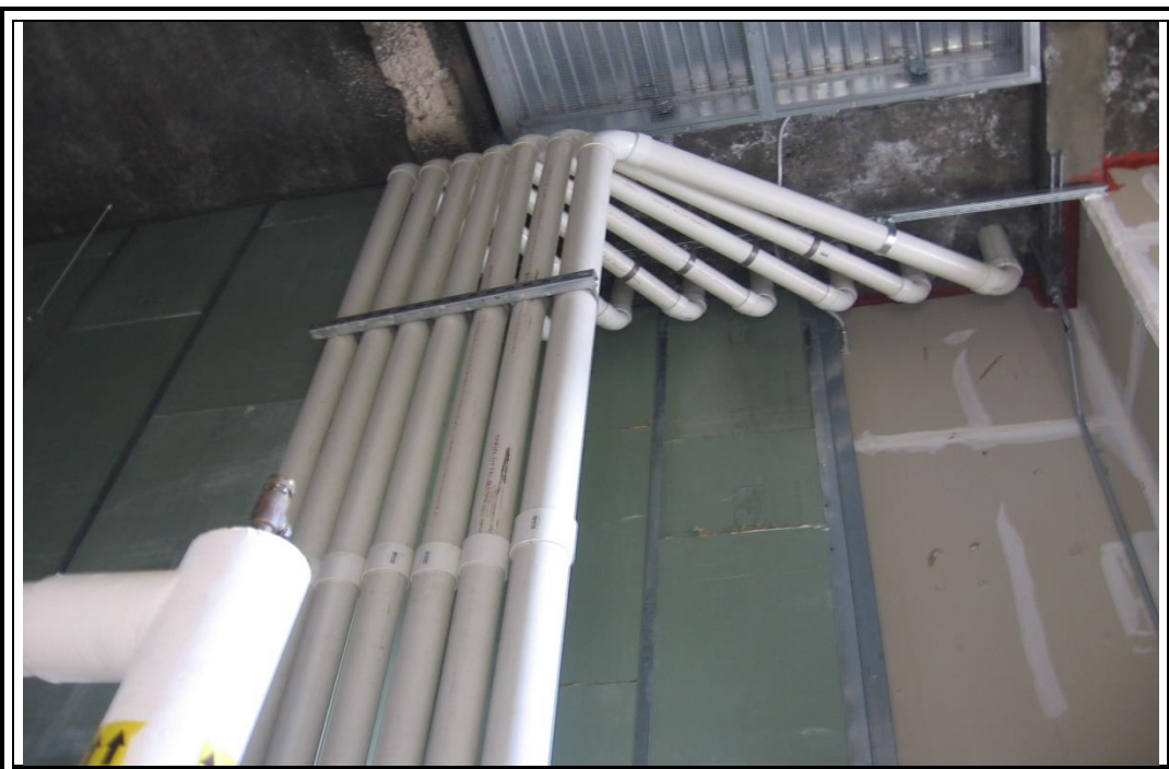
Photo 4: Riser piping for individual subsystems extending to/through the building roof (12/3/20).
