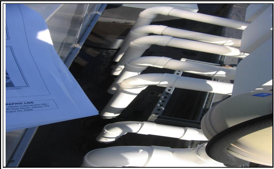
Photo 10: Riser pipes extending through roof and into fan units 12/3/20).
