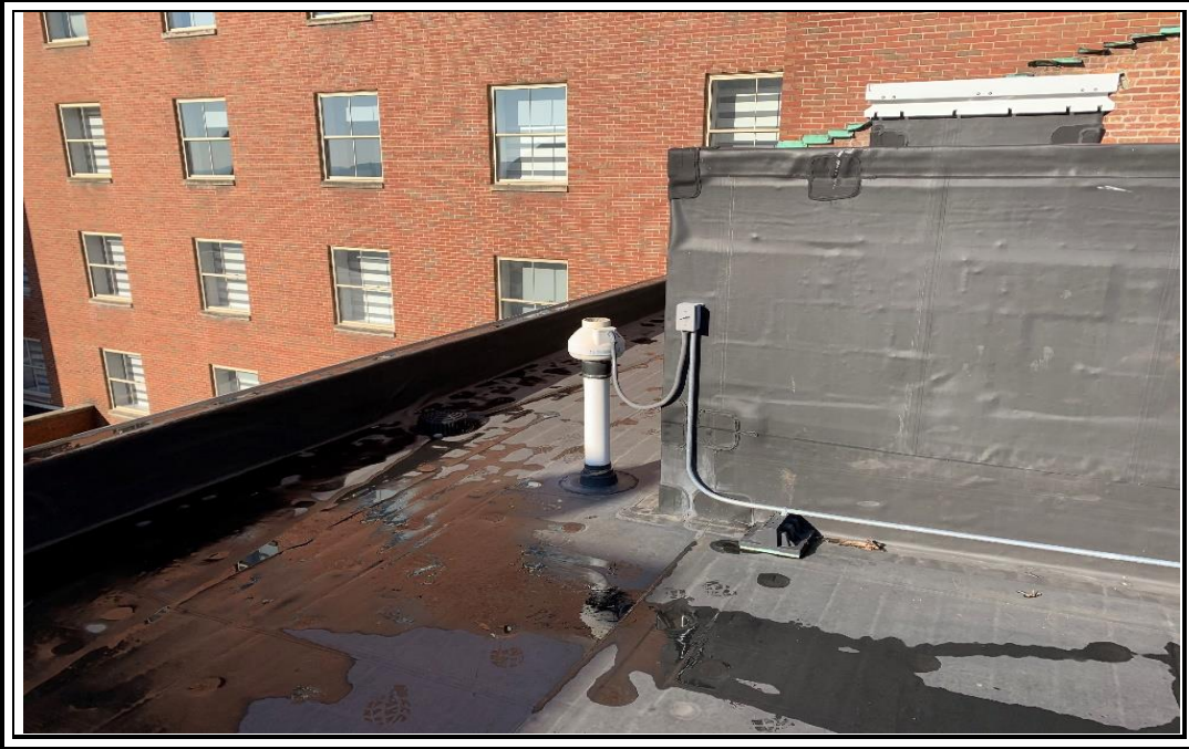
Photo 21: Roof of 140 State Street building; exhaust stack, fan and switch for SSDS (12/3/20).
