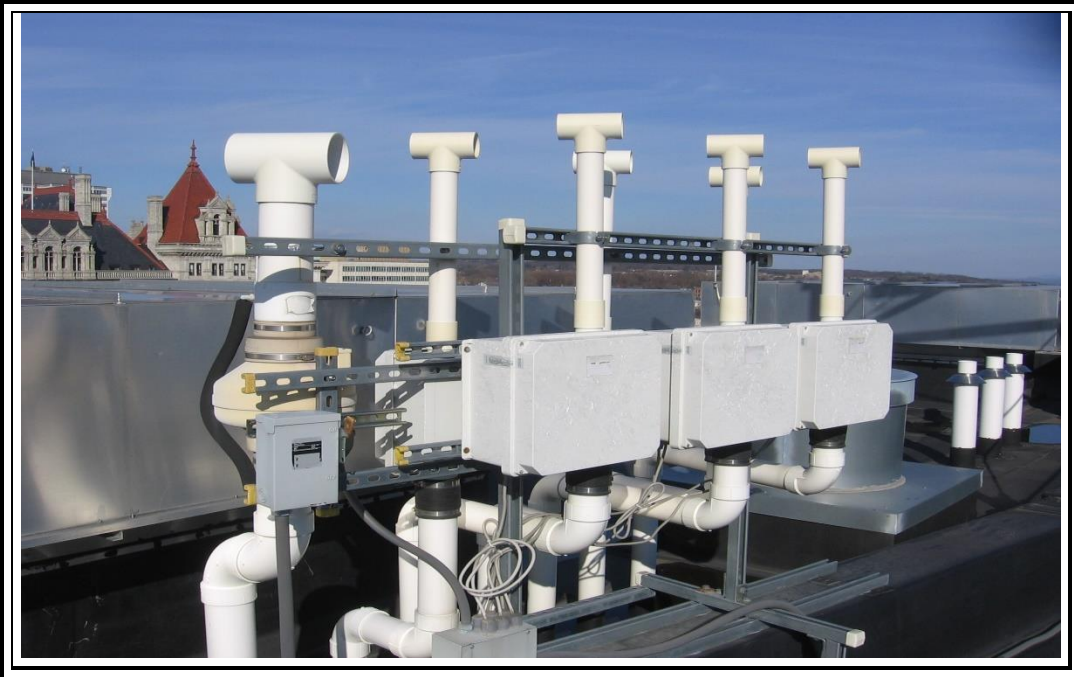
Photo 7: Roof-mounted fan units for individual subsystems at 144 State Street (12/3/20).
