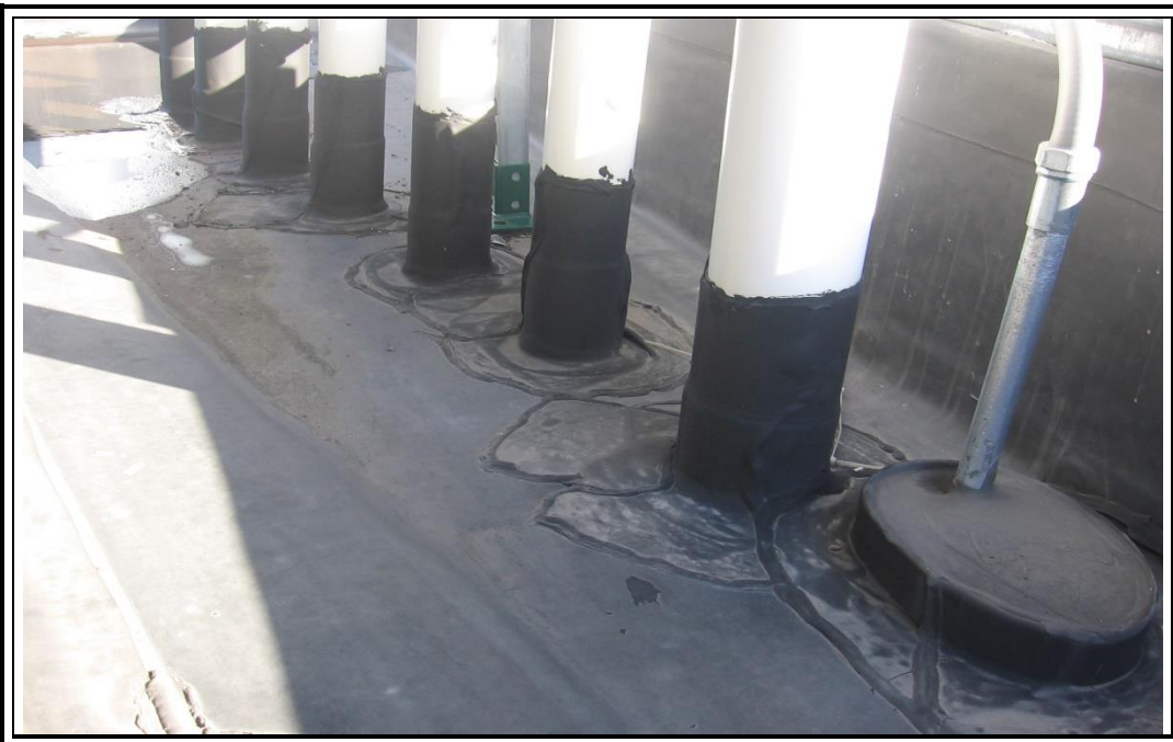
Photo 11: Seals around riser pipes at roof penetrations (12/3/20).
