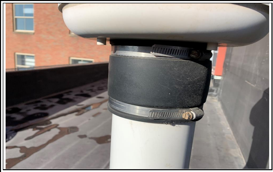
Photo 23: Close-up view of connection between SSDS exhaust stack and fan at 140 State Street (12/3/20).
