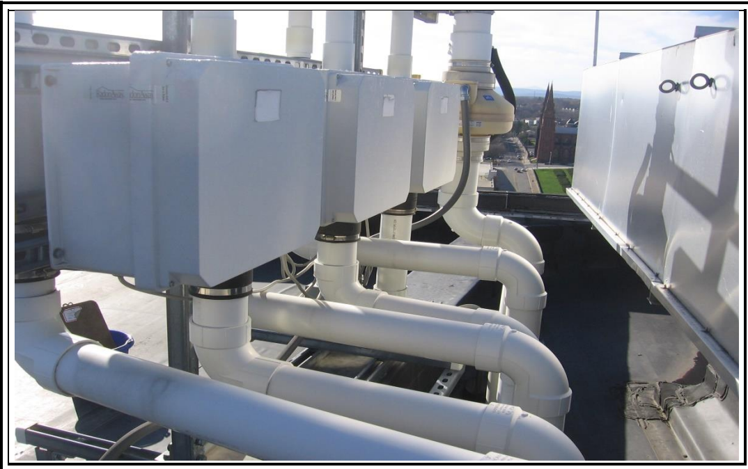
Photo 8: Fan units for subsystems 2, 5, 7 and 3 (left to right); labels worn, require replacement (12/3/20).
