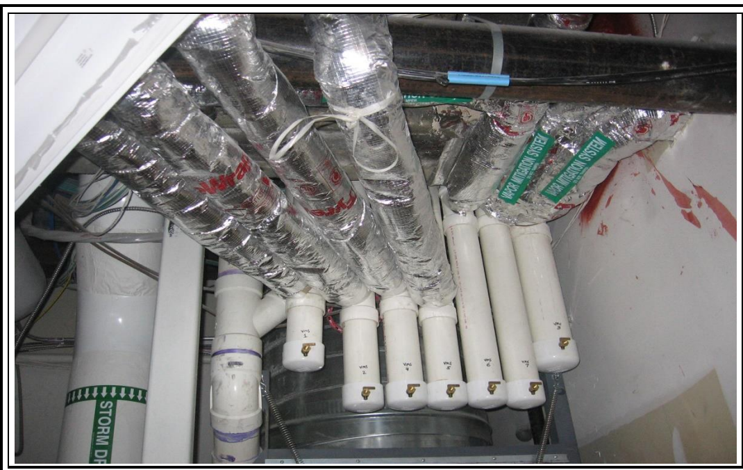
Photo 12: Inside laundry chute room in basement of 144 State Street; horizontal piping for individual subsystems connected to vertical riser pipes (12/3/20).
