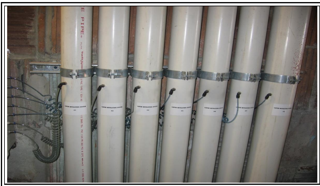
Photo 2: Close-up view of riser piping for individual subsystems and tubing associated with the mannehelic manometers (12/3/20).
