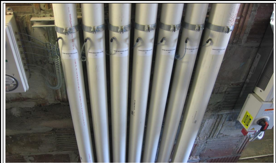
Photo 3: Riser piping for individual subsystems (12/3/20).
