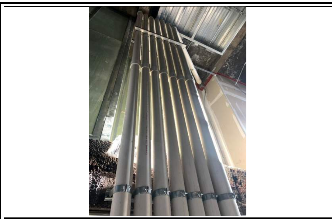
Photo 4: Riser piping for individual subsystems extending to the building roof at 144 State Street (12/14/22).
