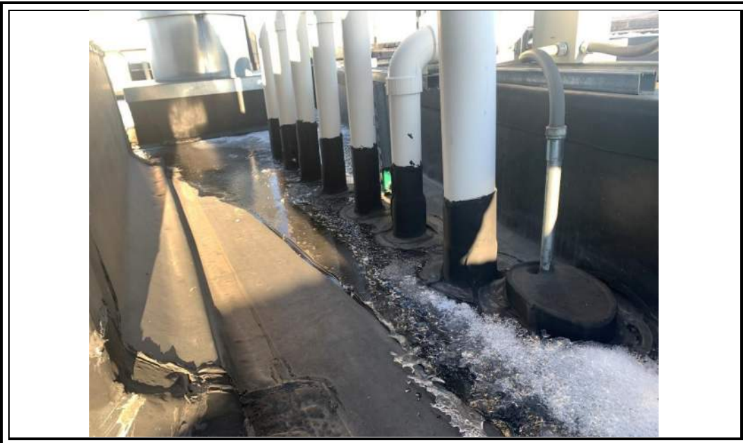
Photo 10: Seals around riser pipes at roof penetrations 12/14/22).
