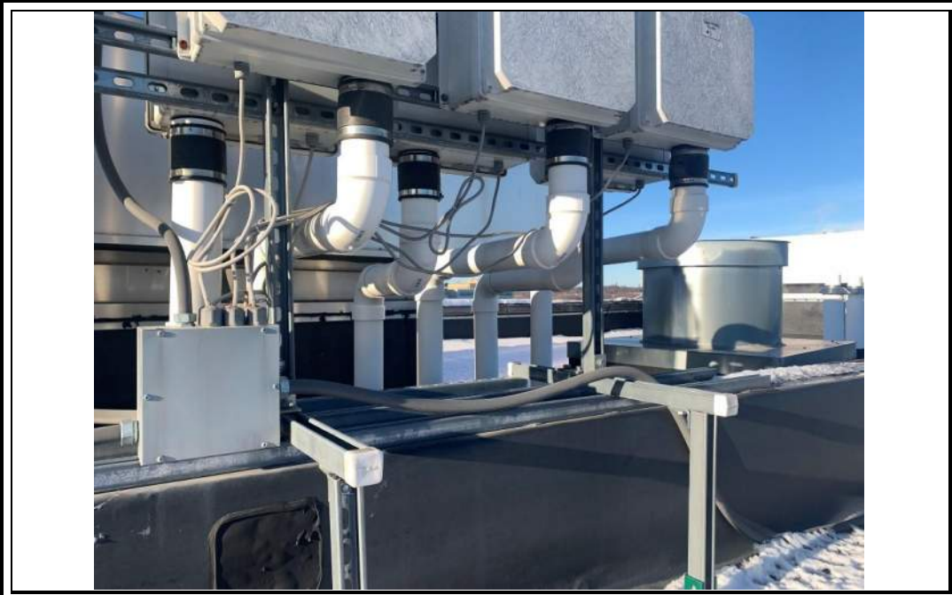
Photo 7: Roof-mounted fan units for individual subsystems at 144 State Street (12/14/22).
