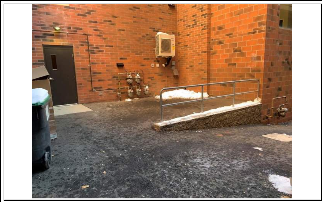
Photo 15: Looking east; paved surface cover in area adjacent to rear side of 140 State Street building (12/14/22).
