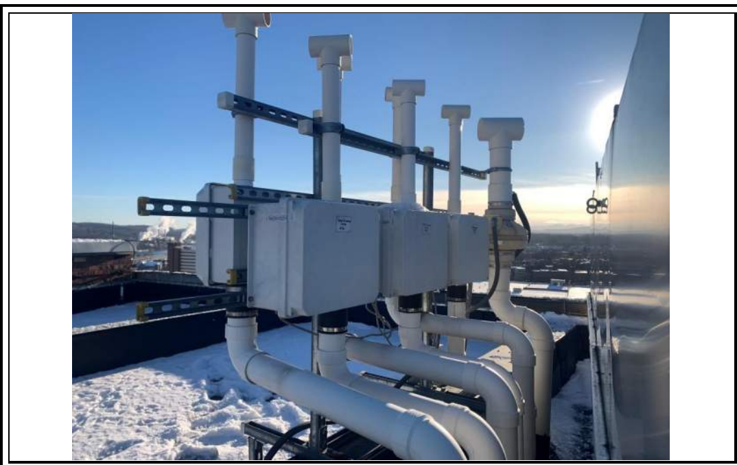
Photo 8: Fan units for subsystems 2, 5, 7 and 3 (left to right) at 144 State Street (12/14/22).
