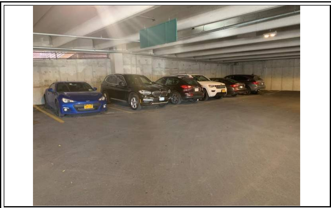
Photo 20: Looking north; paved surface cover within lowest level of the parking garage (12/14/22).
