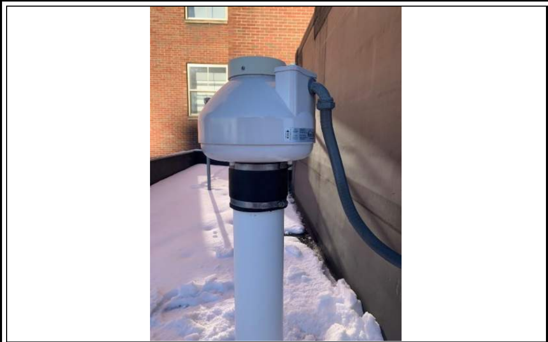
Photo 23: Close-up view of connection between SSDS exhaust stack and fan at 140 State Street (12/14/22).
