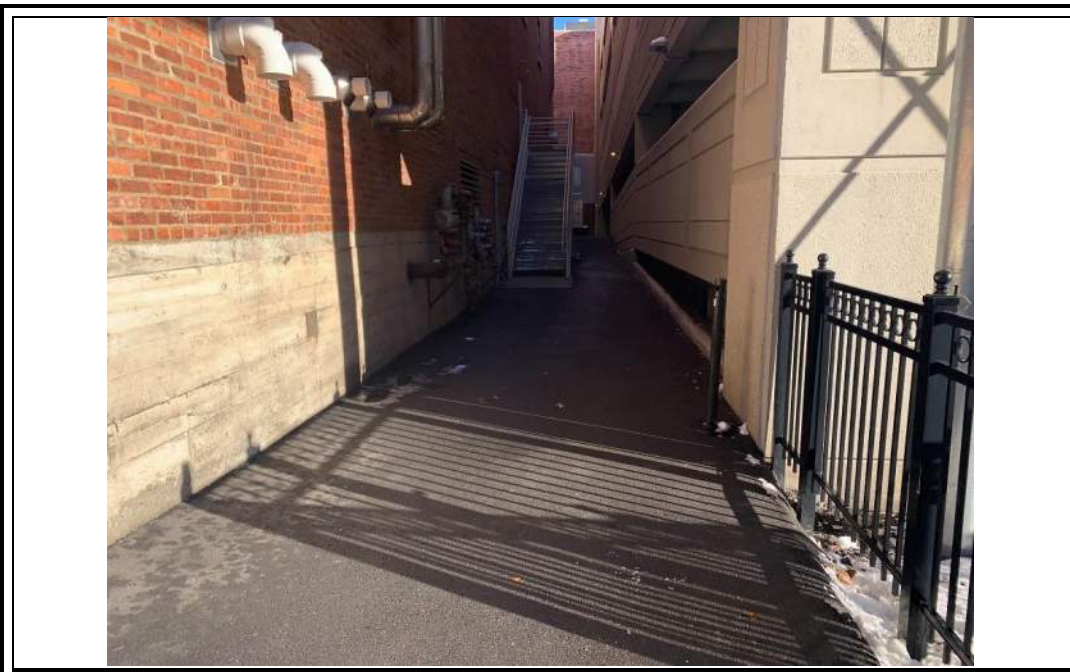
Photo 12: Looking northeast (from Howard Street); paved surface cover in alley between 144 State Street (to the left) and parking garage (to the right) (12/14/22).
