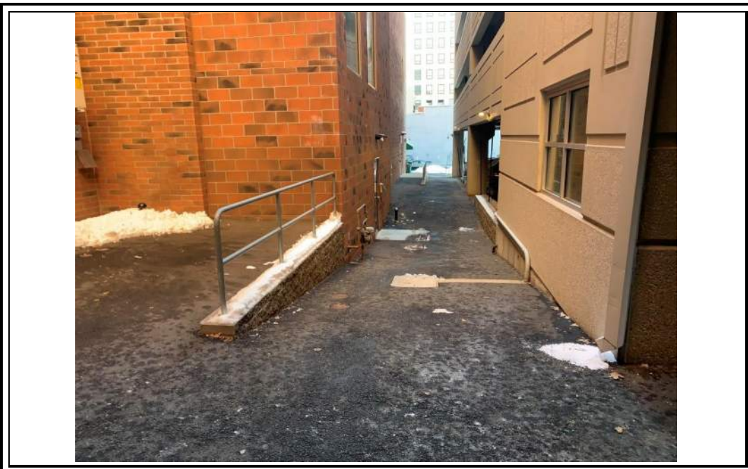
Photo 16: : Looking southeast; paved surface cover between 140 State Street (to the left) and the parking garage (to the right) (12/14/22).
