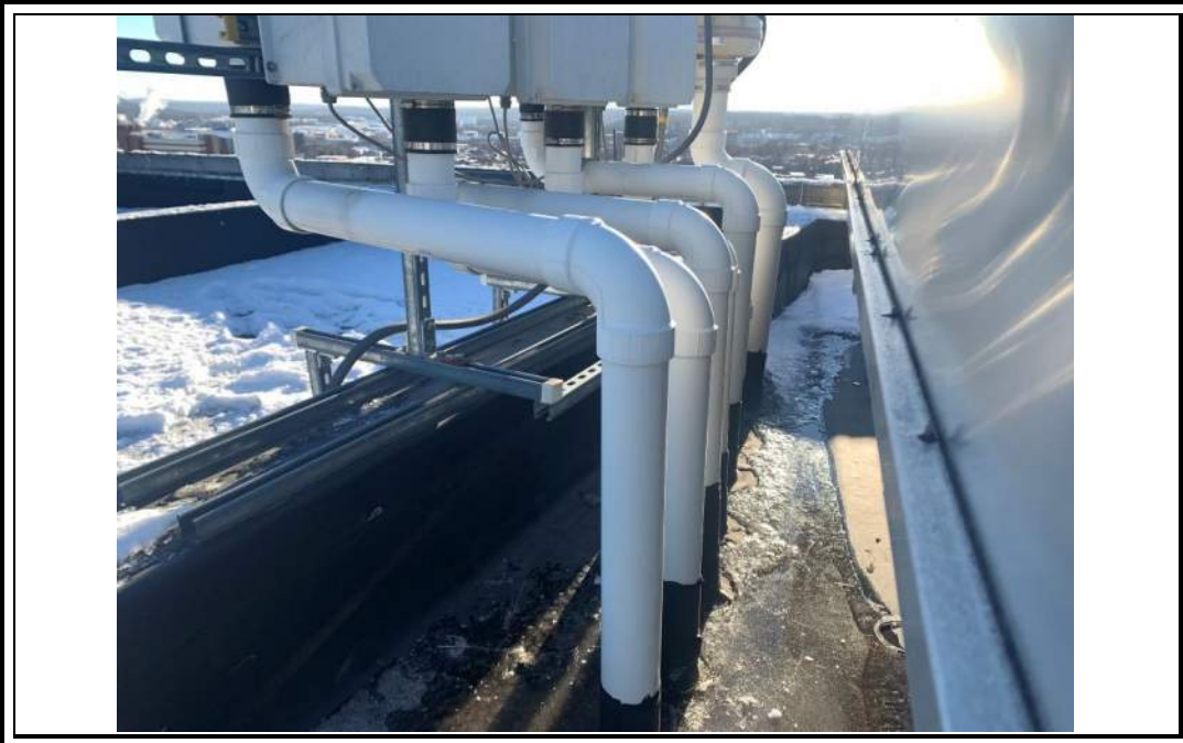
Photo 9: Riser pipes extending through roof and into fan units at 144 State Street (12/14/22).
