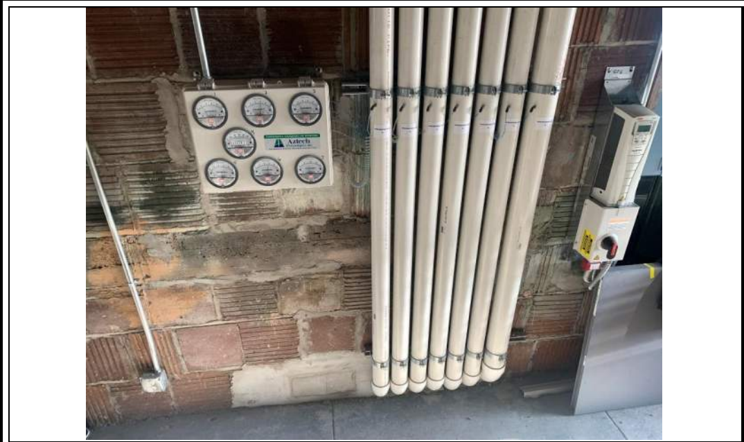
Photo 1: Magnehelic manometer panel and riser piping for the seven individual subsystems comprising the sub-slab depressurization system at 144 State Street (12/14/22).
