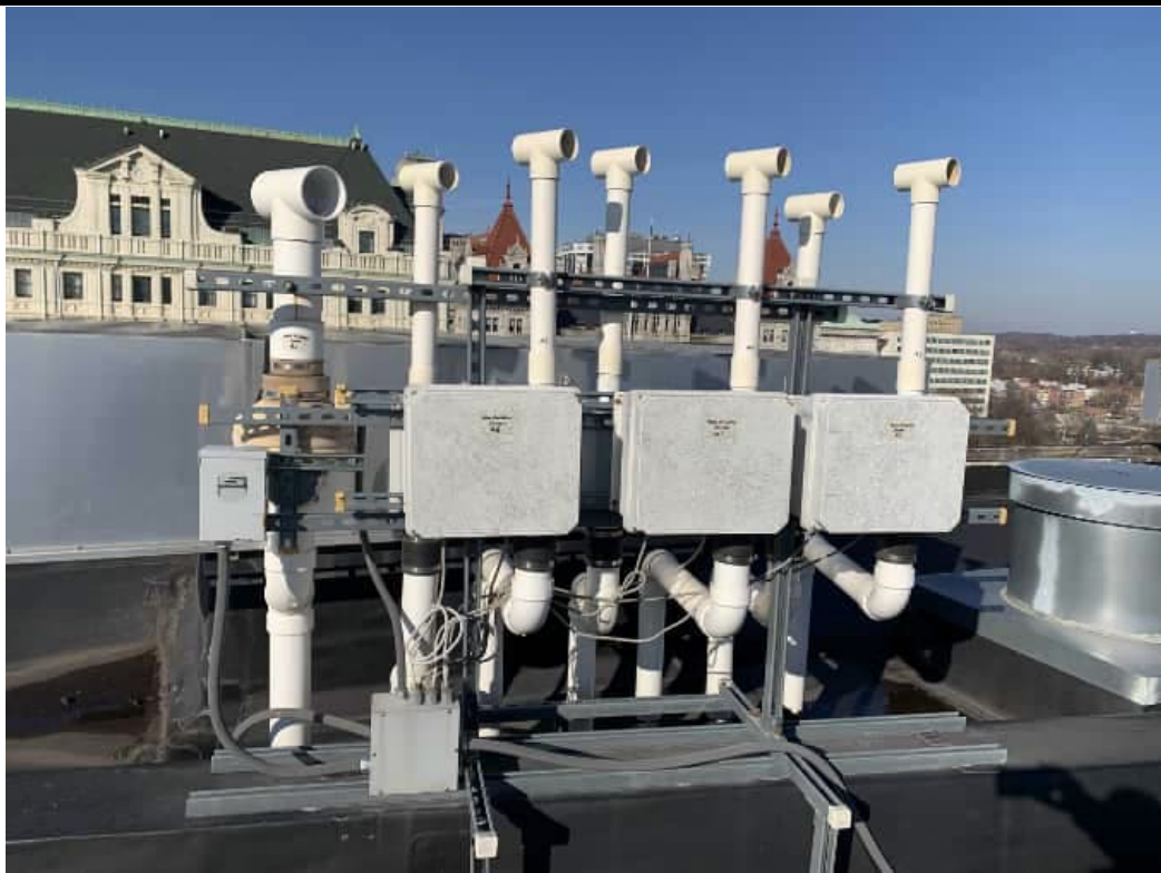
Photograph 5. Roof-mounted fan units for individual sub-systems at 144 State Street (12/15/23).
