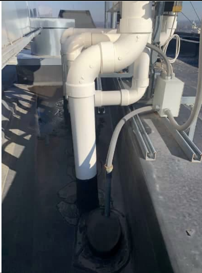
Photograph 7. Riser pipes extending through roof and into fan units at 144 State Street (12/15/23).
