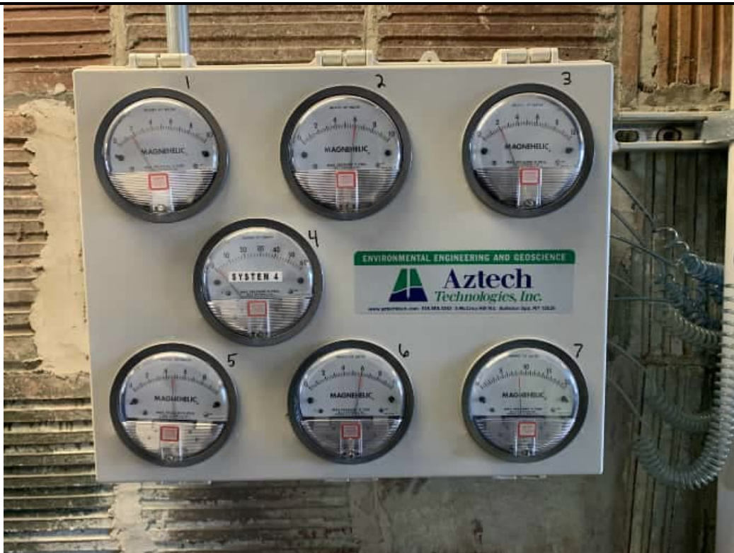
Photograph 2. Close-up view of manometer panel for individual subsystems and tubing associated with the magnehelic manometers (12/15/23).
