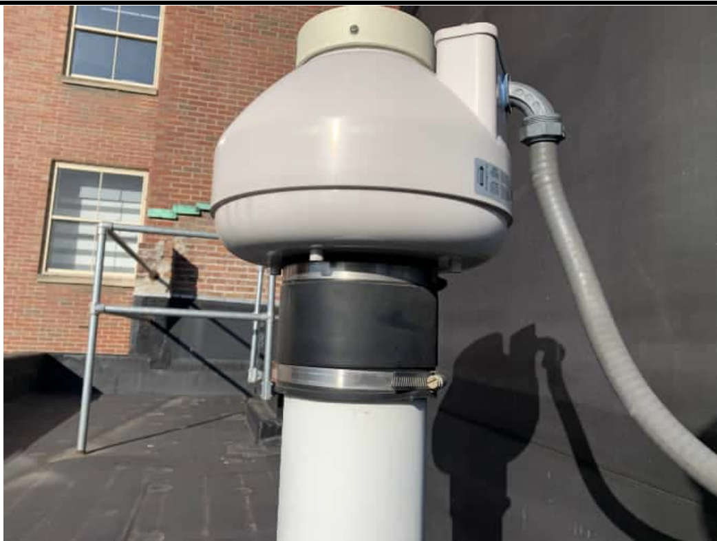
Photograph 19. Close-up view of connection between SSDS exhaust stack and fan at 140 State Street (12/15/23).
