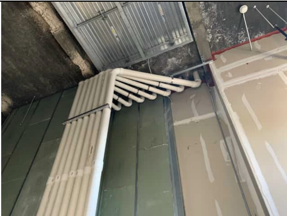
Photograph 4. Riser piping for individual subsystems extending through the building roof at 144 State Street (12/15/23).
