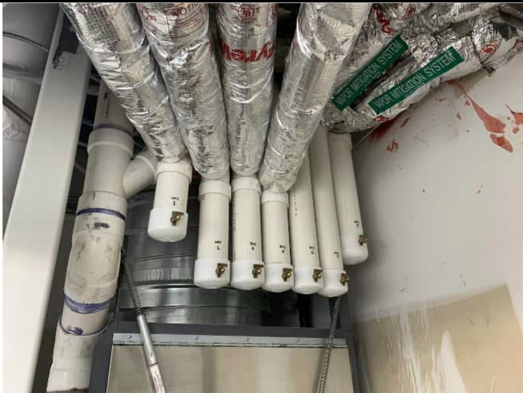
Photograph 9. Inside laundry chute room in basement of 144 State Street; horizontal piping for individual sub-systems connected to vertical riser pipes (12/15/23).
