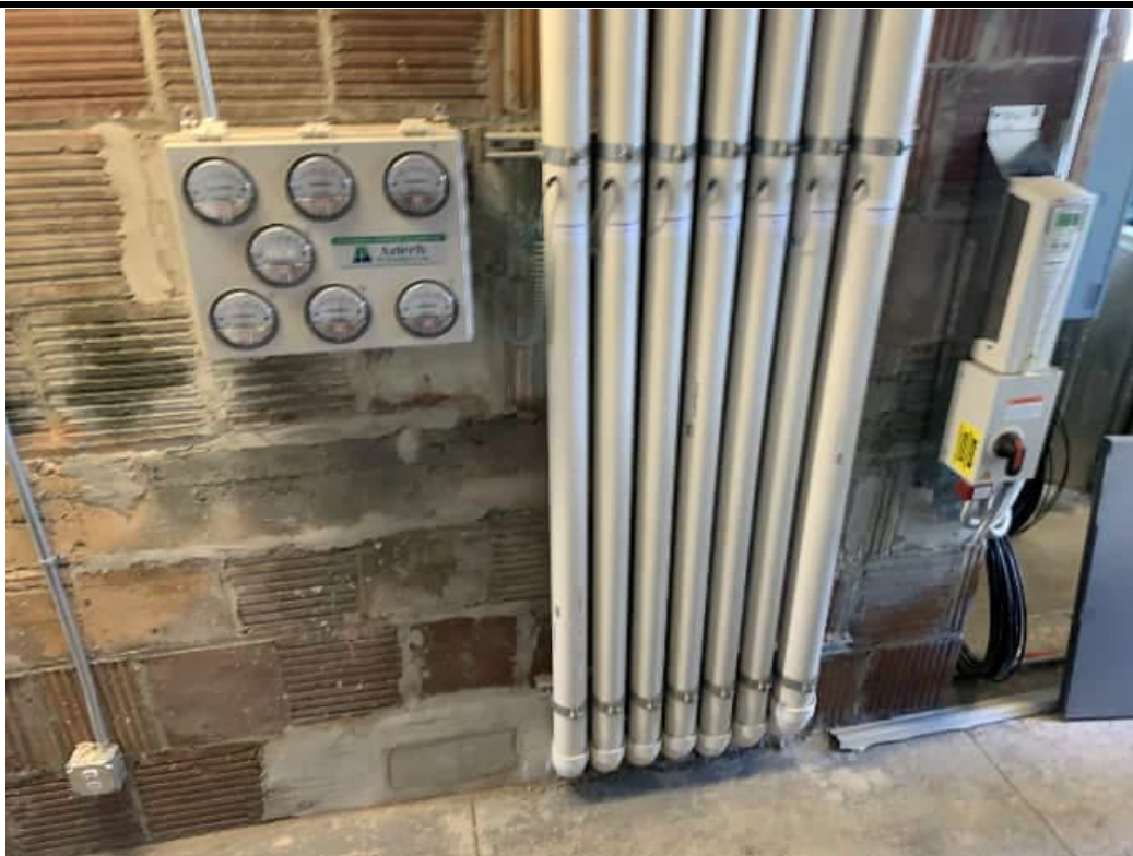
Photograph 1. Magnehelic manometer panel and riser piping for the seven individual subsystems comprising the sub-slab depressurization system at 144 State Street (12/15/23).
