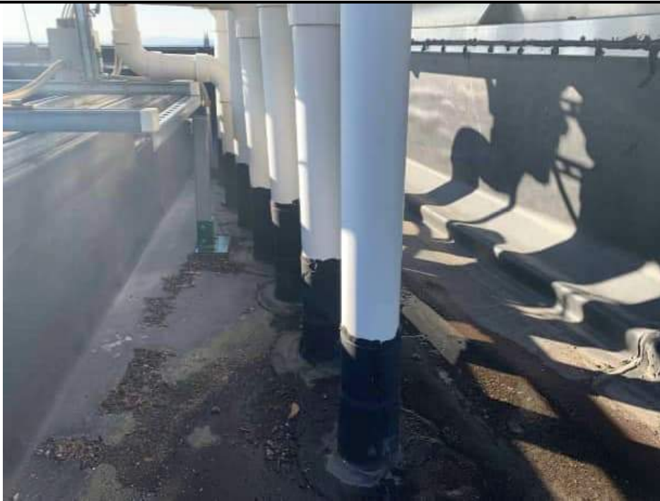
Photograph 8. Seals around riser pipes at roof penetrations (12/15/23).
