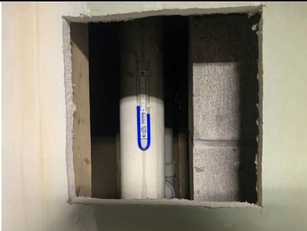
Photograph 21. View of manometer and vertical riser pipe for SSDS at 140 State Street (access via basement level) (12/15/23).
