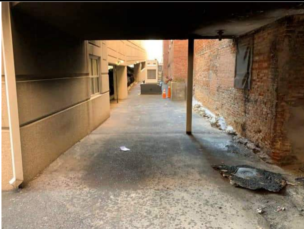
Photograph 13. Looking southwest toward Howard Street; paved surface cover in alley between 144 State Street and the parking garage (12/15/23). Staining was observed on the exterior walls due to a manmade fire. No other damage to the building or pavement was noted.
