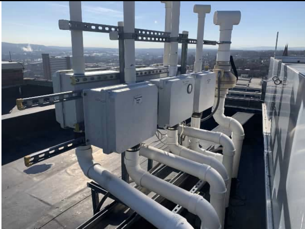
Photograph 6. Fan units for subsystems 2, 5, 7 and 3 (left to right) at 144 State Street (12/15/23).
