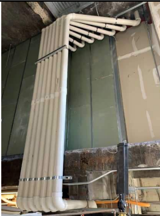
Photograph 3. Riser piping for individual subsystems at 144 State Street (12/15/23).
