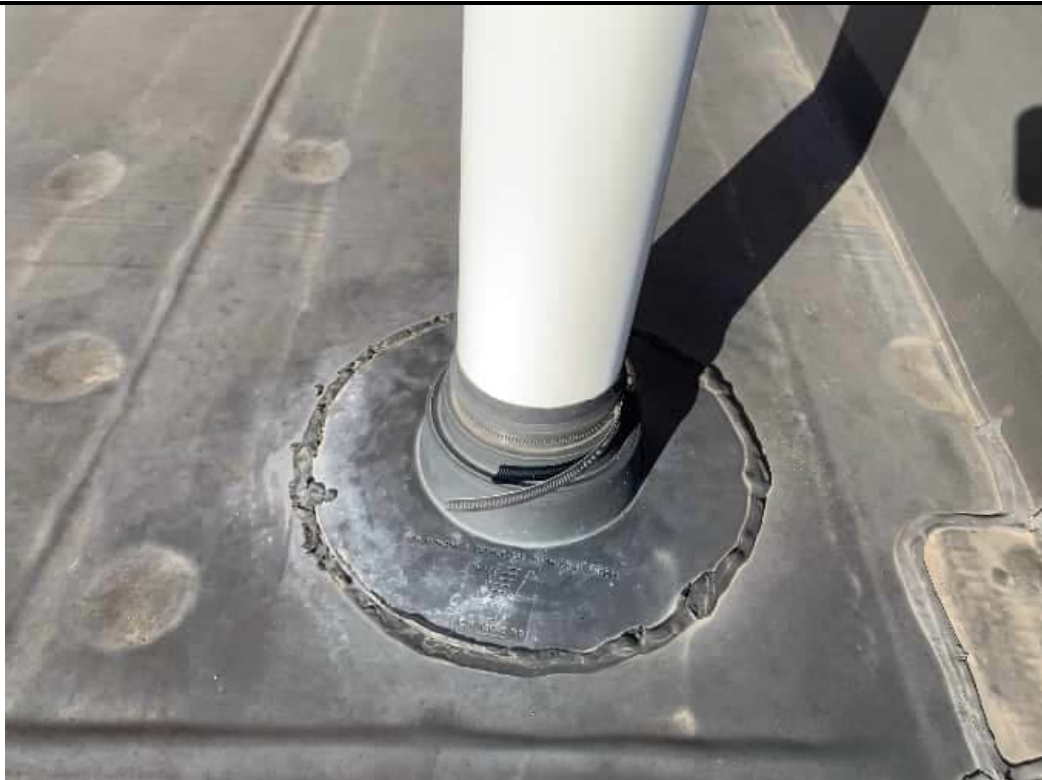
Photograph 20. Close-up view of roof penetration/seal for SSDS exhaust stack at 140 State Street (12/15/23).
