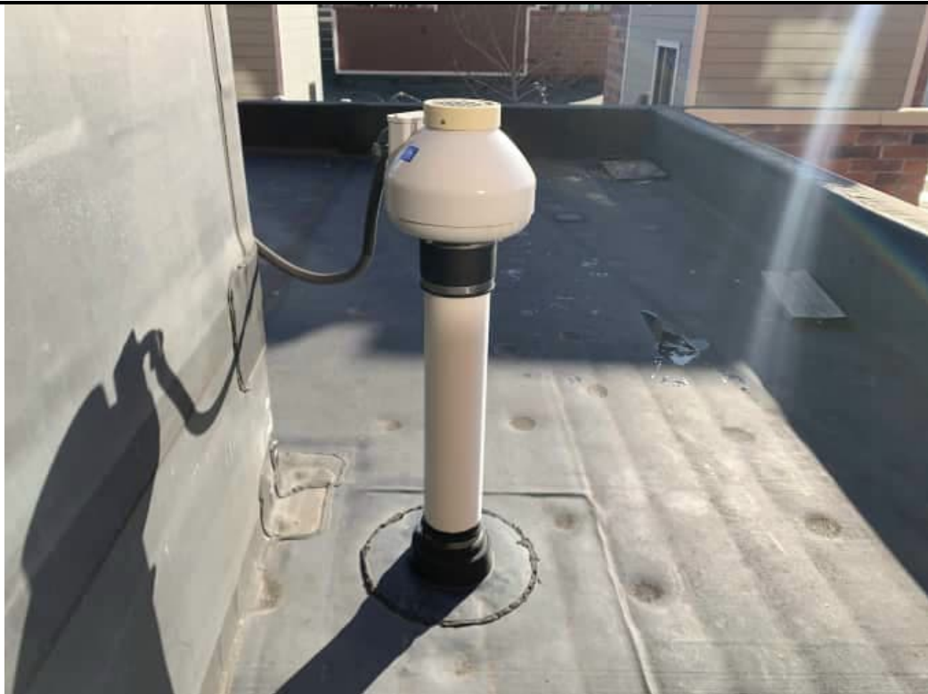
Photograph 18. Roof of 140 State Street building; exhaust stack, fan and switch for SSDS (12/15/23).
