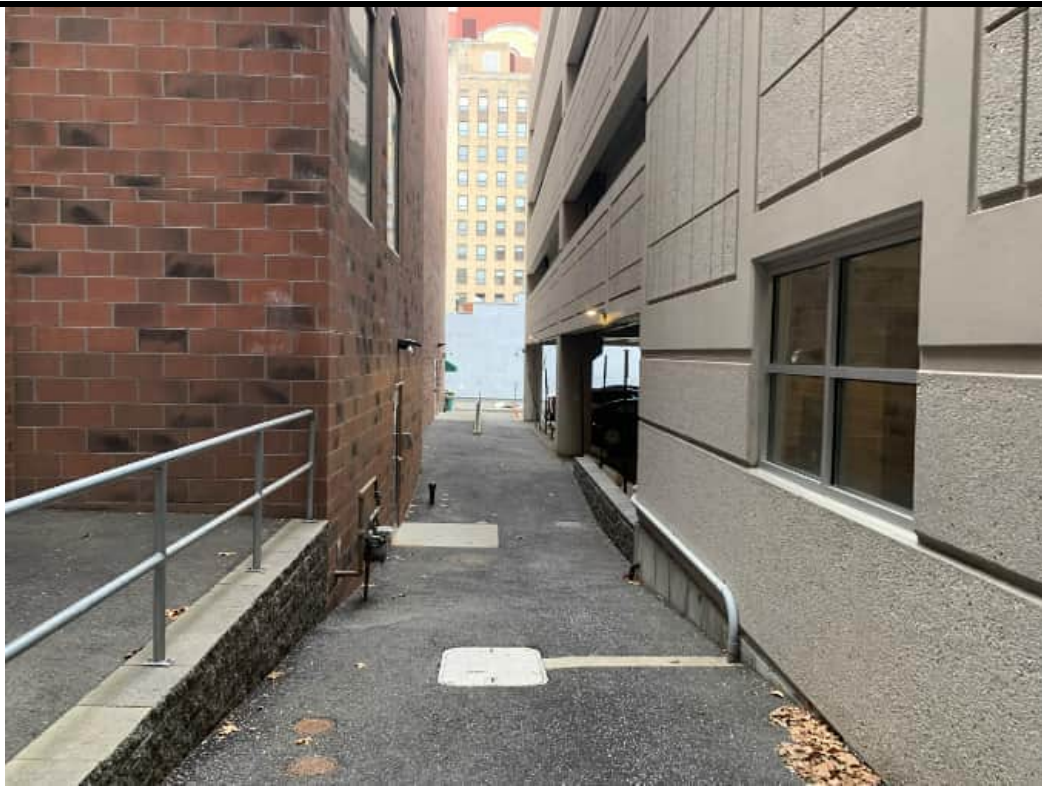
Photograph 11. Looking southeast; paved surface cover between 140 State Street (to the left) and the parking garage (to the right) (12/20/24).
