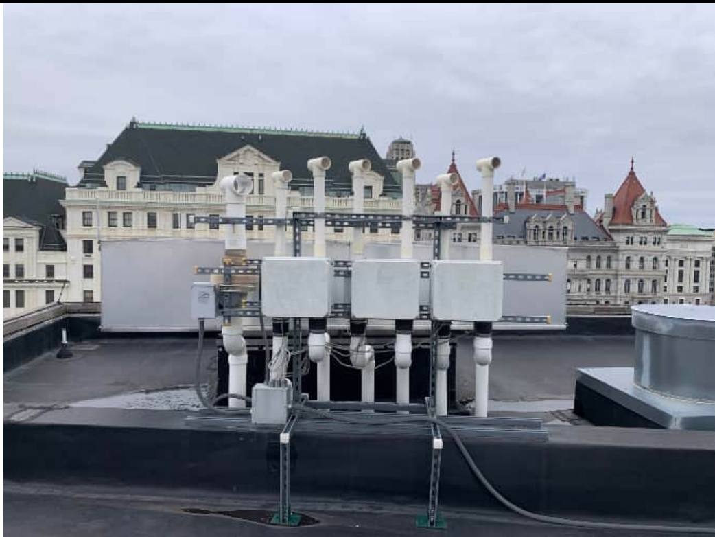
Photograph 5. Roof-mounted fan units for individual sub-systems at 144 State Street (12/20/24).
