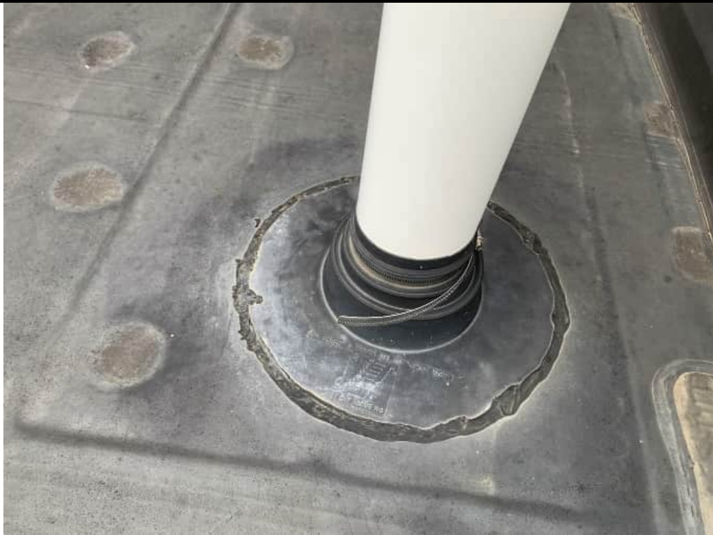
Photograph 18. Close-up view of roof penetration/seal for SSDS exhaust stack at 140 State Street (12/20/24).
