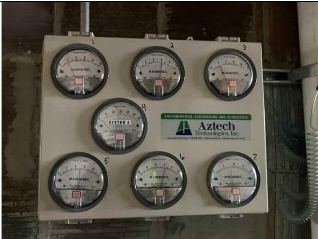
Photograph 2. Close-up view of manometer panel for individual subsystems and tubing associated with the magnehelic manometers (12/20/24).
