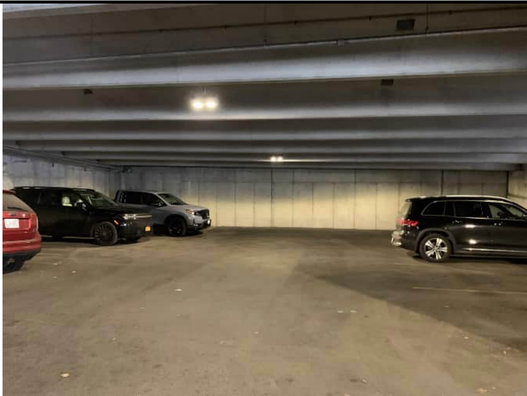
Photograph 15. Looking north; paved surface cover within lowest level of the parking garage (12/20/24).
