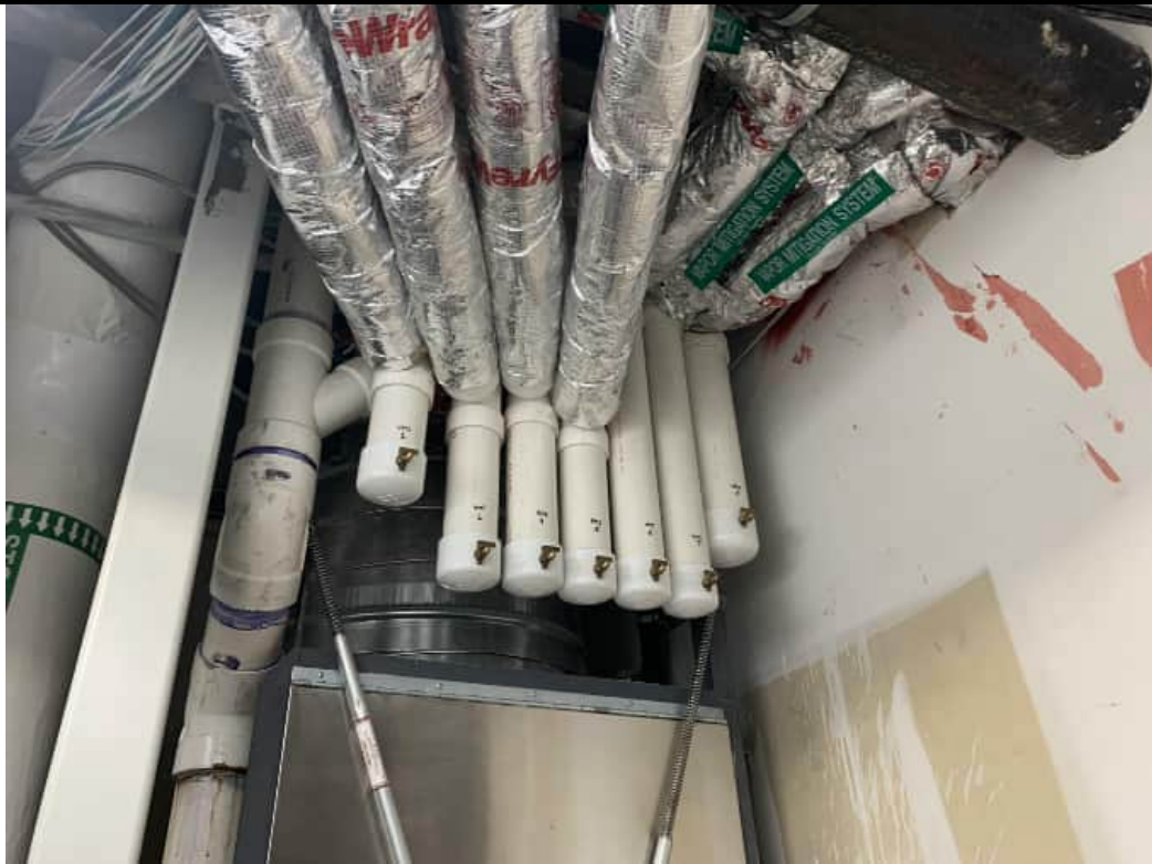
Photograph 8. Inside laundry chute room in basement of 144 State Street; horizontal piping for individual sub-systems connected to vertical riser pipes (12/20/24).
