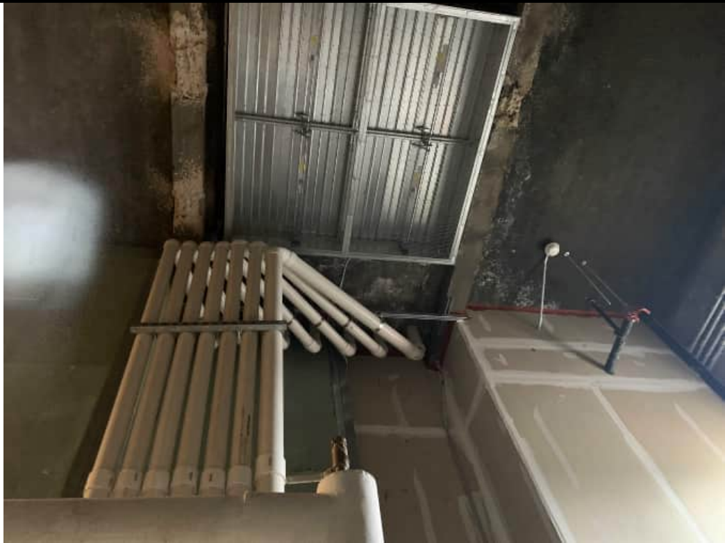
Photograph 4. Riser piping for individual subsystems extending through the building roof at 144 State Street (12/20/24).
