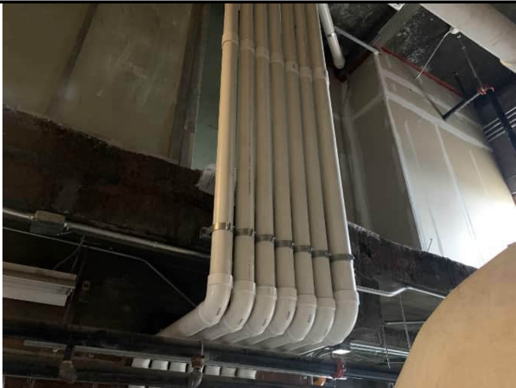
Photograph 3. Riser piping for individual subsystems at 144 State Street (12/20/24).
