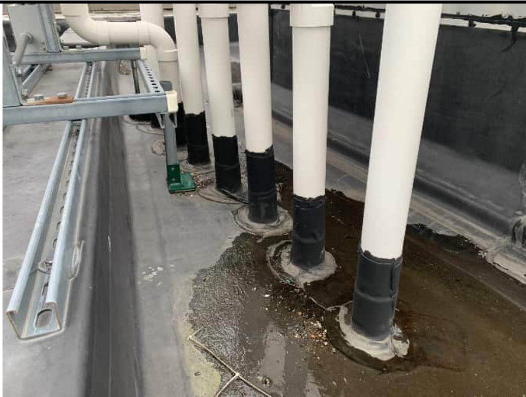
Photograph 7. Seals around riser pipes at roof penetrations (12/20/24).
