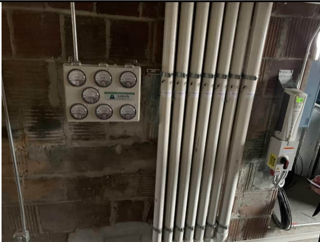
Photograph 1. Magnehelic manometer panel and riser piping for the seven individual subsystems comprising the sub-slab depressurization system at 144 State Street (12/20/24).
