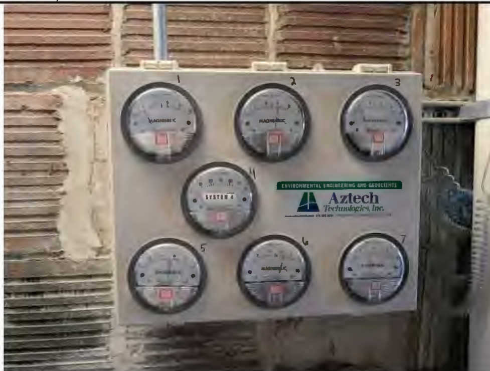
Photograph 2. Close-up view of manometer panel for individual subsystems and tubing associated with the magnehelic manometers (4/13/2026).
