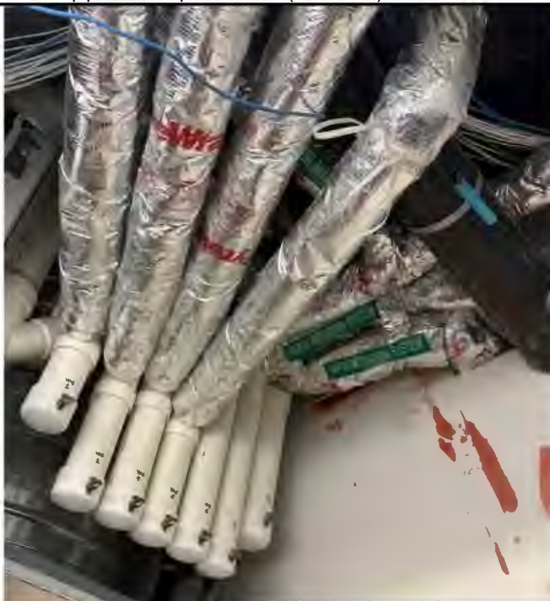
Photograph 6. Inside laundry chute room in basement of 144 State Street; horizontal piping for individual sub-systems connected to vertical riser pipes (4/13/2026).
