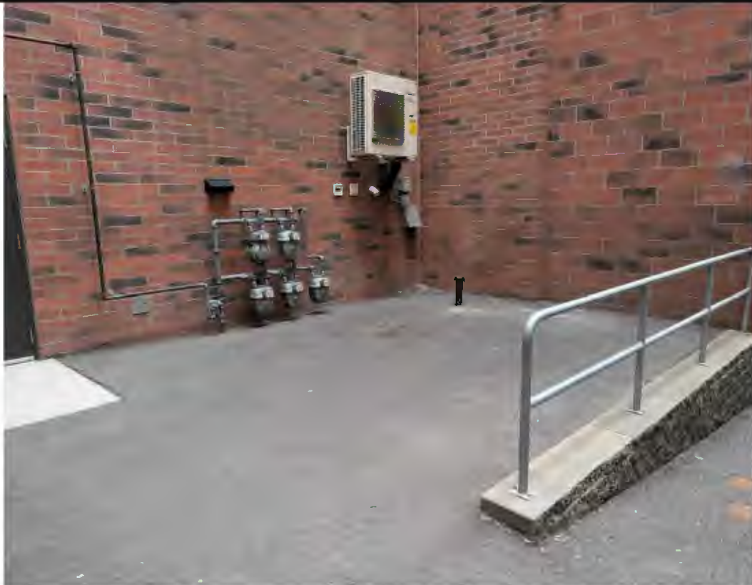
Photograph 8. Looking east; paved surface cover in area adjacent to rear side of 140 State Street building (4/13/26).
