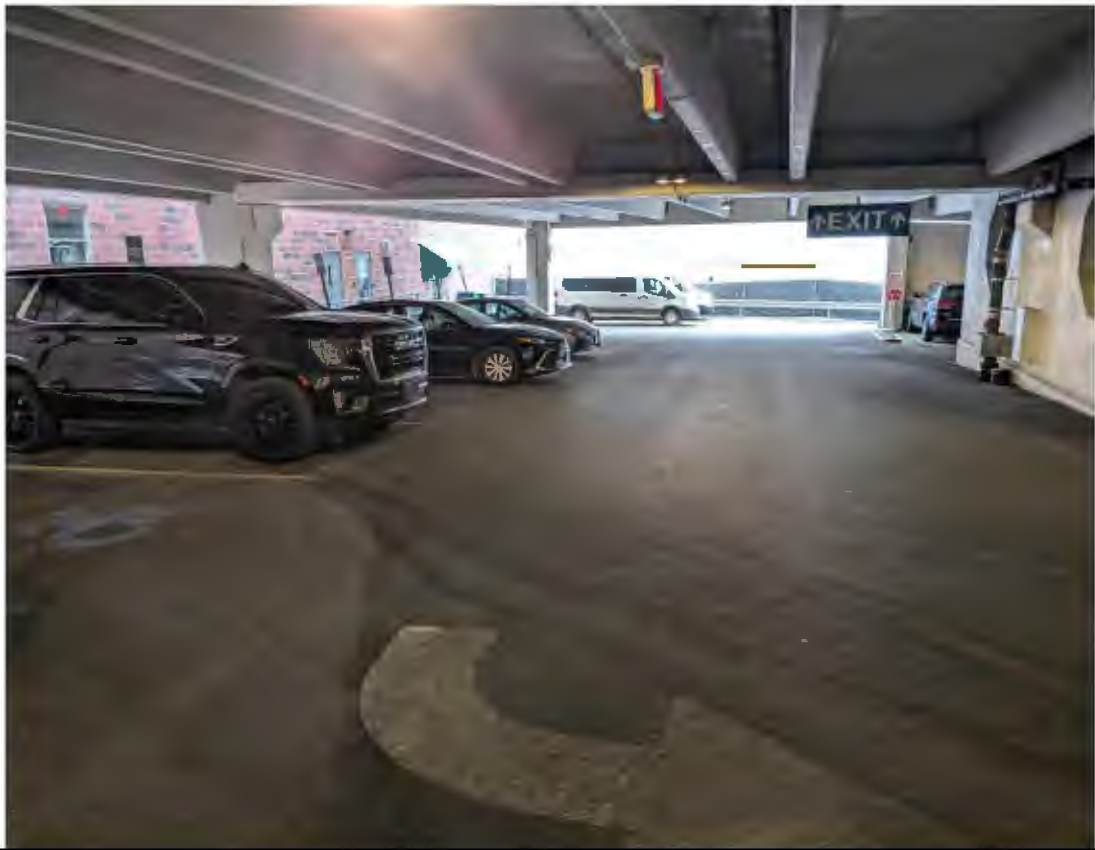
Photograph 11. Looking southeast toward Howard Street; paved surface cover within lowest level of parking garage (4/13/26).
