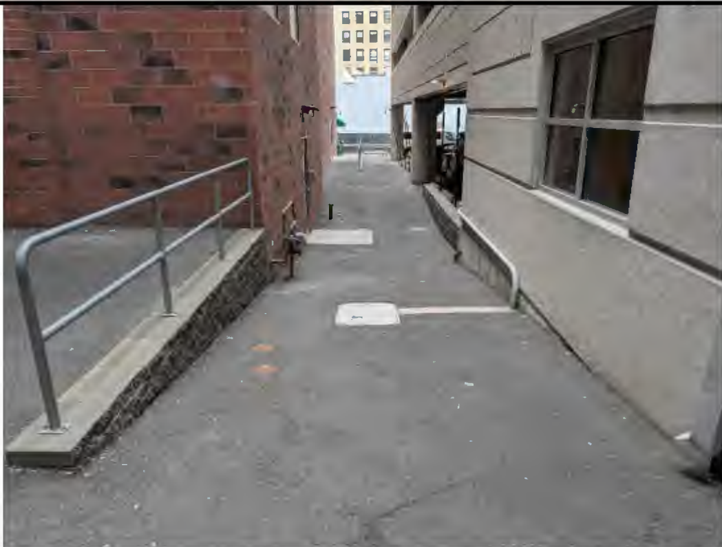
Photograph 9. Looking southeast; paved surface cover between 140 State Street (to the left) and the parking garage (to the right) (4/13/26).
