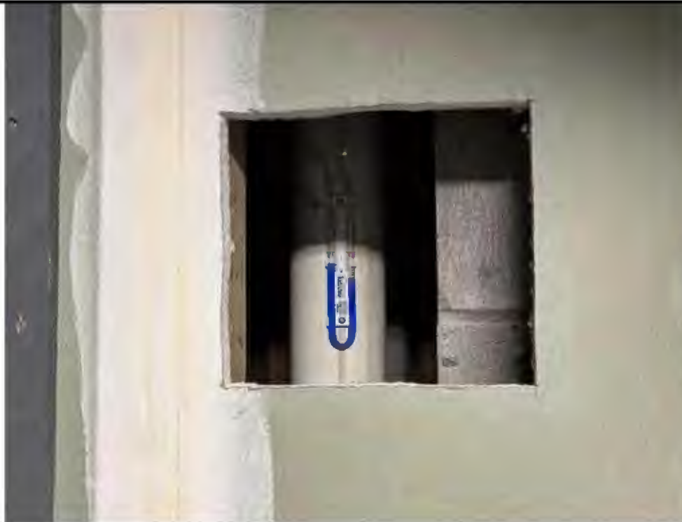
Photograph 14. View of manometer and vertical riser pipe for SSDS at 140 State Street (access via basement level) (4/13/26).
