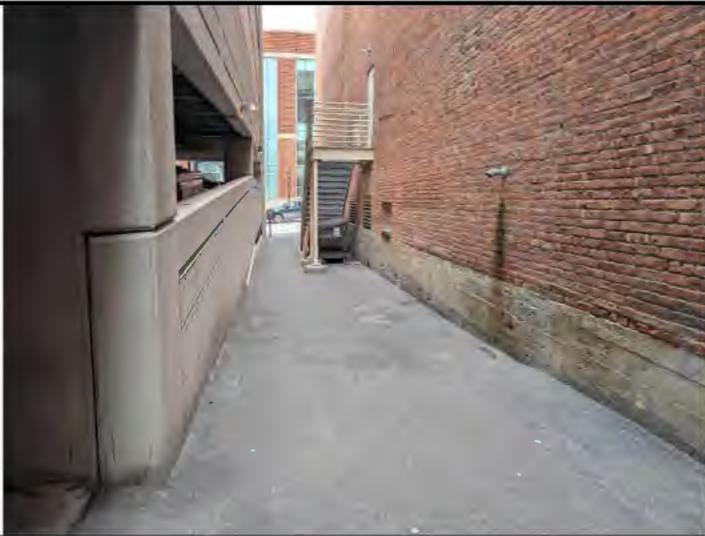
Photograph 7. Looking southwest; paved surface cover in alley between 144 State Street (to the right) and parking garage (to the left) (4/13/2026).
