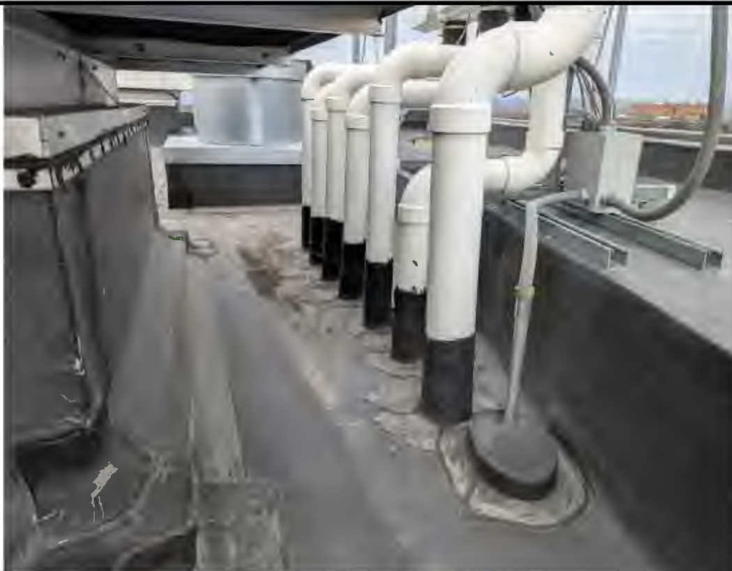
Photograph 5. Seals around riser pipes at roof penetrations (4/13/2026).
