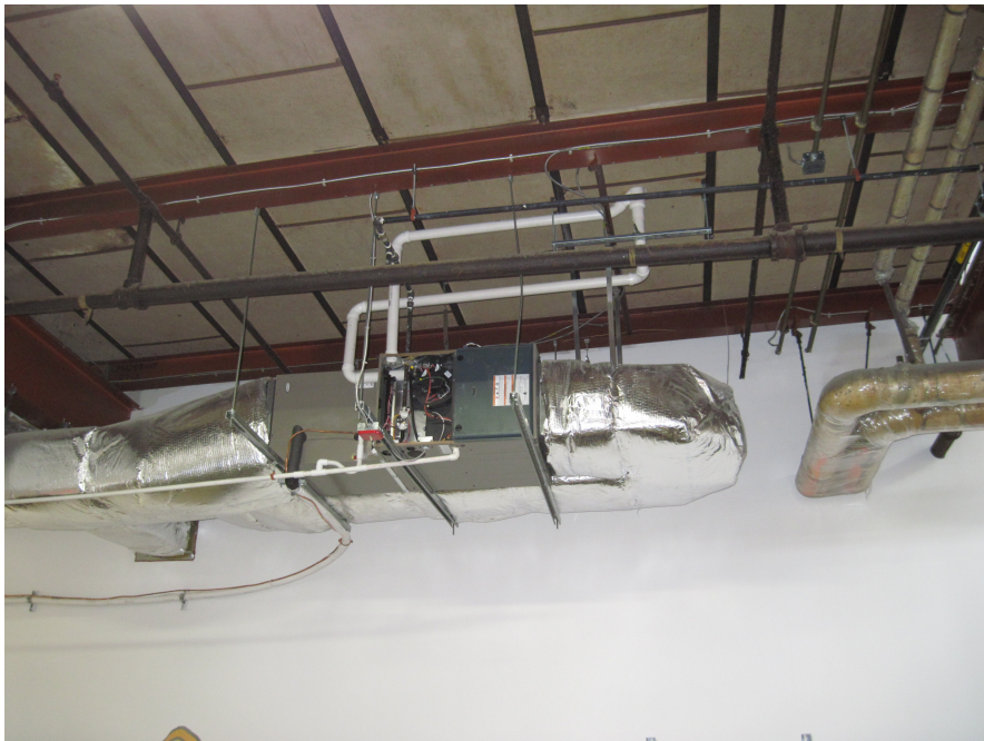
Ceiling ductwork in main hallway.
