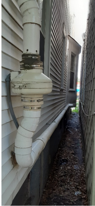
Photograph 6: Pump stack to top of house
