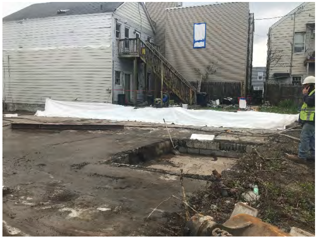
Ledge of exposed soil along west end of foundation covered with two layers of 6 mil poly
