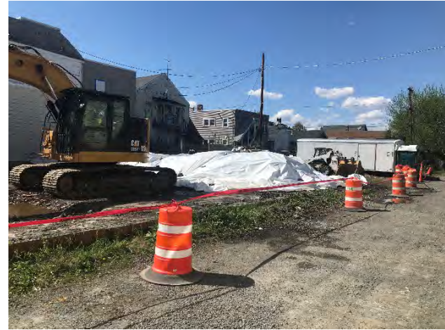
Remaining pile of demo debris covered in poly sheeting located at the north end of the slab.
