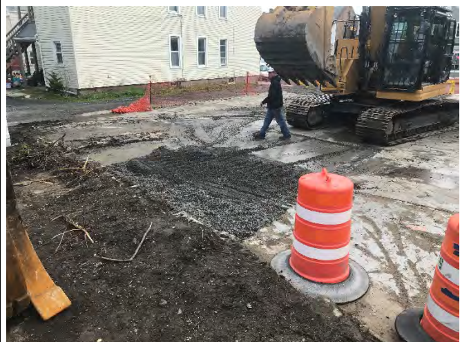
Recessed floor along north wall filled with crusher run (former boiler room)
