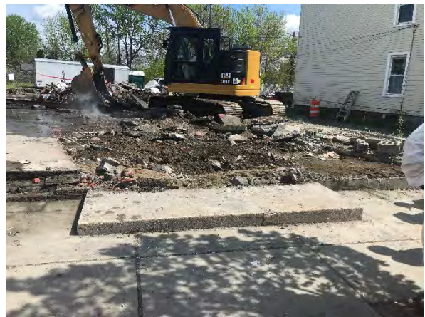
Southeast section of slab removed (approx. 250 sq ft)
