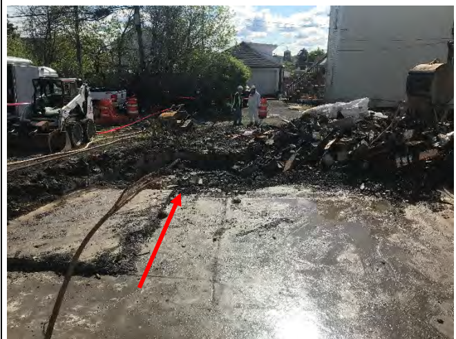
Recessed floor along north wall filled with debris (former boiler room)
