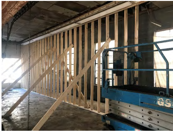
Completed support wall inside building (completed 5/4/20)
