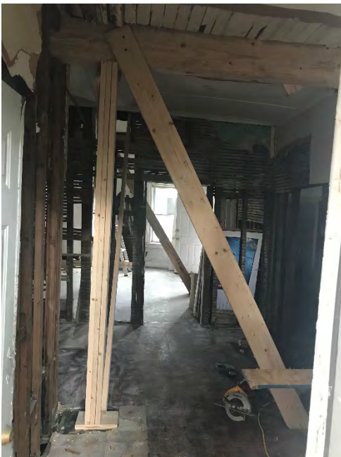
Shoring on first floor of 621 19 th St.
