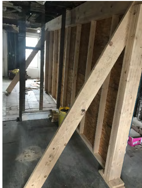
Shoring on second floor of 621 19 th St.
