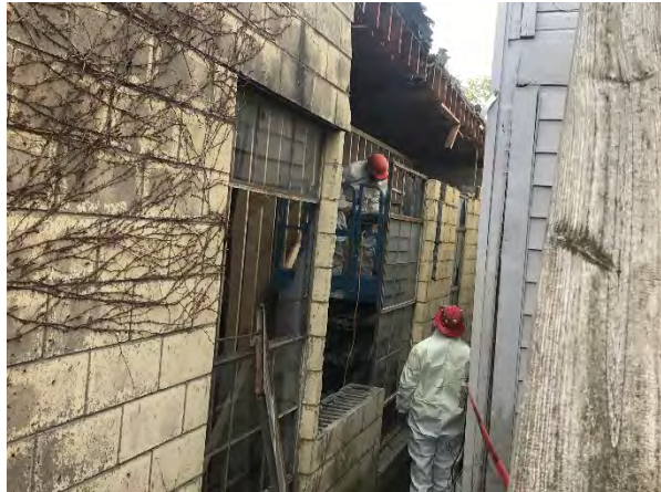
Removing windows on the west wall
