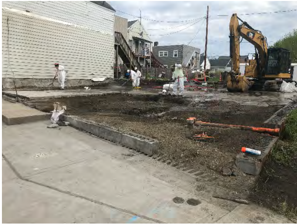
Jackson crew clearing remaining demo debris from slab and surrounding work area
