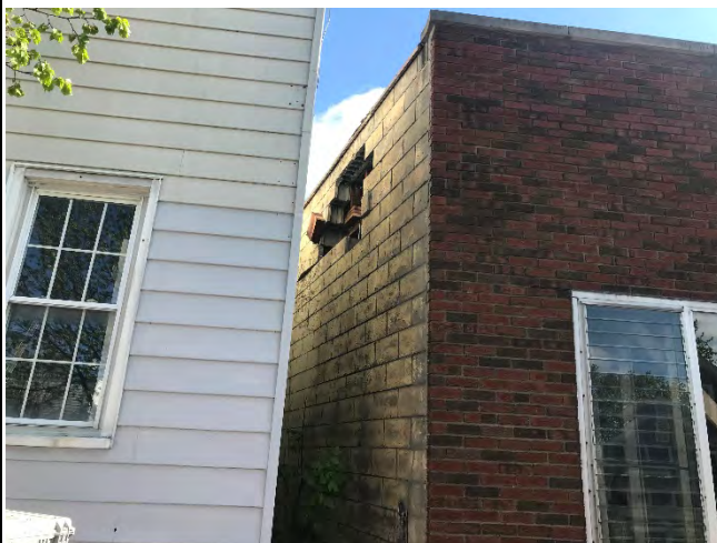
Hand demo started on the south west corner from the inside.
