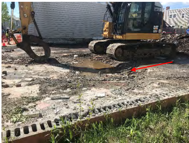
3-6" depression in southeast portion of the slab
