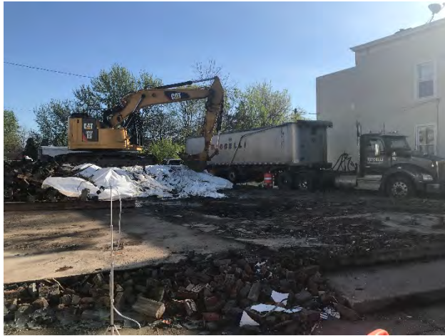
Continuing to load truck with demo debris for haul offsite
