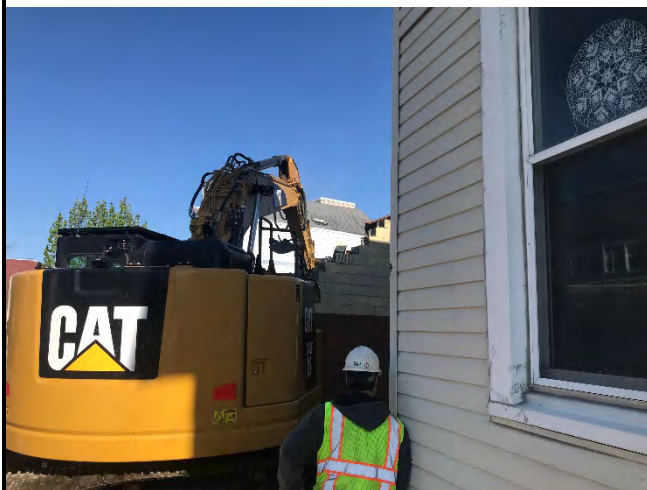
Excavator beginning to tear down east wall
