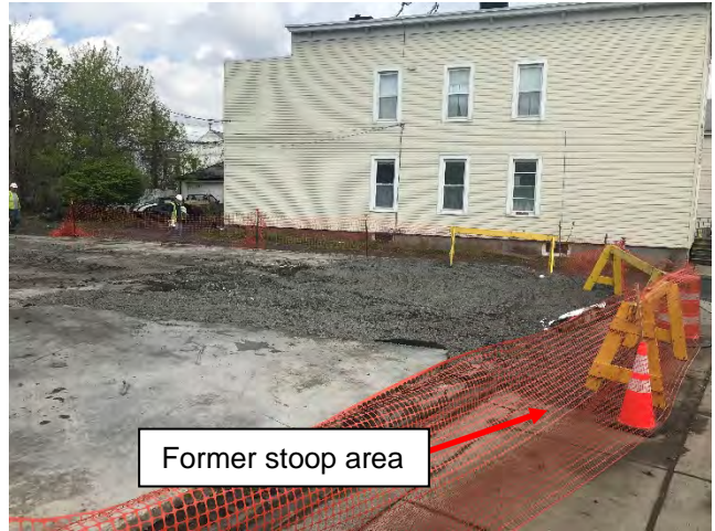
Southeast corner of the slab and former stoop area filled with crusher run looking east
