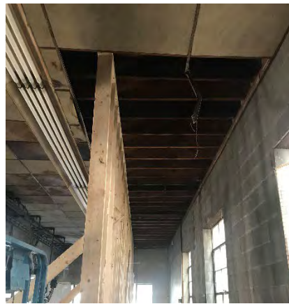
Portion of the ceiling removed for support wall construction (completed 5/4/20)
