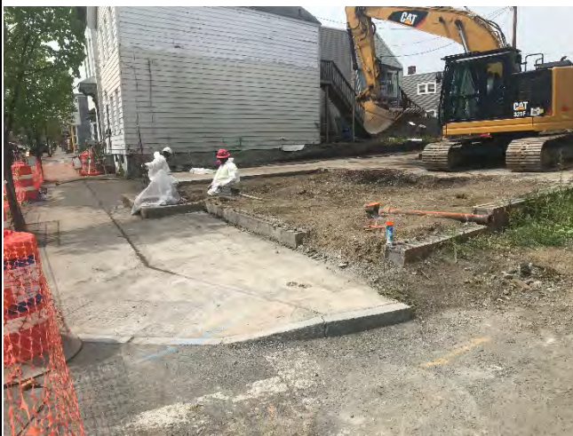
Cleaning demo debris out of gaps in block to pass visual inspection by alpine
