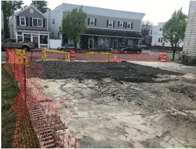
Southeast corner of the slab and former stoop area filled with crusher run looking south
