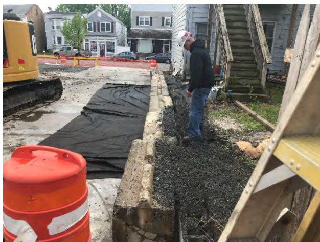
Precast concrete blocks placed over filter fabric along the west edge of foundation looking south
