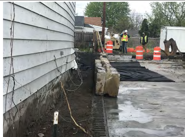
Precast concrete blocks placed over filter fabric the west edge of foundation looking north
