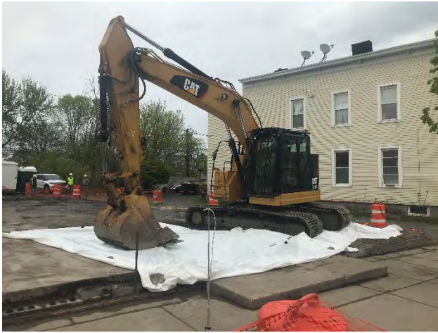
Exposed soil from slab removal covered with 2 layers of 6 mil poly
