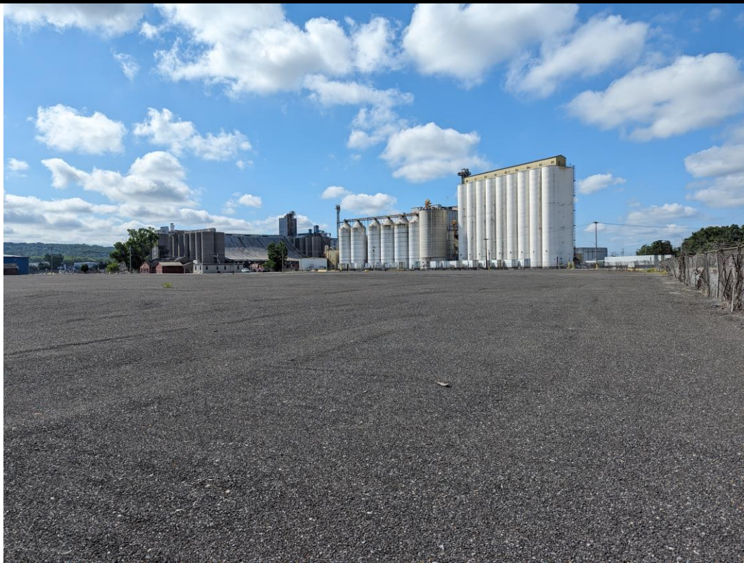
Photograph 1. General overview of the Site, looking southeast.
