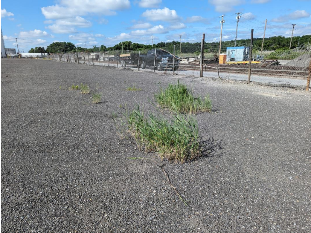
Photograph 4. Example of grass growing on the recycled asphalt pavement cap.
