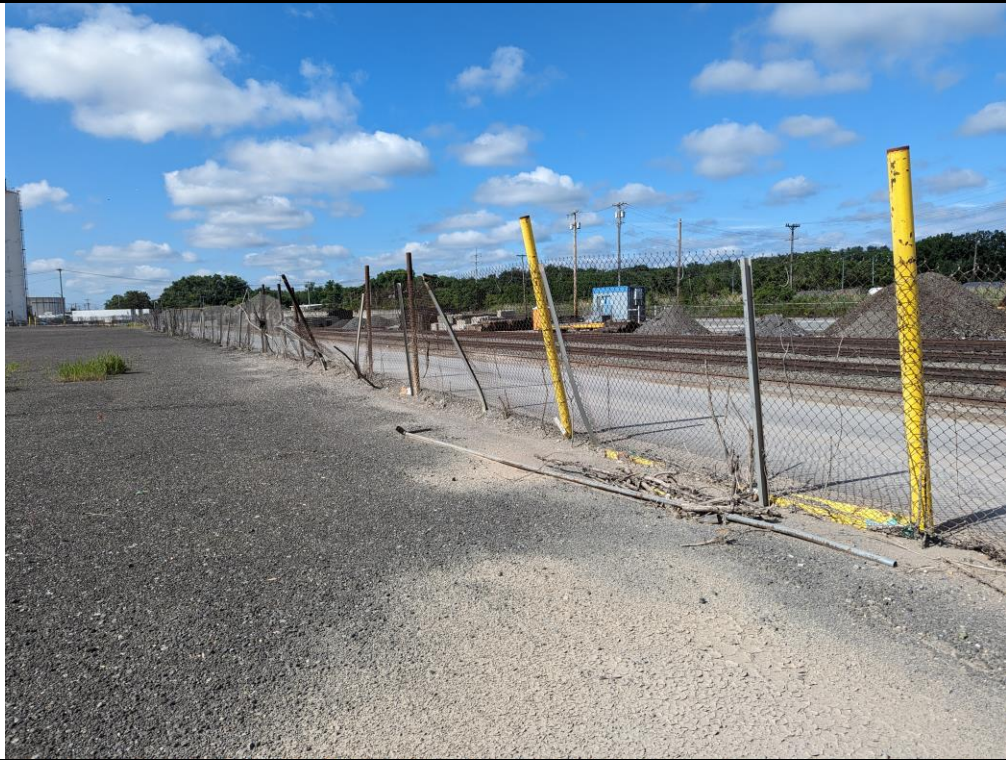
Photograph 7. Fence in place and preventing access. Fence will be replaced during the proposed redevelopment.
