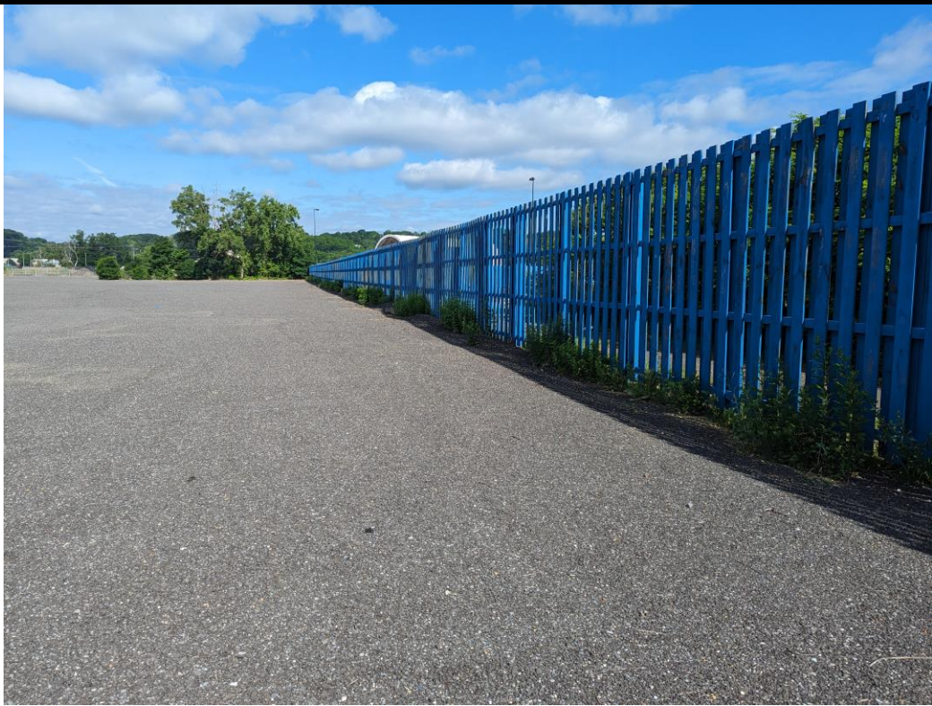
Photograph 3. Fencing along the northern perimeter of the Site with some vegetation growing along the fenceline.
