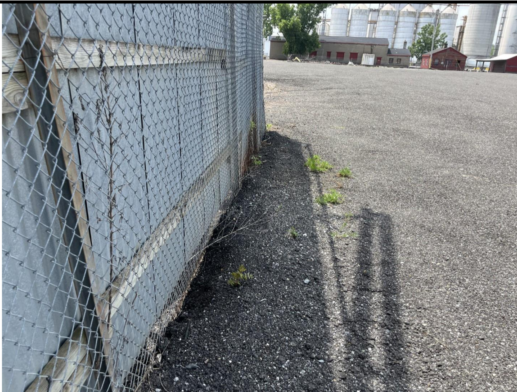
Photograph 5. Location of historical RAP erosion from steam blowdown. Significantly less scour compared to previous site inspections. No repair necessary.
