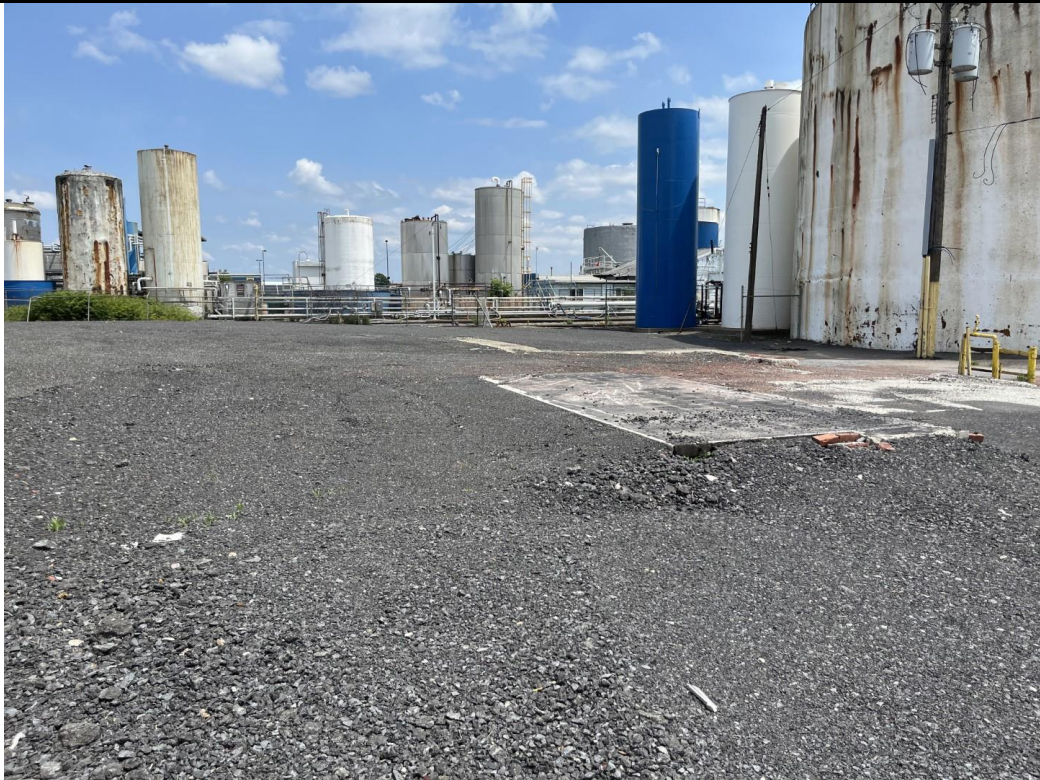
Photograph 4. Overview of the former office building and garage building location. Site cap consisting of concrete and reclaimed asphalt pavement.
