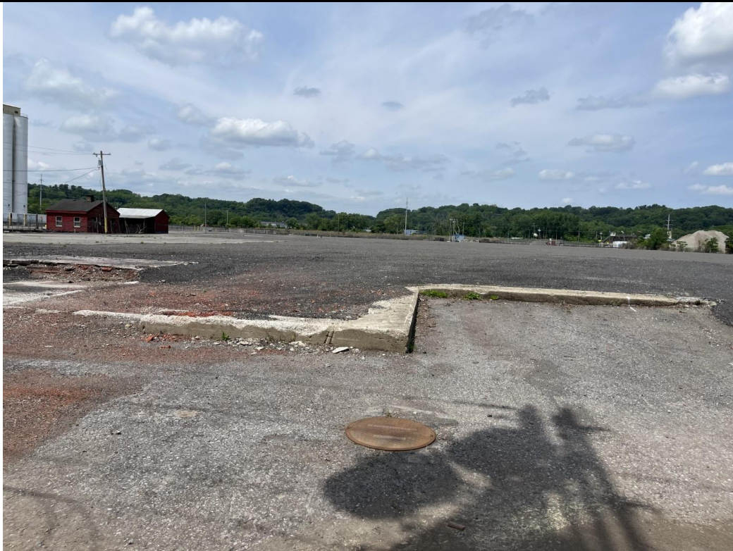
Photograph 3. Former location of the office building and the concrete foundation acting as a site cap.
