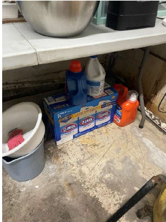
Chemical and tool storage
