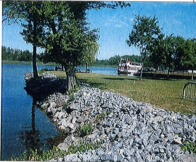
Photo#03 dated 6/2/10 looking N
