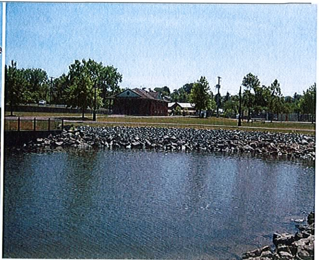
Photo #06 dated 6/2/10 looking S
