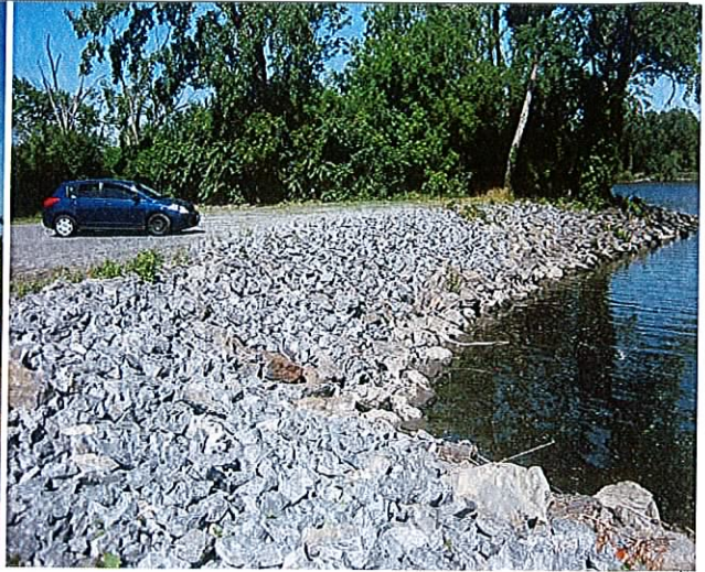
Photo#02 dated 6/2/10 looking W
