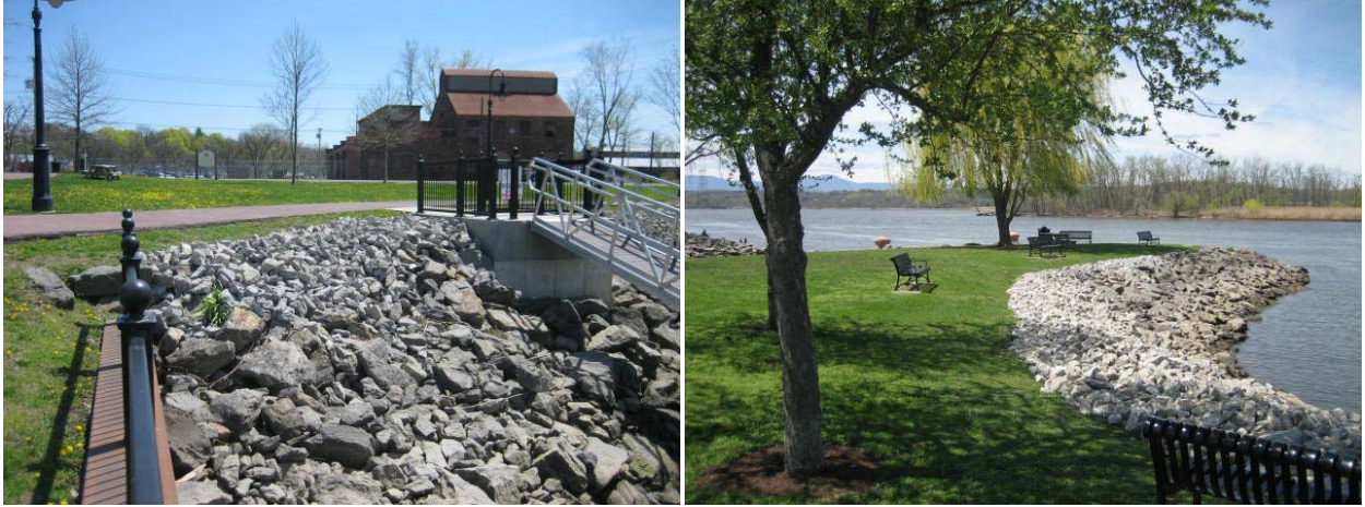
Rip Rap/Stone Riverbank Protection Improvements. Photos Taken: 4/20/13
