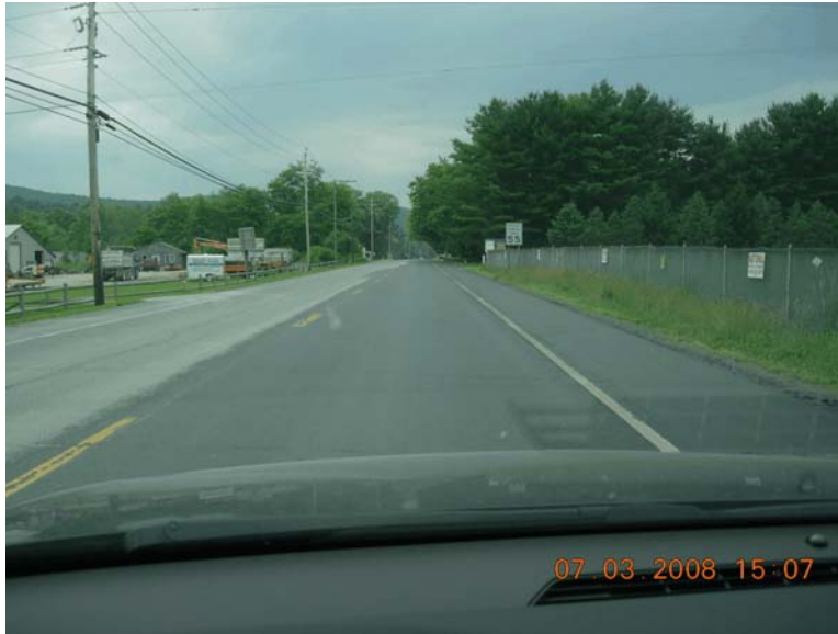
Rte. 20 - Roadway wet down with water truck
