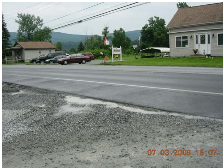
Rte. 20 - Roadway Wet down with water truck
