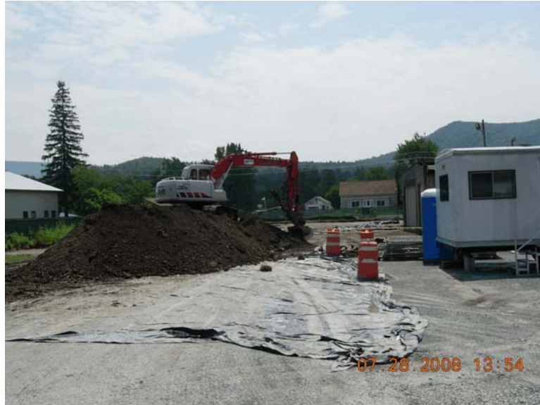
Looking West - Excavating grid J6/K6
