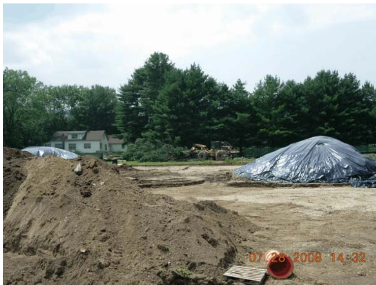
Looking West - Galusha removing trees at west end of site
