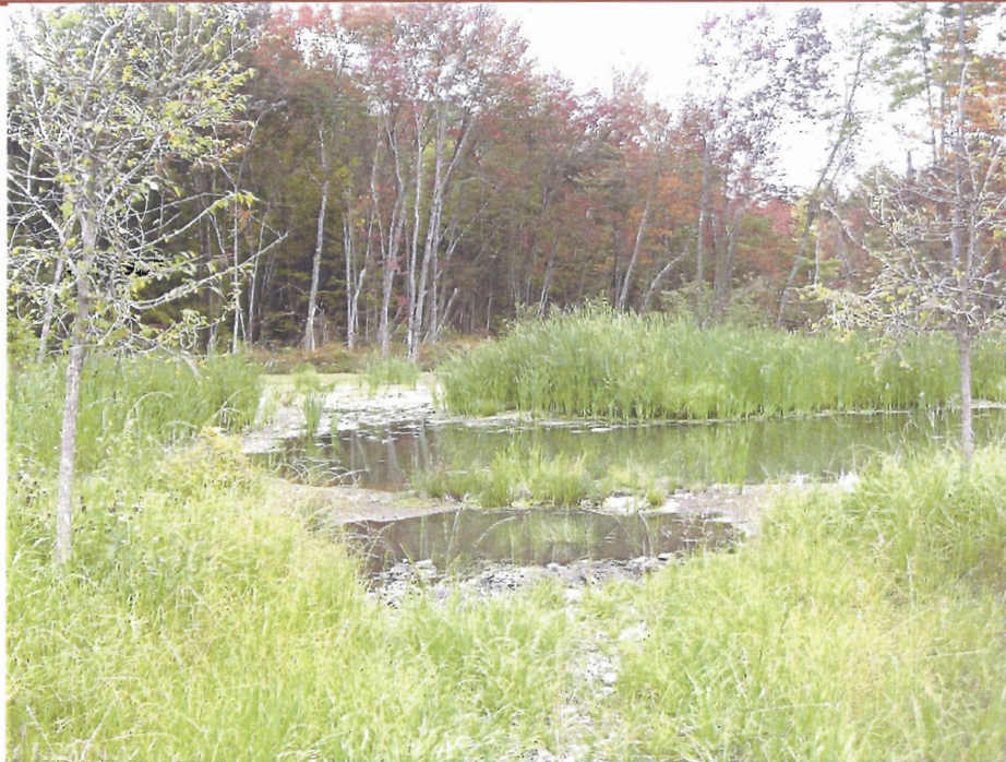
View south of wetland mitigation area/rock lined channel (rip-rap).
