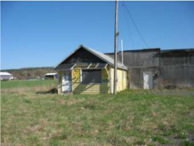
Site #411014 5/2/2013 Photo 4 – Looking N , Yellow building
