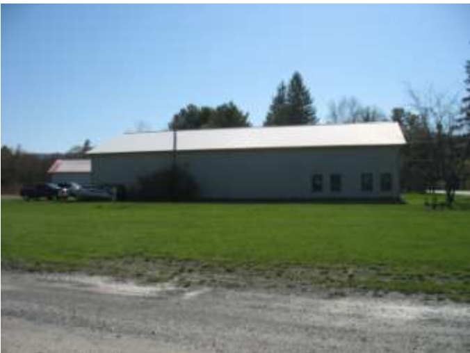
Site #411014 5/2/2013 Photo 9 – Looking E at Theater Barn
