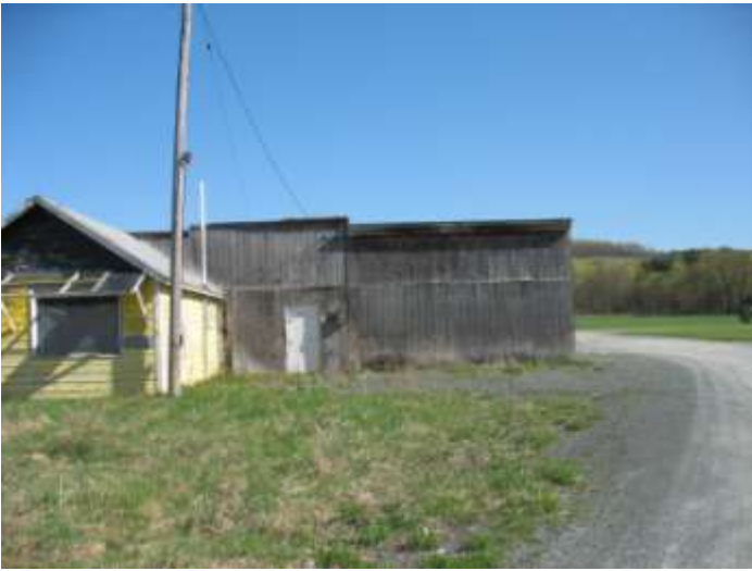
Site #411014 5/2/2013 Photo 5 – Looking N, Yellow building
