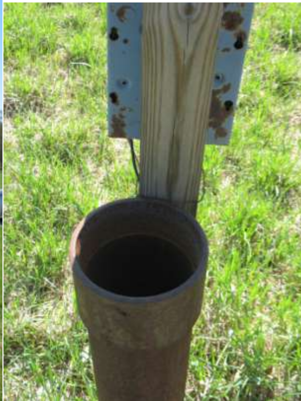
Site #411014 5/2/2013 Photo 16 – Well WSW-4, no cap/lock
