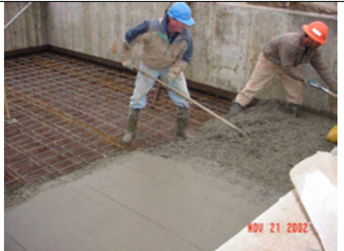
Picture No.: 128 Date Taken: November 21, 2002 Description: Concrete placement within exterior containment area.
