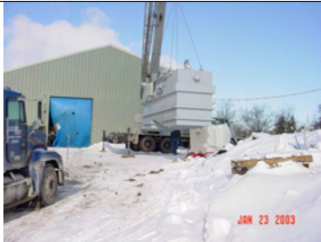
Picture No.: 230 Date Taken: January 23, 2003 Description: Rigging Oil Water Separator.
