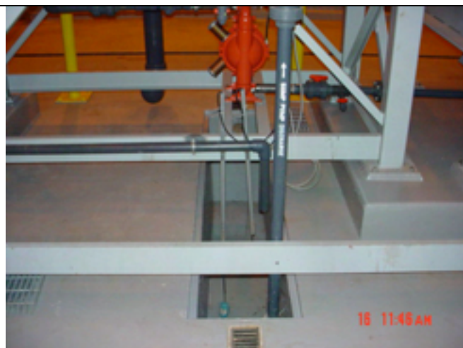
Picture No.: Date Taken: June 16, 2003 Description: Completed main sump/pump (grate temporarily removed).
