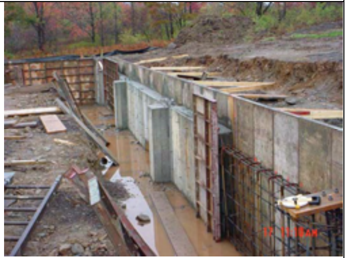
Picture No.: 060 Date Taken: October 17, 2002 Description: Eastern grade wall following removal of inside forms.
