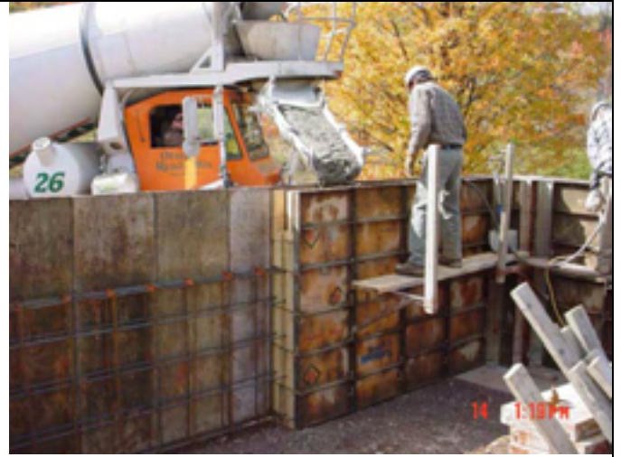
Picture No.: 054 Date Taken: October 15, 2002 Description: Placing concrete for grade wall.
