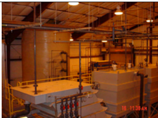
Picture No.: Date Taken: June 16, 2003 Description: Completed system process piping.
