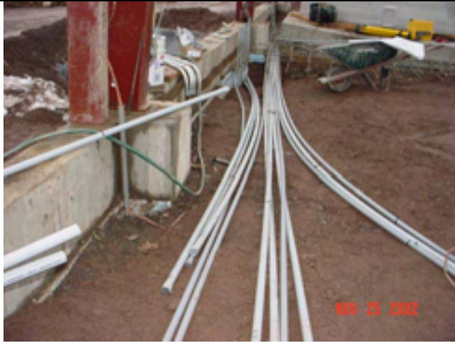
Picture No.: 141 Date Taken: November 25, 2002 Description: Underground electrical conduit.
