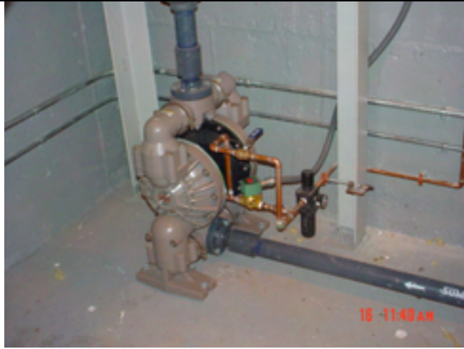
Picture No.: Date Taken: June 16, 2003 Description: Completed air diaphragm pump (exterior sump and recycle flows).
