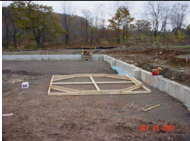
Picture No.: 093 Date Taken: October 30, 2002 Description: Building forms for T-6 concrete pad.
