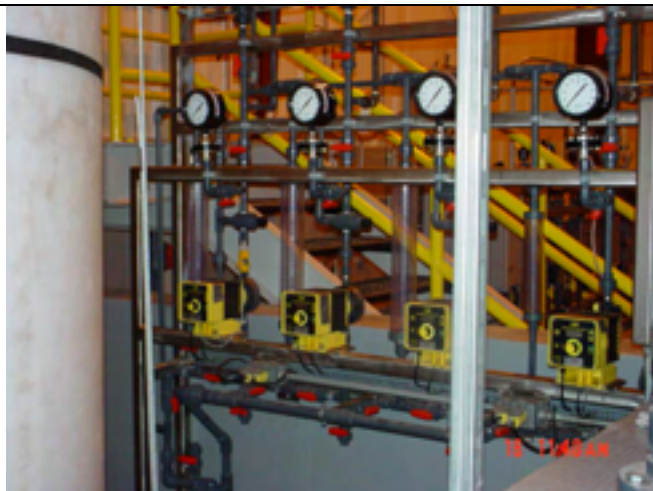
Picture No.: Date Taken: June 16, 2003 Description: Completed caustic feed pumps.
