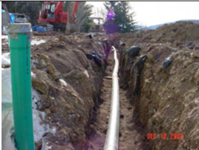
Picture No.: 163 Date Taken: December 10, 2002 Description: Gravity effluent line.
