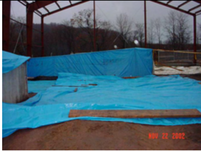
Picture No.: 136 Date Taken: November 22, 2002 Description: GWTP subbase covered overnight due to expected inclement weather.
