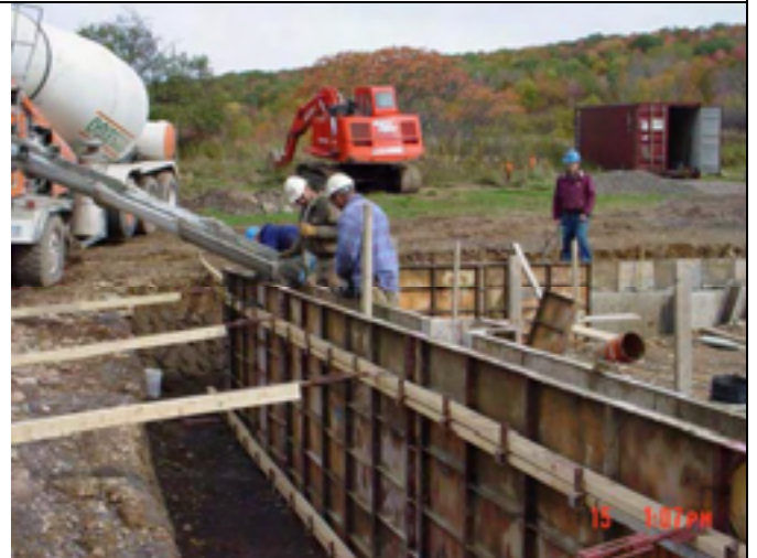
Picture No.: 056 Date Taken: October 15, 2002 Description: Placing concrete for northern grade wall.
