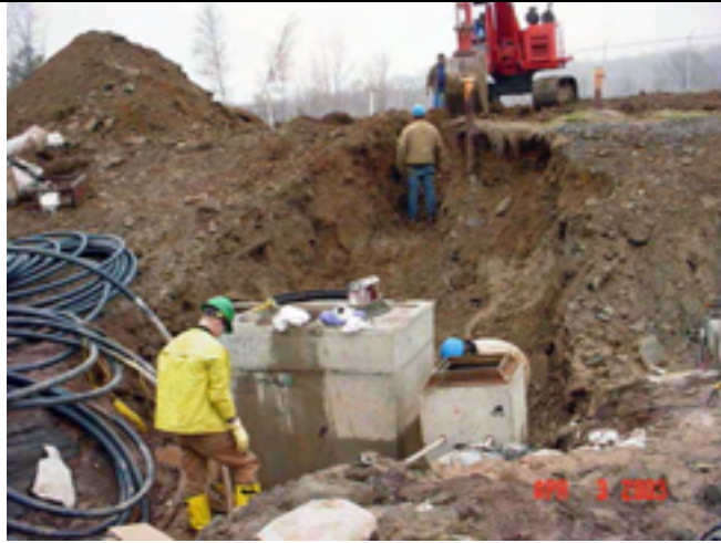
Picture No.: 299 Date Taken: April 2, 2003 Description: Pullbox 7A&B for recovery wells.
