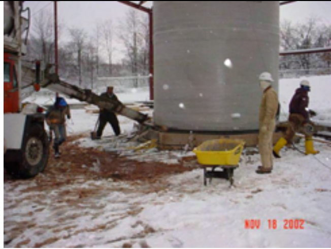
Picture No.: 124 Date Taken: November 18, 2002 Description: Clearing snow to complete subbase backfill activities.
