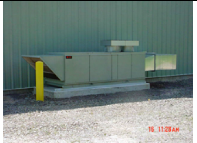
Picture No.: Date Taken: June 16, 2003 Description: Completed air makeup unit.
