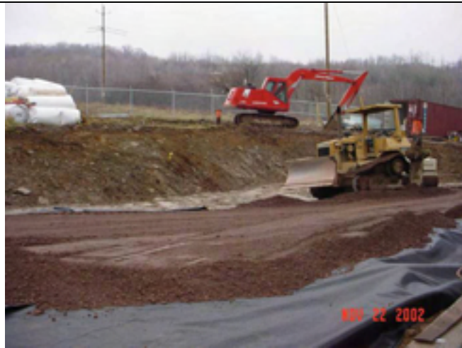
Picture No.: 133 Date Taken: November 22, 2002 Description: Access road along the east side of GWTP consisting of woven geotextile below 6-inch compacted NYSDOT Item 304 Type 4 structural fill.
