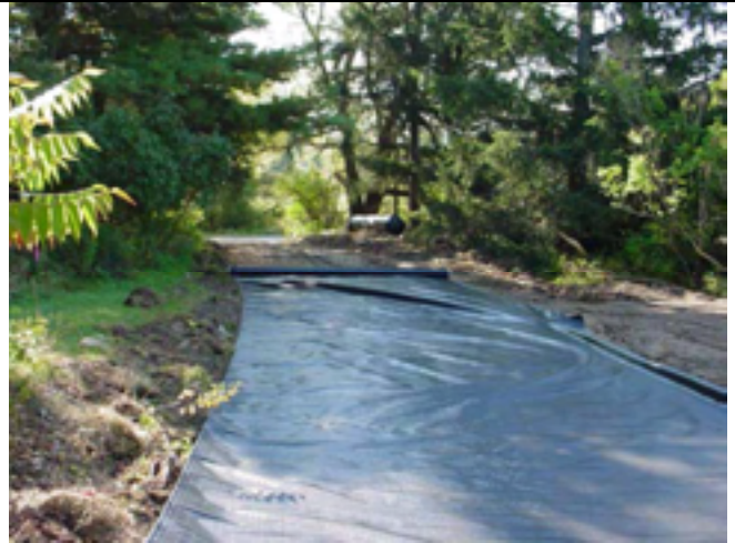
Picture No.: 014 Date Taken: September 30, 2002 Description: Woven geotextile installation for access road.
