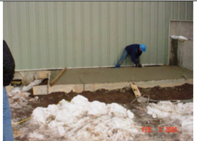
Picture No.: 242 Date Taken: February 3, 2003 Description: Pouring and finishing Diesel Generator Pad.
