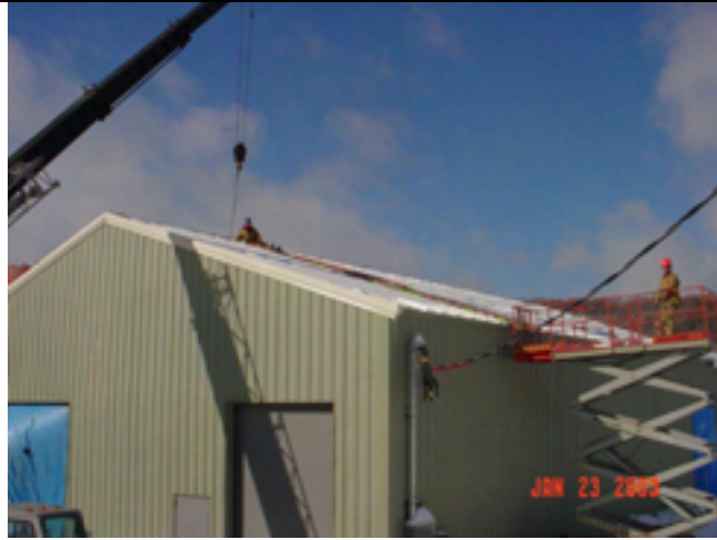
Picture No.: 232 Date Taken: January 23, 2003 Description: Rigging Oil Water Separator utilizing a crane hook through a temporary hole in the roof.
