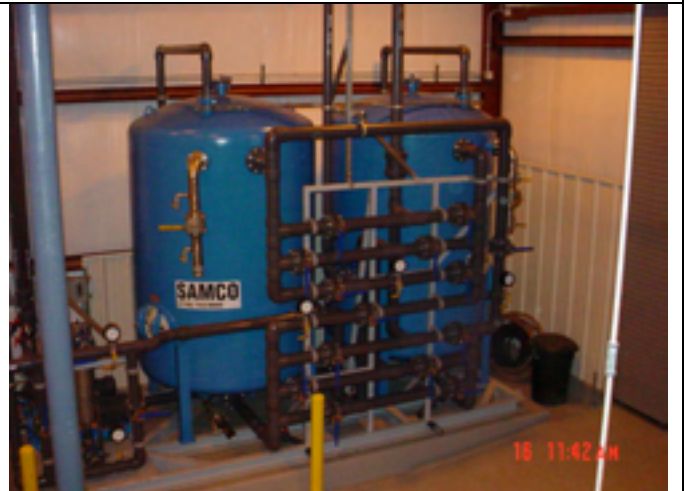
Picture No.: Date Taken: June 16, 2003 Description: Completed carbon unit skid.
