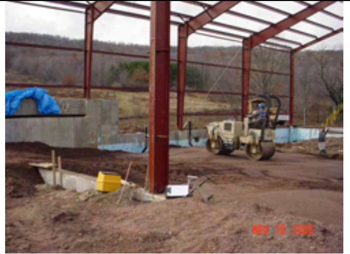
Picture No.: 121 Date Taken: November 15, 2002 Description: Interior subbase compaction.
