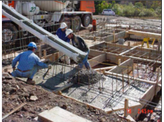
Picture No.: 064 Date Taken: October 18, 2002 Description: Placing concrete for continuous footer within interior containment area.
