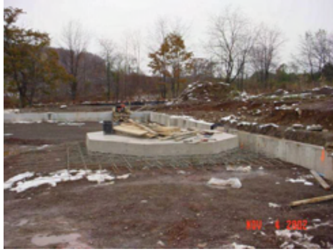
Picture No.: 103 Date Taken: November 4, 2002 Description: Completed T-6 concrete pad.
