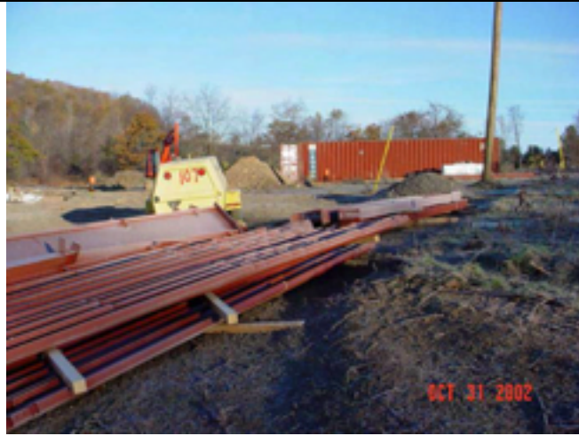
Picture No.: 095 Date Taken: October 31, 2002 Description: Red iron shake out.
