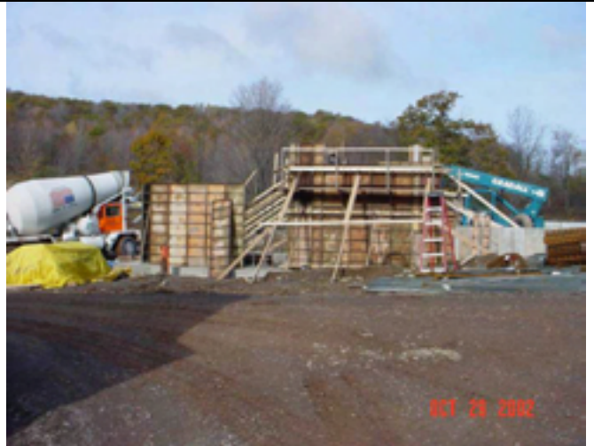
Picture No.: 090 Date Taken: October 29, 2002 Description: Looking north, pouring concrete for interior containment walls.
