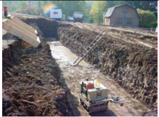
Picture No.: 018 Date Taken: October 1, 2002 Description: Footer excavation bottom leveled and compacted. Constructed footer forms.
