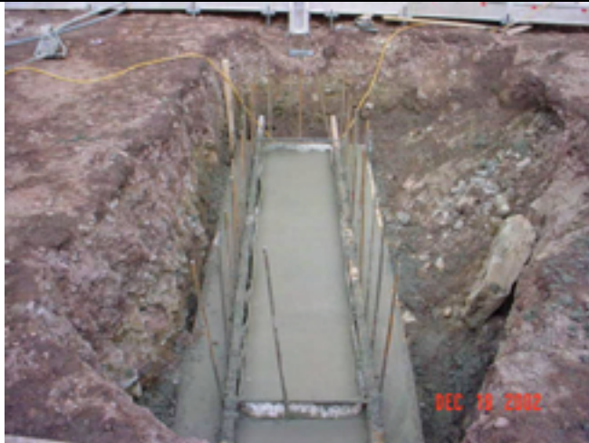
Picture No.: 184 Date Taken: December 19, 2002 Description: GWTP main sump bottom.
