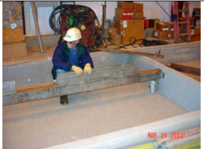
Picture No.: 288 Date Taken: March 24, 2003 Description: Chemical containment area installation. Stainless steel supports.
