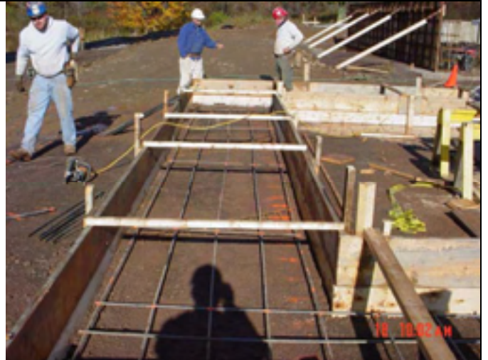
Picture No.: 062 Date Taken: October 18, 2002 Description: Installation of reinforced steel within continuous footer area.
