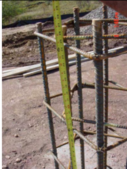
Picture No.: 038 Date Taken: October 8, 2002 Description: Inspecting rebar spacing.
