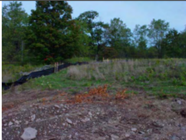
Picture No.: 003 Date Taken: September 25, 2002 Description: Silt fence installed downgradient of work area.
