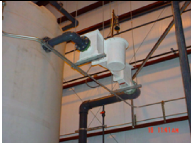
Picture No.: Date Taken: June 16, 2003 Description: Completed Parshall Flume (gravity effluent flow measurement).
