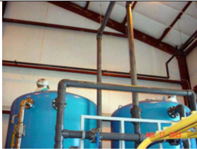
Picture No.: 282 Date Taken: March 17, 2003 Description: GAC units installation with process piping.
