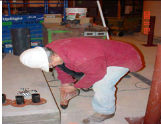
Picture No.: 255 Date Taken: February 17, 2003 Description: Installing interior bollards.
