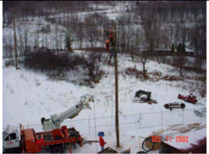
Picture No.: 167 Date Taken: December 11, 2002 Description: From above, NYSEG installing 3-phase transformer tubs and electrical lines.
