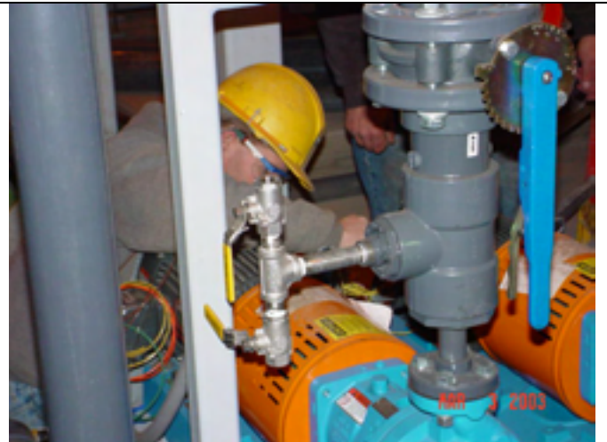
Picture No.: 272 Date Taken: March 3, 2003 Description: Air stripper pump installation.
