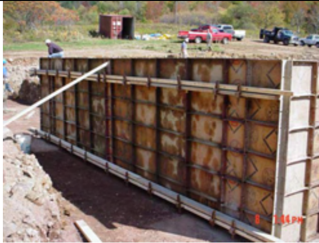
Picture No.: 037 Date Taken: October 8, 2002 Description: Forming grade wall.
