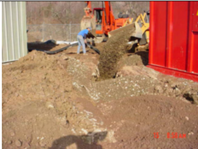
Picture No.: 316 Date Taken: April 15, 2003 Description: Drainage trench backfilling.
