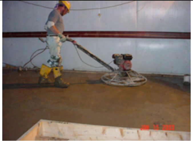
Picture No.: 215 Date Taken: January 13, 2003 Description: Finishing concrete slabs.
