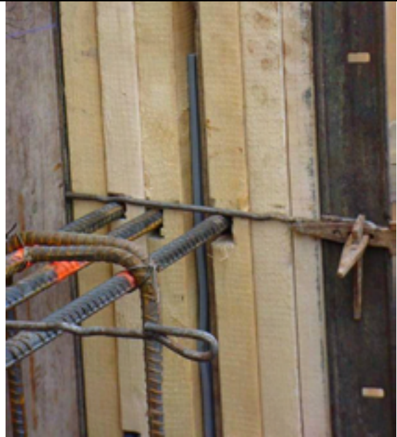
Picture No.: 046 Date Taken: October 10, 2002 Description: Temporary bracing for rebar.
