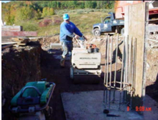
Picture No.: 033 Date Taken: October 8, 2002 Description: Structural backfill compaction around footers
