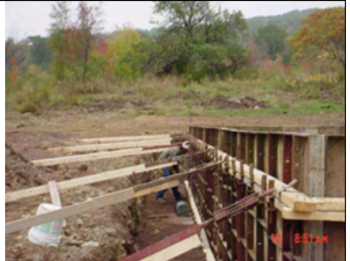
Picture No.: 042 Date Taken: October 10, 2002 Description: Temporary bracing for grade wall forms.
