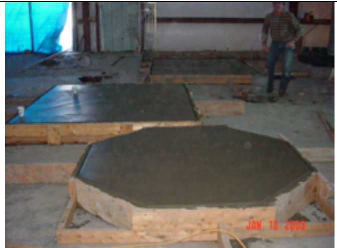
Picture No.: 210 Date Taken: January 10, 2003 Description: Forming equipment pads.
