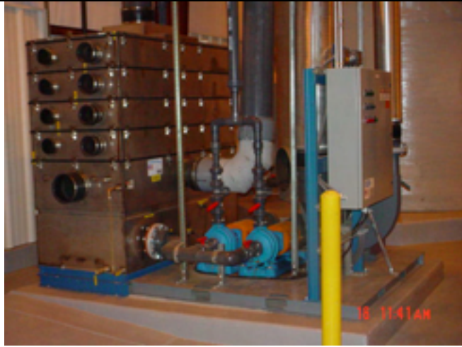
Picture No.: Date Taken: June 16, 2003 Description: Completed air stripper skid.
