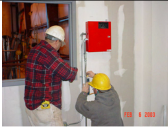
Picture No.: 248 Date Taken: February 6, 2003 Description: Fire alarm panel installation.
