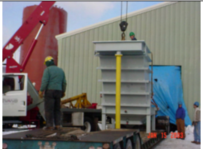
Picture No.: 218 Date Taken: January 18, 2003 Description: Rigging Inclined Plate Clarifier.
