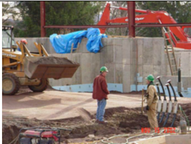
Picture No.: 122 Date Taken: November 15, 2002 Description: GWTP interior subbase backfill/compaction. Groundwater influent line stickups from RW1-4.
