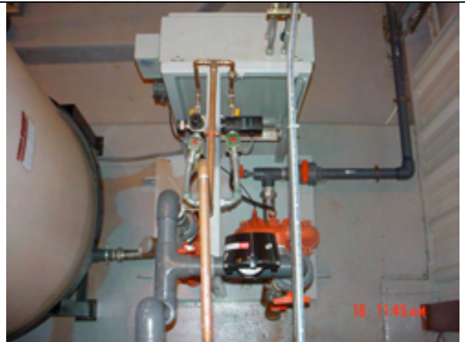
Picture No.: Date Taken: June 16, 2003 Description: Completed filter press sludge pumps and panel from above.
