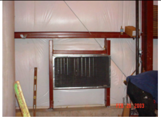
Picture No.: 266 Date Taken: February 25, 2003 Description: Air makeup exhaust.
