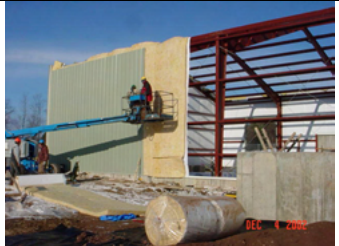
Picture No.: 154 Date Taken: December 4, 2002 Description: Installation of exterior panels/insulation on west side of GWTP.
