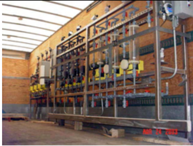
Picture No.: 289 Date Taken: March 24, 2003 Description: Chemical feed skid delivery.
