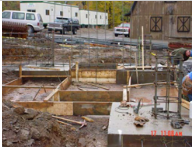
Picture No.: 059 Date Taken: October 17, 2002 Description: Continuous footer forming.
