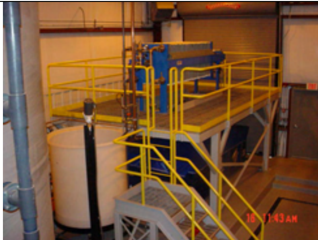
Picture No.: Date Taken: June 16, 2003 Description: Completed filter press, precoat tank and safety stairs/platform/railings.
