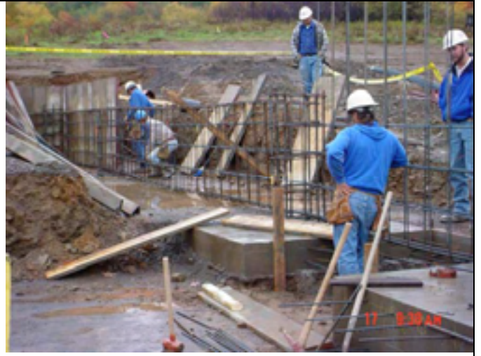
Picture No.: 058 Date Taken: October 17, 2002 Description: Continuous footer forming.
