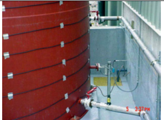
Picture No.: 369 Date Taken: May 5, 2003 Description: T-1 heat tracing.
