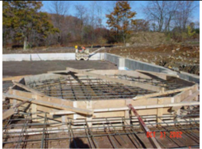
Picture No.: 096 Date Taken: October 31, 2002 Description: Looking north, T-6 concrete pad forms and rebar prior to pour.
