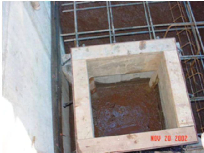
Picture No.: 127 Date Taken: November 20, 2002 Description: Concrete sump within exterior containment area.
