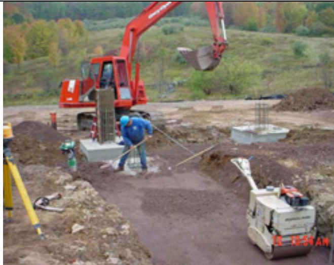
Picture No.: 043 Date Taken: October 10, 2002 Description: Structural backfill below GWTP.
