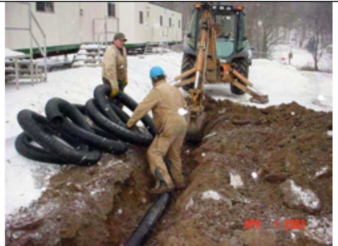
Picture No.: 295 Date Taken: April 1, 2003 Description: Drainage trench installation (6 inch perforated pipe within 2 ft wide trench).
