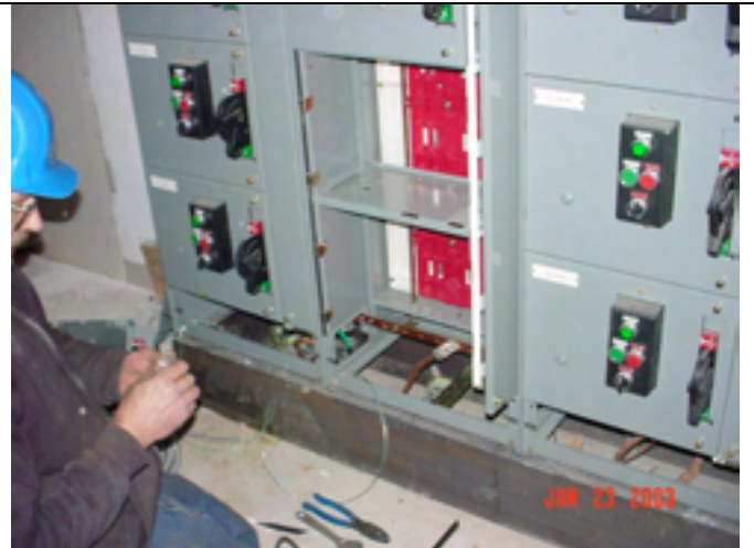
Picture No.: 231 Date Taken: January 23, 2003 Description: Installation of Main Control Center.
