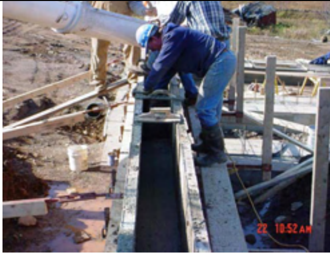
Picture No.: 073 Date Taken: October 22, 2002 Description: Concrete placement within eastern grade wall.
