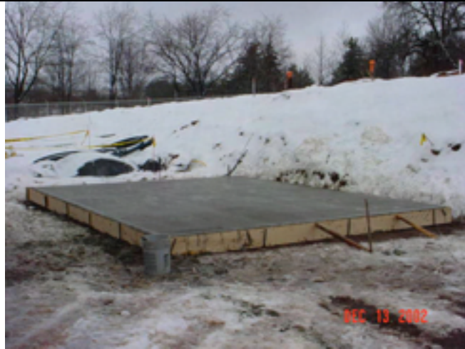
Picture No.: 172 Date Taken: December 13, 2002 Description: Propane tank concrete pad.
