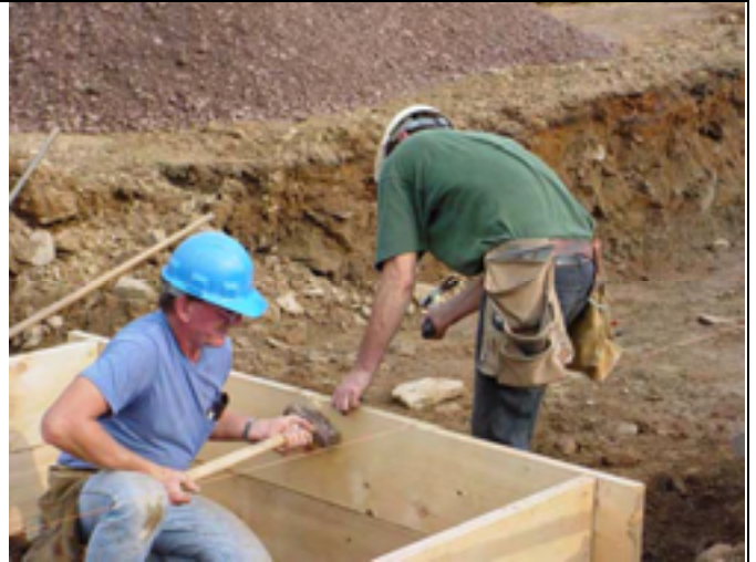
Picture No.: 022 Date Taken: October 2, 2002 Description: Footer form construction.
