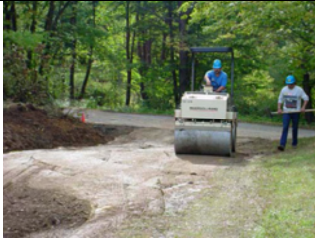
Picture No.: 001 Date Taken: September 25, 2002 Description: Compacting access road at the North Area.
