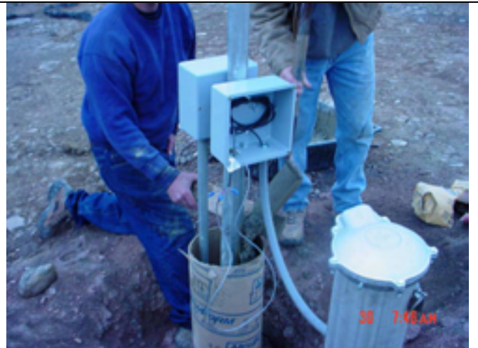
Picture No.: 355 Date Taken: April 30, 2003 Description: Recovery well electrical/instrumentation connections.
