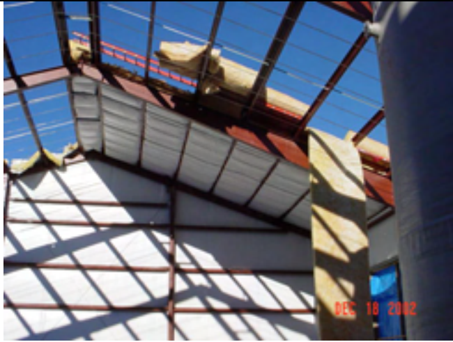
Picture No.: 180 Date Taken: December 18, 2002 Description: Roof panels/insulation installation.
