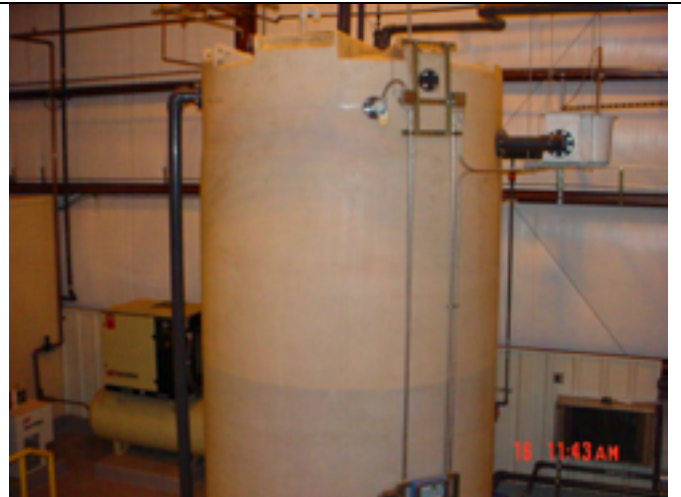
Picture No.: Date Taken: June 16, 2003 Description: Completed effluent tank (T-14).
