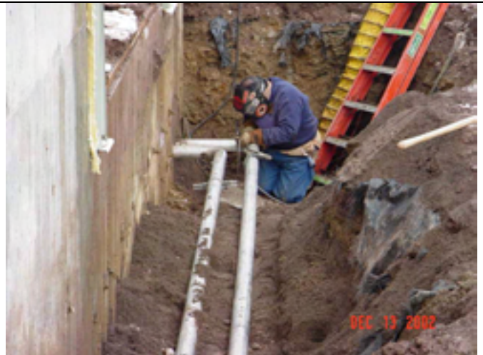
Picture No.: 171 Date Taken: December 13, 2002 Description: Stainless steel process piping installation located below ground on the south side of the GWTP.
