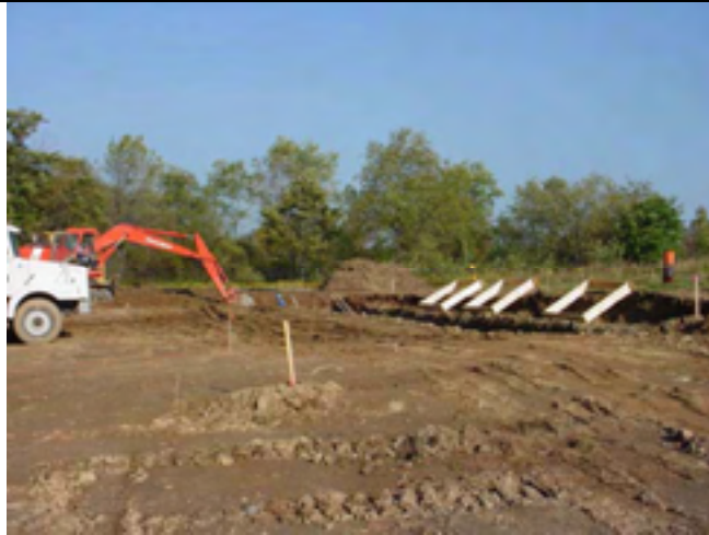
Picture No.: 017 Date Taken: October 1, 2002 Description: Footer excavation. Constructed footer forms.
