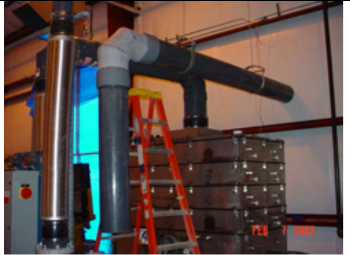
Picture No.: 249 Date Taken: February 7, 2003 Description: Air stripper installation.
