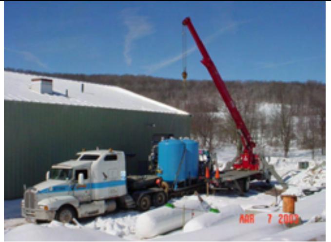
Picture No.: 277 Date Taken: March 7, 2003 Description: GAC unit delivery.
