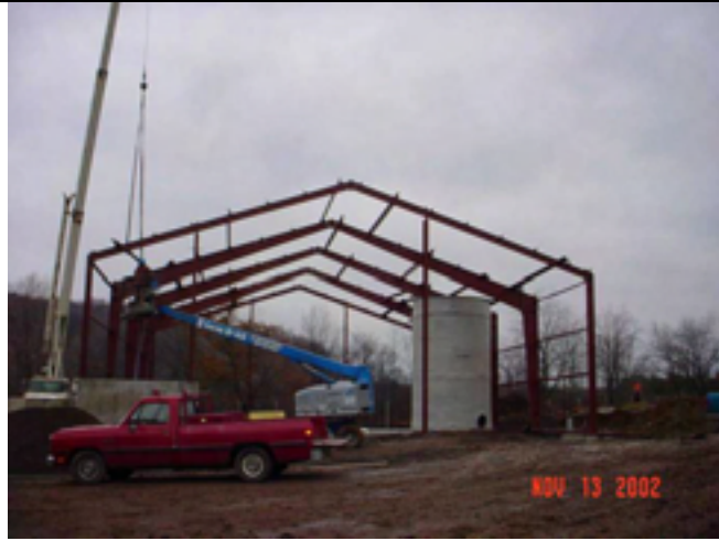
Picture No.: 118 Date Taken: November 13, 2002 Description: T-6 tank set on concrete pad. Craine installing red iron framing.
