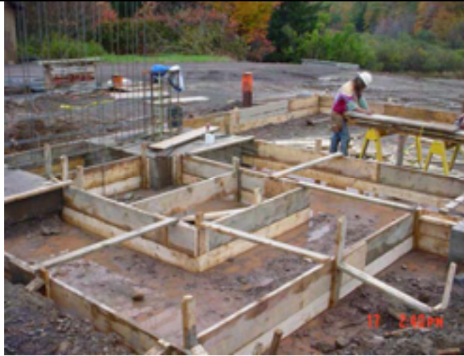
Picture No.: 061 Date Taken: October 17, 2002 Description: Continuous footer forms at interior and exterior containment areas.
