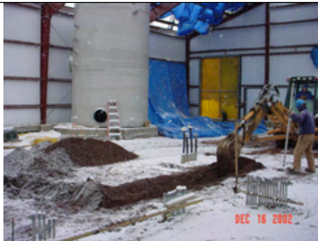
Picture No.: 175 Date Taken: December 16, 2002 Description: Floor drain trenching.
