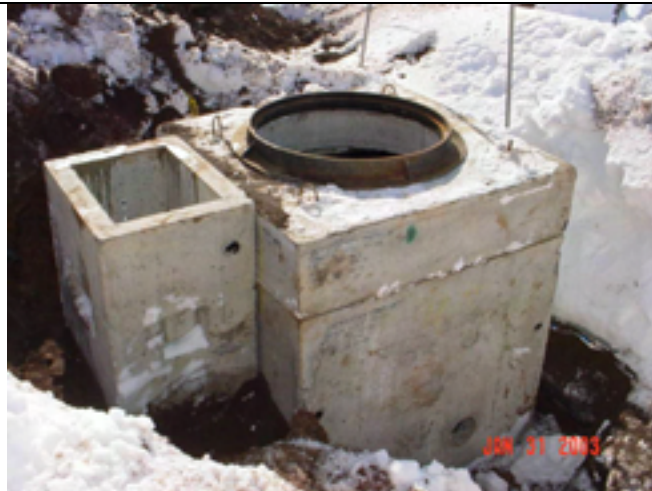
Picture No.: 240 Date Taken: January 31, 2003 Description: Installation of precast concrete Pullboxes 1A and 1B.
