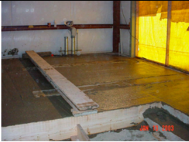
Picture No.: 213 Date Taken: January 13, 2003 Description: Main slab and raised slab concrete.
