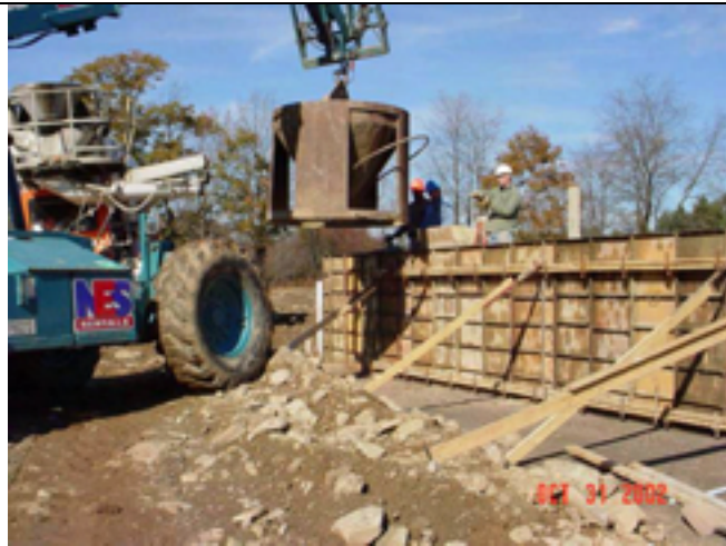
Picture No.: 098 Date Taken: October 31, 2002 Description: Pouring containment wall utilizing the lull and funnel drop.
