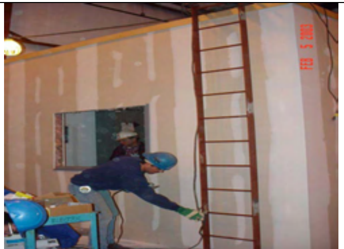
Picture No.: 246 Date Taken: February 5, 2003 Description: Installation of Office safety ladder to loft above. Office window in background.
