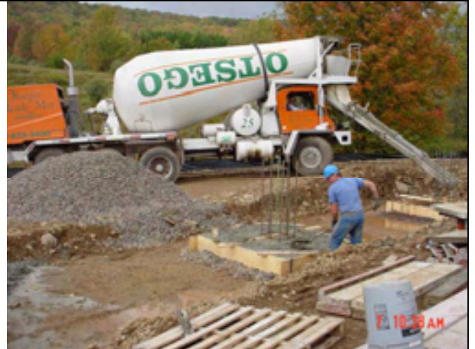
Picture No.: 032 Date Taken: October 7, 2002 Description: Footer installation.
