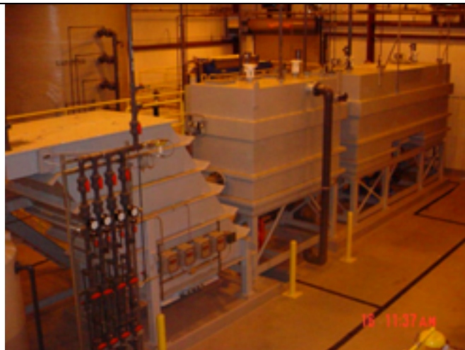
Picture No.: Date Taken: June 16, 2003 Description: Completed main treatment train – oil/water separator, Reaction Tank Unit, and inclined plate clarifier.
