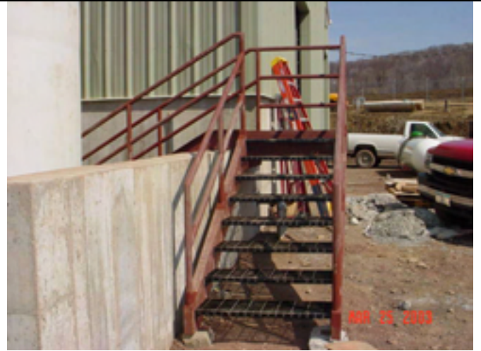
Picture No.: 290 Date Taken: March 25, 2003 Description: Exterior containment area stair installation.
