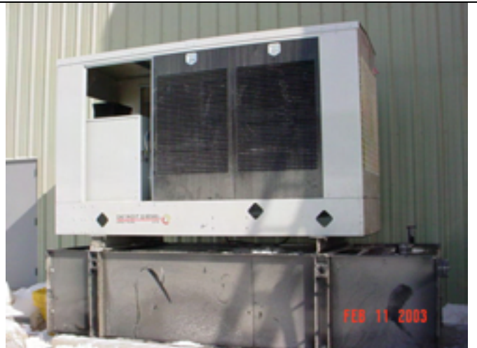
Picture No.: 252 Date Taken: February 11, 2003 Description: Emergency Diesel Generator.
