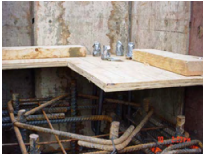
Picture No.: 047 Date Taken: October 10, 2002 Description: Forming corner column with anchor bolts.
