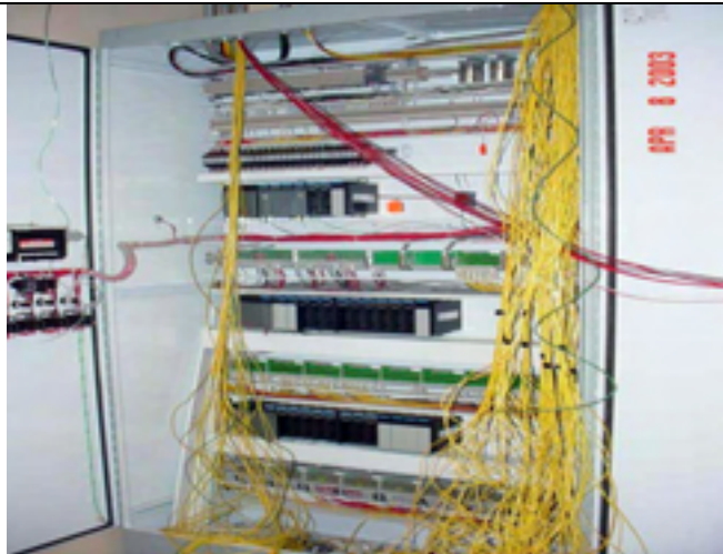
Picture No.: 306 Date Taken: April 8, 2003 Description: Wiring PLC within MCP.
