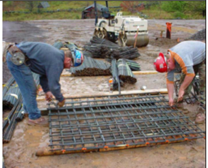
Picture No.: 024 Date Taken: October 3, 2002 Description: Bending reinforcing steel for footer
