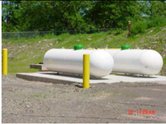
Picture No.: Date Taken: June 16, 2003 Description: Completed propane tanks.
