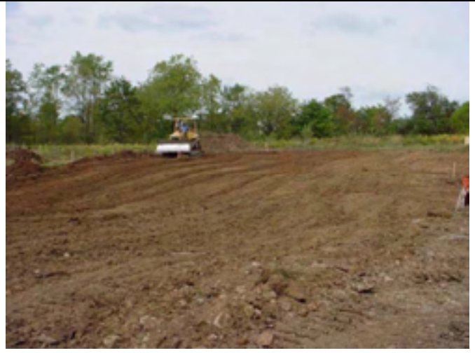
Picture No.: 010 Date Taken: September 25, 2002 Description: Top soil removal; site grading.
