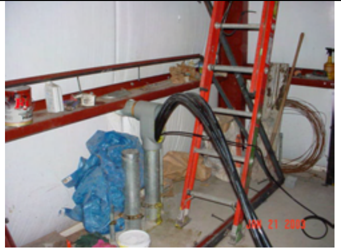
Picture No.: 227 Date Taken: January 21, 2003 Description: Pulling electrical cables (3 phase wire) from below ground at southeast corner .
