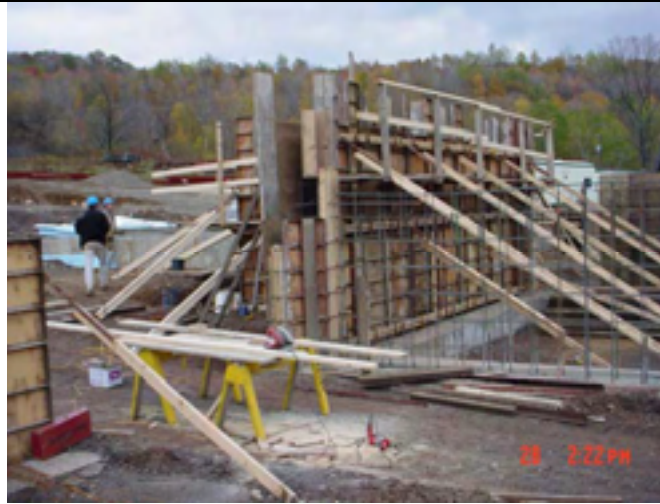
Picture No.: 088 Date Taken: October 28, 2002 Description: Completed forms for interior containment walls. Temporary bracing and scaffolding for placing concrete.
