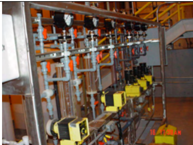
Picture No.: Date Taken: June 16, 2003 Description: Completed acid/polymer feed pumps.
