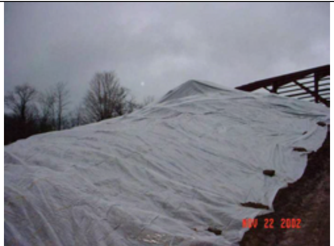
Picture No.: 135 Date Taken: November 22, 2002 Description: Staged soil was covered to minimize soil erosion.
