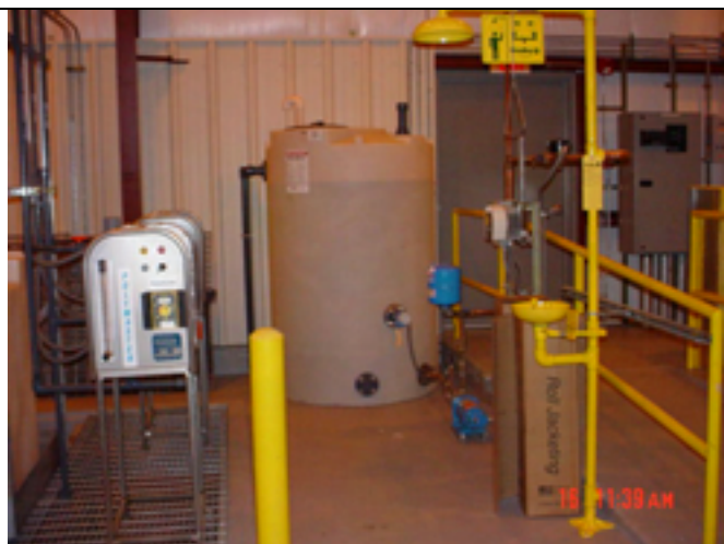
Picture No.: Date Taken: June 16, 2003 Description: Completed polymer pumps, potable water tank/pump, safety shower/eye wash.
