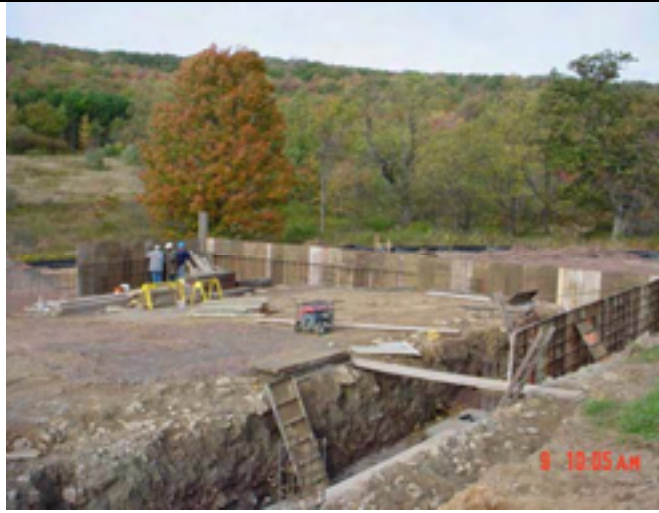
Picture No.: 041 Date Taken: October 9, 2002 Description: Forming grade wall.
