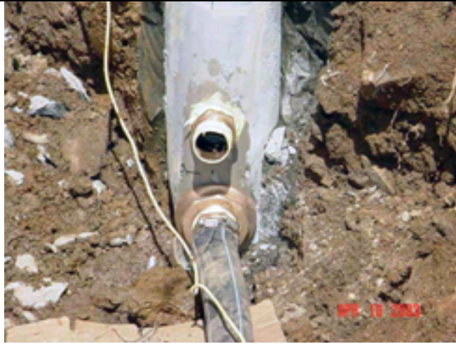
Picture No.: 310 Date Taken: April 10, 2003 Description: Recovery well pitless adapter connection.
