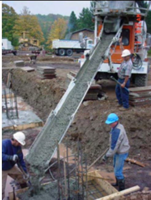
Picture No.: 029 Date Taken: October 7, 2002 Description: Placement of concrete in GWTP footer
