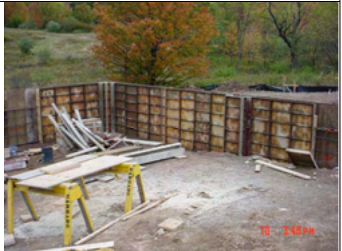
Picture No.: 048 Date Taken: October 10, 2002 Description: Grade wall forms.
