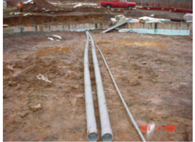
Picture No.: 104 Date Taken: November 4, 2002 Description: Looking east, electrical conduit prior to underground placement.
