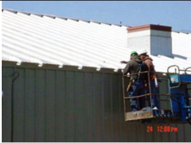
Picture No.: 337 Date Taken: April 24, 2003 Description: Roof gutters and ice breaker installation.
