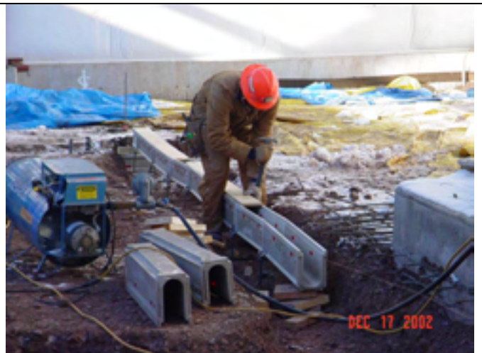
Picture No.: 177 Date Taken: December 17, 2002 Description: Floor drain installation.
