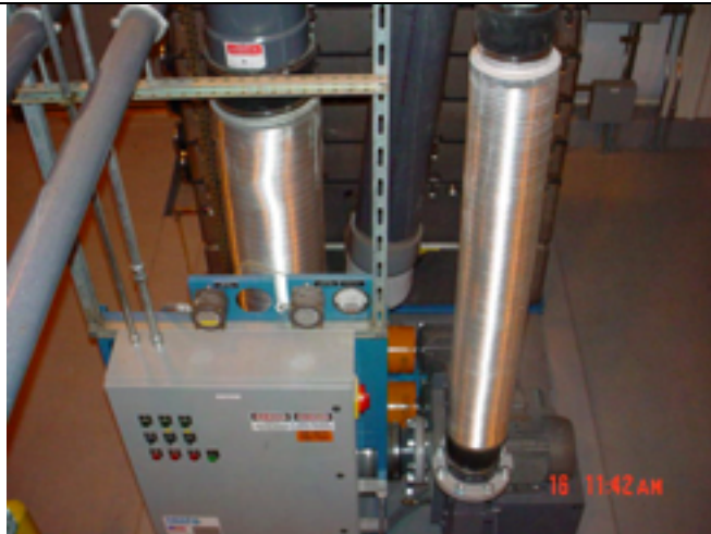
Picture No.: Date Taken: June 16, 2003 Description: Completed air stripper silencers and panel..
