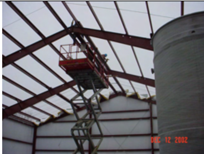
Picture No.: 170 Date Taken: December 12, 2002 Description: Sissor lift used to install roof straps for insulation support.
