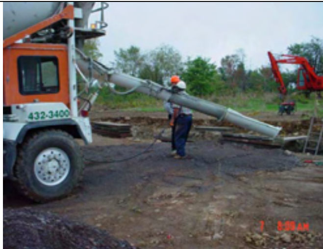
Picture No.: 027 Date Taken: October 7, 2002 Description: Concrete truck placing concrete in formed footers.
