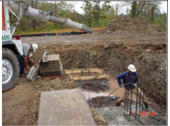
Picture No.: 028 Date Taken: October 7, 2002 Description: Concrete placement
