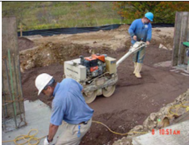
Picture No.: 035 Date Taken: October 8, 2002 Description: Backfill compaction.
