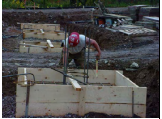
Picture No.: 026 Date Taken: October 3, 2002 Description: Footer forms and reinforcing steel ready in preparation for concrete pour.
