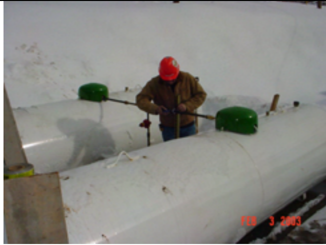
Picture No.: 243 Date Taken: February 3, 2003 Description: Installation of two 1,000 gallon propane tanks (for permanent heating).
