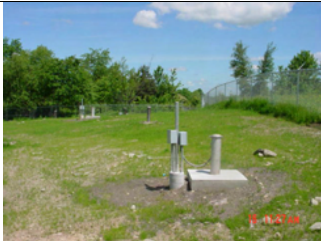
Picture No.: Date Taken: June 16, 2003 Description: Completed RW1-4 and NMW1-10 with pads and seeding.
