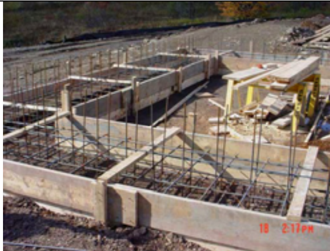
Picture No.: 063 Date Taken: October 18, 2002 Description: Completed reinforced steel installation within exterior containment area continuous footer.
