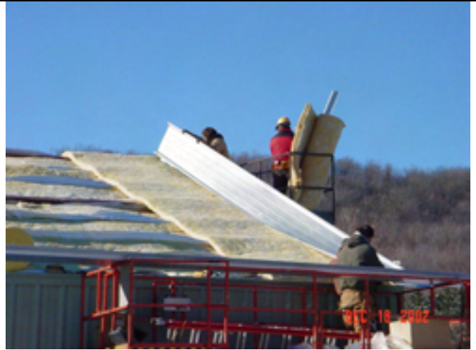
Picture No.: 181 Date Taken: December 18, 2002 Description: Roof insulation/panel installation.
