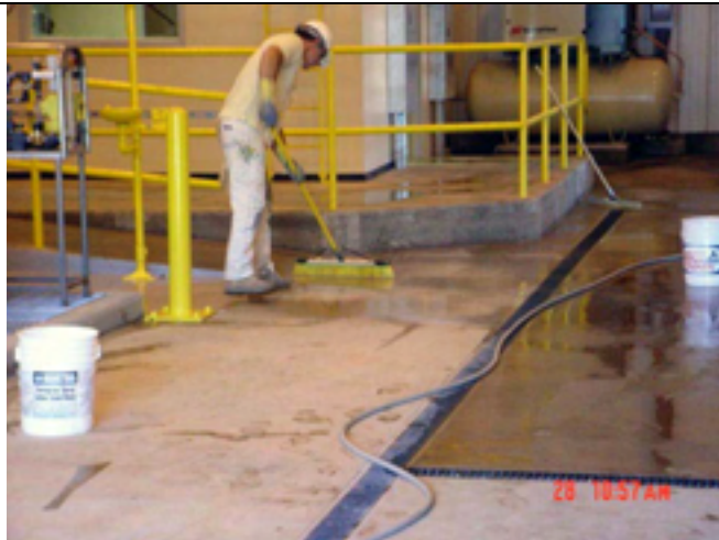
Picture No.: 347 Date Taken: April 28, 2003 Description: GWTP main slab acid etching.
