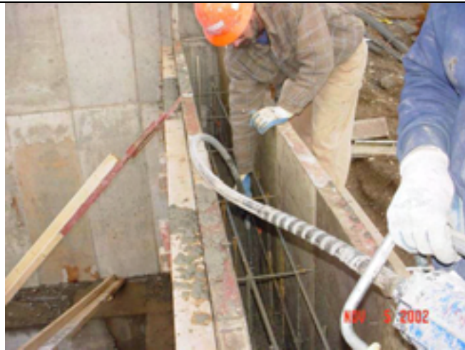
Picture No.: 107 Date Taken: November 5, 2002 Description: Pouring and vibrating concrete within the containment walls.
