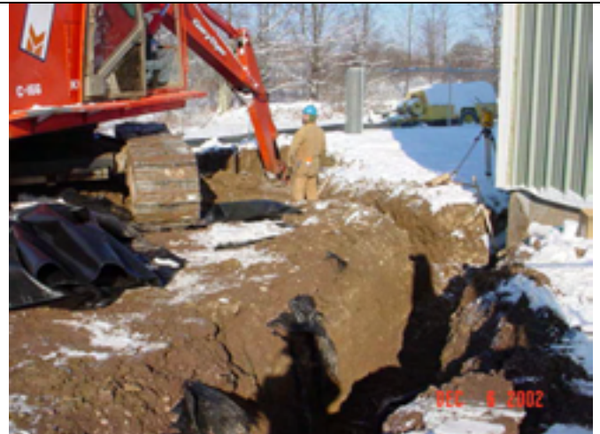
Picture No.: 157 Date Taken: December 6, 2002 Description: Underground septic tank installation at northwest corner of GWTP. Effluent pipe trenching.
