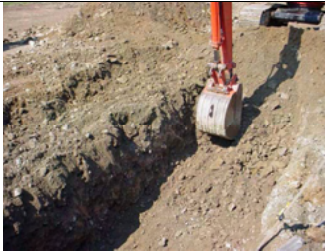
Picture No.: 015 Date Taken: September 30, 2002 Description: Footer excavation.
