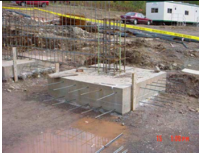
Picture No.: 057 Date Taken: October 15, 2002 Description: Completed footer with rebar connections for continuous footer at containment areas.
