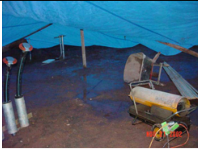
Picture No.: 131 Date Taken: November 21, 2002 Description: Covering and heating the GWTP subbase.
