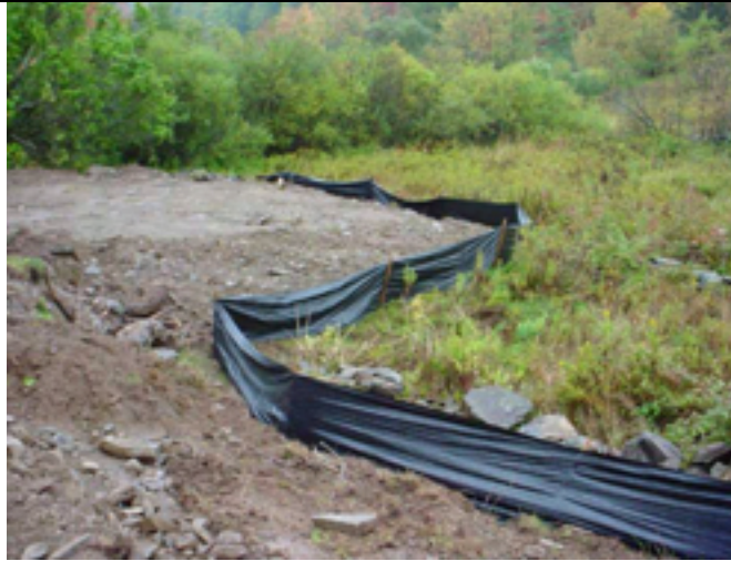
Picture No.: 025 Date Taken: October 3, 2002 Description: Silt fence installation along west side of site.
