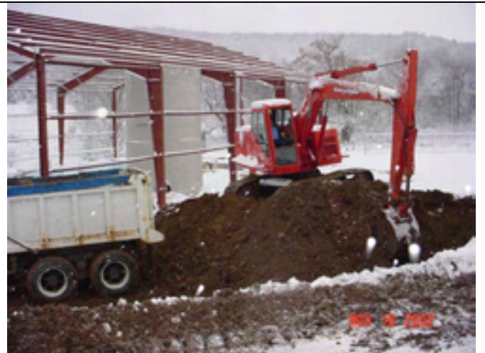
Picture No.: 123 Date Taken: November 18, 2002 Description: Site cuts and fills along east side of GWTP. Material from east side used for fills on west side.
