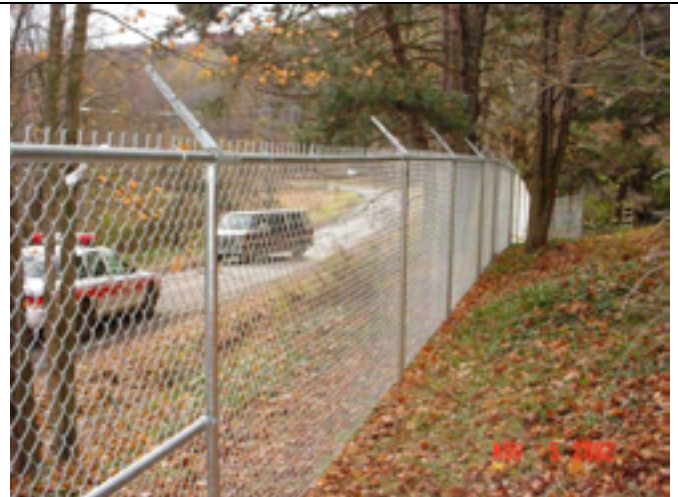
Picture No.: 108 Date Taken: November 5, 2002 Description: Completed 6 foot high chain link fence along RHR at the North Area site.
