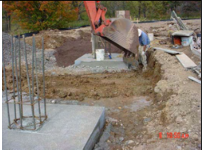
Picture No.: 034 Date Taken: October 8, 2002 Description: Completed footers (6 ft by 6 ft by 2 ft); backfill around footers.
