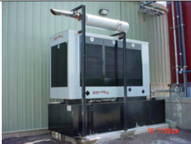
Picture No.: Date Taken: June 16, 2003 Description: Completed emergency diesel generator.
