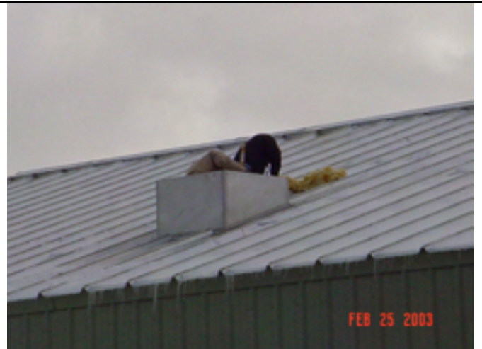
Picture No.: 263 Date Taken: February 25, 2003 Description: Hatch for T-6 mixer motor access.
