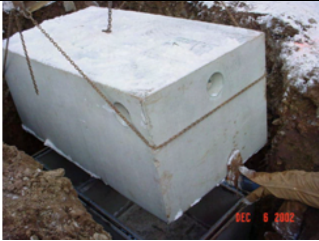
Picture No.: 159 Date Taken: December 6 2002 Description: 1000 gallon concrete underground septic tank installation.
