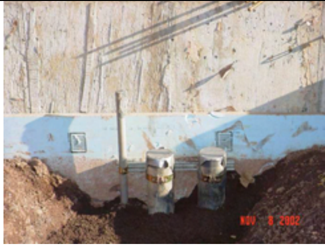
Picture No.: 110 Date Taken: November 8, 2002 Description: Temporarily capped process piping lines leading to P1 and P2. Insulation board installed along subsurface concrete wall.
