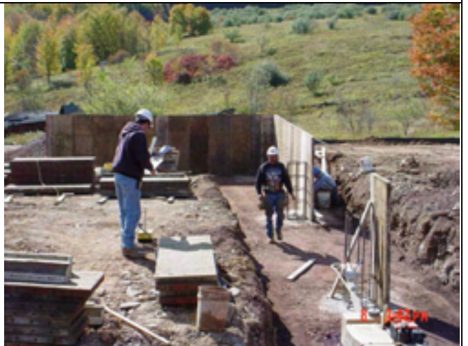
Picture No.: 036 Date Taken: October 8, 2002 Description: Forming grade wall.
