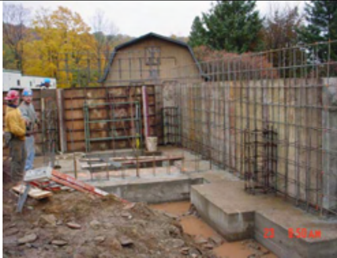
Picture No.: 075 Date Taken: October 23, 2002 Description: Installation of reinforcing steel for interior containment walls.
