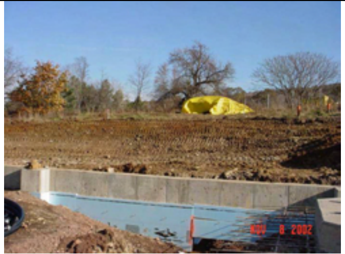
Picture No.: 111 Date Taken: November 8, 2002 Description: Rough grade along east side of GWTP.
