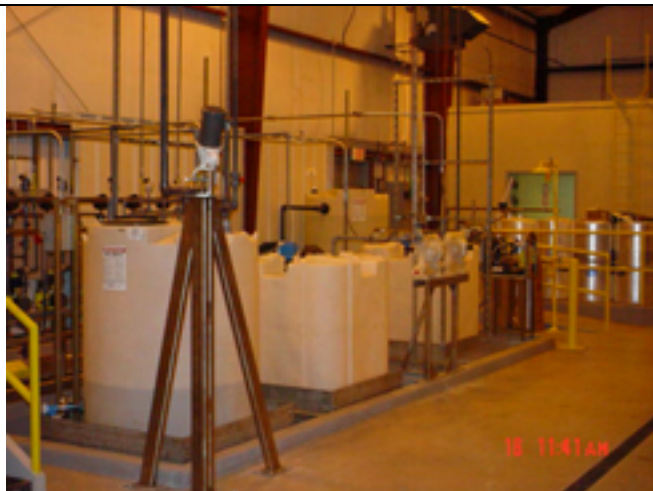
Picture No.: Date Taken: June 16, 2003 Description: Completed dilute acid, bulk acid, and bulk polymer tanks, pumps, mixers..
