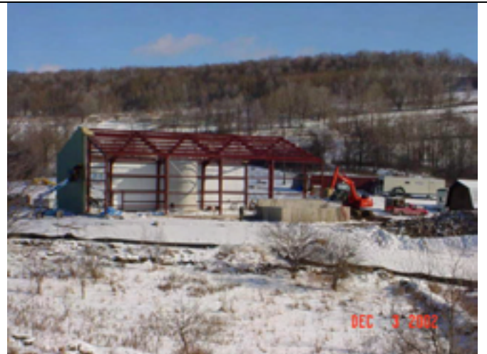
Picture No.: 152 Date Taken: December 3, 2002 Description: Looking east, GWTP building. Exterior wall panels/insulation complete on east side and mostly complete on north side.
