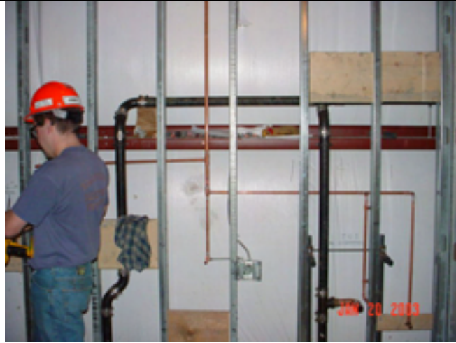
Picture No.: 226 Date Taken: January 20, 2003 Description: Mechanical piping and electrical conduit installation on east wall.
