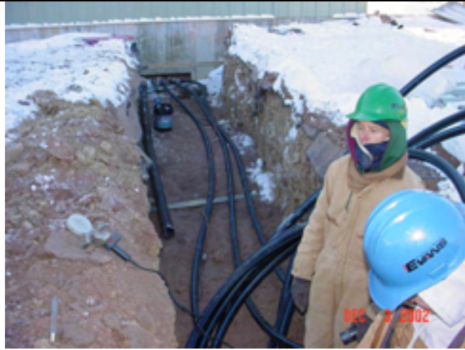
Picture No.: 153 Date Taken: December 3, 2002 Description: Trench excavation and groundwater piping installation on east side of GWTP.
