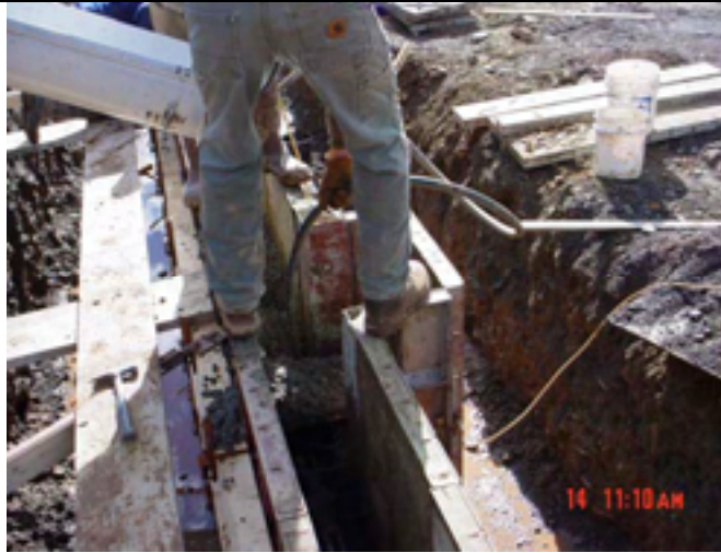
Picture No.: 053 Date Taken: October 14, 2002 Description: Placing concrete for grade wall.
