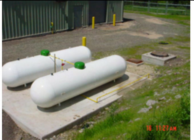
Picture No.: Date Taken: June 16, 2003 Description: Completed propane tanks, pad, piping, and Pullbox 7A&B.
