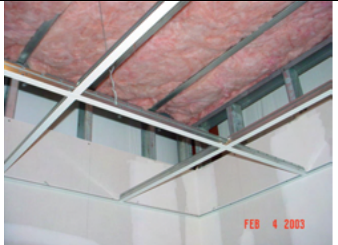
Picture No.: 244 Date Taken: February 4, 2003 Description: GWTP Office drywall, ceiling insulation, and drop ceiling panels.
