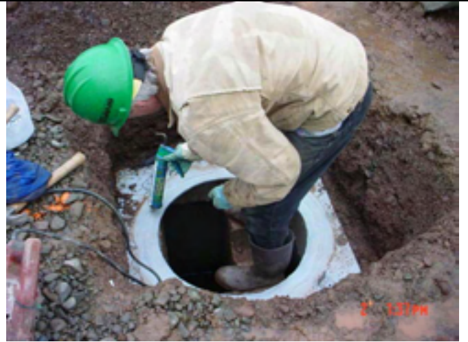
Picture No.: 364 Date Taken: May 2, 2003 Description: Sealing pullbox cover.
