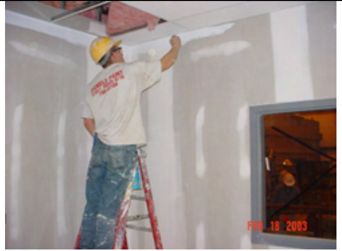
Picture No.: 256 Date Taken: February 18, 2003 Description: Spackling office walls.
