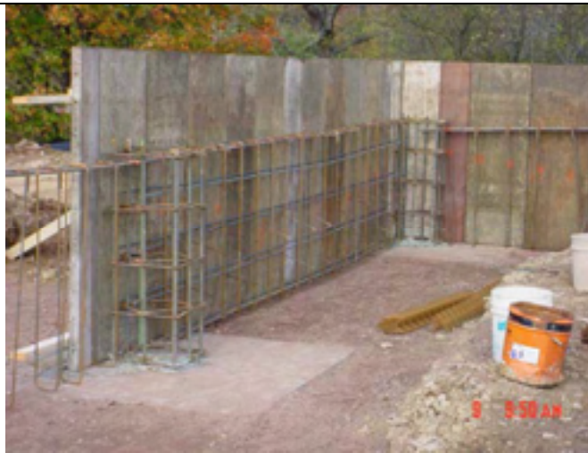
Picture No.: 039 Date Taken: October 9, 2002 Description: Reinforced steel for grade wall and columns.
