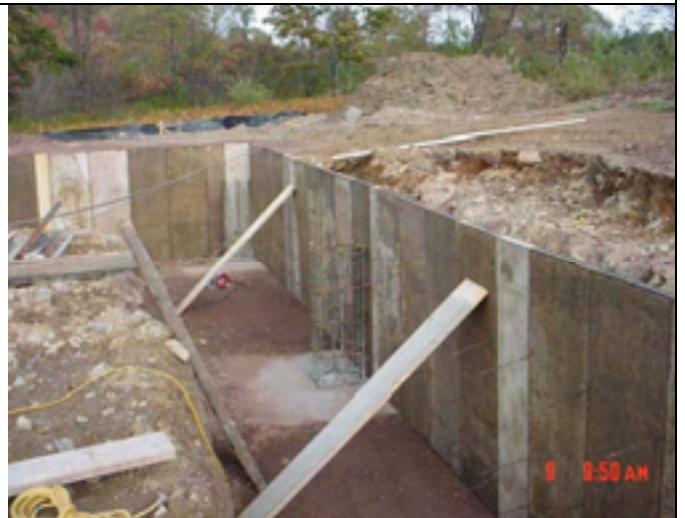
Picture No.: 040 Date Taken: October 9, 2002 Description: Forming grade wall.
