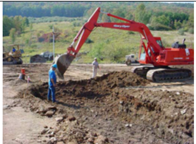
Picture No.: 020 Date Taken: October 1, 2002 Description: Continuous footer excavation.
