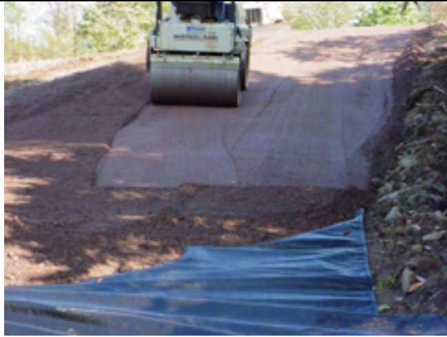
Picture No.: 013 Date Taken: September 30, 2002 Description: Compaction of Item #4 fill for access road.
