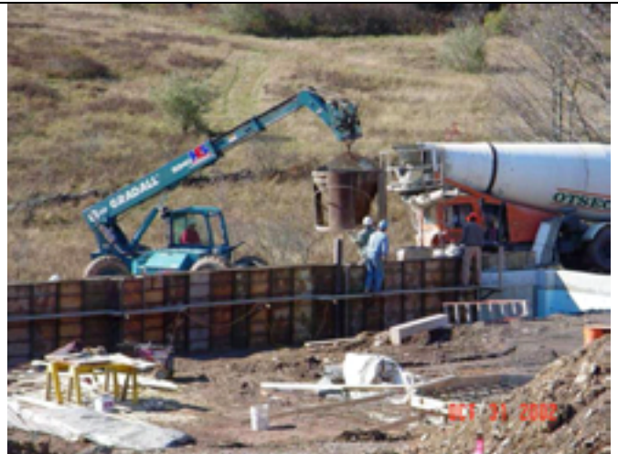
Picture No.: 099 Date Taken: October 31, 2002 Description: Looking west, containment wall concrete pour.
