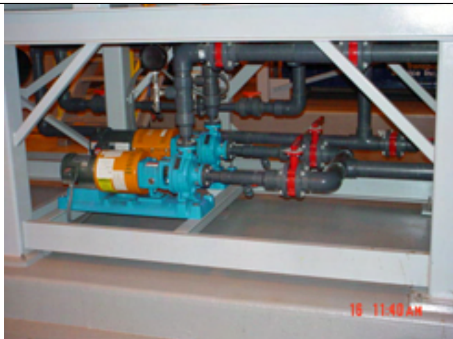
Picture No.: Date Taken: June 16, 2003 Description: Completed influent tank pumps (P1&P2).
