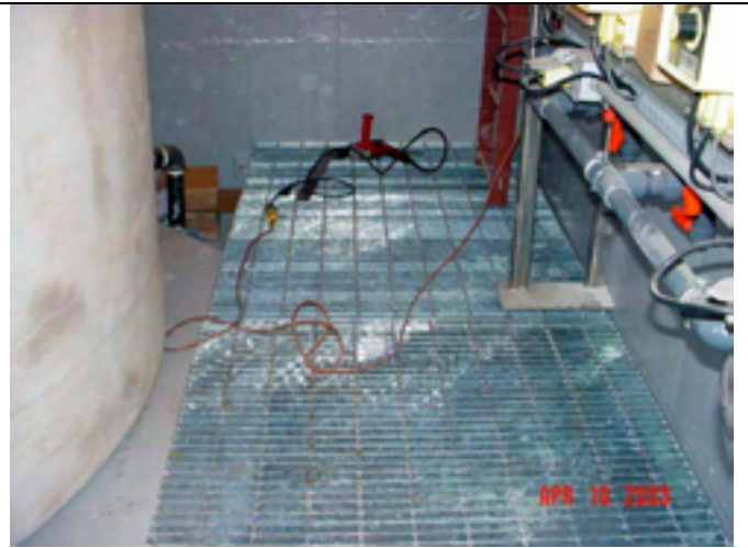
Picture No.: 309 Date Taken: April 10, 2003 Description: Caustic containment area grating.
