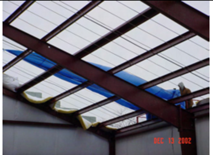
Picture No.: 173 Date Taken: December 13, 2002 Description: Temporary tarp covering GWTP roof.
