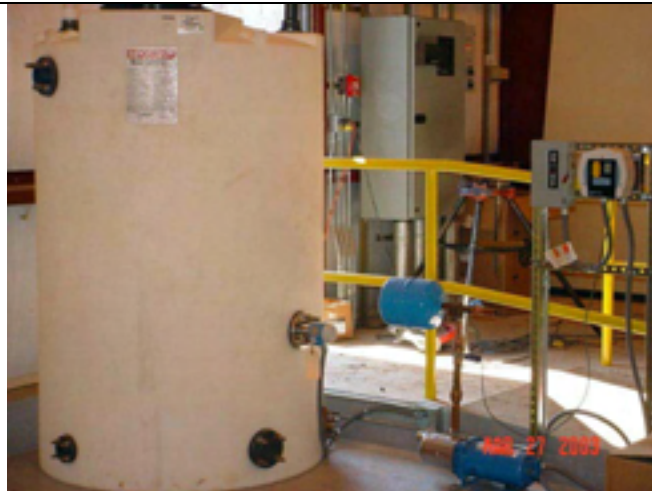
Picture No.: 292 Date Taken: March 27, 2003 Description: Potable Water tank and pump.
