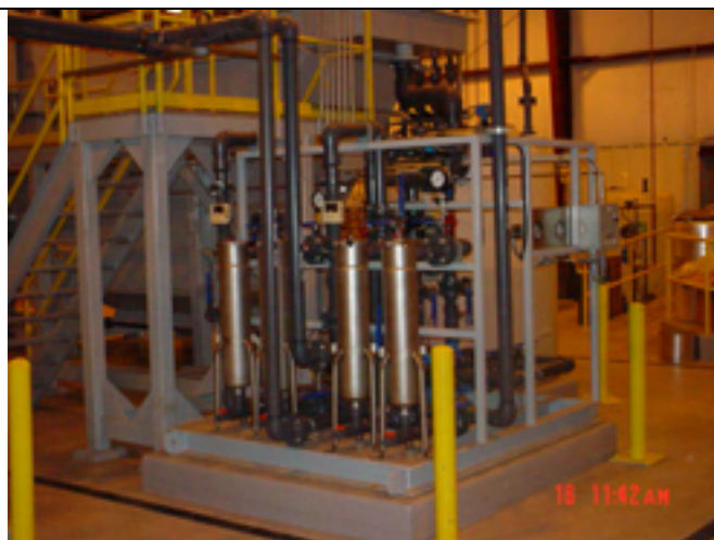
Picture No.: Date Taken: June 16, 2003 Description: Completed bag filter and pump skid.
