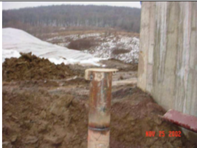
Picture No.: 139 Date Taken: November 25, 2002 Description: Observation Well 001 (OW1) cut and recapped for flush-mounting.
