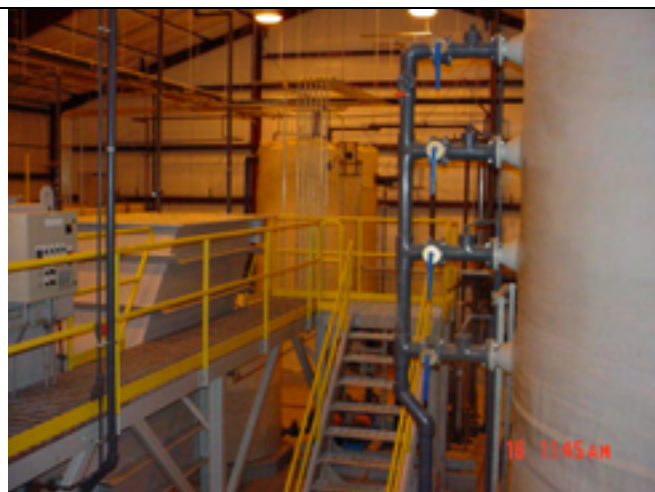
Picture No.: Date Taken: June 16, 2003 Description: Completed sludge tank (T-6) decant lines.
