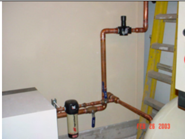
Picture No.: 267 Date Taken: February 26, 2003 Description: Air compressor bypass and dryer.
