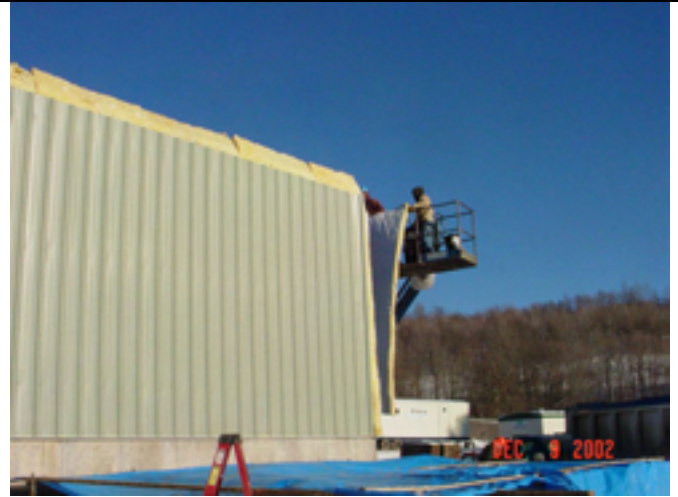
Picture No.: 162 Date Taken: December 9, 2002 Description: Installing exterior panels/insulation on south side of GWTP.
