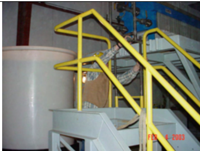
Picture No.: 245 Date Taken: February 4, 2003 Description: Installation of Filter Press stairs and railing. Pre-Coat Tank in background.
