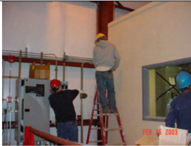
Picture No.: 262 Date Taken: February 25, 2003 Description: Wiring generator panel.
