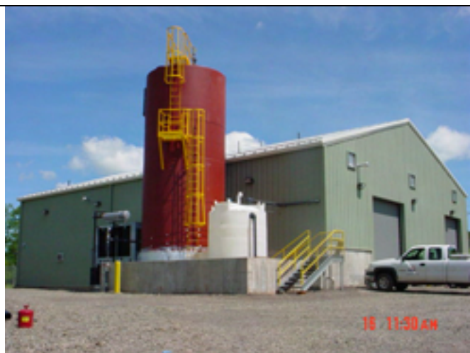
Picture No.: Date Taken: June 16, 2003 Description: Completed T-1 and T-16 (partial insulation on T-1).
