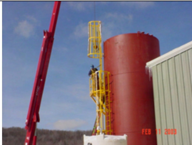
Picture No.: 251 Date Taken: February 11, 2003 Description: Equalization Tank (T-1) ladder installation.
