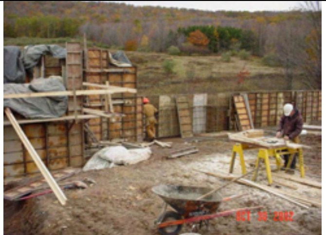
Picture No.: 094 Date Taken: October 30, 2002 Description: Looking west, forms for containment walls and grade beam.
