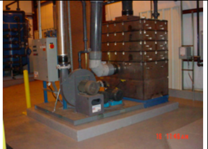
Picture No.: Date Taken: June 16, 2003 Description: .Completed air stripper skid.
