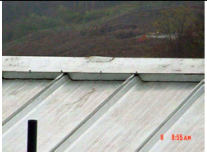
Picture No.: 385 Date Taken: May 8, 2003 Description: Roof ice breaker installation.
