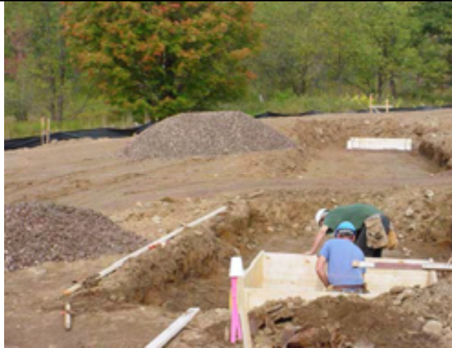
Picture No.: 021 Date Taken: October 2, 2002 Description: Footer form construction.
