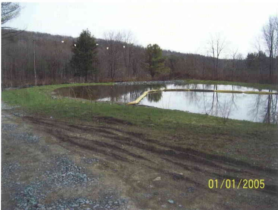
26. The existing stormwater detention basin near stream station 1+00 was converted to a micro-pool, greatly enhancing it's habitat value.
