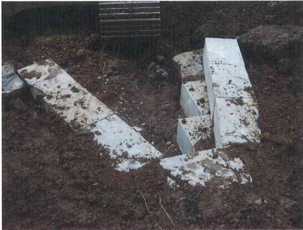
17. Step 11 - Constructed cross vanes were backfilled with soil and fine gravel.
