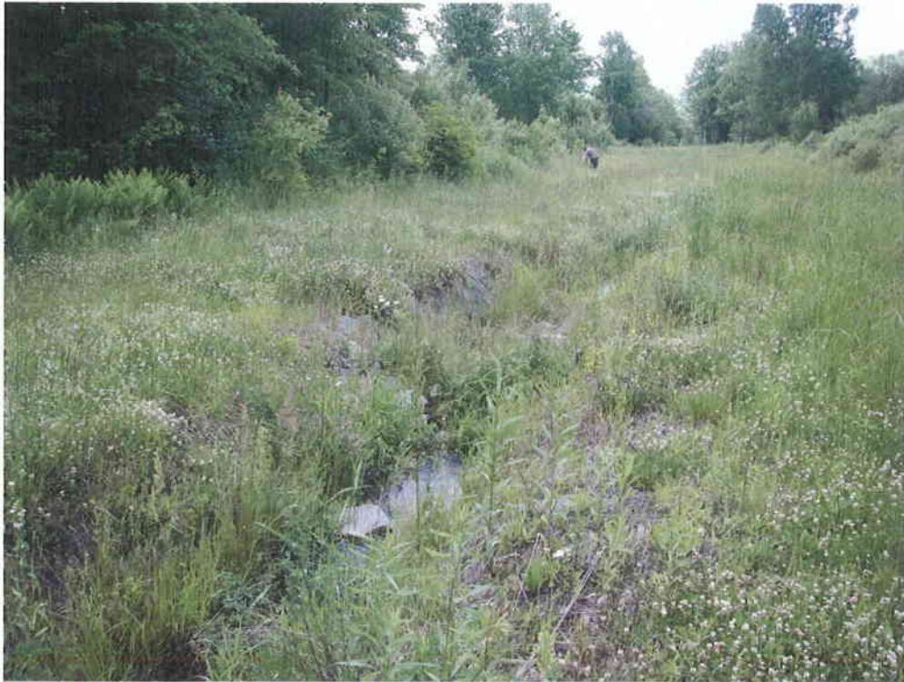
1. Pre-construction view of stream Segment I. The channel is straightened and incised as a result of impaired morphology and repeated storm events.
