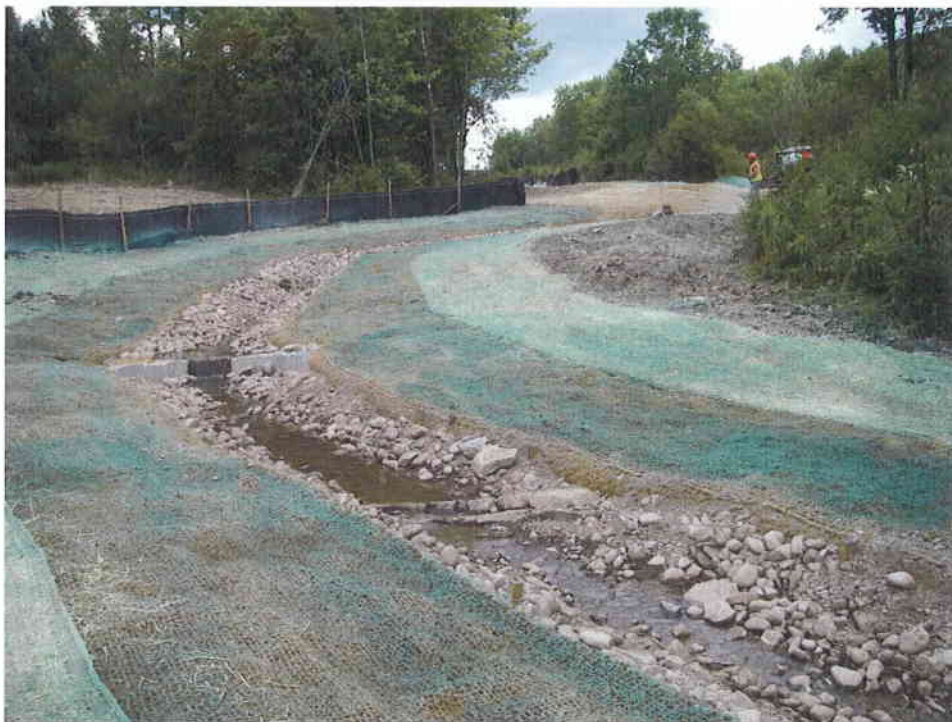
22. Step 16 - The finished portion of the stream channel was hydroseeded.
