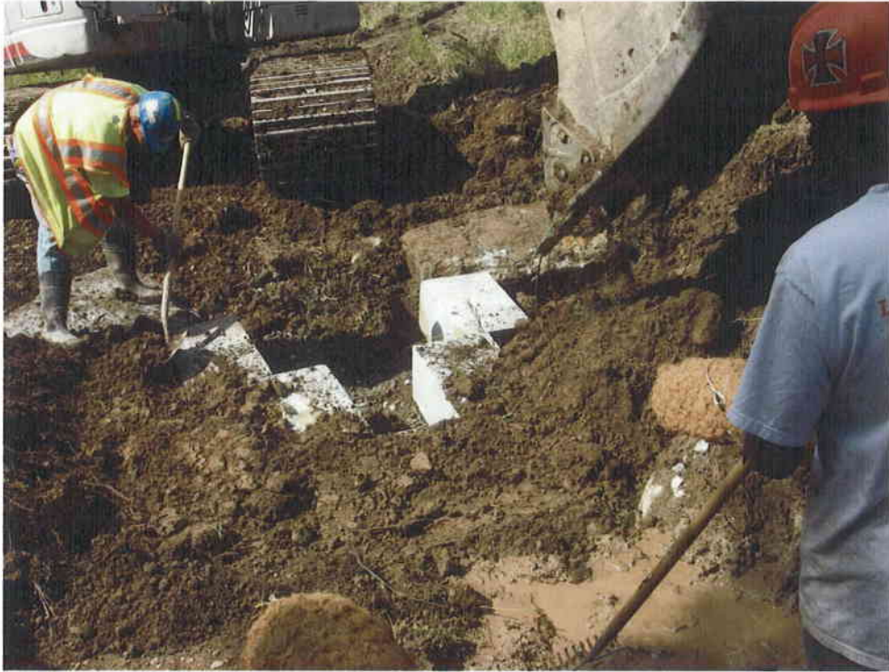
15. Step 9 - Footer rocks were placed and backfilled.
