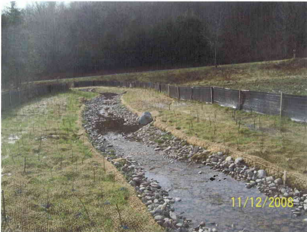
6. Post-construction view of stream Segment III. Increased bankfull cross-sectional area (derived from stable reference reach conditions) will allow for maintenance of flood flows without excessive sediment aggrading or channel braiding.
