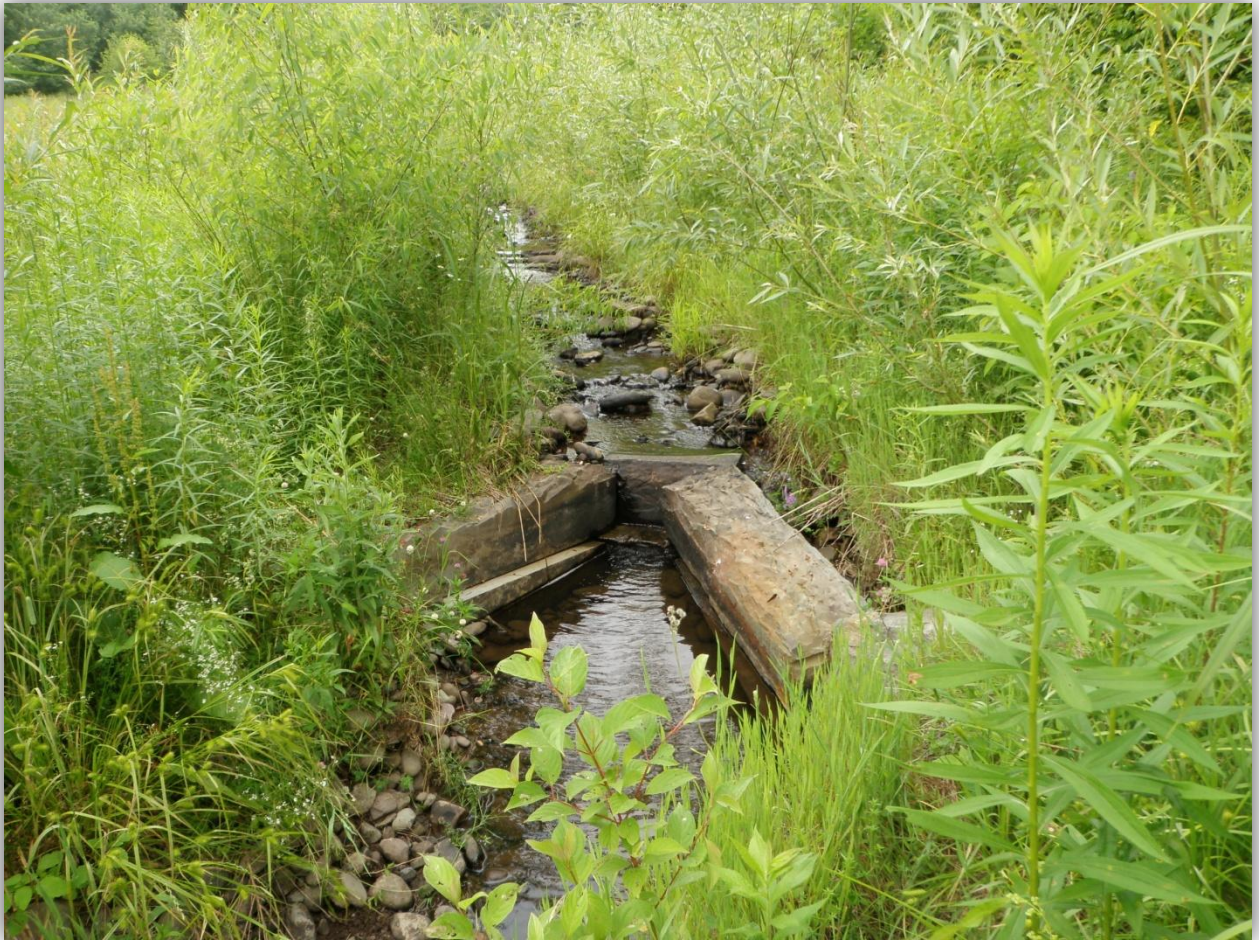
Figure 5. Sliding of left vane arm at Cross Vane #21, Station 13+58 (Segment II)
