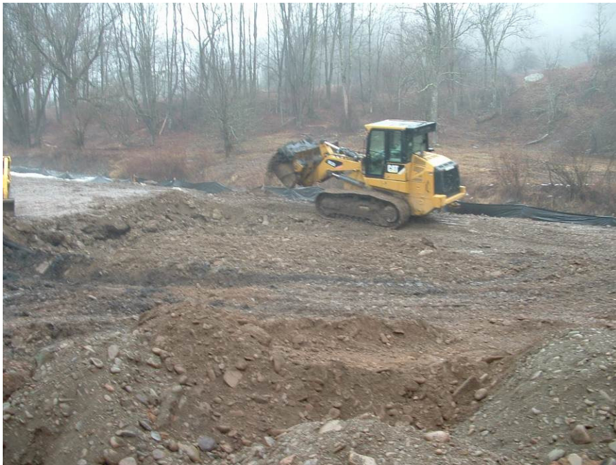
Photo 18: ERRS backfilled the excavation with imported pre-analyzed soil starting from the southeast portion of the Site.
