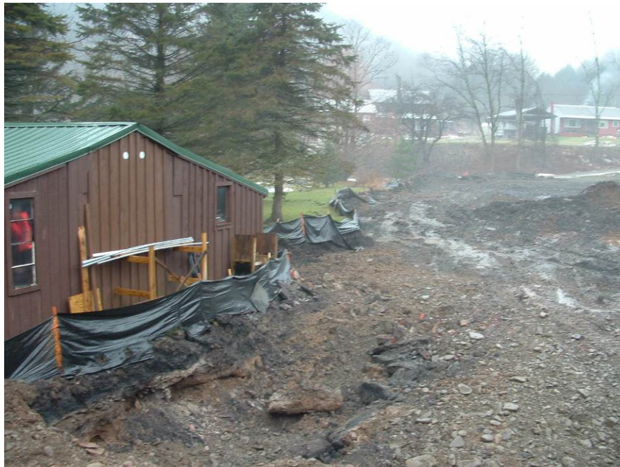
Photo 16: Grid-D1 along the southwest portion of the Site was excavated to approximately 24 inches bgs and tapered to the west and northwest direction to a depth of approximately 18 inches bgs at grid-J1. Although material suspected to be wood tar was observed to be progressing beneath the foundation of the property's garage, the excavation was terminated in this direction at the request of the property owner.
