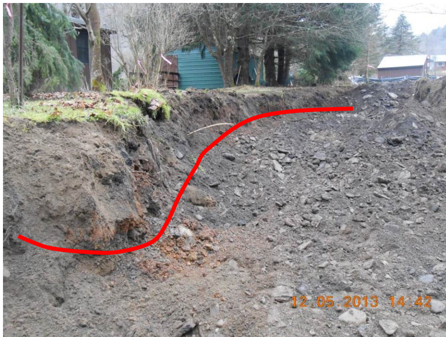
Photo 10: This southern portion of the Site encompassing all of grid-A1 and portions of grid-B1 was excavated to a depth of 4 feet bgs. The red line indicates the location where a layer of material suspected to be wood tar was observed to be progressing towards the foundation of on-site residential property.
