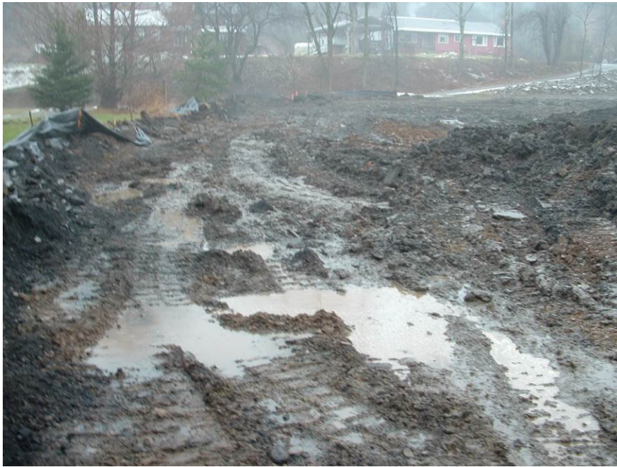
Photo 17: A view of the southwest portion of the Site after it was excavated to a depth of approximately 18 inches bgs along grid-F through grid-J.
