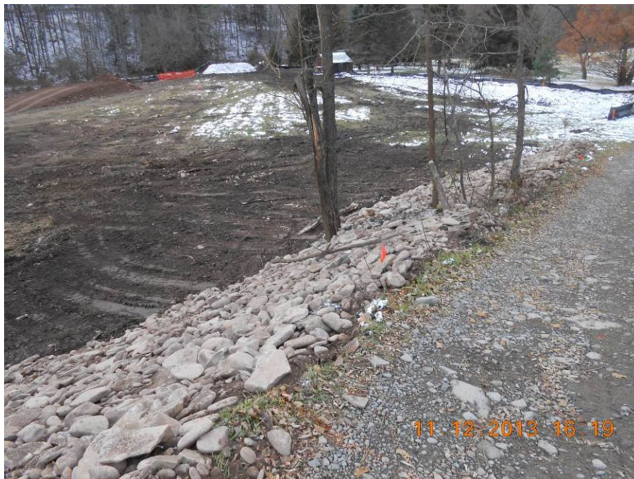
Photo 4: A northwest view of the Site looking south, before excavation activities commenced. ERRS placed large rocks and cobble stones along the sloped northwest area along Readburn Road to prevent erosion.
