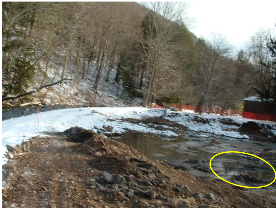
Photo 14: The yellow ellipse indicates the location within the excavation from where groundwater sample RW2-81GWAB was collected. This location encompassed groundwater that had seeped into grids A and B.
