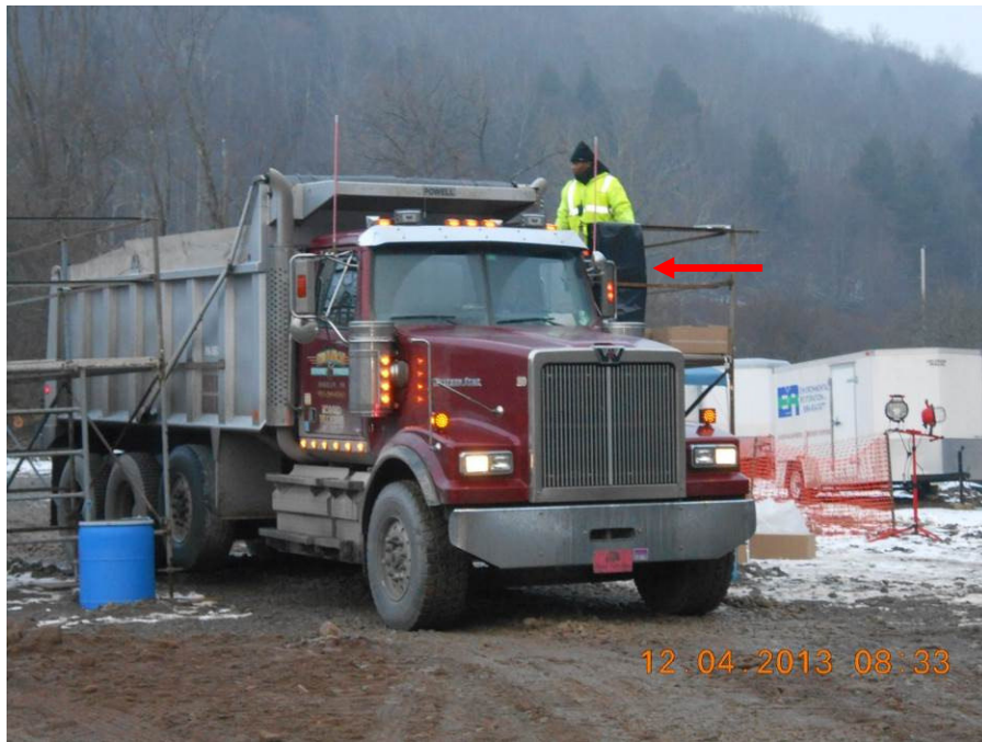
Photo 7: Trucks were lined with poly sheets (red arrow) before they were loaded with contaminated soils for off-site disposal.
