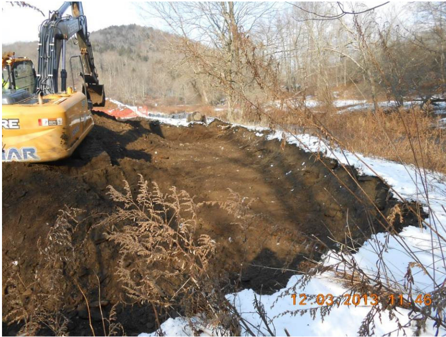
Photo 5: Excavation of wood tar-contaminated soils started from the southeast portion of the Site. The southeast sidewall was later removed completely. No sidewall sample was collected from this portion (grid AA2) of the excavation.
