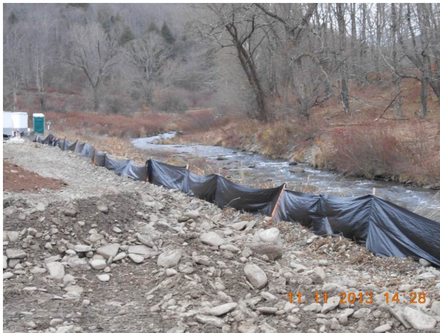
Photo 2: EPA's ERRS contractor established work zones and delineated the active work areas by installed silt fences along the proposed excavation boundaries of the Site. From this southeast portion of the Site, Read Creek can be seen east of the silt fence.
