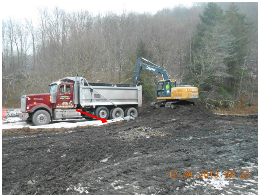
Photo 8: Poly sheets (red arrow) were placed along the truck access path to the soil loading area to prevent the vehicles from tracking contaminated soils offsite when exiting the Site.
