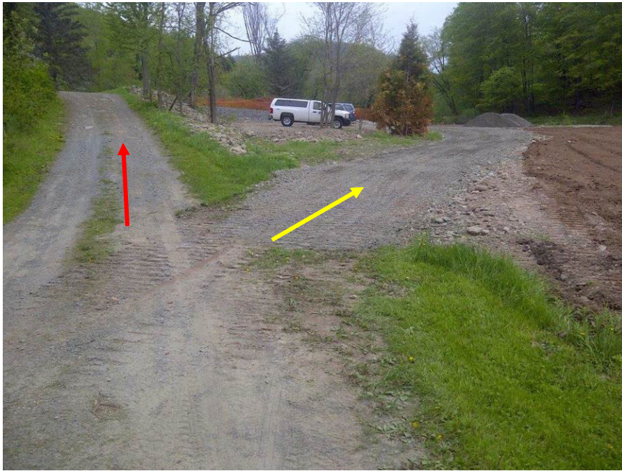
Photo 23: Approximately 66 tons of 2-inch crushed stones was repurposed from the Site's CRZ and trailer staging area and used in the construction of an alternative north driveway to the on-site residence. The red arrow indicates the old drive way and the yellow arrow indicates the new drive way.
