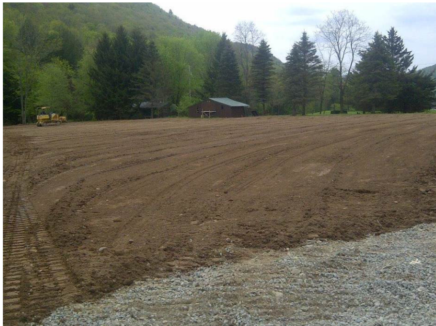
Photo 22: Approximately 900 tons of pre-analyzed top soil was placed throughout the approximately 65,000 ft 2 area of the Site, including the approximately 43,000 ft 2 excavation area, to a depth of 3 to 4 inches, thereby raising the ground surface to its original grade.
