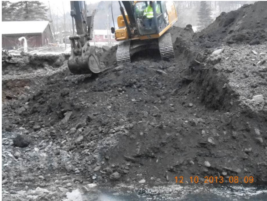
Photo 13: ERRS excavated portions of grid-B1 and all of grid-B2 to a depth of 8 feet bgs. Both grids were filled with large quantities of wood tar which were transferred directly to trucks for off-site disposal.
