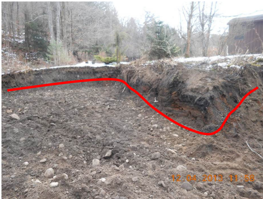
Photo 6: The red line indicates the depth, approximately 2 to 3 feet bgs, where material suspected to be wood tar was observed. This area was excavated southward to 4 feet bgs and eastward to 3 feet bgs.
