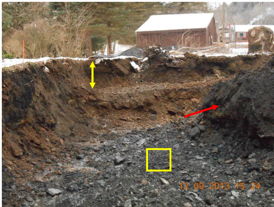
Photo 12: Large chunks of wood tar (red arrow) were excavated from grid-B1. Grid-C1 was excavated to 3 feet bgs (yellow arrow). The yellow square indicates the location where post excavation soil sample RW2-81-B1-08B was collected.
