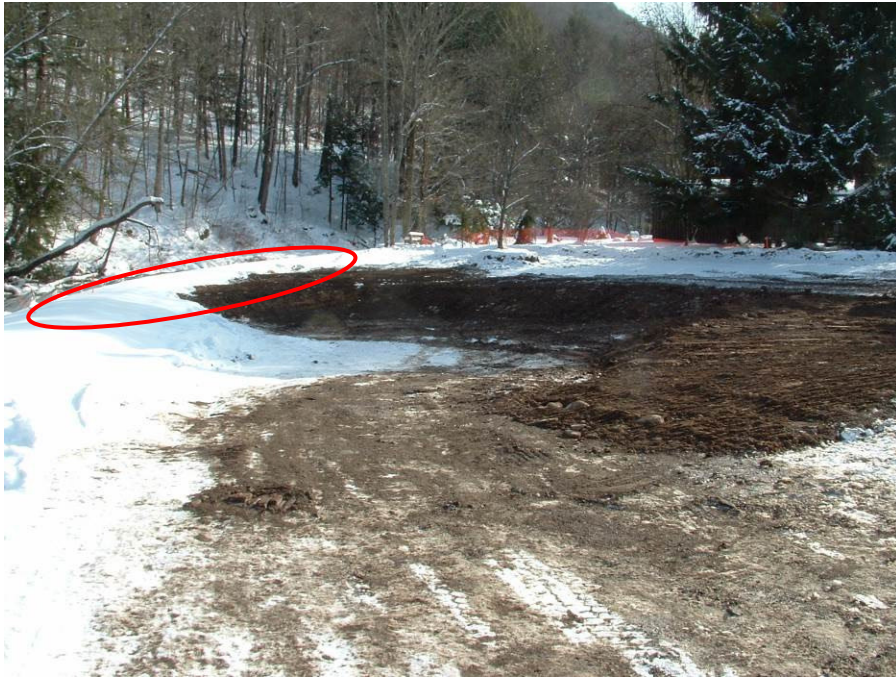
Photo 19: The west bank of the Creek which was completely removed during the excavation of the southeast portion of the Site was reconstructed with backfill material. The red ellipse shows portions of the west bank that was reconstructed.
