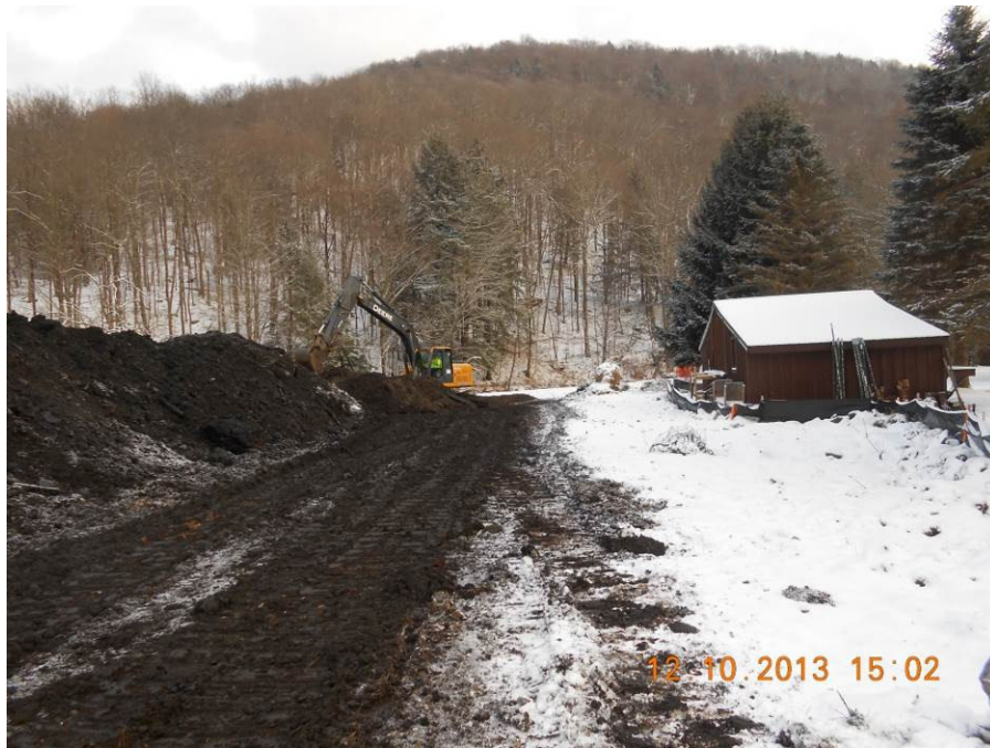
Photo 15: Wood tar-contaminated soils were staged onsite while waiting for trucks to arrive for loading and off-site disposal.
