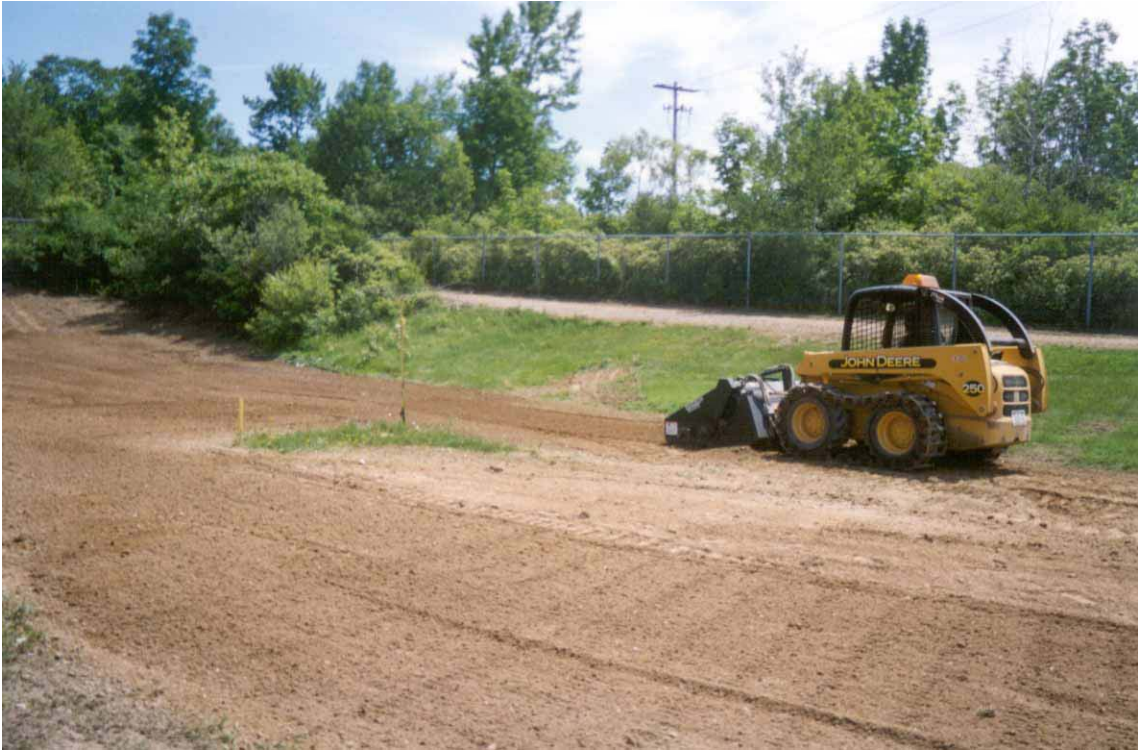
Topsoil Surface Preparation with Stone Rake
