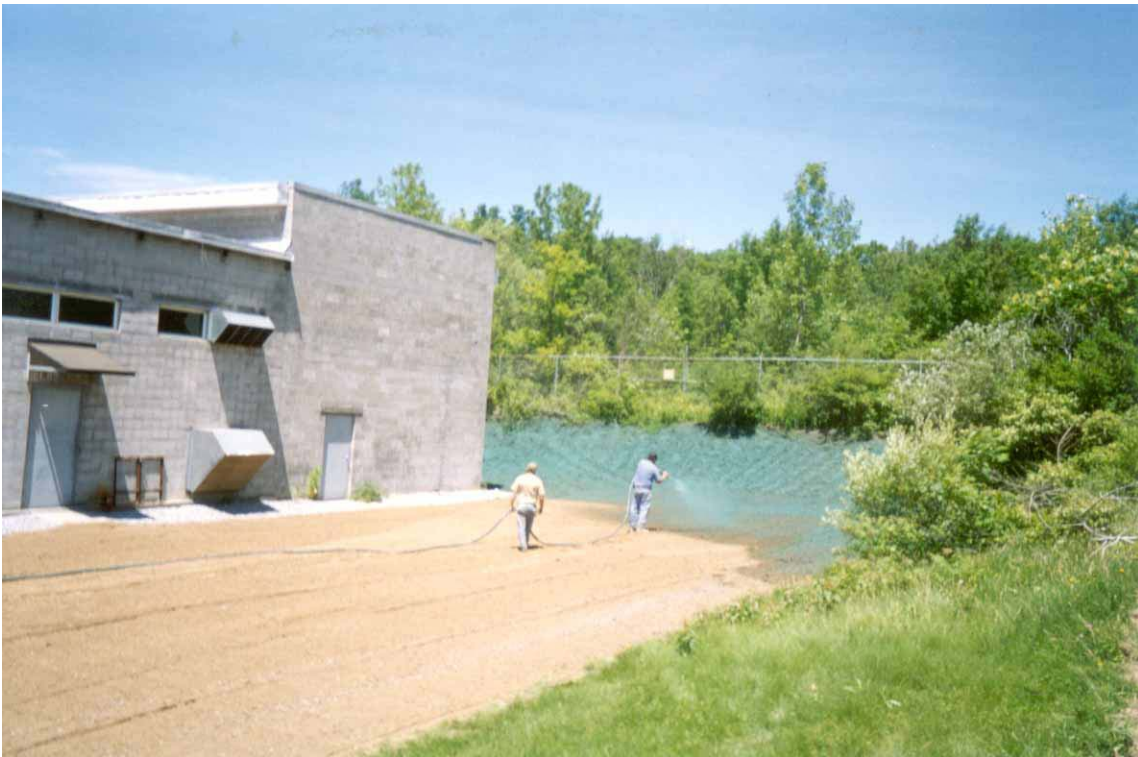
Placing Hydroseed on Finished Topsoil
