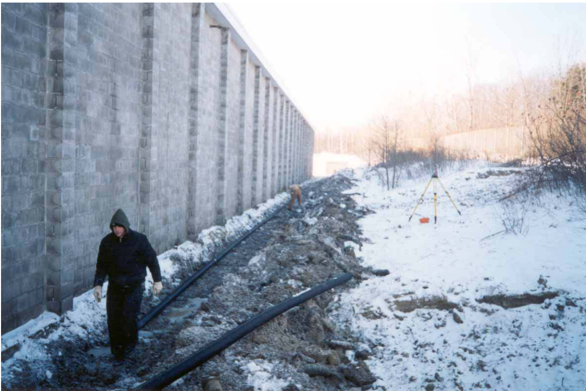
Drain Tile Placement Behind Building
