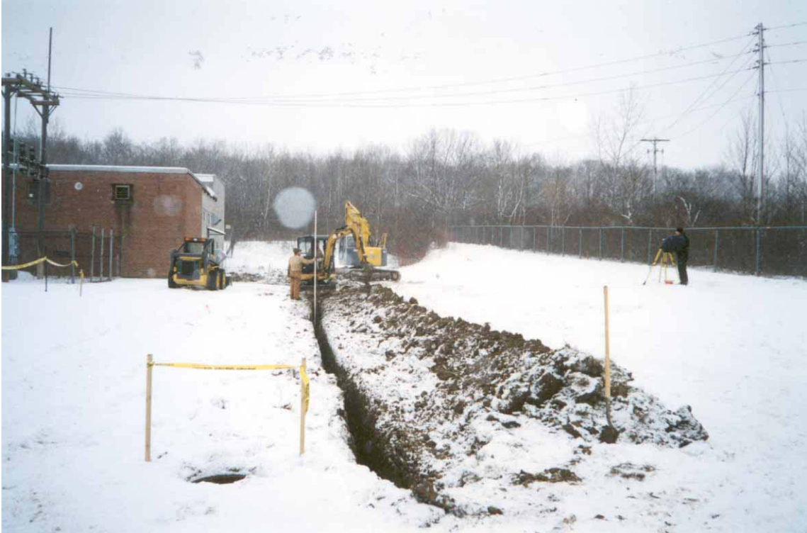
Trenching for Drain Tile
