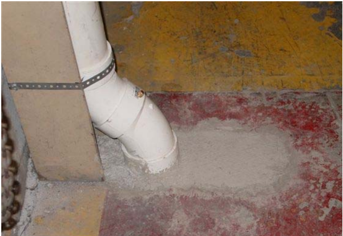
Photo 5: Typical Floor Penetration (note brass sample port plug)
