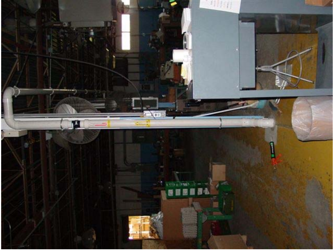
Photo 1: Typical Vent Riser with Labels, Flow Valve, Manometer
