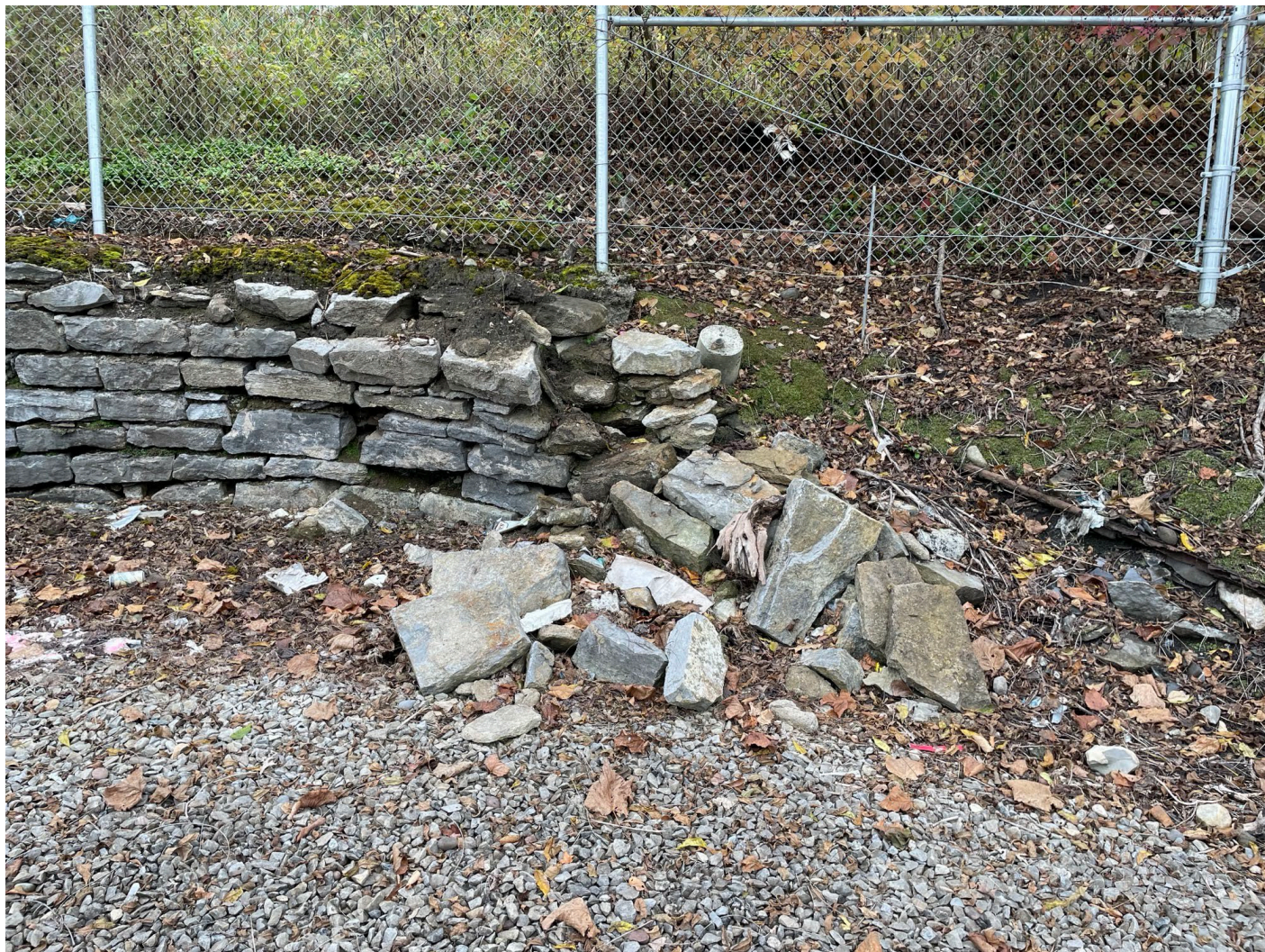
Damaged retaining wall, southern portion of substation
