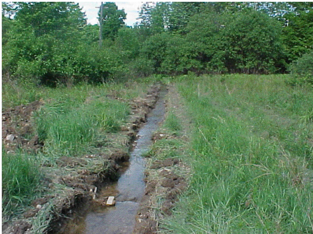
(Photo # 6-6-MVC-010F) June 6, 2001 – Construction of the passive temporary diversion ditch north of the NWDD. View toward the west.
