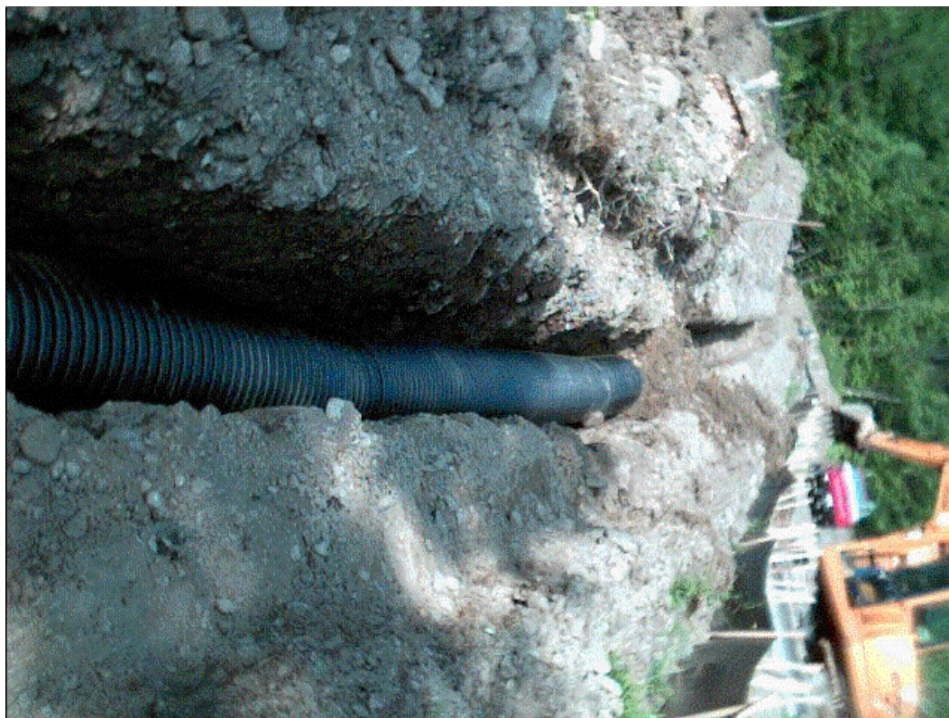
(Photo # 6-14-12) June 14, 2001 – Installation of piping in the temporary passive diversion ditch north of MRP. View toward the west.
