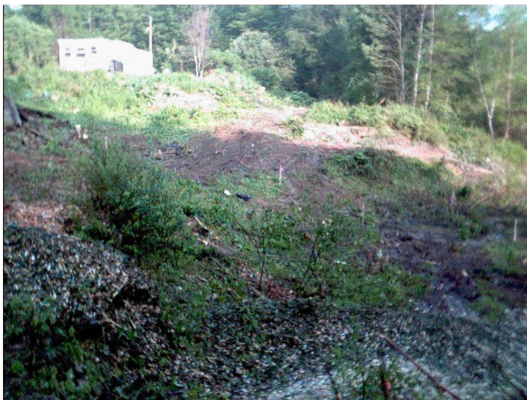
(Photo # 6-14-6) June 14, 2001 – Pre-excavation conditions at MRP Spoil Banks. Clearing and grubbing completed. Excavation limits surveyed and staked. View toward the west.
