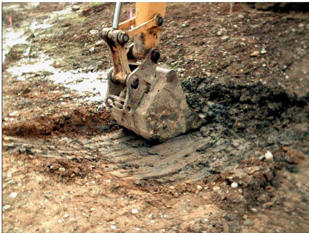
(Photo # 7-18-3) July 18, 2001 – Excavation of 1 foot of material from a 6-foot by 6-foot area in NWDD to address NYSDEC post-excavation sampling results.
