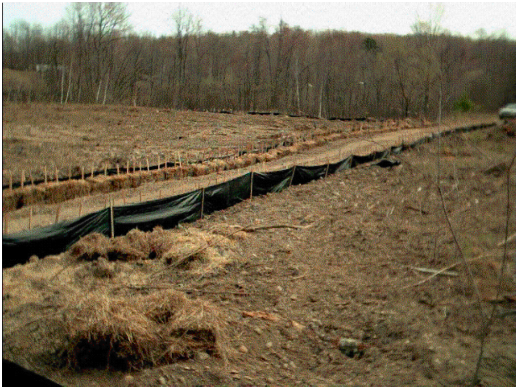
(Photo # 4-23-5) April 23, 2001 – Staging area after clearing and grubbing and silt fencing was installed. View toward the northeast.
