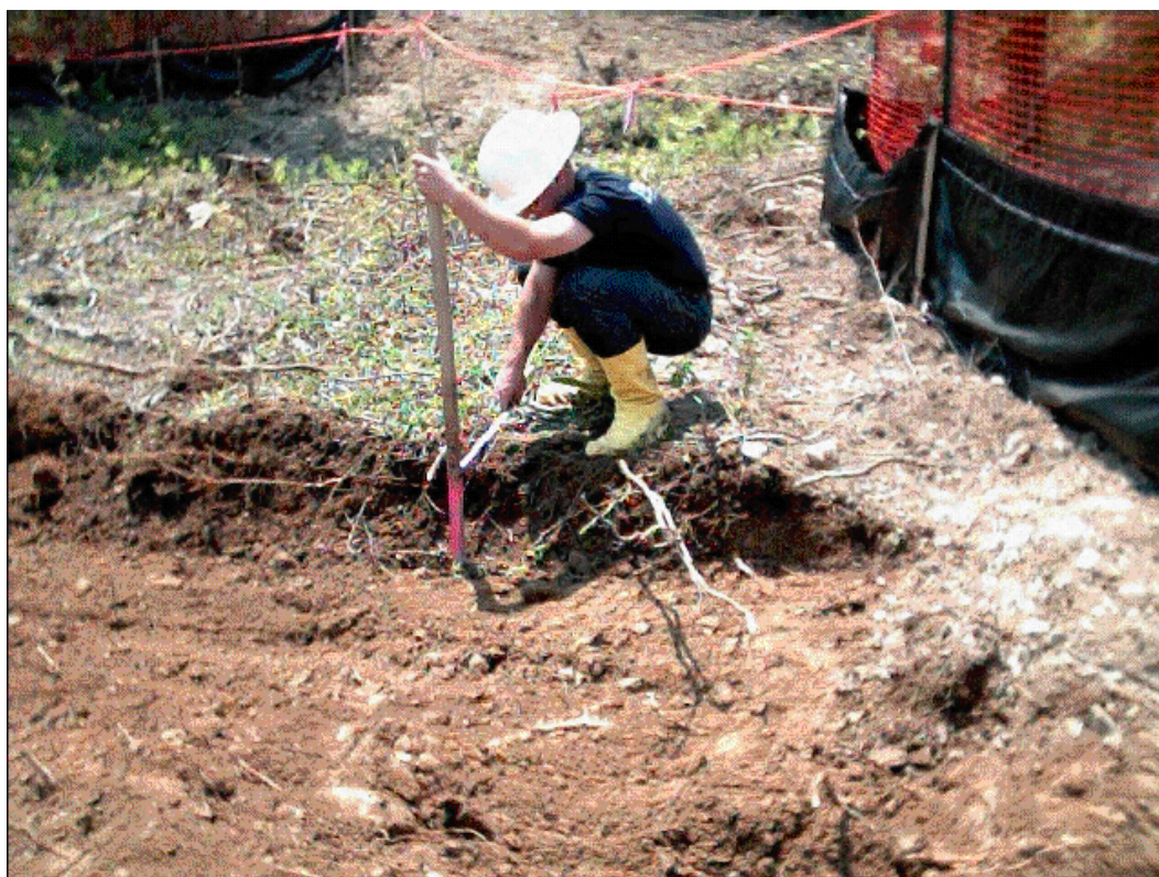
(Photo # 6-20-5) June 20, 2001 – Real-time verification of a one foot excavation in the east end of the NWDD.
