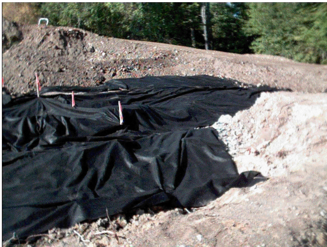
(Photo # 9-19-3) September 19, 2001 – Installation of a geotextile to act as a marking layer in the base of excavations. View toward the southwest.
