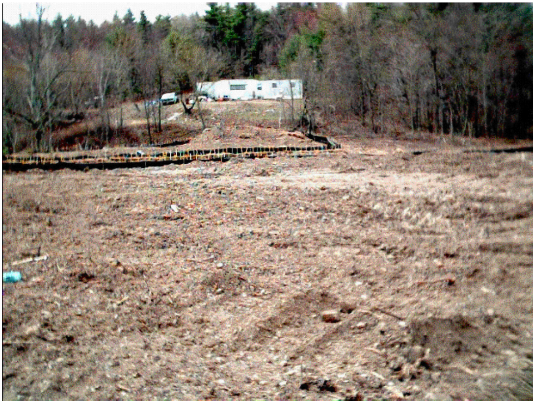
(Photo # 4-23-13) April 23, 2001 – Staging area and MRP Spoil Banks after clearing and grubbing and silt fencing was installed. Original location of house trailer on the Spoil Banks. View toward the south.
