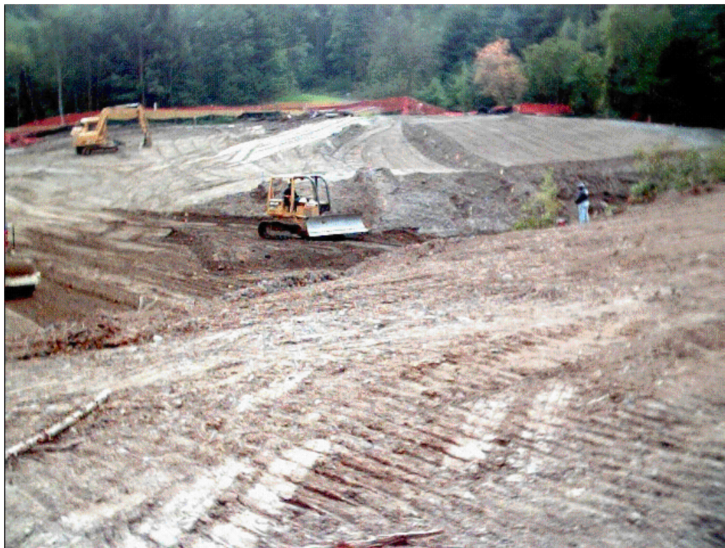
(Photo # 9-24-2) September 24, 2001 – Backfilling MRP and MRP Spoil Banks. View toward the southwest.
