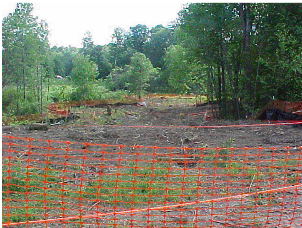
(Photo # 6-6-MVC-004F) June 6, 2001 – Clearing and grubbing completed at the NWDD; silt and construction fencing installed; excavation limits surveyed, staked, and marked with a string line. View toward the northeast.
