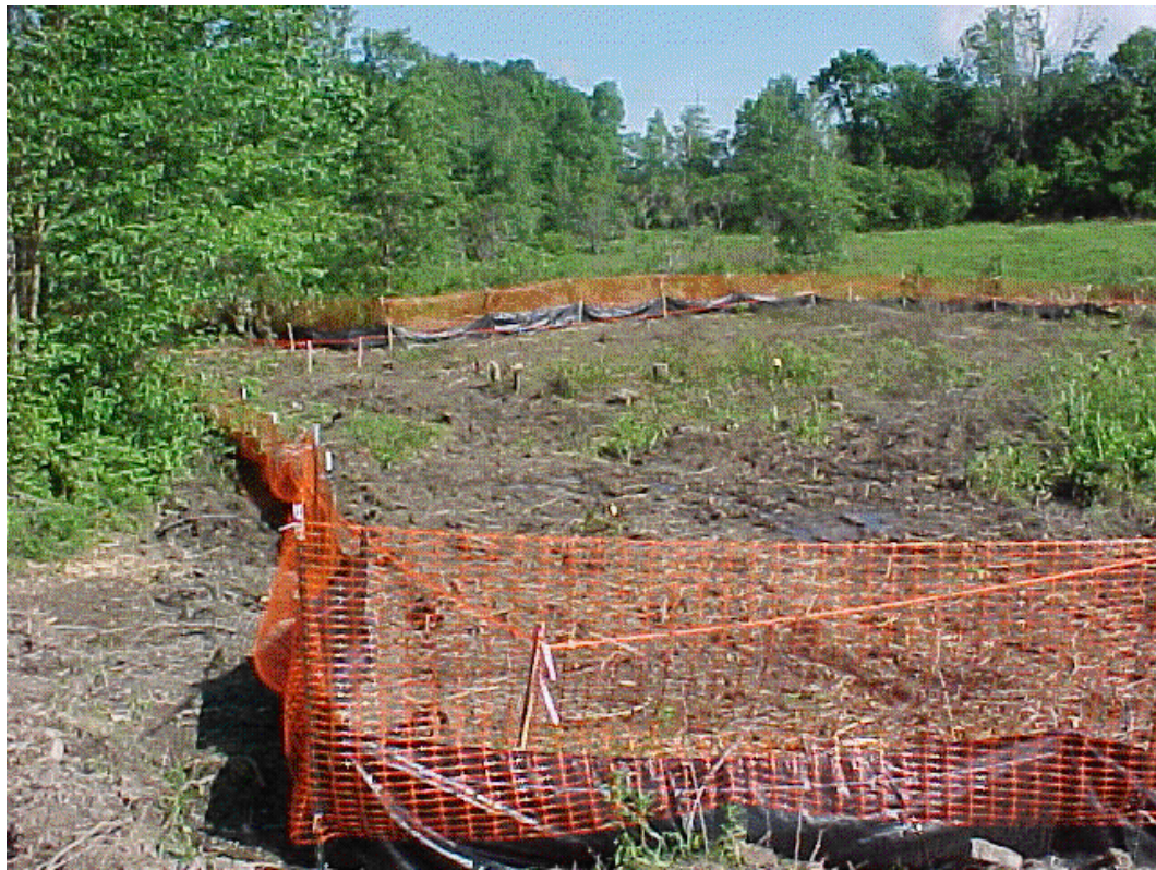
(Photo # 6-6-MVC-005F) June 6, 2001 – Clearing and grubbing completed at the NWDD; silt and construction fencing installed; excavation limits surveyed, staked, and marked with a string line. View toward the southeast.
