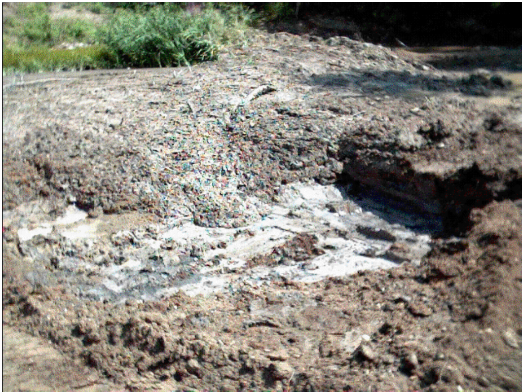
(Photo # 8-14-7) August 14, 2001 – Excavation of MRP upper soft materials to the underlying clay layer. View toward the northeast.
