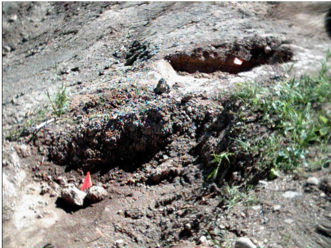
(Photo # 9-5-4) September 5, 2001 – Excavations of from 6-foot by 6-foot areas on the MRP Spoil Banks to address NYSDEC post-excavation soil sampling results.
