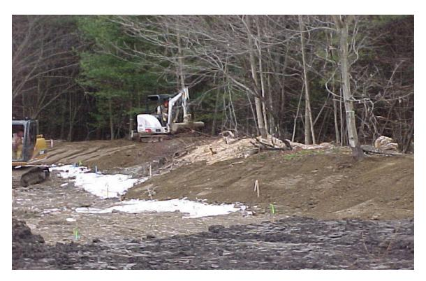
December 5, 2003 – Northwestern View; SLC installed topsoil on bank above wetland for soft armor and installation in the area of polygons NA-62, NA-70, NA-61, and NA-66
