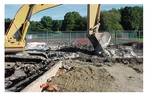
October 7, 2003 – Eastern View: SLC mixing lime with material on MSDP for stabilization purposes (Lime proved to be an inadequate stabilizing material and after this photograph was taken, cement kiln dust successfully replaced lime as the stabilization material)
