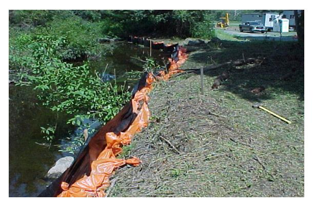
August 20, 2003 – Northern View: Silt fence anchored with sand bags
