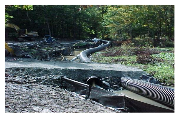
October 2, 2003 – Southwestern View; SLC completed installation of the temporary access road extending across the Valatie Kill for access to NA polygons
