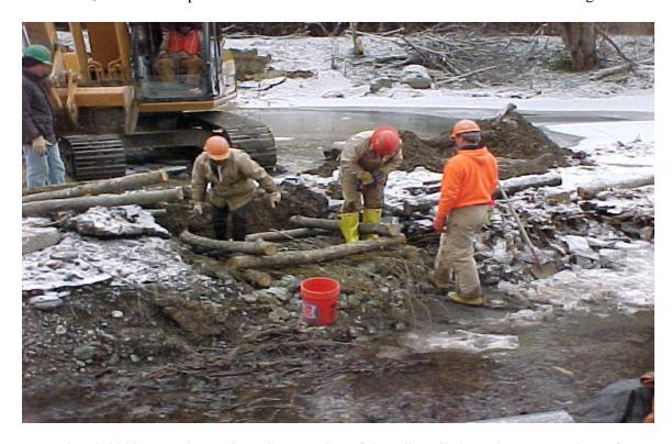
December 4, 2003 – Northern View; Construction of the crib wall along the eastern edges of polygons NA-71 and NA-78 and along the western edges of polygons SB-47 and SB-48
