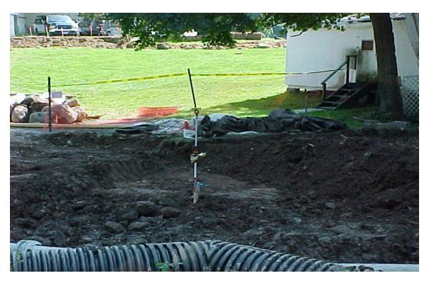
September 10, 2003 – Northeastern View: Excavation of polygon SA-97 with a confirmatory sample point in the center
