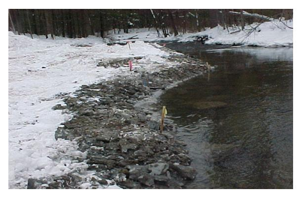
December 10, 2003 – Western View; SLC completed installation of hard armor on the eastern bank at downstream end of Area 28 along polygon NA-75
