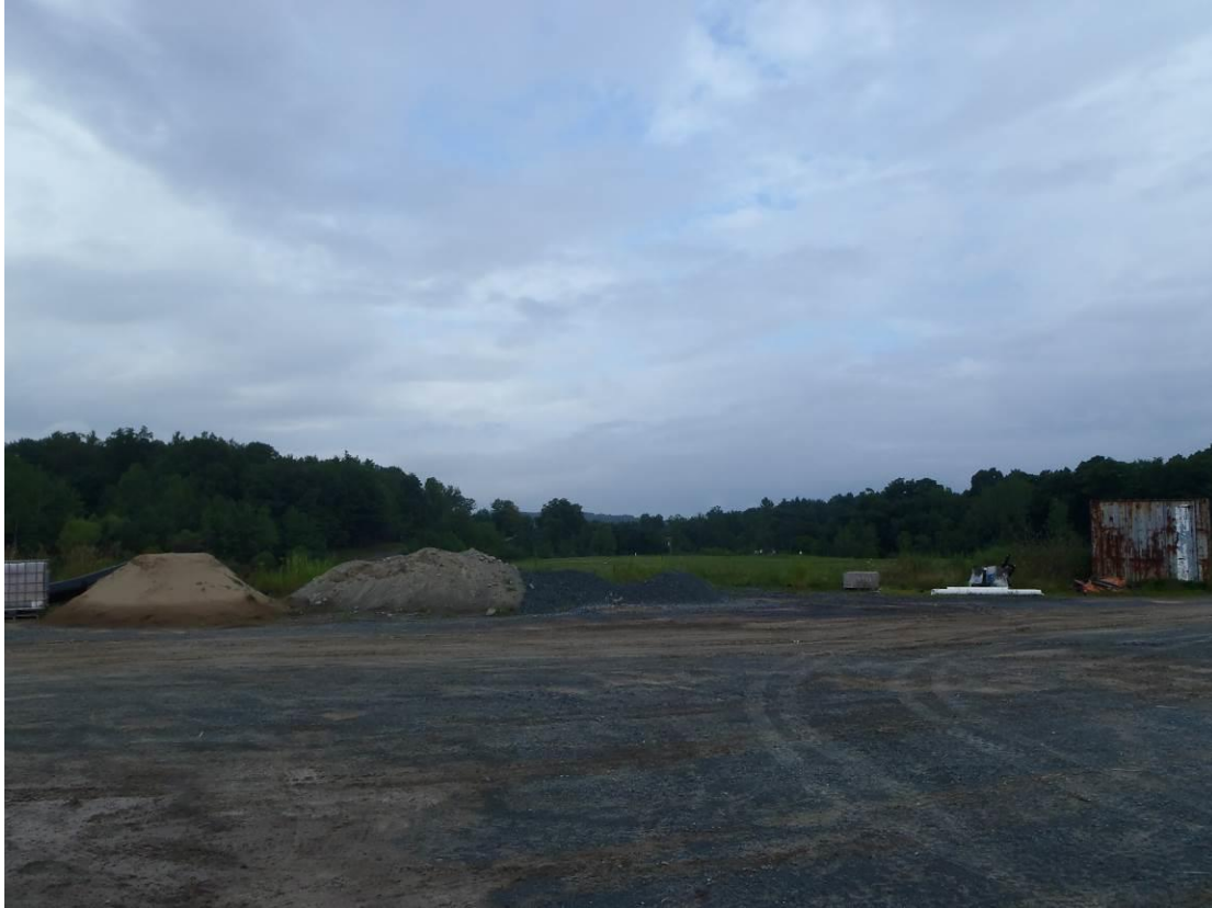
Photo 1. View northwest across capped Landfill.
