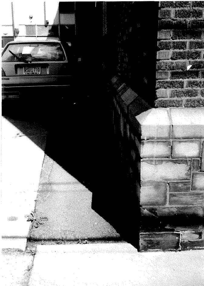
A2. SOUTHEAST WALL OF MAIN BUILDING.
