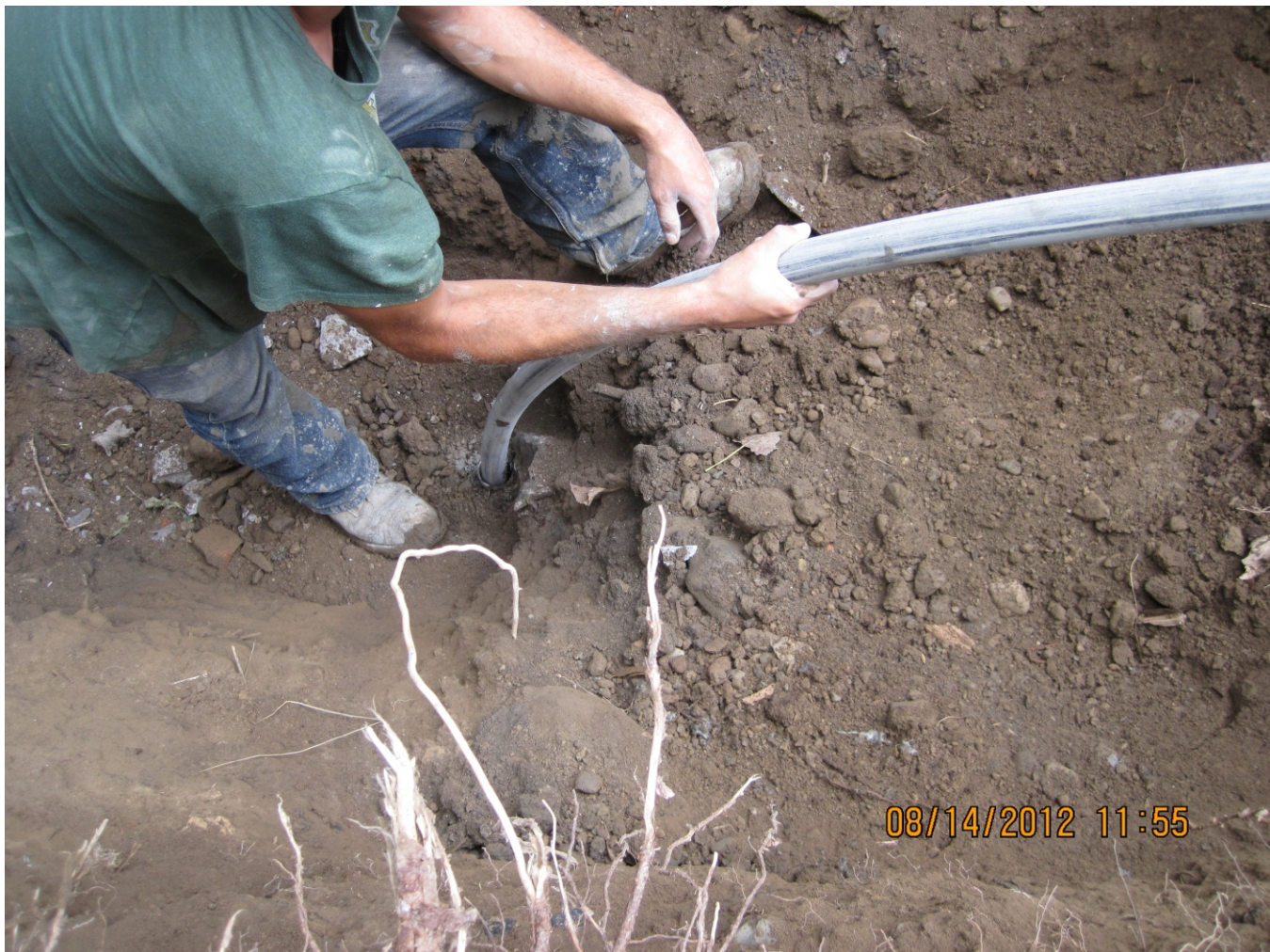
Tremie line installed in 2" well
