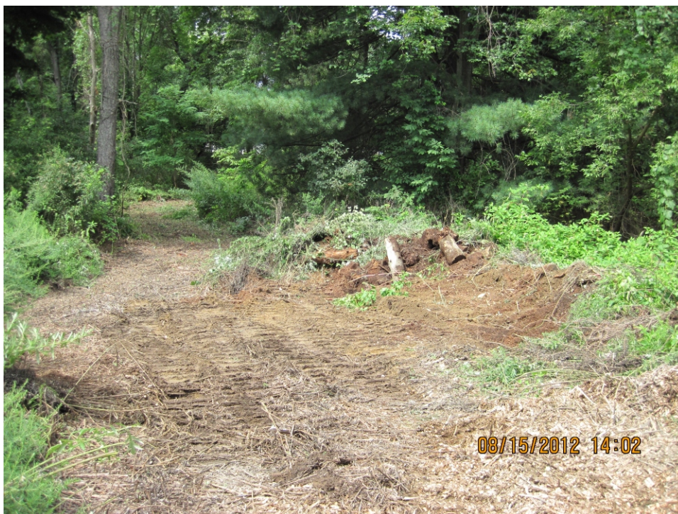
Backfilled and graded well locations
