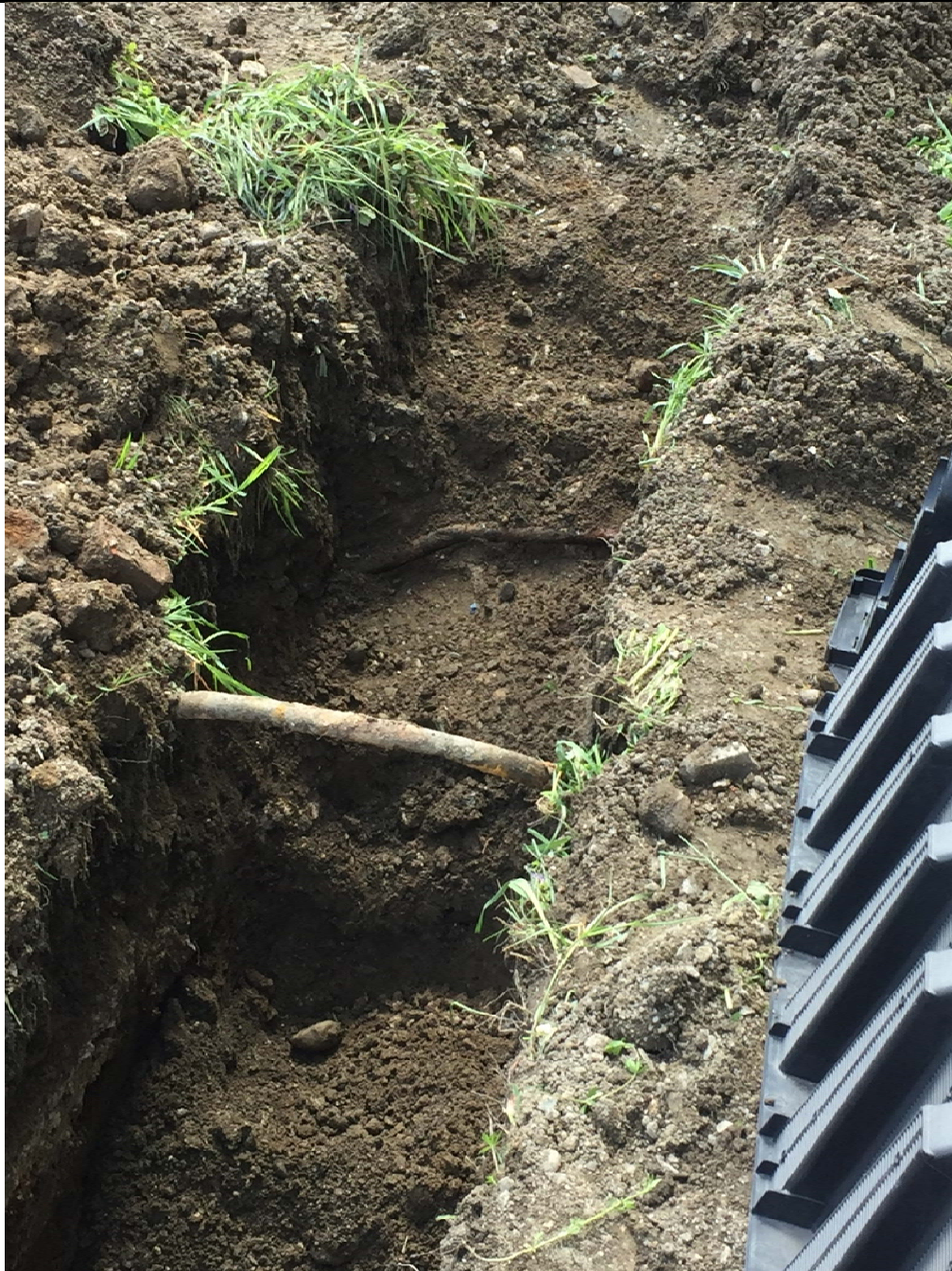
Two former gas lines encountered during trenching
