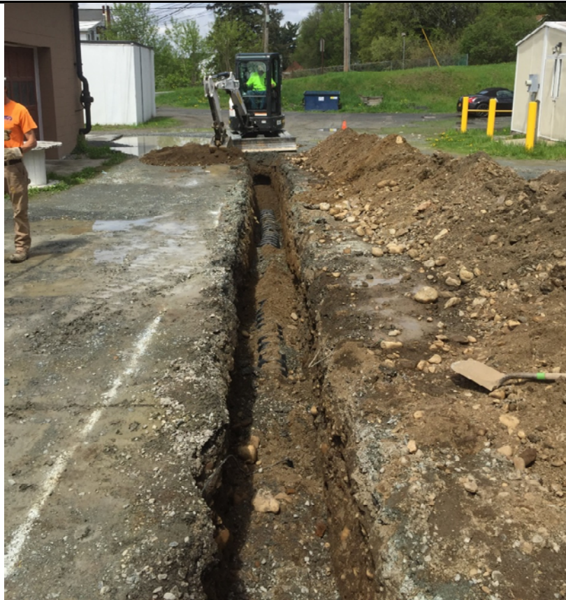
Final bio-diffuser installed in injection trench on the northeast side of the building
