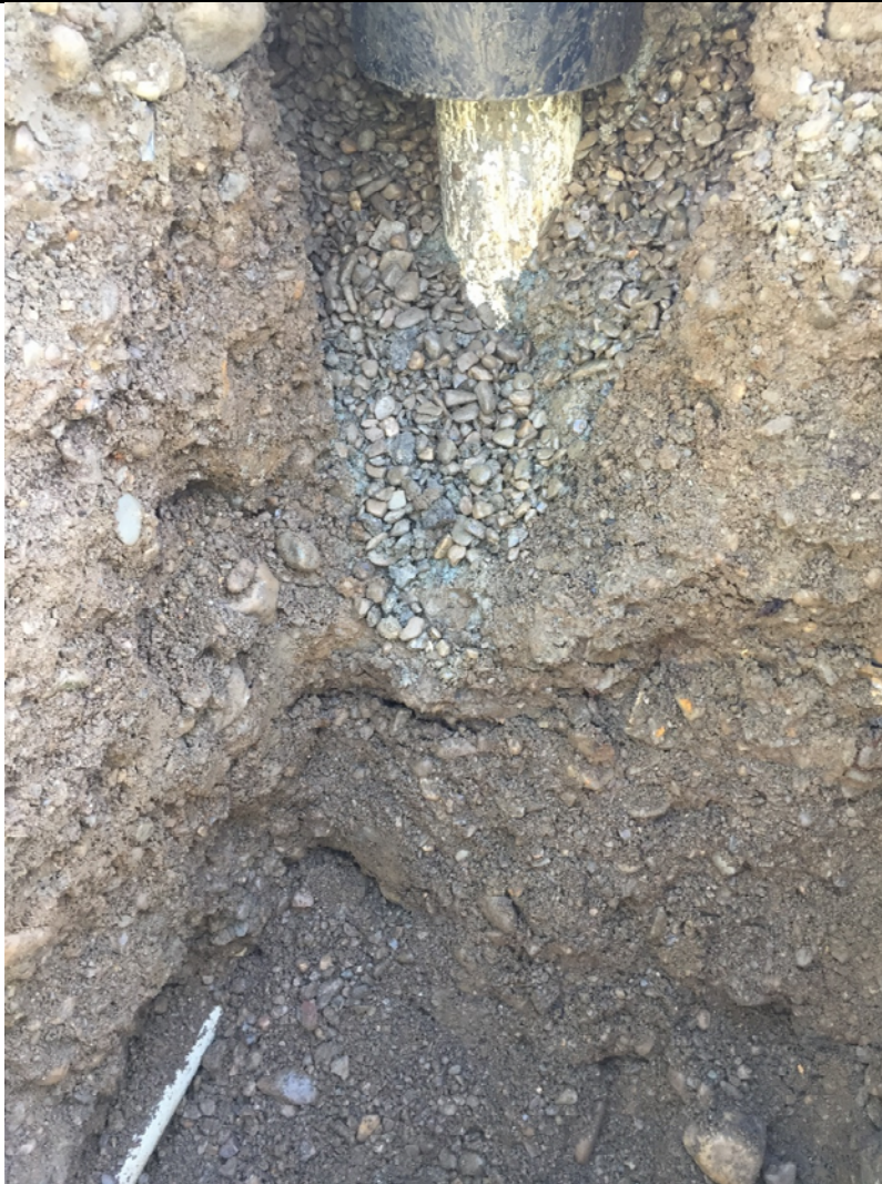
Damaged PVC transducer line located next to well INJ-3 located 3' below grade
