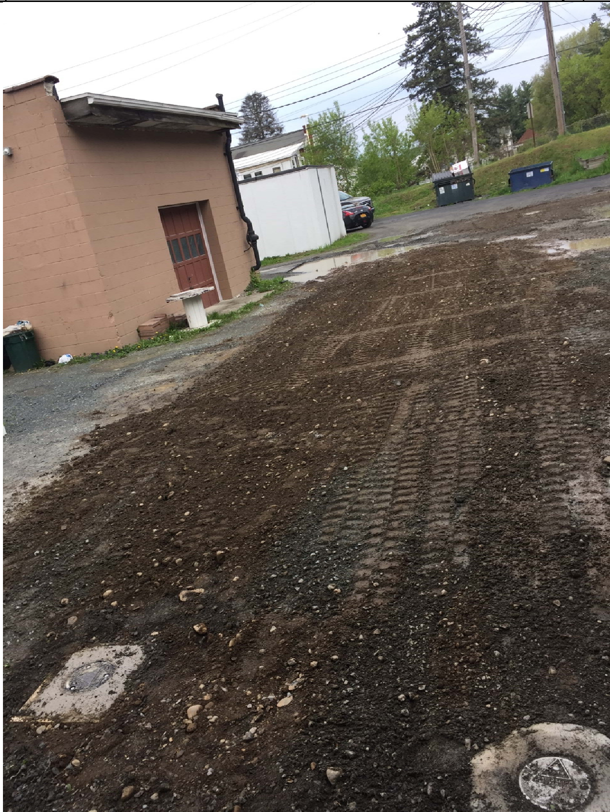
Final grade of trench on the northeast side of the building as well as where transducer line was repaired near well INJ-3
