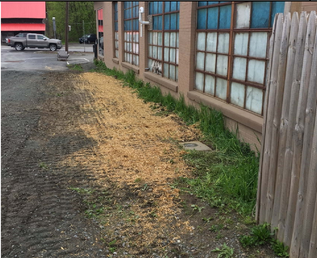
2" of straw spread over the location of the trench on the southeast side of the building where grass was disturbed
