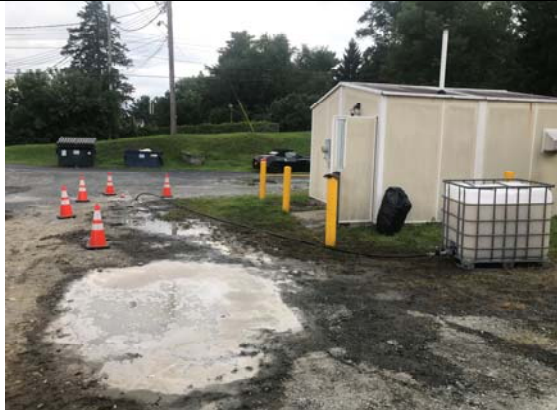
Injections at INJ-3 via gravity feed with packer
