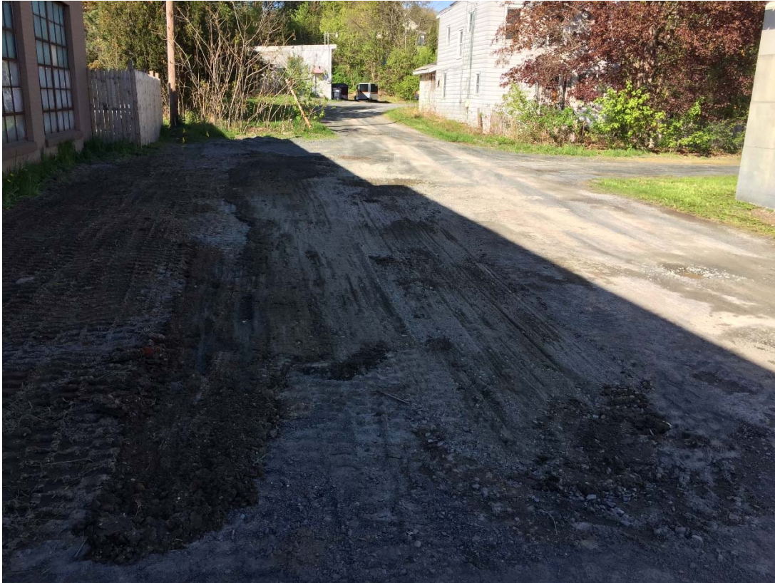
Final grade of trench and driveway to cleaned up tracks from the excavator
