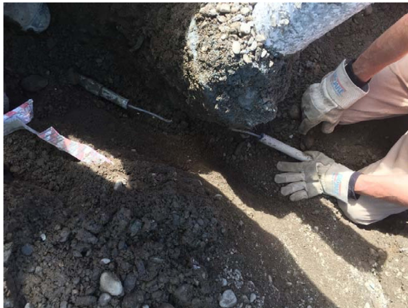
Location of damaged line located, approximately 18' of PVC line was repaired
