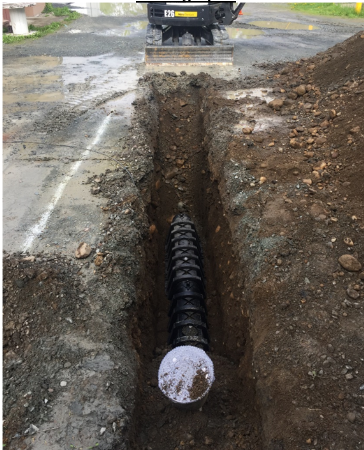
First bio-diffuser installed in injection trench on the northeast side of the building
