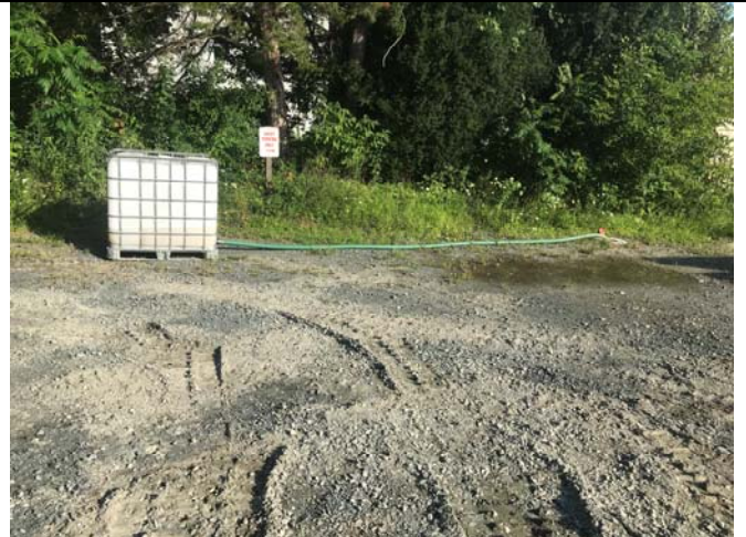
Injection at INJ-1 via gravity feed
