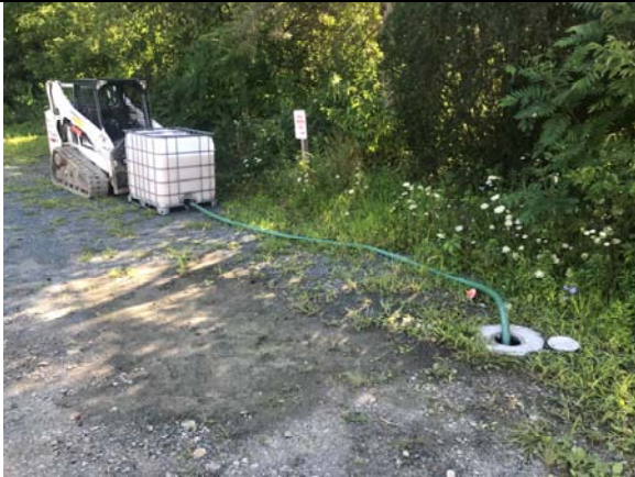
Injection at INJ-1 via gravity feed
