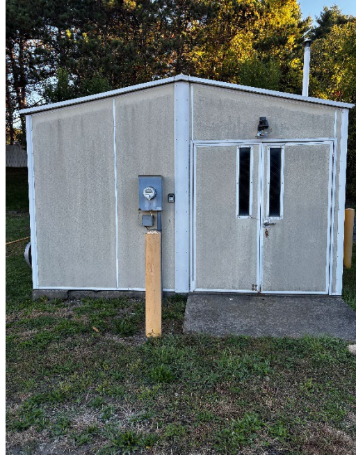
Treatment building secured at end of day
