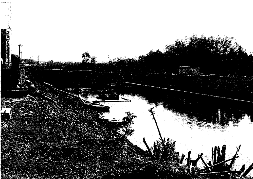
View of South Lagoon looking south
