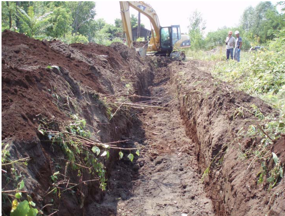
Photograph #13 – Facing west, extent of excavation for TP-222b
