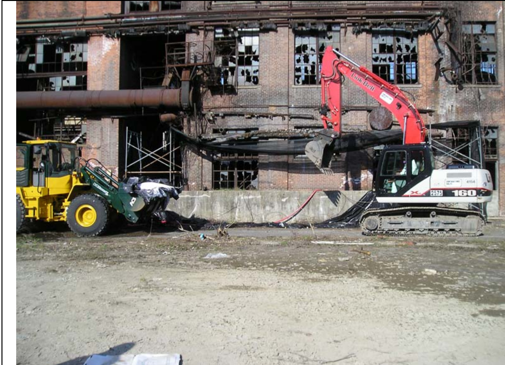
Photograph #11 Description: OWS – stabilization of coal tar sludge with lime
