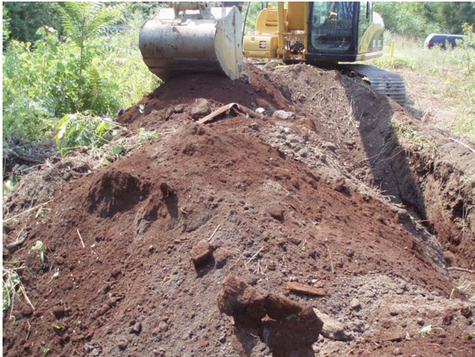
Photograph #6 – Western view of excavated spoils pile from TP-222b
