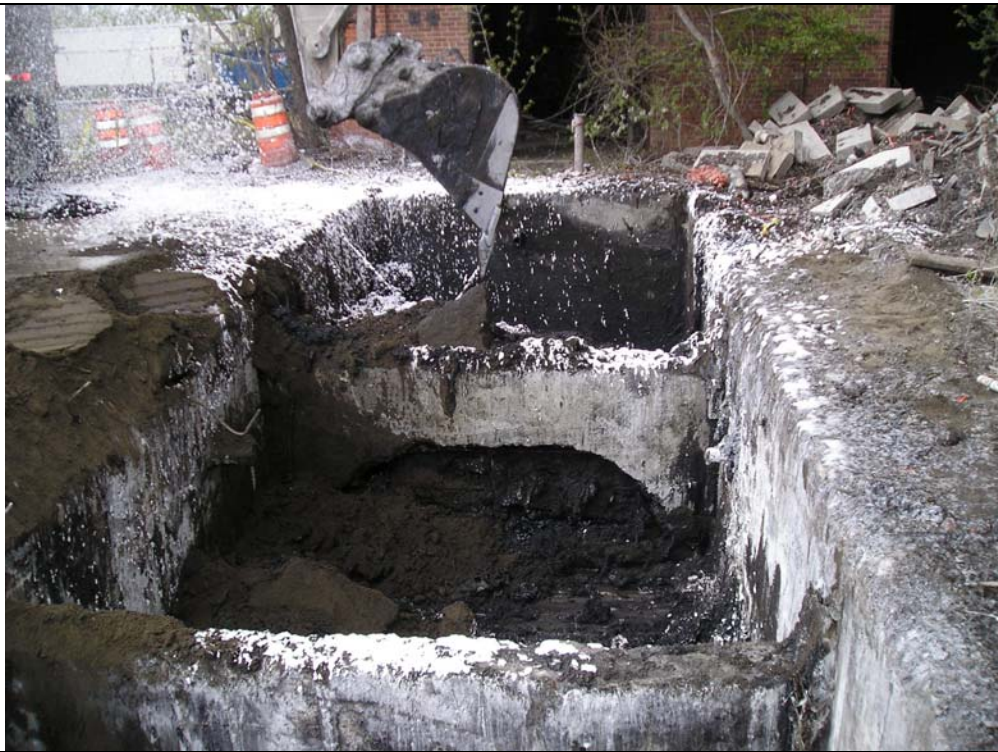
Photograph #20 Description: Removal of stabilized TLS materials
