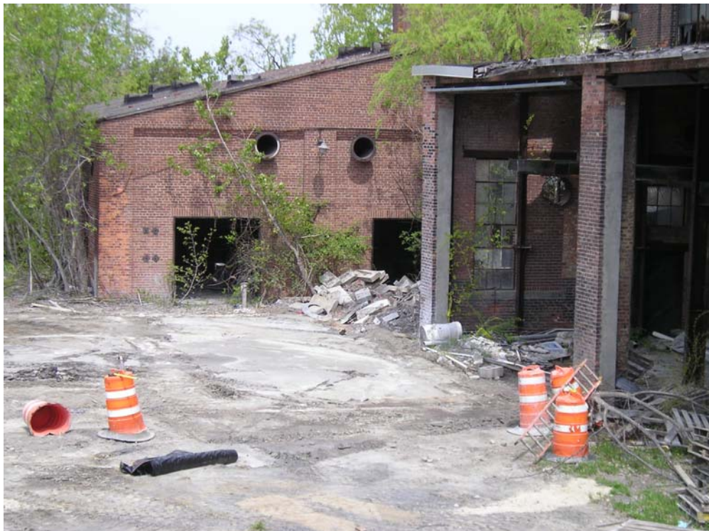
Photograph #23 Description: TLS backfilled to grade
