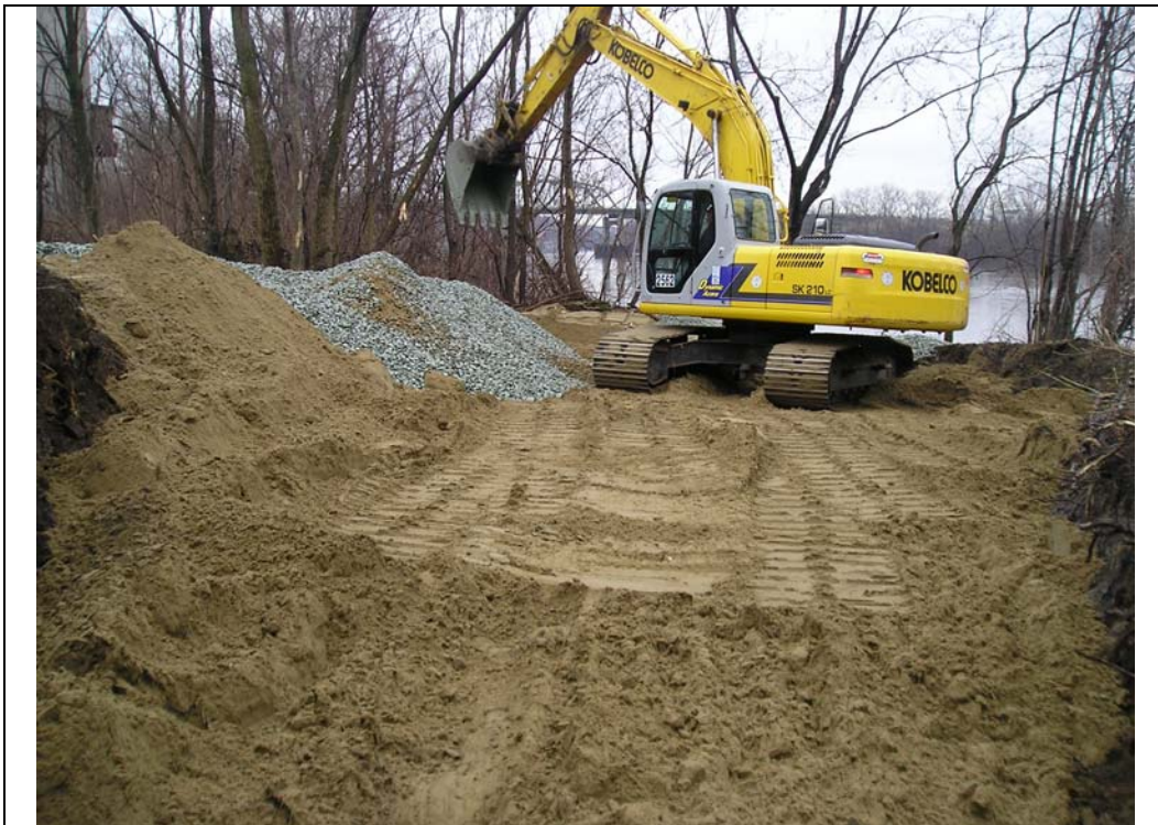
Photograph #6 Description: Backfilling of Purifier Waste Area with soil
