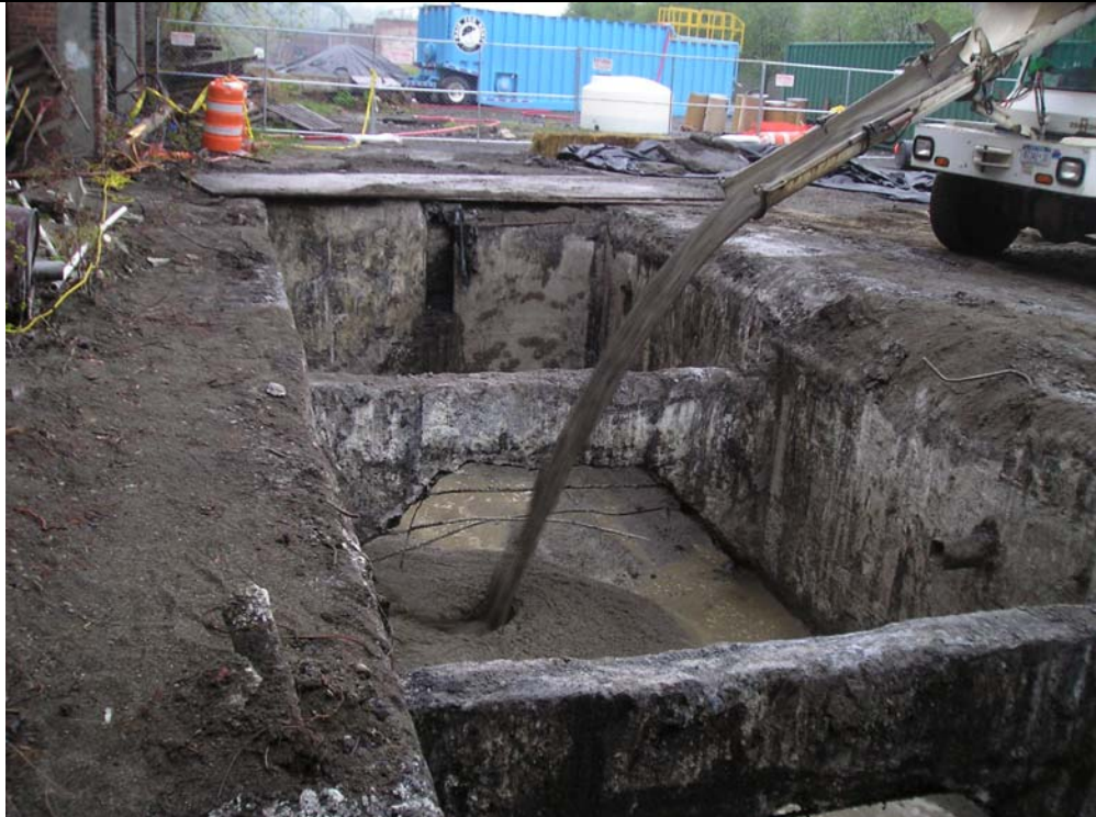
Photograph #22 Description: Backfilling TLS with flowable fill
