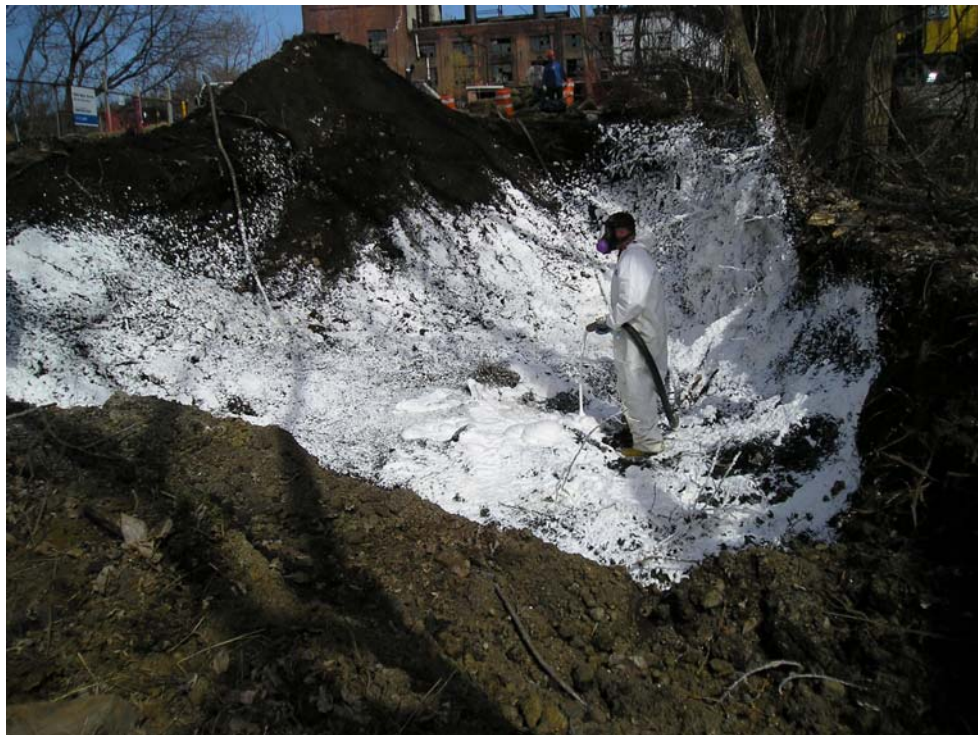
Photograph #4 Description: Purifier Waste – application of foam as dust and odor control measure
