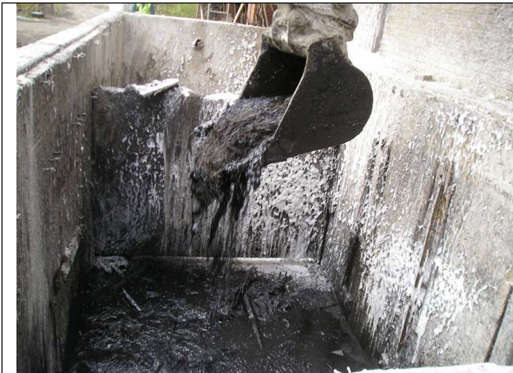
Photograph #12 Description: Removal of materials from OWS
