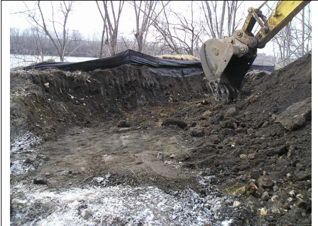
Photograph #5 Description: Excavation of Purifier Waste Deposits
