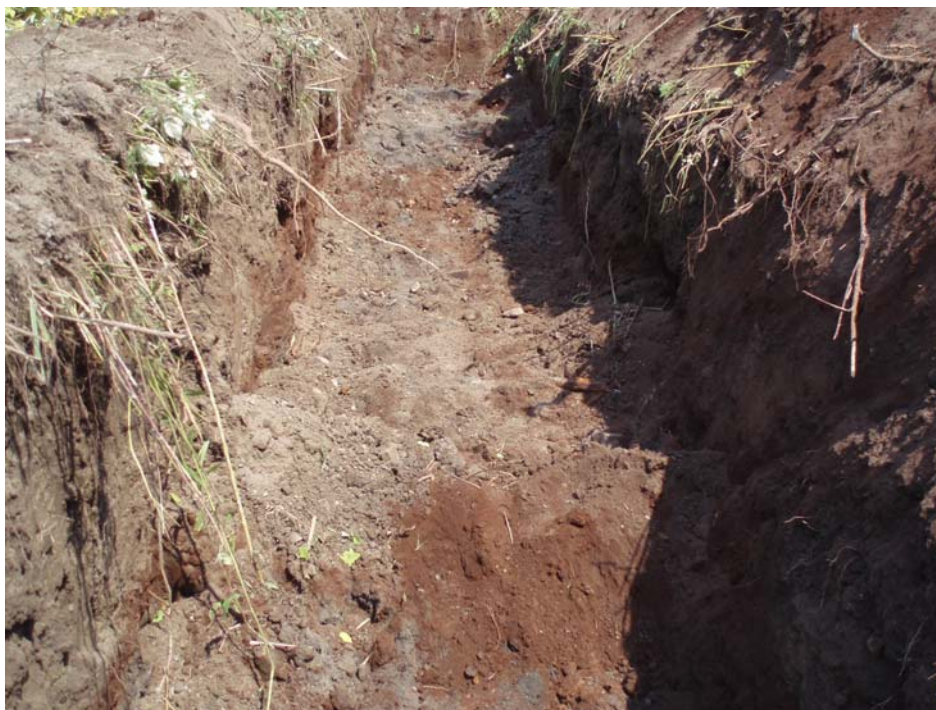
Photograph #10 – Facing east along TP-222b
