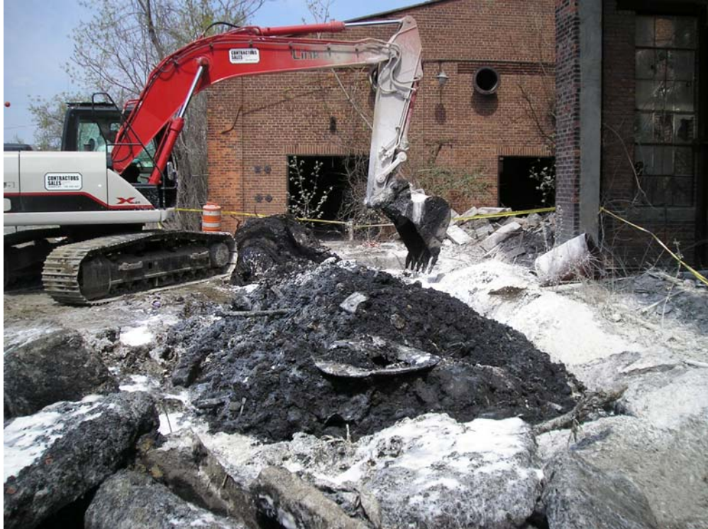
Photograph #19 Description: Removal of stabilized TLS materials
