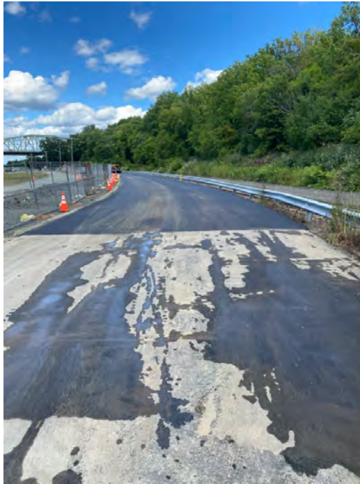
Photograph #65 – View looking north. Asphalt paving activities to restore River Road on CSX property (vicinity of Sta. 25+00). (Photo Taken 9/1/2022).
