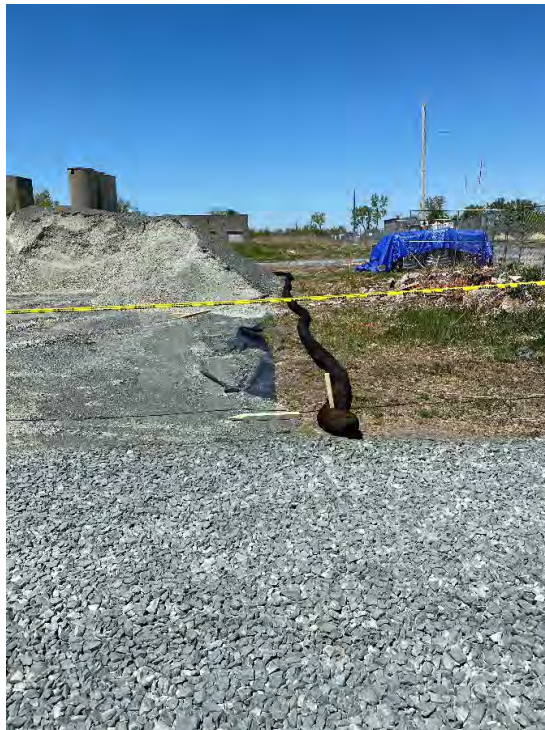
Photograph #18 – View looking north. Installation of additional erosion and sediment controls around stockpiles of imported backfill on Area 2. (Photo Taken 5/11/2022).
