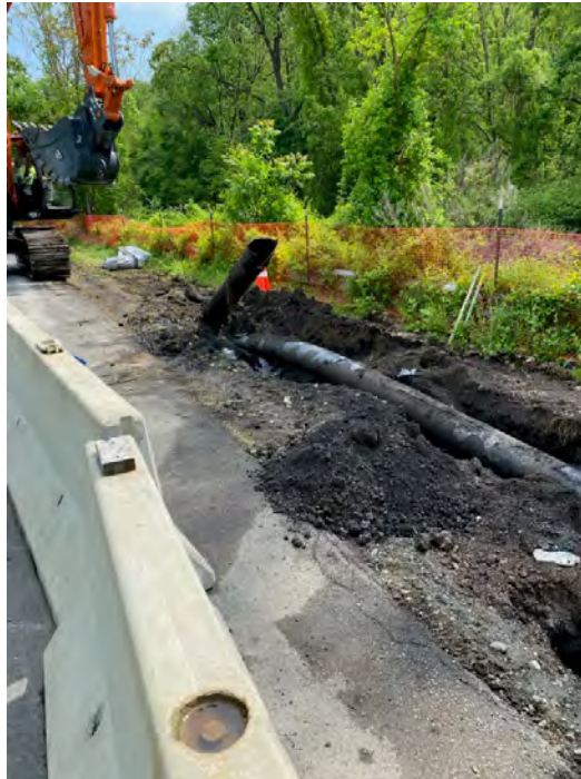
Photograph #29 – View looking northwest. Removal of pre-existing gas transmission line on CSX property (vicinity of Sta. 30+00). (Photo Taken 5/20/2022).
