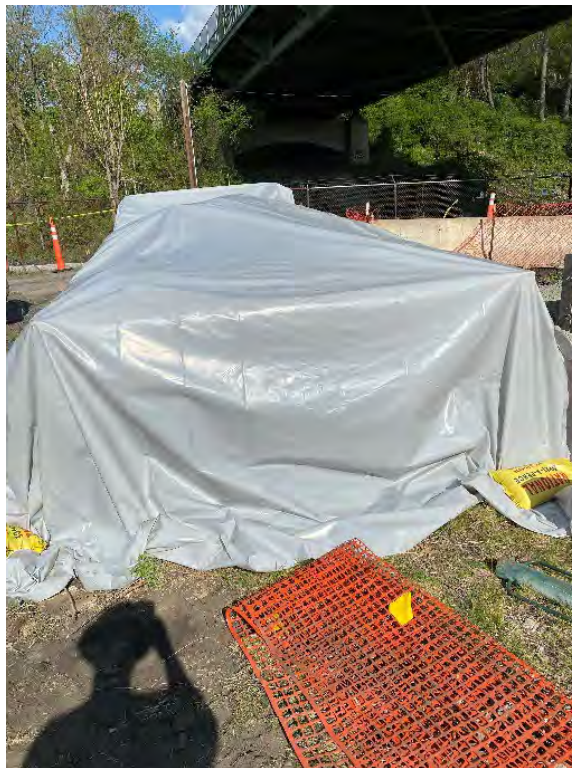
Photograph #20 – View looking east. Photo depicts covered excavated soils staged in a rock box on Area 3. (Photo Taken 5/12/2022).
