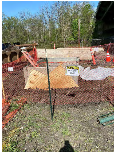
Photograph #22 – View looking east. Installation of the trench box on Area 3 at the location of the northern cut and cap of the pre-existing gas line (vicinity of Sta. 15+00). (Photo Taken 5/12/2022).
