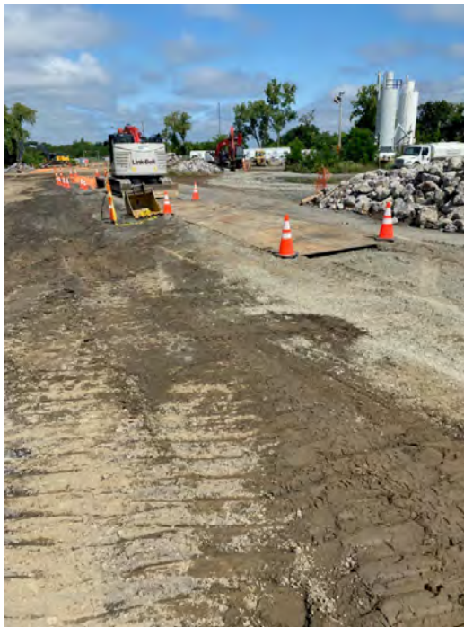
Photograph #66 – View looking north. Steel plates installed for temporary hardened crossing on Area 2 to facilitate movement of equipment for nearby Phase 1A remediation activities. (Photo Taken 9/8/2022).
