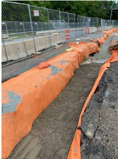
Photograph #47 – View looking southeast. Placement of flowable fill over bedding sand on Area 2 (vicinity of Sta. 11+00). (Photo Taken 7/21/2022).
