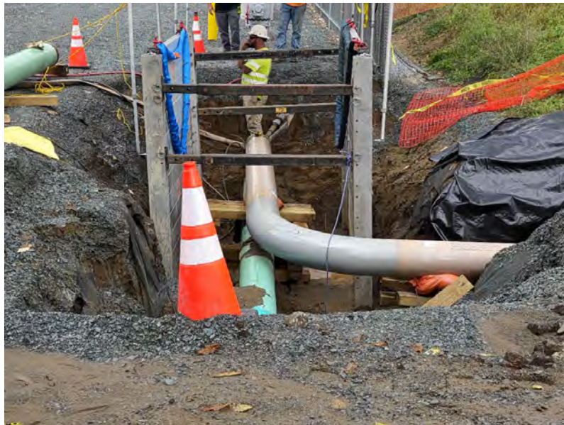
Photograph #70 – View looking north. Water releasing from the installed gas transmission line on Area 2 (vicinity of Sta. 00+00) into a 3-inch water hose following hydrostatic pressure testing. (Photo Taken 9/20/2022).
