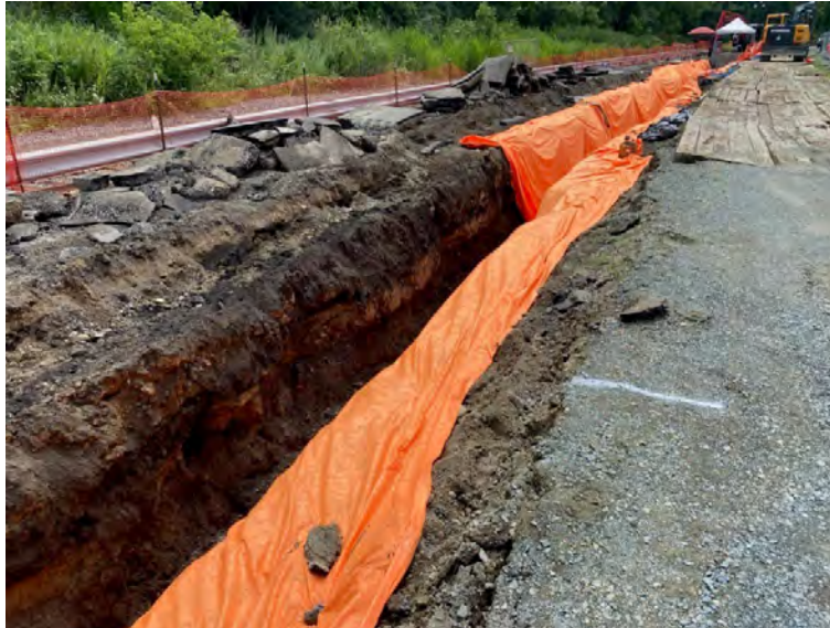
Photograph #56 – View looking southeast. Installation of non-woven, orange-colored geotextile fabric within the trench on CSX property. White line is approximately 10 feet north of last visual observation of tar-like material. LLDPE liner, sandwiched between non-woven, orange-colored geotextile fabric, was installed within the trench up to at least that line (approx. Sta. 23+32) from approx. Sta. 24+78. (Photo Taken 8/5/2022).
