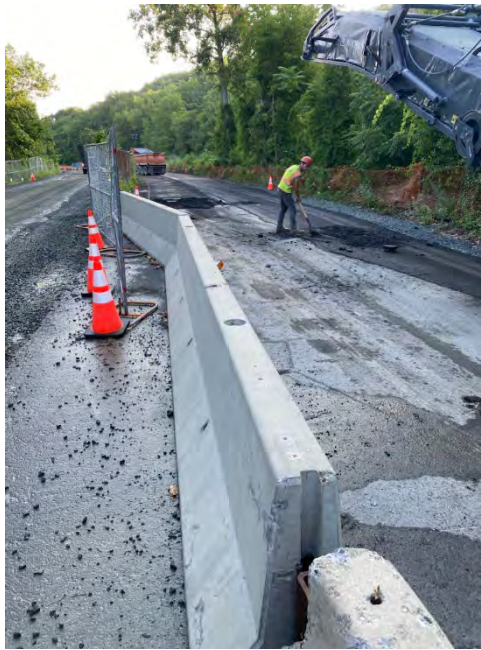
Photograph #51 – View looking northeast. Milling of asphalt on CSX property in preparation for paving/restoration (vicinity of Sta. 29+00). (Photo Taken 8/2/2022).
