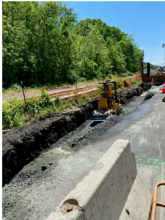
Photograph #32 – View looking southeast. Photo depicts backfill and compaction activities on CSX property (vicinity of Sta. 31+00). (Photo Taken 5/24/2022).
