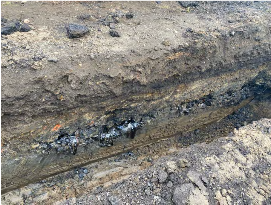
Photograph #37 – View looking west. Tar-like material visible on the west wall of the trench of the new gas transmission line on CSX property at Sta. 24+78. The layer of tar-like material is approximately 5 feet (ft.) below ground surface (bgs). (Photo Taken 6/8/2022).
