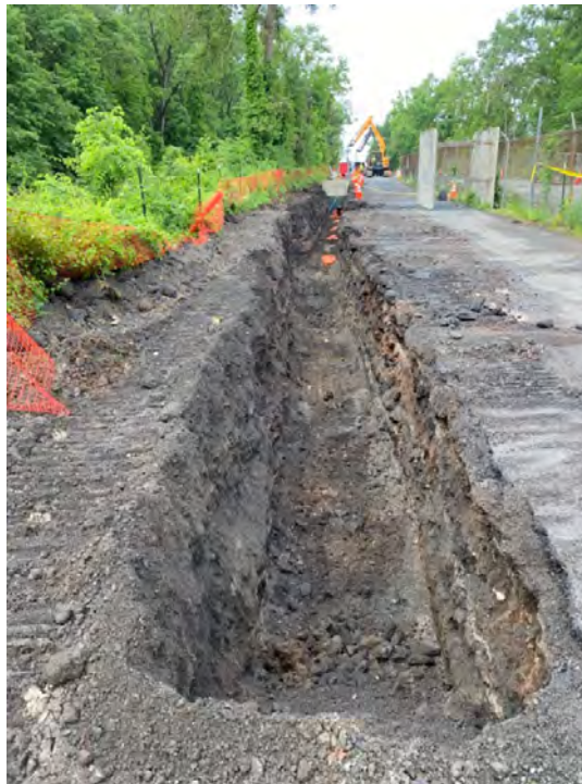
Photograph #36 – View looking south. Trench excavation for installation of new gas transmission line on CSX property (vicinity of Sta. 28+00). (Photo Taken 6/2/2022).
