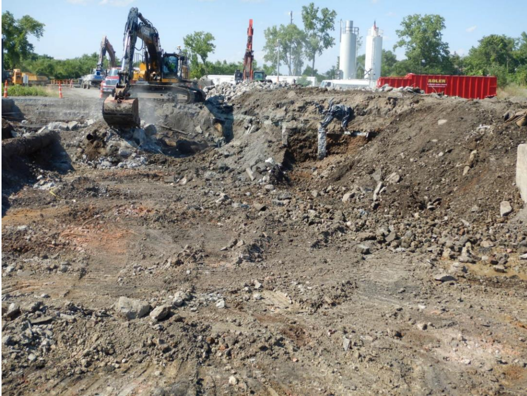
Photo 3. Remediation excavation at the Area 2 location, to approximately 10 feet below surface. View facing north.
