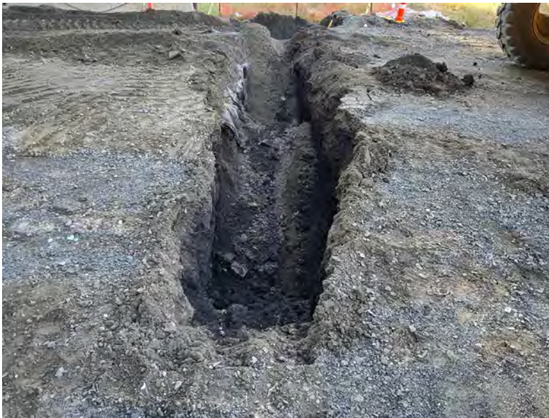
Photograph #74– View looking west. Trench excavated for retirement of the pre-existing pipeline at the boundary of Areas 2 and 3. (Photo Taken 9/29/2022).
