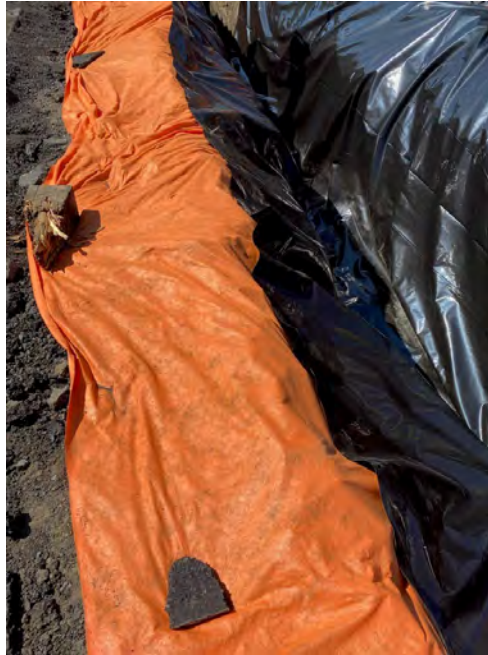
Photograph #53 – View looking southwest. Installation of linear-low density polyethylene (LLDPE) liner within the utility trench on CSX property (vicinity of Sta. 23+00). (Photo Taken 8/4/2022).
