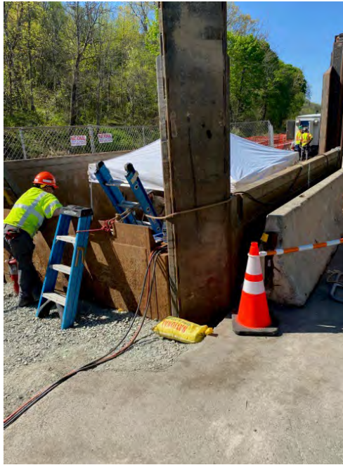
Photograph #17 – View looking south. Photo depicts welding activities occurring on the pre-existing gas transmission line on CSX property at the southern tie-in location (vicinity of Sta. 31+45). (Photo Taken 5/10/2022).
