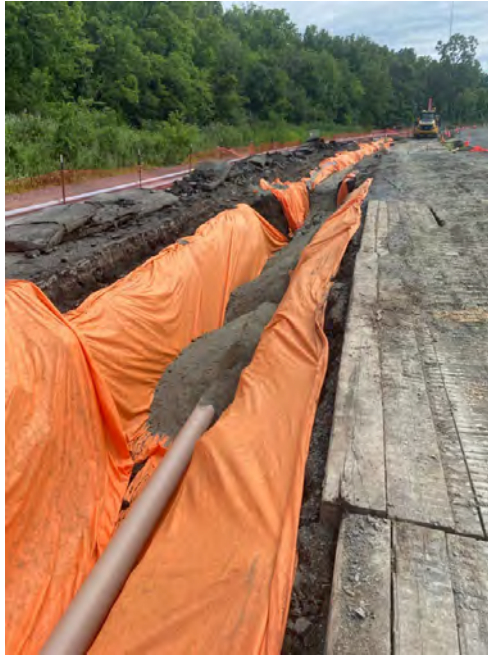
Photograph #57 – View looking south. Installation of non-woven, orange-colored geotextile fabric within the trench and backfill activities over newly installed gas transmission line on CSX property (vicinity of Sta. 22+50). (Photo Taken 8/10/2022).
