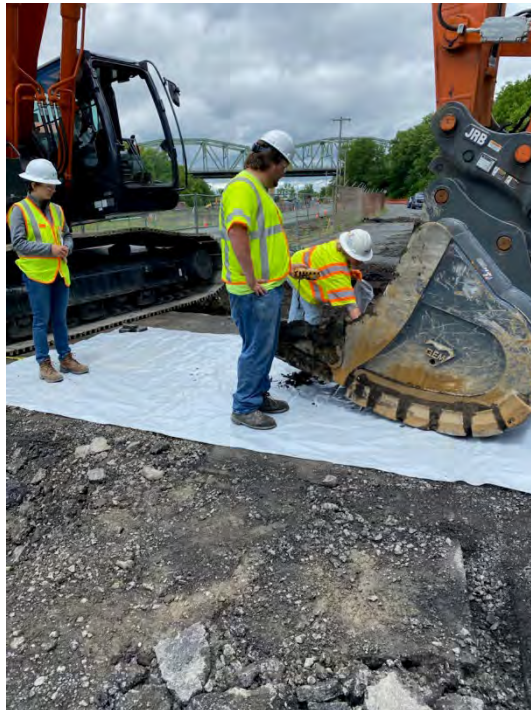
Photograph #38 – View looking north. Collection of waste characterization samples of soils impacted with tar-like material on CSX property. (Photo Taken 6/9/2022).
