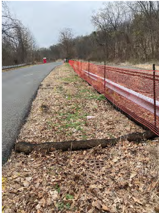
Photograph #3 – View looking north. Installation of sediment filter sock and orange construction fence on CSX Corporation (CSX) property. (Photo Taken 4/26/2022).
