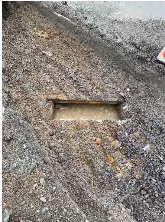
Photograph #48 – View looking east. Photo depicts a historic concrete structure that was encountered on Area 2 (vicinity of Sta. 09+00). The structure contained approximately 6 inches of water, clay/soil fill, and five pipes (1 to 2-inch diameter, oriented northeast to southwest). (Photo Taken 7/25/2022).
