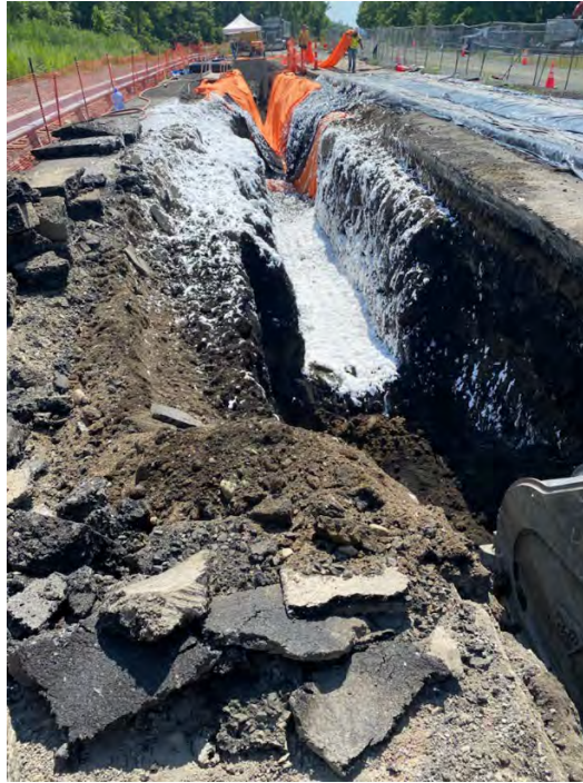
Photograph #55 – View looking south. Application of Rusmar Long Duration Foam within the trench on CSX property where tar-like material was encountered (vicinity of Sta. 23+00). (Photo Taken 8/4/2022).
