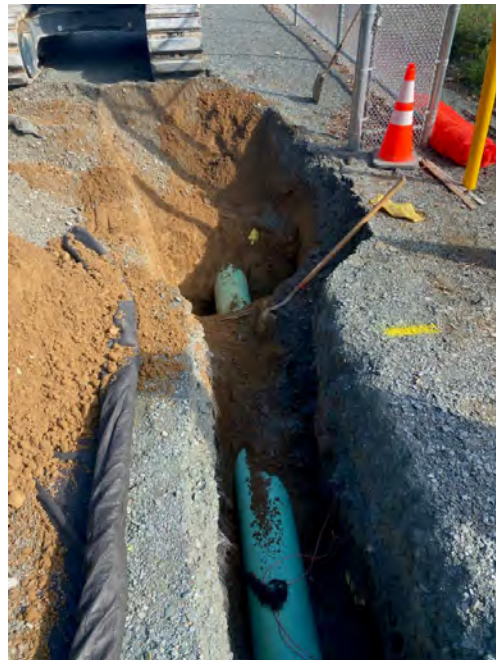
Photograph #64 – View looking north. Exposure of pre-existing gas transmission line at the regulator station on Area 2 (Sta. 0+00) to evaluate existing line for tie-in of new gas transmission line. (Photo Taken 8/31/2022).
