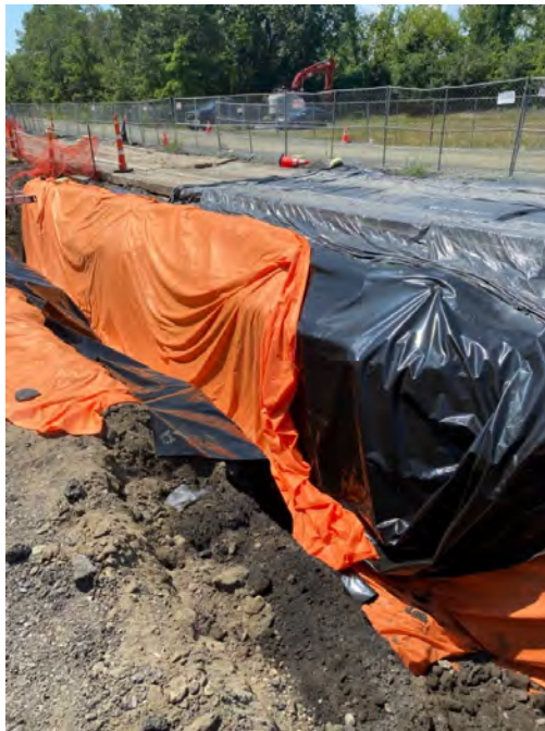
Photograph #54 – View looking southwest. Installation of non-woven, orange-colored geotextile fabric over the LLDPE liner within the utility trench on CSX property (vicinity of Sta. 23+00). (Photo Taken 8/4/2022).
