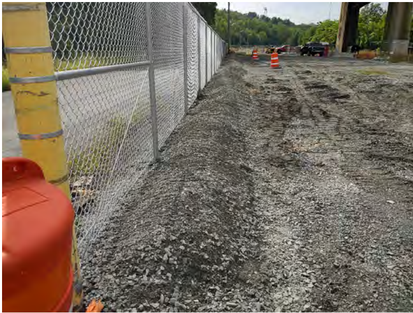
Photograph #69 – View looking south. Photo depicts replacement of fencing and stormwater berm on Chevron property (vicinity of Sta. 14+00). (Photo Taken 9/19/2022).
