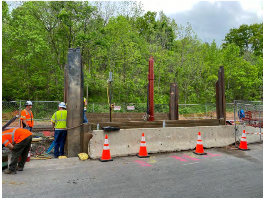
Photograph #25 – View looking west. Purging of existing gas transmission line on CSX property prior to cut and cap at the southern tie-in location (vicinity of Sta. 31+45). (Photo Taken 5/17/2022).
