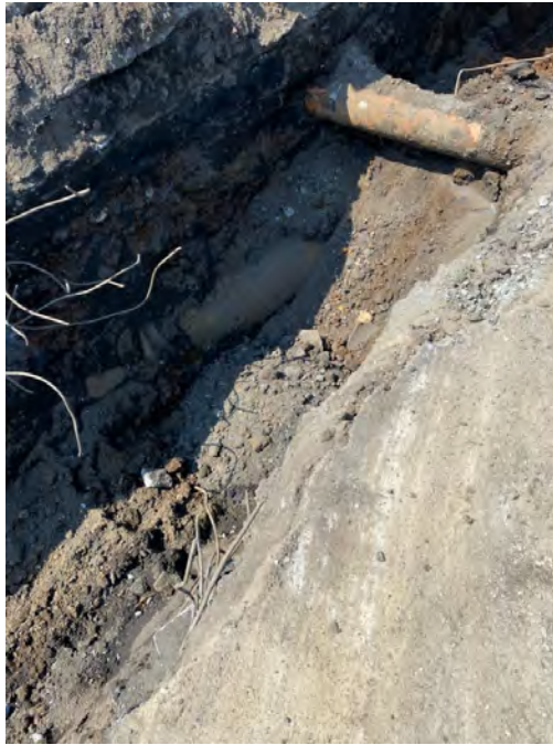
Photograph #59 – View looking northwest. Photo depicts approx. 30" bell-spigot pipe (oriented north-south) encountered at approximately 5.5 ft. bgs on Area 2 (vicinity of Sta. 4+00). Pipe is at a slight northeast to southwest angle and will intercept the trench excavation from approximately Sta. 4+30 to 4+50. Additional east-west oriented pipes also shown in the photo. (Photo Taken 8/25/2022).
