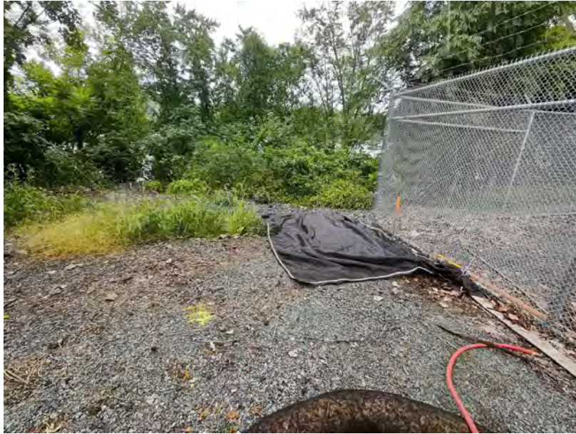
Photograph #71 – View looking west. Photo depicts the filter bag that the water from hydrostatic pressure testing was released into on Area 2. (Photo Taken 9/20/2022).
