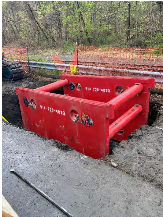
Photograph #12 – View looking east. Installation of trench box on CSX property at the southern tie-in location (vicinity of Sta. 31+45). (Photo Taken 5/4/2022).
