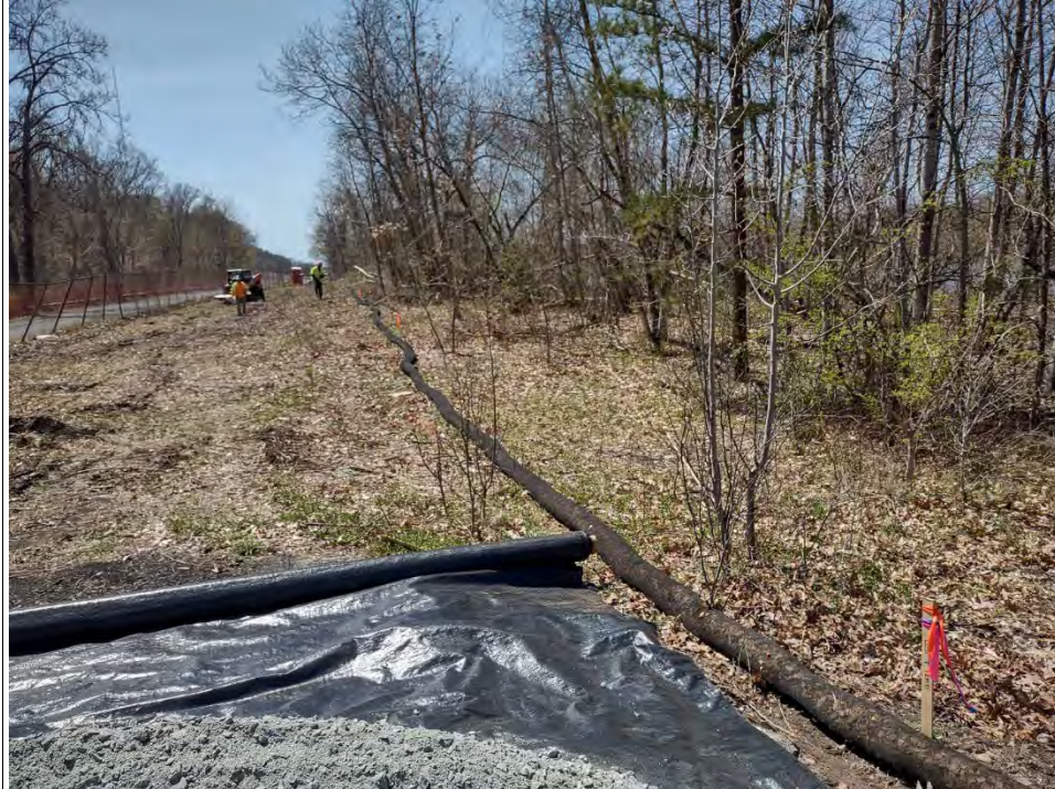
Photograph #7 – View looking south. Installation of sediment filter sock on the western side of the Limit of Disturbance on Chevron property. (Photo Taken 4/28/2022).
