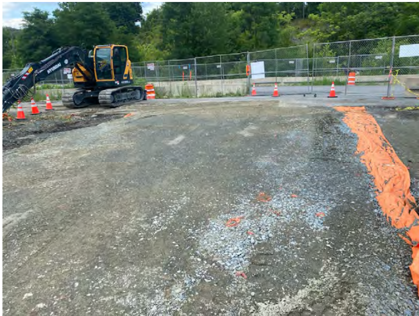
Photograph #50 – View looking east. Final installation of permanent hardened crossing over newly installed gas transmission line on Area 2 (vicinity of Sta. 10+00) to allow for access to current support zone (construction trailers). (Photo Taken 7/28/2022).
