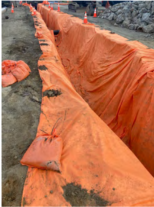
Photograph #63 – View looking northeast. Installation of non-woven, orange geotextile demarcation fabric. Photo also depicts an existing 12-inch steel pipe oriented east-west across the trench in Area 2 (approximately Sta. 4+50). Gas transmission line was installed underneath this existing pipe. (Photo Taken 8/30/2022).
