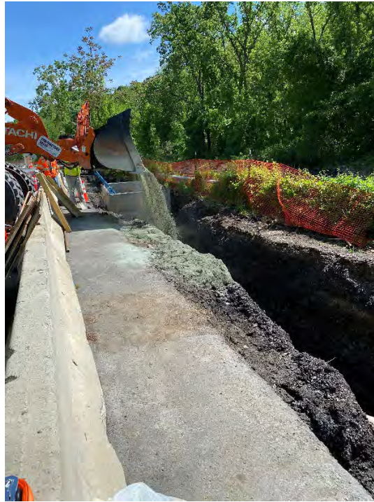
Photograph #31 – View looking northeast. Backfilling with bedding sand around the new gas transmission line on CSX property (vicinity of Sta. 31+00). (Photo Taken 5/23/2022).
