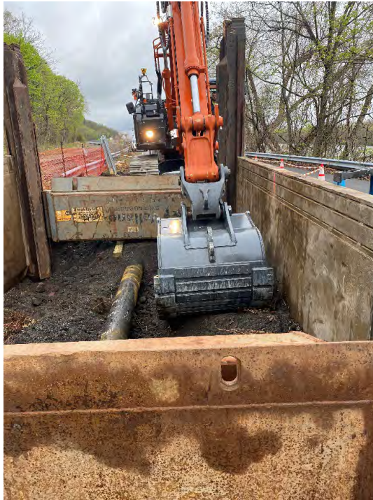
Photograph #11 – View looking south. Excavation within slide rail system on CSX property at the southern tie-in location (vicinity of Sta. 31+45). (Photo Taken 5/4/2022).
