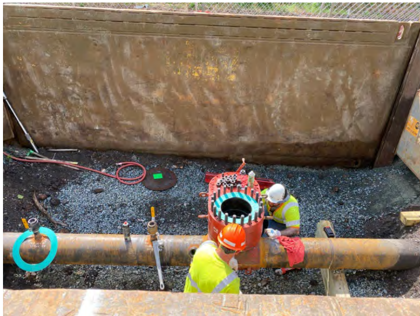
Photograph #24 – View looking west. Installation of TD Williamson tooling on CSX property at the southern tie-in location (vicinity of Sta. 31+45). (Photo Taken 5/16/2022).
