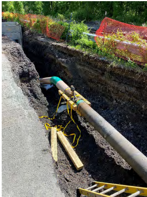
Photograph #30 – View looking northeast. Installation of new gas transmission line on CSX property (vicinity of Sta. 31+45) at southern tie-in location. (Photo Taken 5/23/2022).
