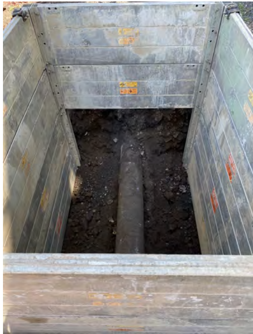
Photograph #21 – Photo depicts the excavation area on Area 3 at the location of the northern cut and cap of the pre-existing gas line (vicinity of Sta. 15+00). (Photo Taken 5/12/2022).
