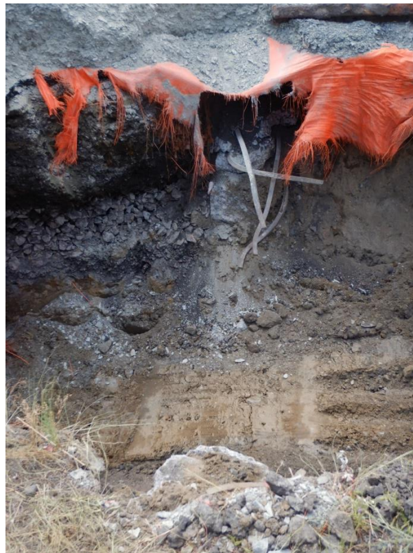
Photo 6. Concrete garage wall foundation crossing the trench at about Station 10+00 (approx. 600 feet north of the Troy-Menands Bridge). Note the rebar in the concrete wall. View facing west.
