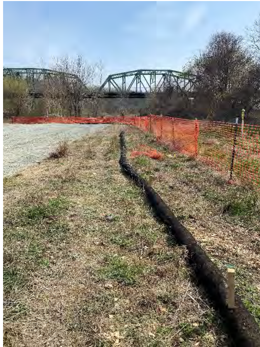
Photograph #1 – View looking south. Installation of sediment filter sock and orange construction fence around the support zone being constructed on Troy (Water St.) Site - Area 2 (Area 2). (Photo Taken 4/25/2022).
