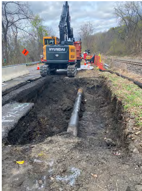
Photograph #10 – View looking north. Excavation around pre-existing gas transmission line on CSX property to facilitate installation of a slide rail system at the southern tie-in location (vicinity of Sta. 31+45). (Photo Taken 5/3/2022).
