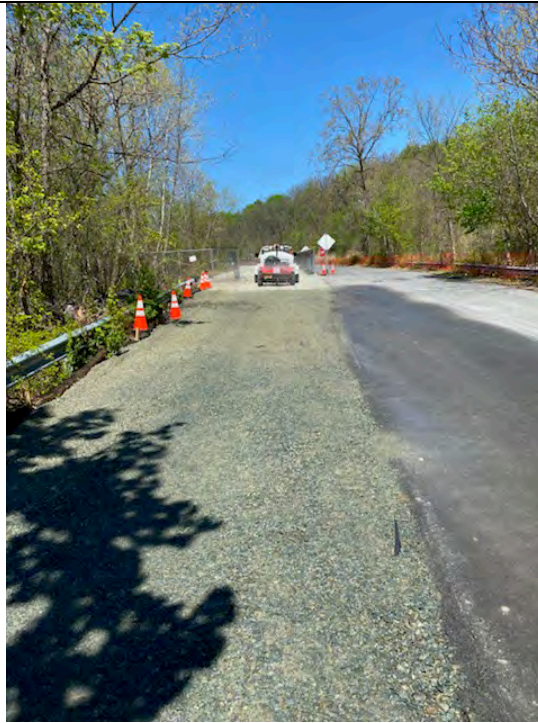
Photograph #15 – View looking north. Implementation of dust control on the temporary access road on Chevron property. (Photo Taken 5/9/2022).
