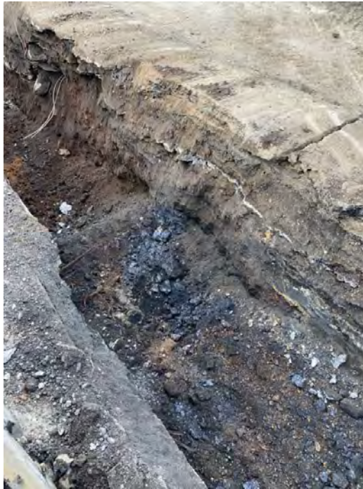
Photograph #61 – View looking east. Excavation and encountered hardened tar-like material at approximately Sta. 3+70 on Area 2. (Photo Taken 8/29/2022).
