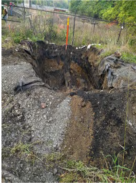
Photograph #75 – View looking south. Excavated trench and pre-existing gas transmission line prior to cutting and capping the pre-existing gas transmission line at the boundary of Areas 2 and 3. (Photo Taken 9/30/2022).
