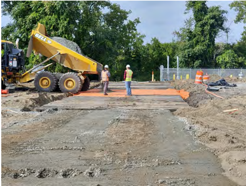
Photograph #77 – View looking west. Installation of the permanent timber mat hardened crossing on Area 2 north of the former E-lot Building (vicinity of Sta. 1+00). (Photo Taken 9/30/2022).
