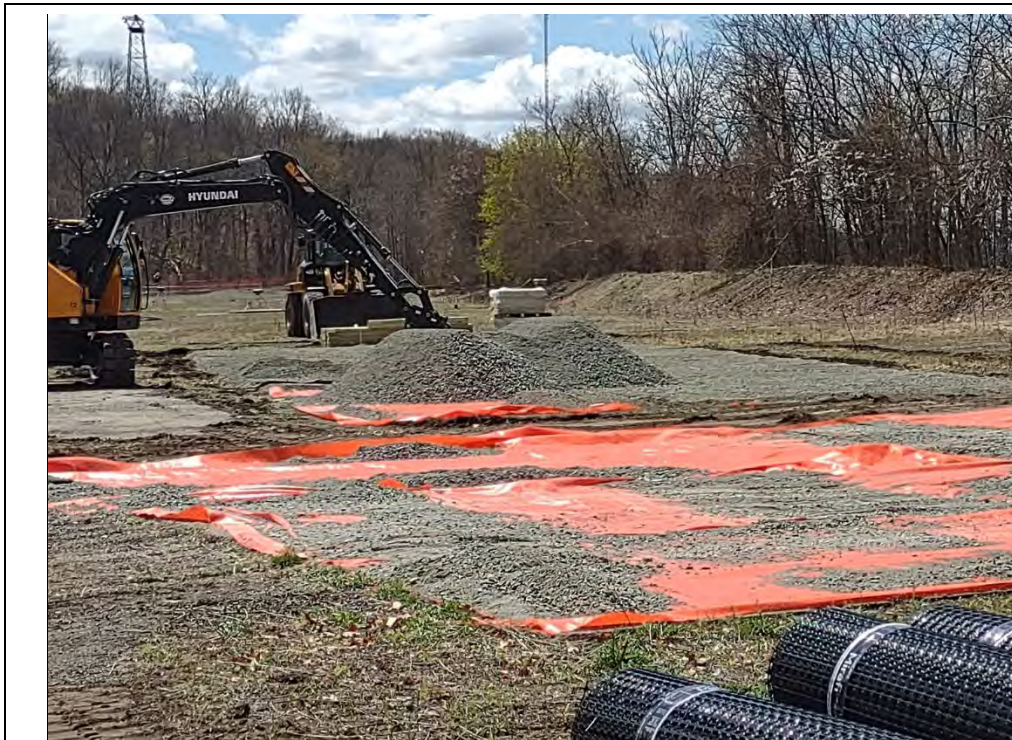
Photograph #5 –View looking south. Installation of a staging area for imported fill material stockpiling and pipeline pre-fabrication on Chevron property. (Photo Taken 4/27/2022).
