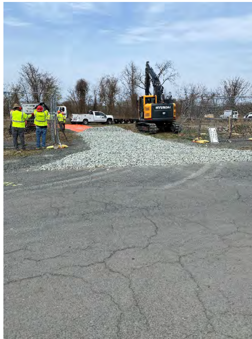
Photograph #2 – View looking west. Installation of geotextile fabric and #3 stone for the access road to the support zone (Area 2). (Photo Taken 4/25/2022).
