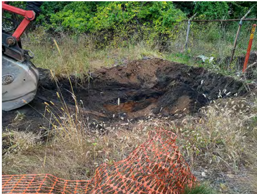
Photograph #76 – View looking west. Trench prior to cutting and capping the pre-existing gas transmission line at the boundary of Areas 2 and 3. (Photo Taken 9/30/2022).
