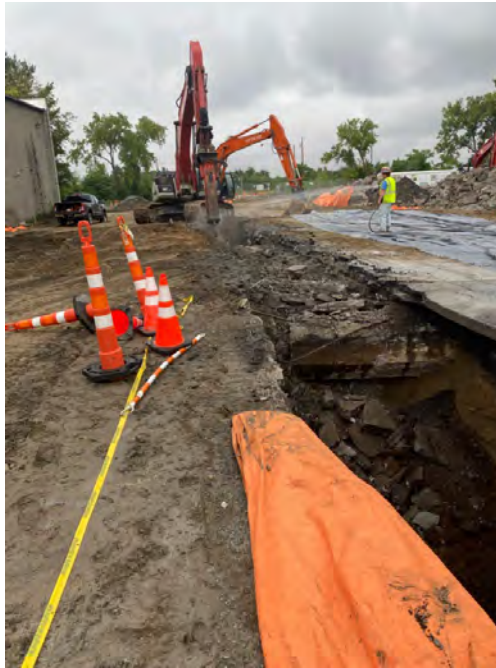
Photograph #67 – View looking north. Excavation of trench and removal of unknown concrete structure at approximately Sta. 3+00 to 3+20 on Area 2. (Photo Taken 9/12/2022).
