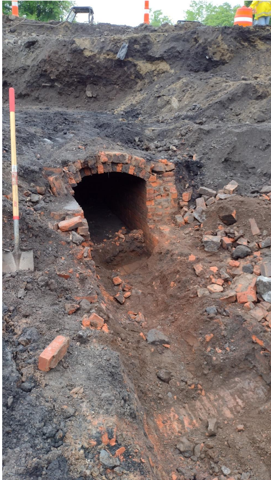
Photo 7. Culvert found perpendicular to trench within Area 3. View facing east
