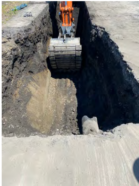
Photograph #40 – View looking north. Trench excavation starting at Sta. 22+00 on CSX property after skipping approximately 278 linear feet north due to potential for tar-like material. Photo also depicts the north-south orientated 42" diameter sewer force main (left) approximately 4.7 ft. bgs. (Photo Taken 6/14/2022).
