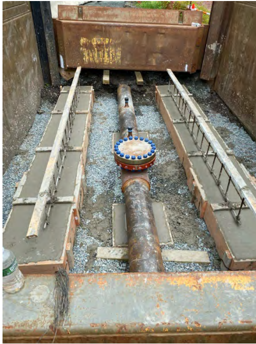
Photograph #35 – View looking north. Photo depicts poured concrete for construction of T.D. Williamson charging port installation on CSX property at the southern tie-in location (vicinity of Sta. 31+45). (Photo Taken 6/2/2022).
