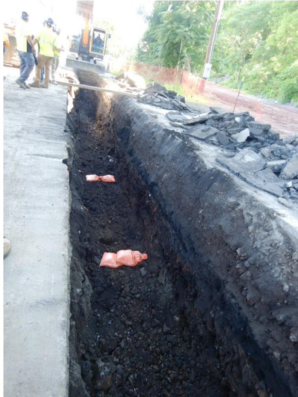
Photo 1. Typical trench excavation, near Station 16+50. The orange sand bags will support the new gas pipeline once lowered into the trench. View facing north northeast.
