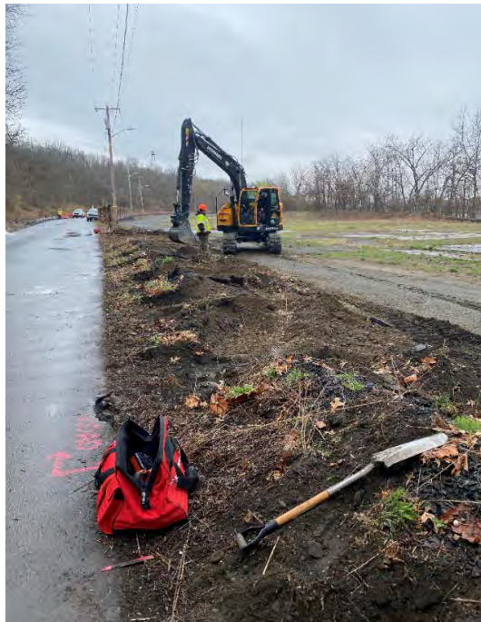
Photograph #4 – View looking south. Flattening of berm for installation of temporary access road on the Chevron Former Asphalt Facility Site (Chevron). (Photo Taken 4/26/2022).
