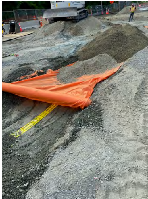
Photograph #44 – View looking southeast. Placement of orange demarcation fabric and 1-foot final Site Cover on Area 3 above newly installed gas transmission line (vicinity of Sta. 14+00). (Photo Taken 7/14/2022).
