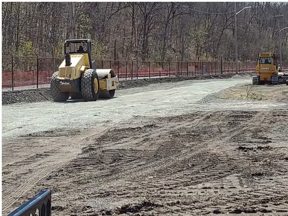
Photograph #6 – View looking south. Installation of the temporary road on the eastern side of the Chevron property. (Photo Taken 4/27/2022).
