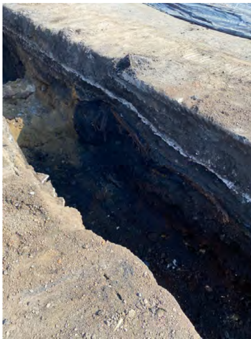
Photograph #62 – View looking east. Excavation and east-west oriented historical pipes encountered within trench at approximately Sta. 3+60 on Area 2. Four 12-inch steel pipes were encountered. All pipes were evaluated, determined to be empty and were removed from the trench and plugged. (Photo Taken 8/29/2022).
