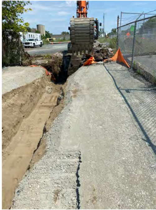
Photograph #43 – View looking north. Photo depicts trench excavation activities on Area 3 and exposure of concrete foundation walls on Area 2 (vicinity of Sta. 13+00). (Photo Taken 7/12/2022).
