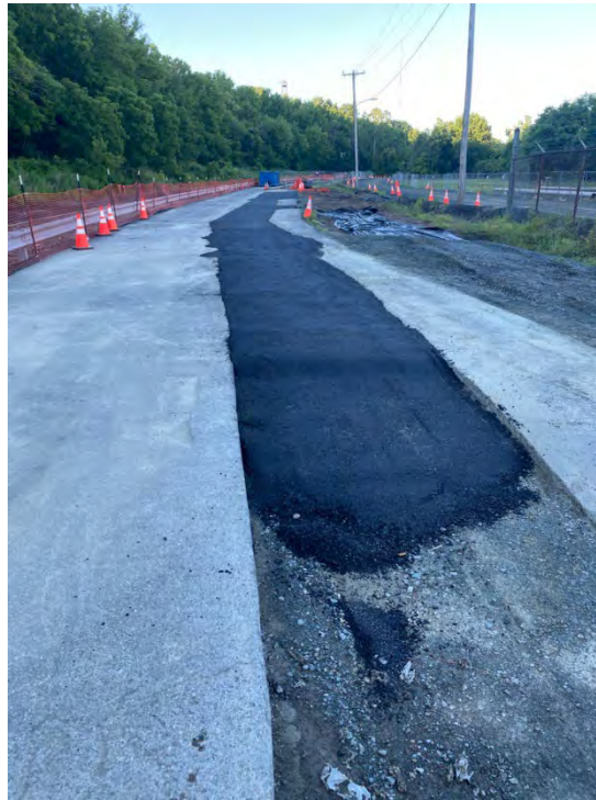
Photograph #41 – View looking south. Paving/restoration over completed gas transmission line installation on CSX property (vicinity of Sta. 19+00). (Photo Taken 7/6/2022).
