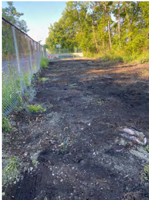
Photograph #58 – View looking south. Restoration of temporary access road footprint in the southern portion of the Chevron property. Restoration included removal of crusher run and geotextile fabrics, scraping existing soil and placement of seed. (Photo Taken 8/19/2022).
