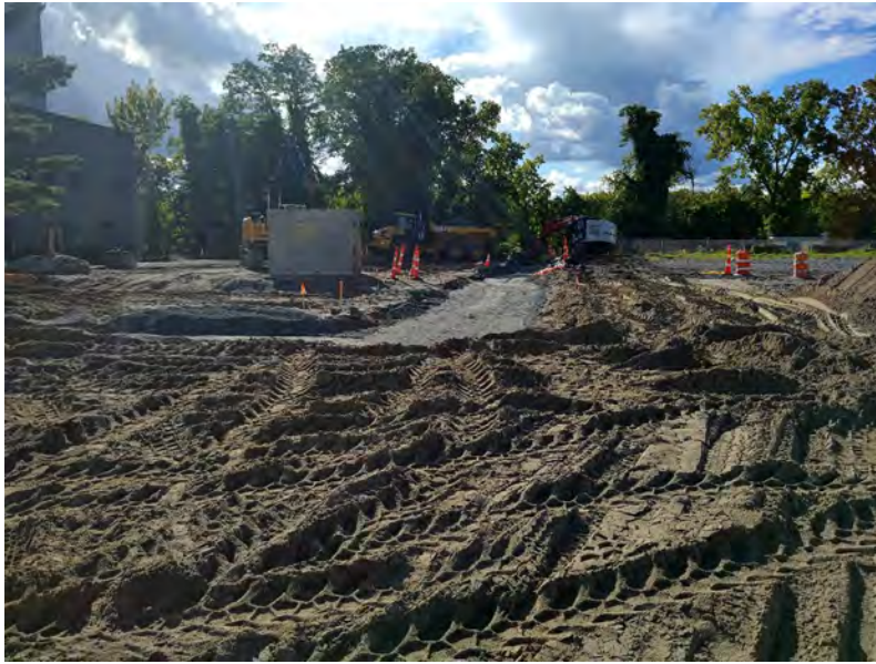
Photograph #73 – View looking west. Backfilling activities at the north tie-in location (Sta. 01+50) and in the utility trench on Area 2. (Photo Taken 9/28/2022).
