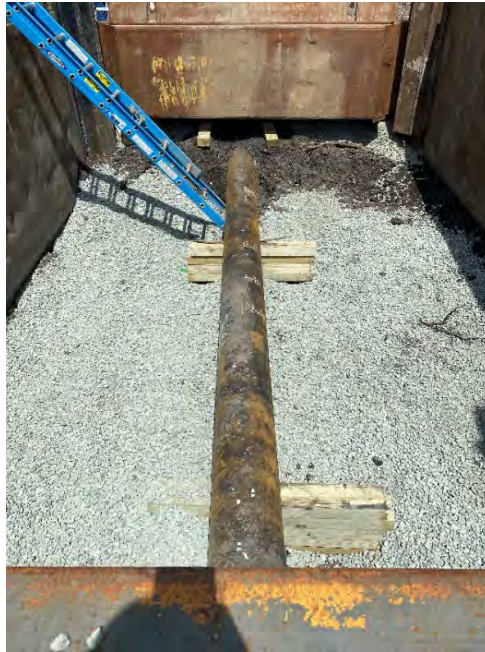
Photograph #13 – View looking north. Addition of NYSDOT No. 2 stone within excavation around pre-existing gas transmission line to facilitate welding and cutting activities on CSX property at the southern tie-in location (vicinity of Sta. 31+45). (Photo Taken 5/5/2022).
