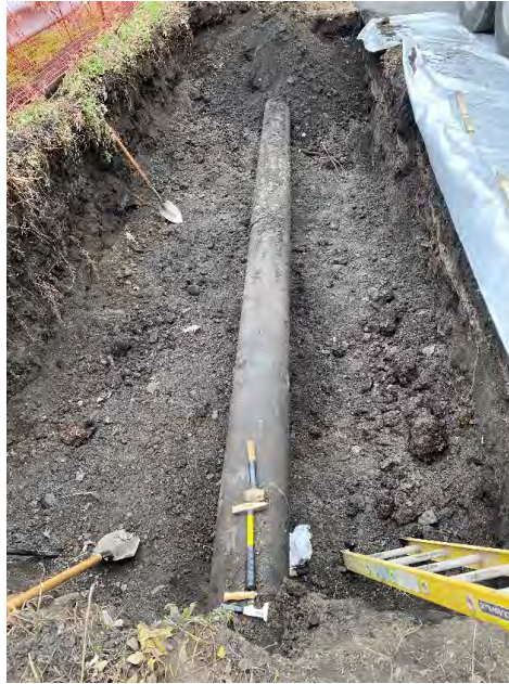
Photograph #9 – View looking south. Excavated area around pre-existing gas transmission line on CSX property to expose pipe to facilitate scanning (vicinity of Sta. 31+45). (Photo Taken 5/2/2022).
