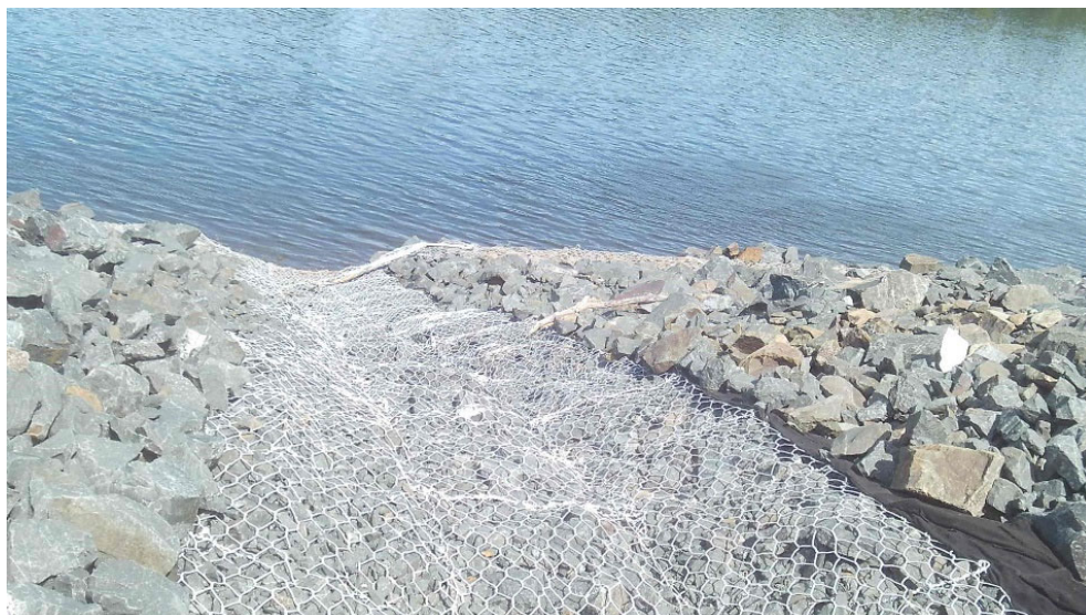
Rip Rap along eastern shore of Hudson River. View is to the west.
