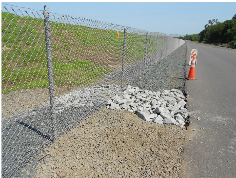
Completed repair of the riprap.
