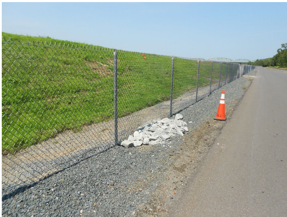
Completed repair of the riprap.
