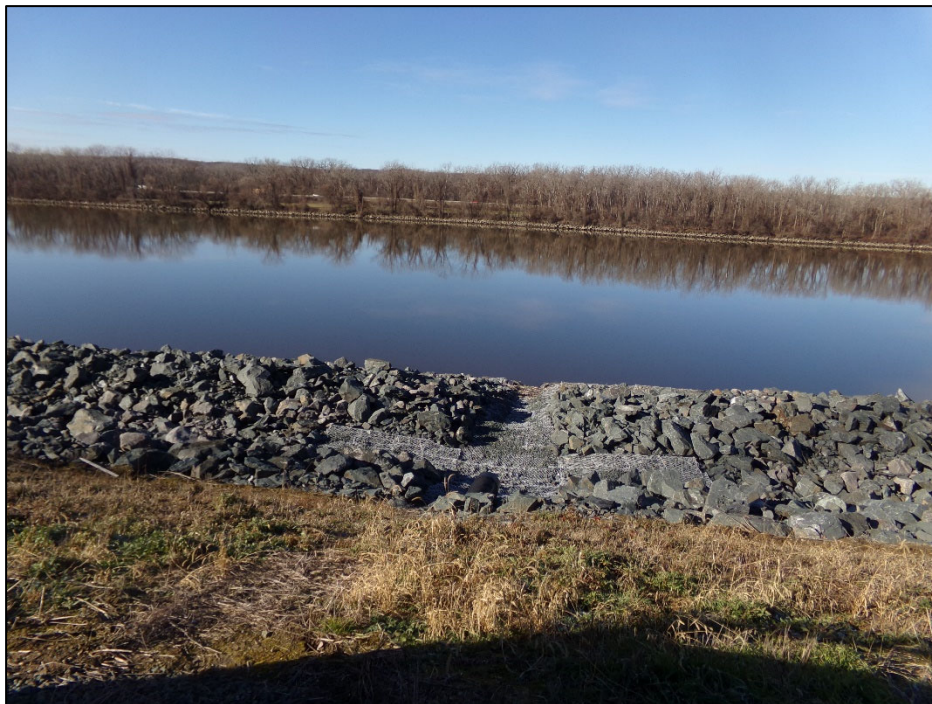
Rip Rap along the eastern shore of Hudson River. View is to the West.
