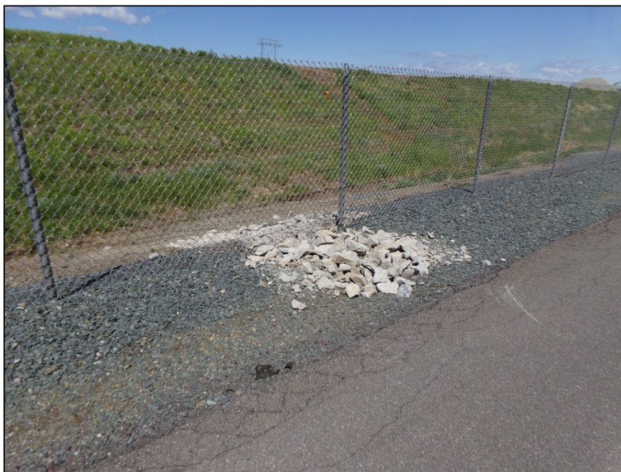
Restored fence line with new gravel.
