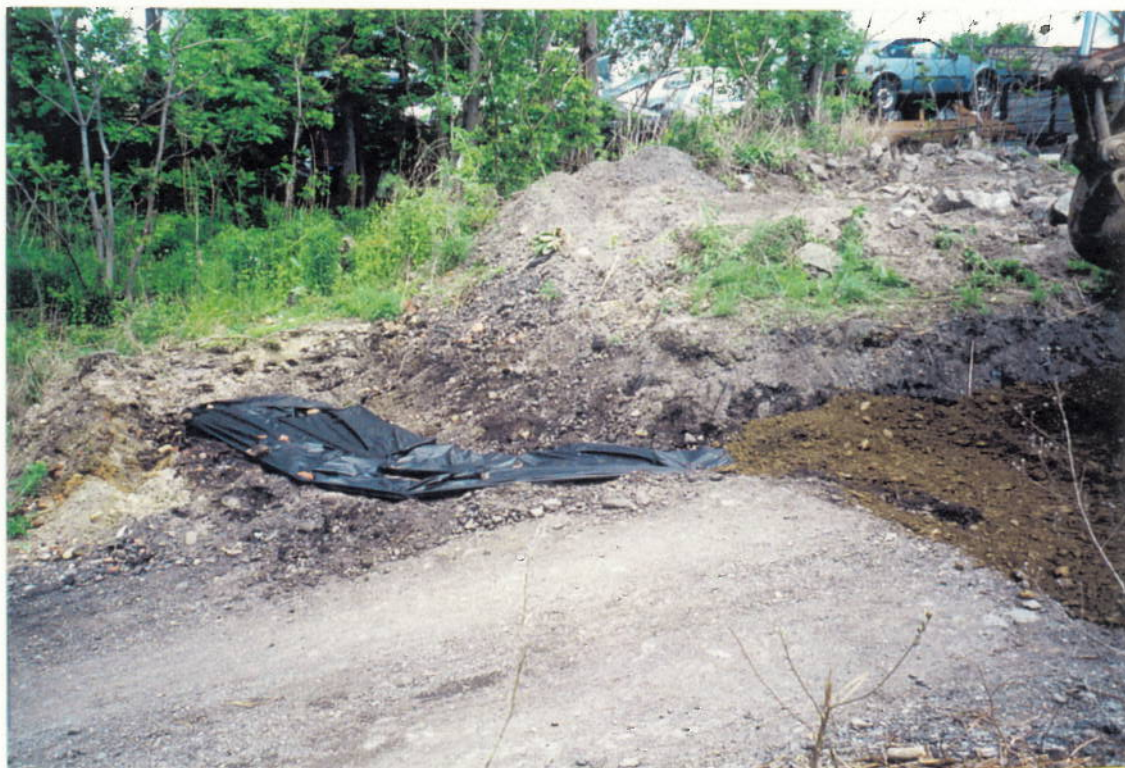
Photo 8: Placement of filter fabric in excavation prior to backfilling.
