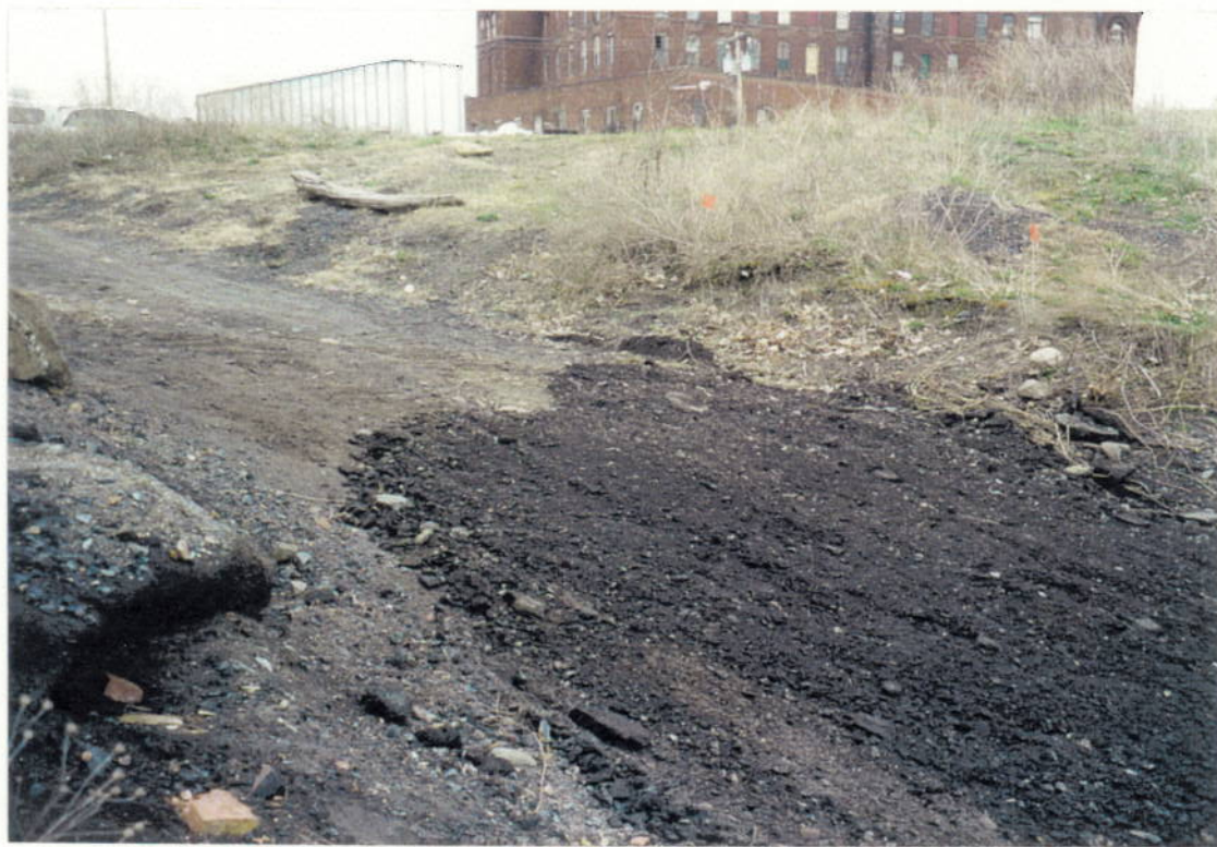
Photo 3: Ingalls Avenue Site prior to waste removal activities. Photograph, facing southeast, shows milled asphalt placed over road bed by the City of Troy.
