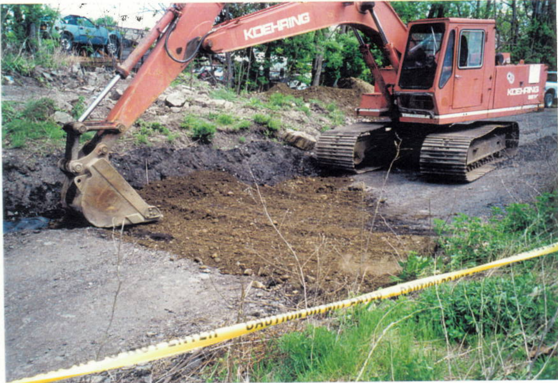
Photo 9: Backfilling of excavation.
