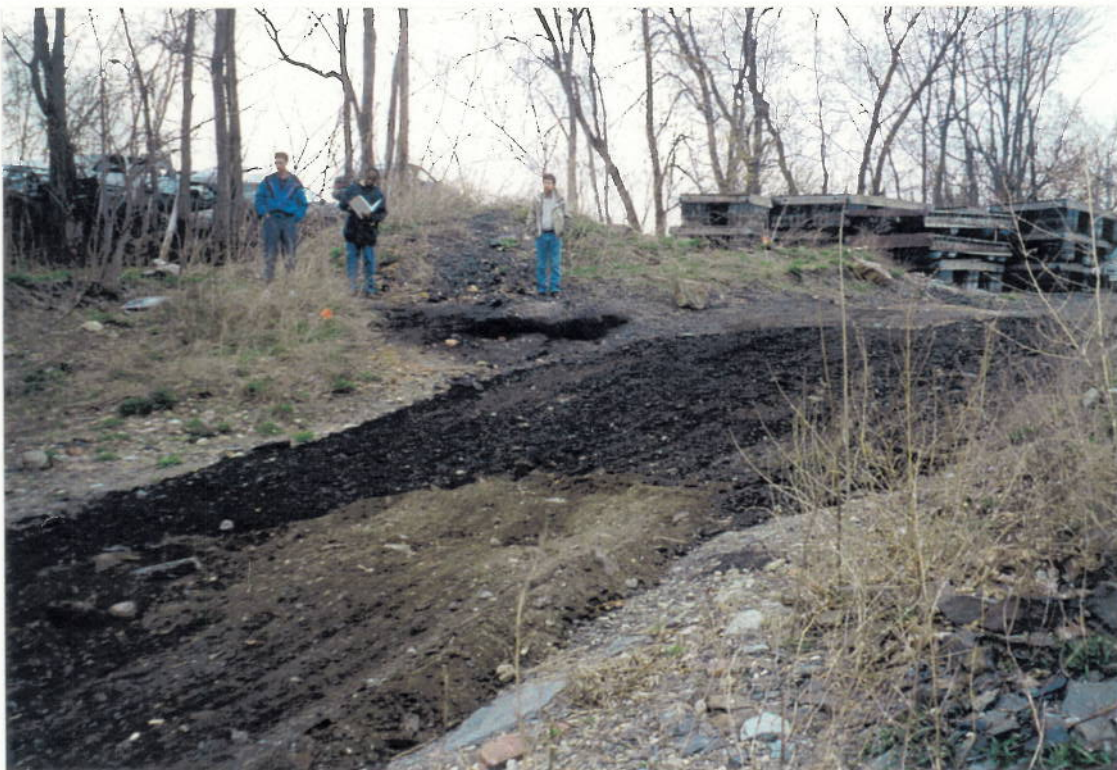
Photo 4: Ingalls Avenue Site prior to waste removal activities. Photograph, facing northeast, shows milled asphalt placed over road bed by the City of Troy.
