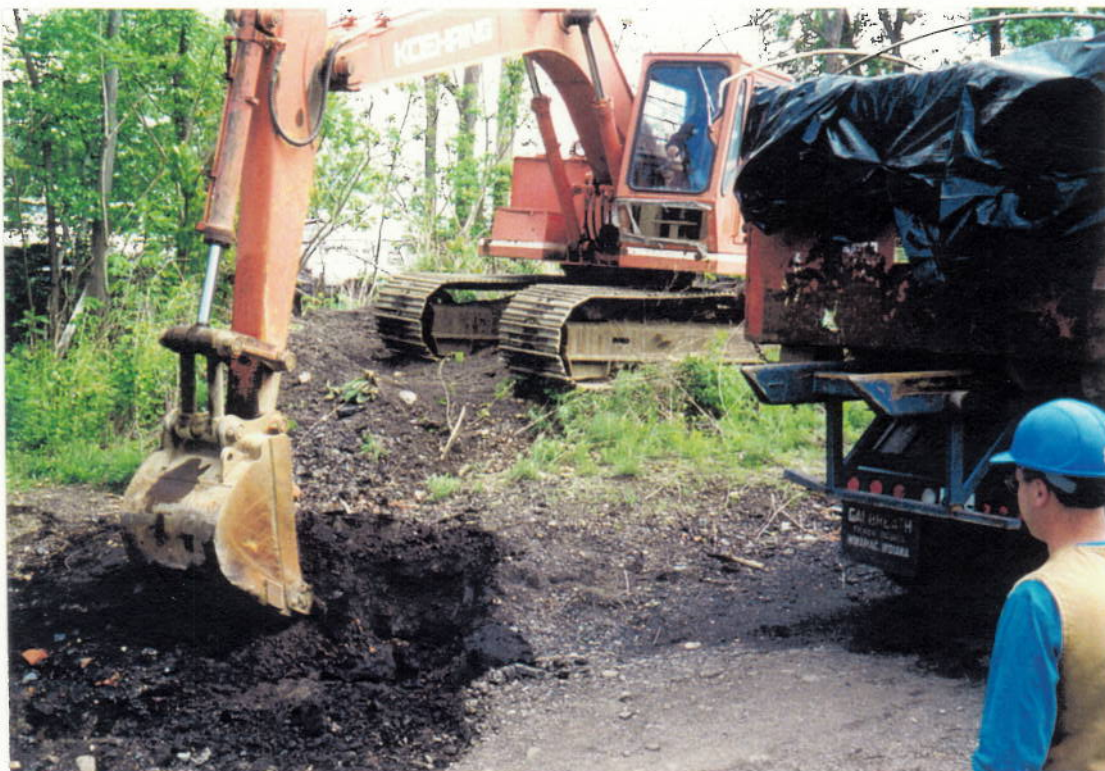
Photo 5: Excavation of waste material by trackhoe.
