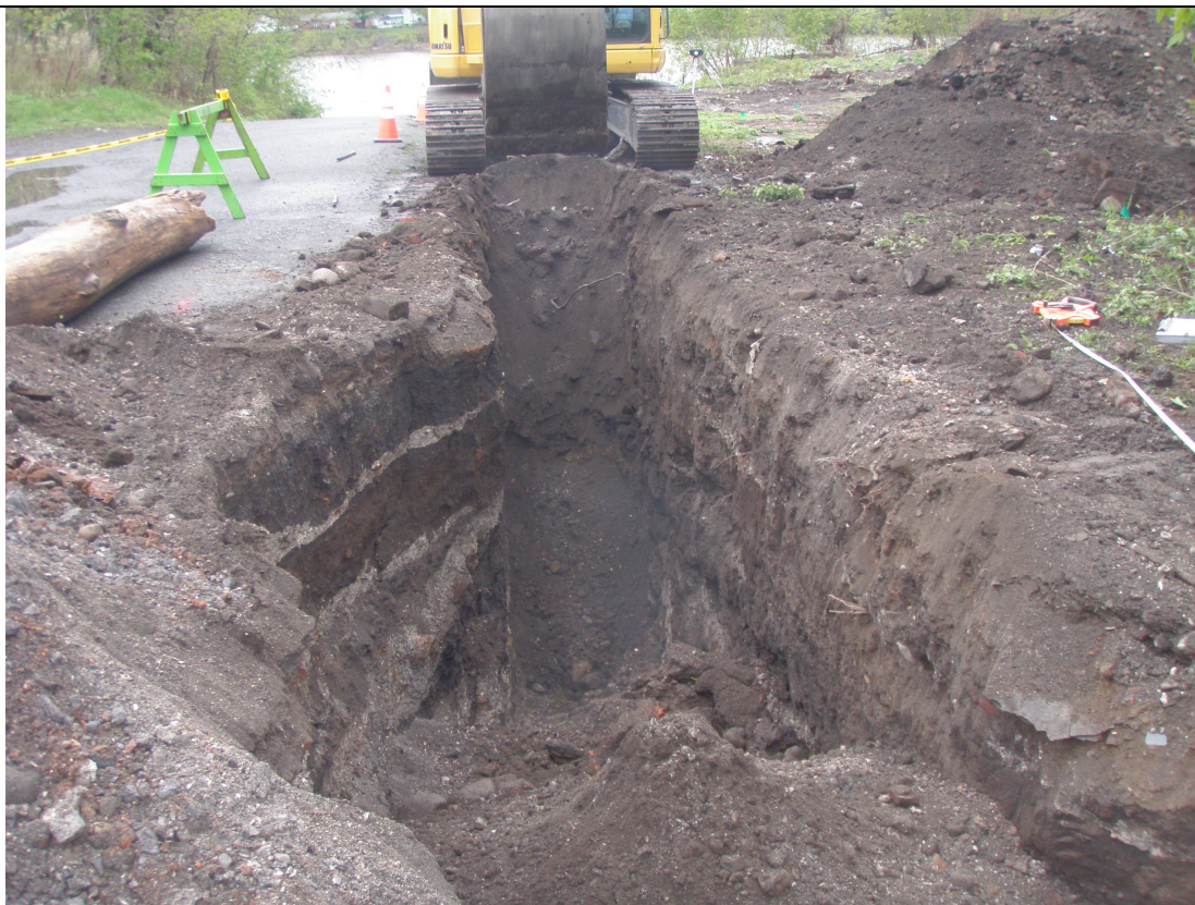
Photo 1: Fill Material Test Pit 16
