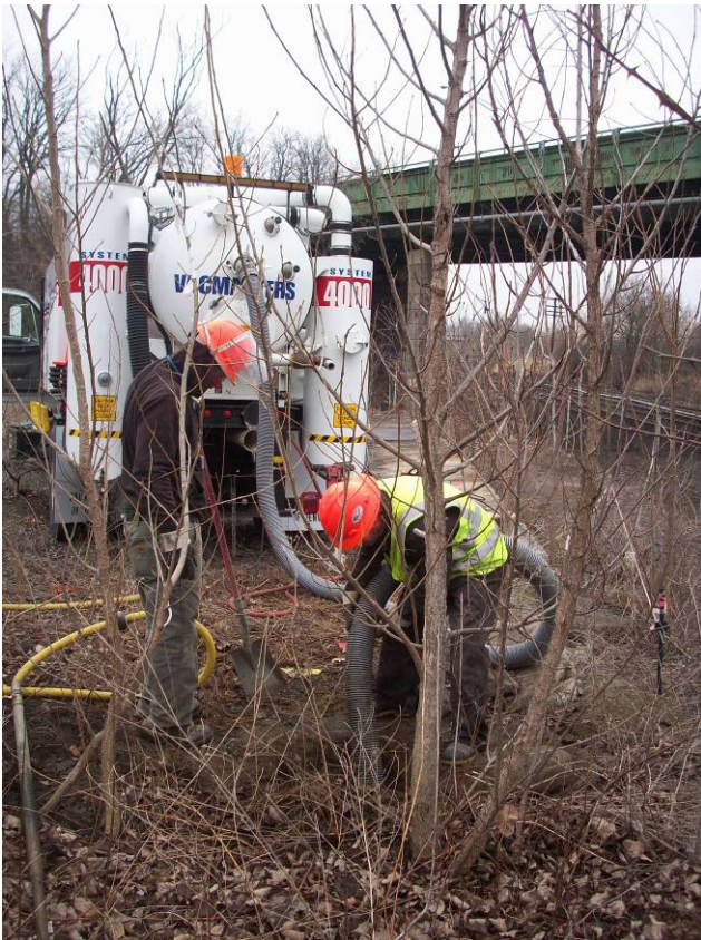
Air Knifing at IW-A2
