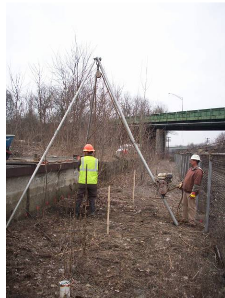
Tripod Drilling at MW-20
