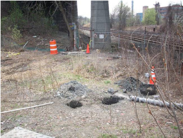
Hand Clearing of IW-A5 and IW-A6 Looking South Hits Concrete at 3.5' bgs
