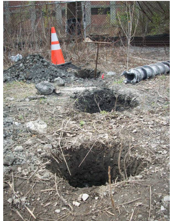
IW-A5 Searching for Concrete Boundary via Hand Clearing. T-rod Marks Possible Western Edge
