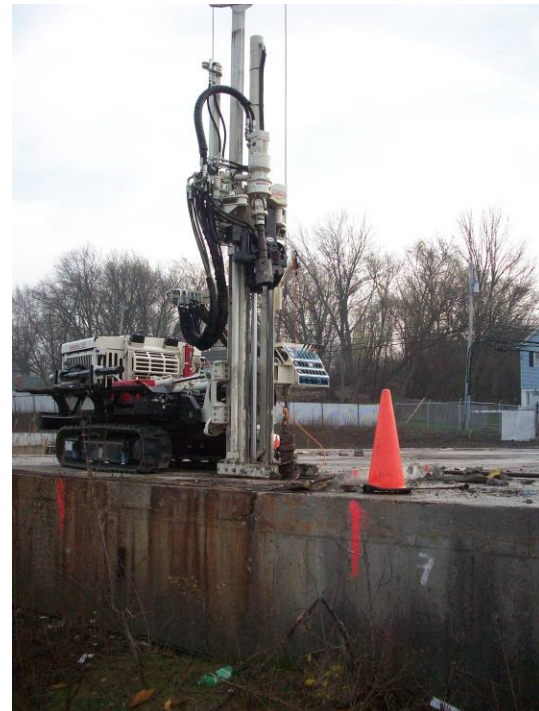
Drilling IW-B5 with ATV Rig
