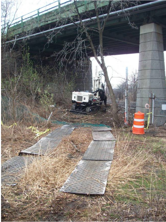
Drilling at IW-A7 Using ATV Rig
