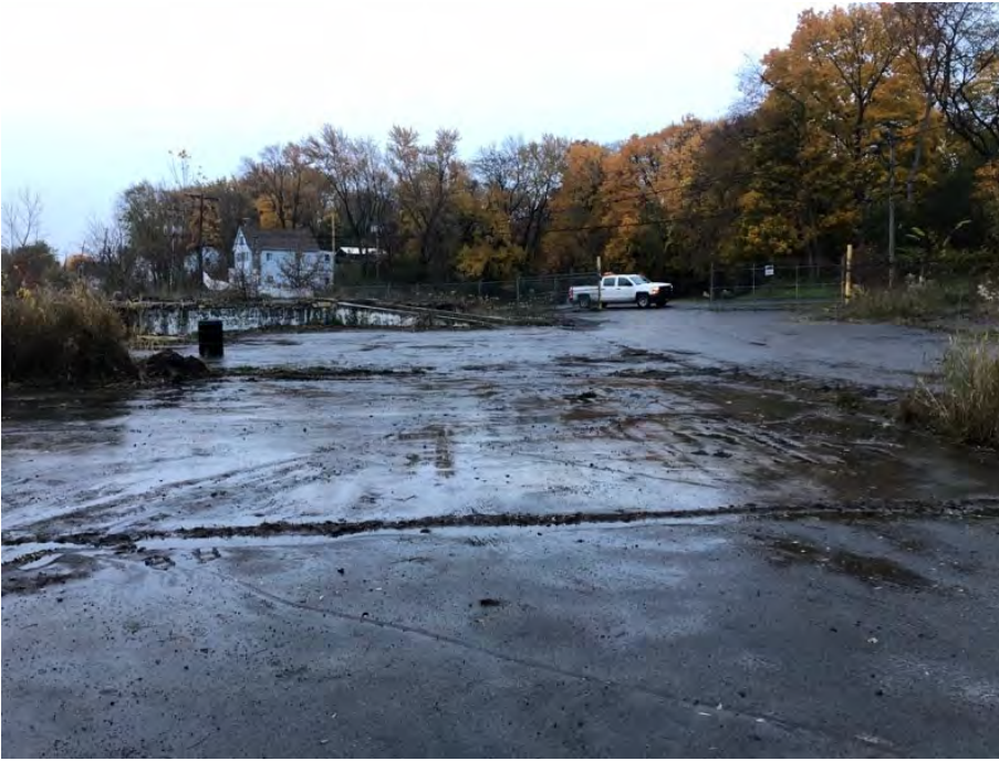
South entrance looking northeast. Fence appears in good condition.
