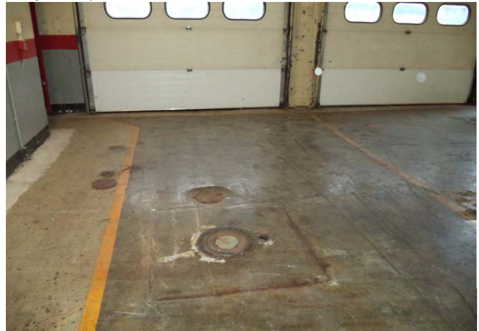
Trench and lift cylinder with free product
