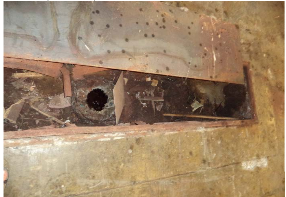
Trench and lift cylinder with free product
