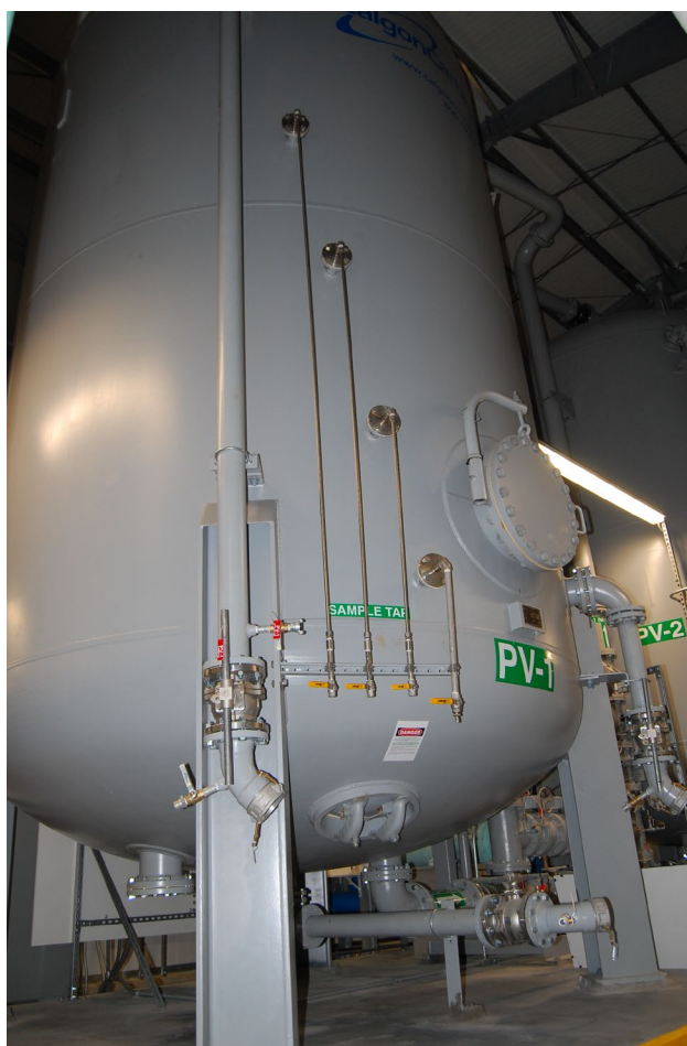
Figure 2: Steel vessel containing granular activated carbon.
