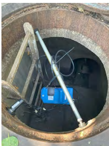
Graphic 2: Deployment of example flow monitoring equipment.
