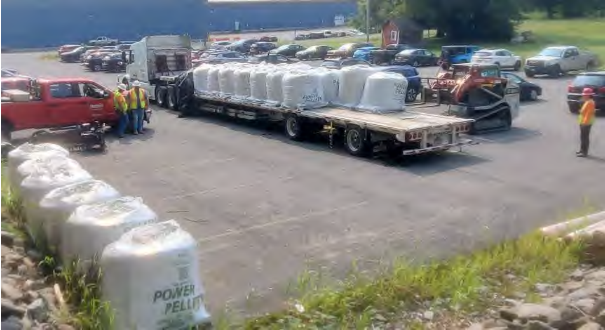
Photo 3: Unloading and staging Power Pellet supersacks using skidsteer
