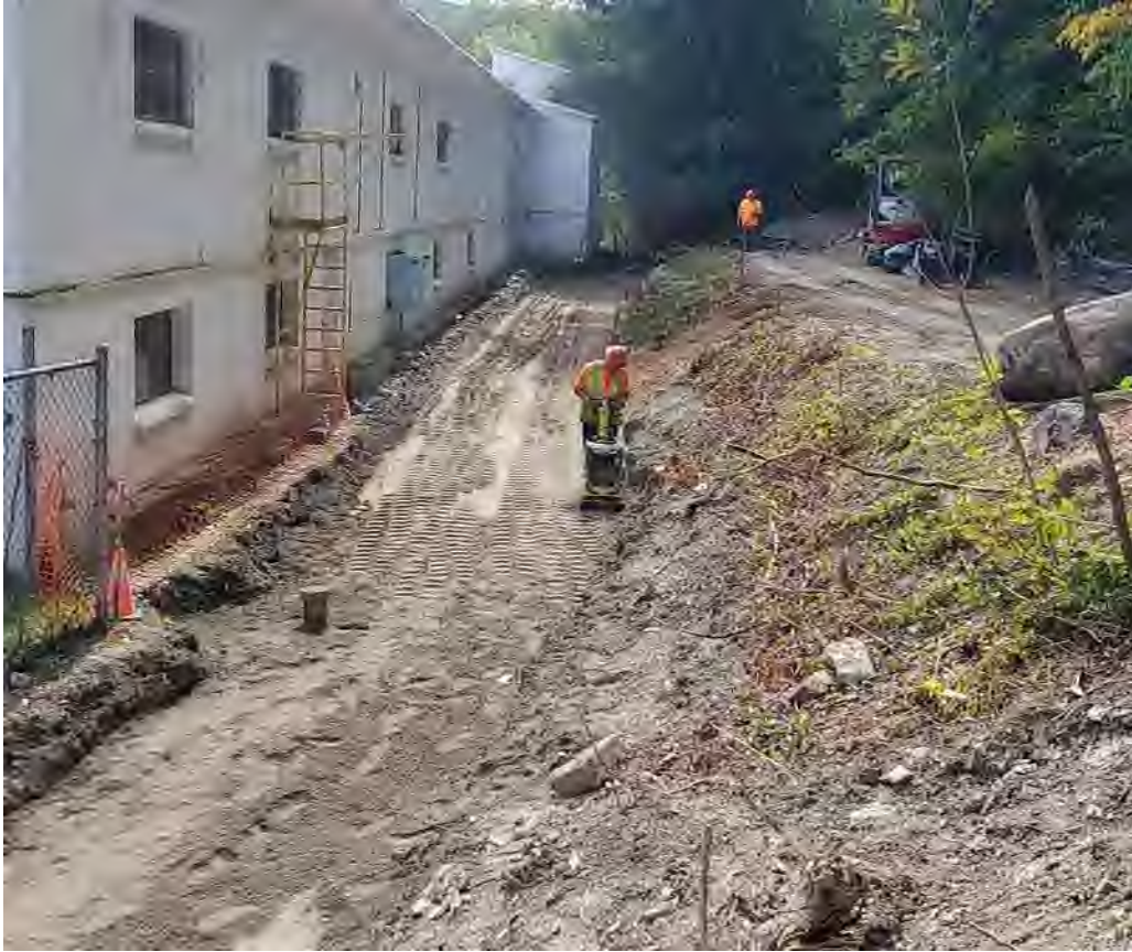
Photo 3: Using plate compactor to compact ROB backfill in swale
