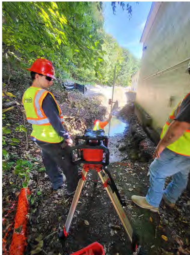
Photo 4: Setting up Rotary Laser Level at western limit of swale
