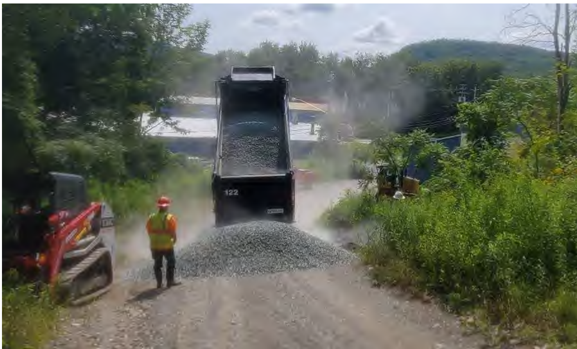
Photo 3: Unloading, spotting delivery of #2 crushed stone
