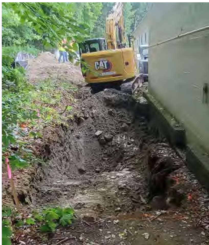
Photo 2: Excavation at northwest end of swale, looking northeast
