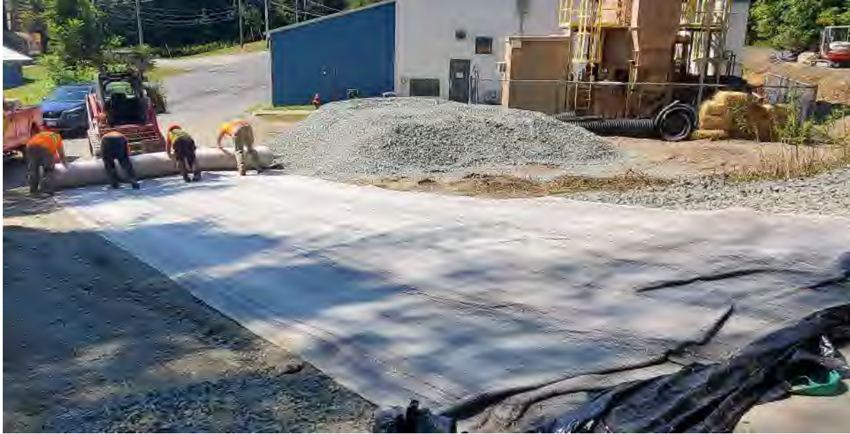
Photo 1: Crew unrolling GCL along road to cut into segment for placement
