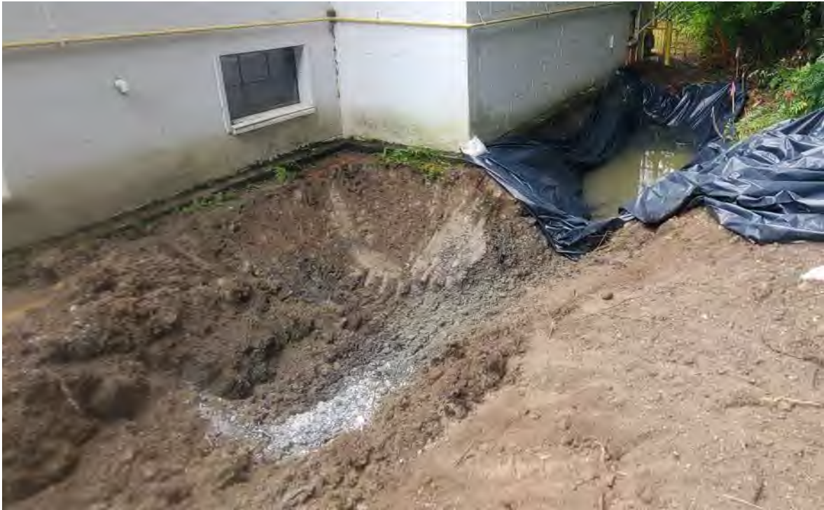
Photo 1: Northwestern end of swale excavation after heavy rainfall event
