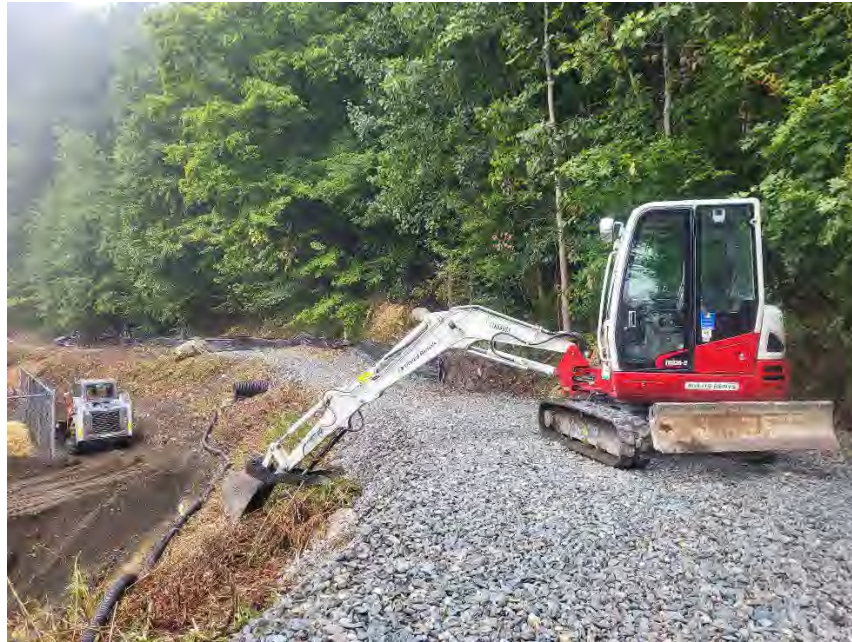
Photo 1: Mini-Excavator blocking entrance to road along swale overnight
