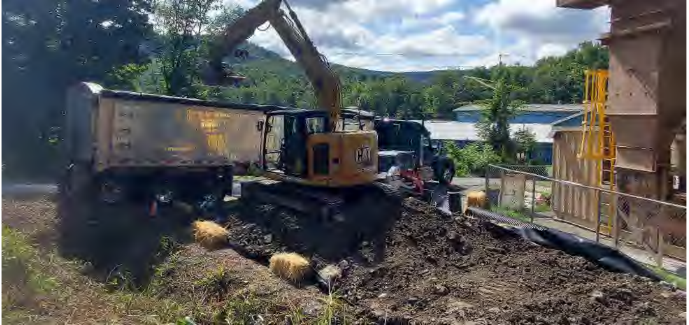
Photo 1: Excavator loading stockpiled soils into lined end-dump for hauling to disposal facility
