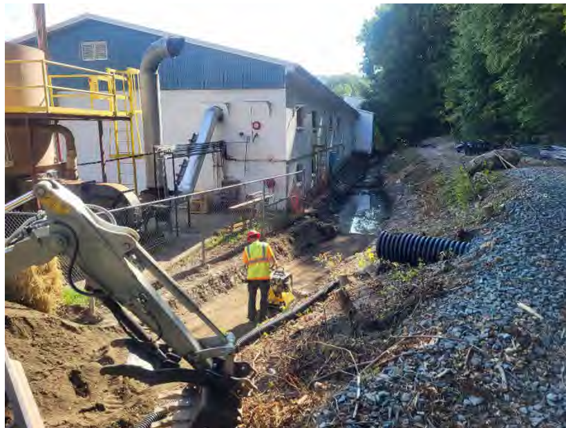
Photo 4: Compacting first layer of ROB with Compactor
