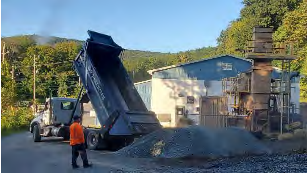
Photo 1: Spotting delivery and dumping of #1 stone, for cover placement in swale
