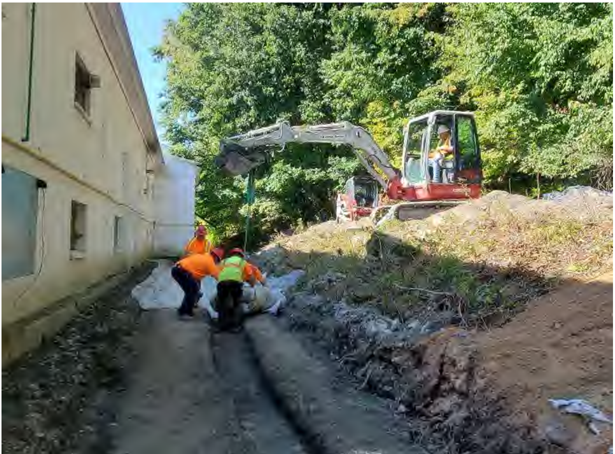
Photo 2: Using straps and mini-excavator to lower bundled GCL into swale for placement
