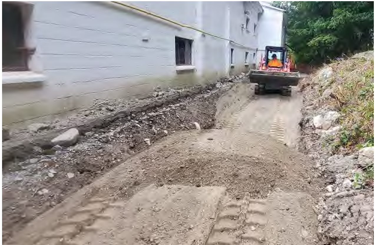
Photo 2: Skidsteer placing ROB backfill into swale
