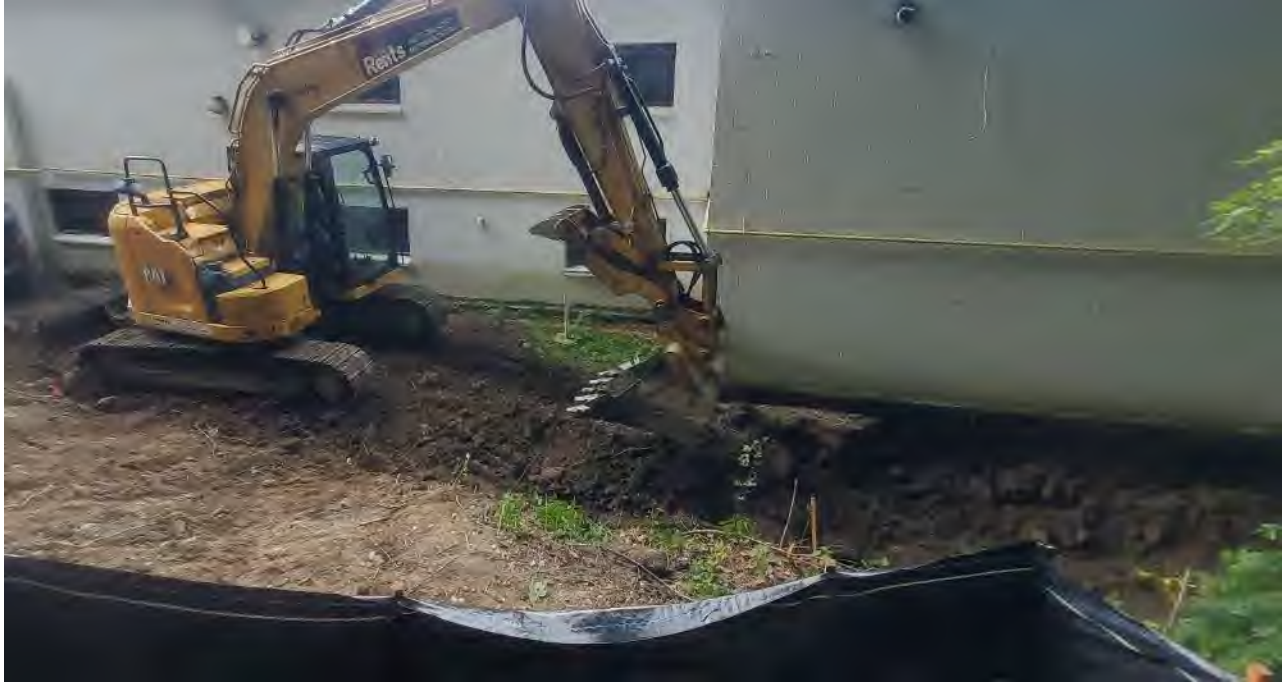
Photo 3: Swale excavation along north side of Building I, looking south
