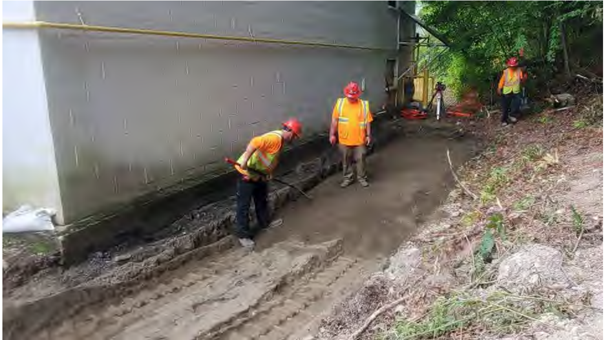
Photo 1: Hand-grading backfill surface at western end of swale
