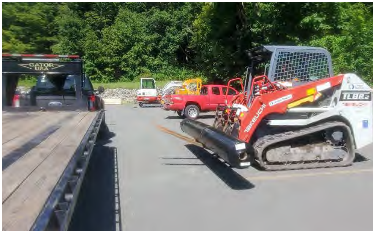
Photo 1: Clean Harbors unloading geotextile roll using skidsteer
