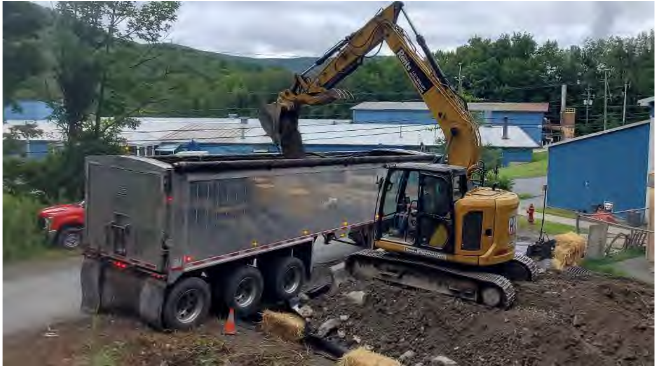
Photo 1: Excavator loading stockpiled soils into lined end-dump for hauling to disposal facility
