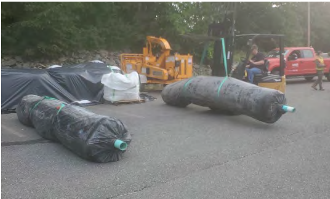
Photo 1: Unloading, staging GCL rolls
