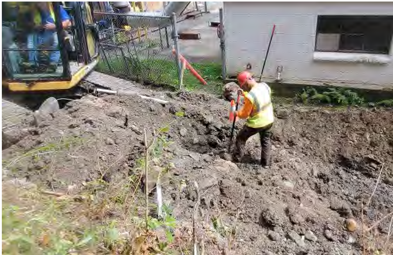
Photo 2: Hand-digging around existing water valve withing excavation limits
