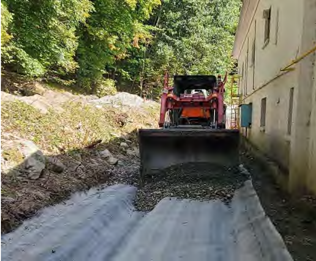
Photo 3: Placing stone cover over GCL using skidsteer
