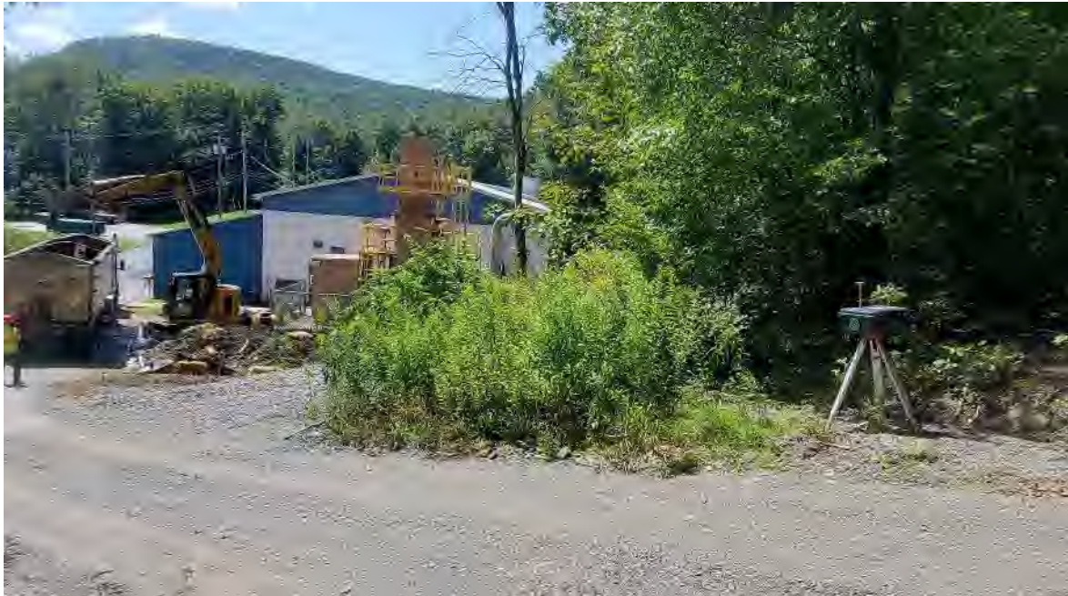
Photo 3: CAMP equipment setup to monitoring dust/particulate downwind from soil loadout area
