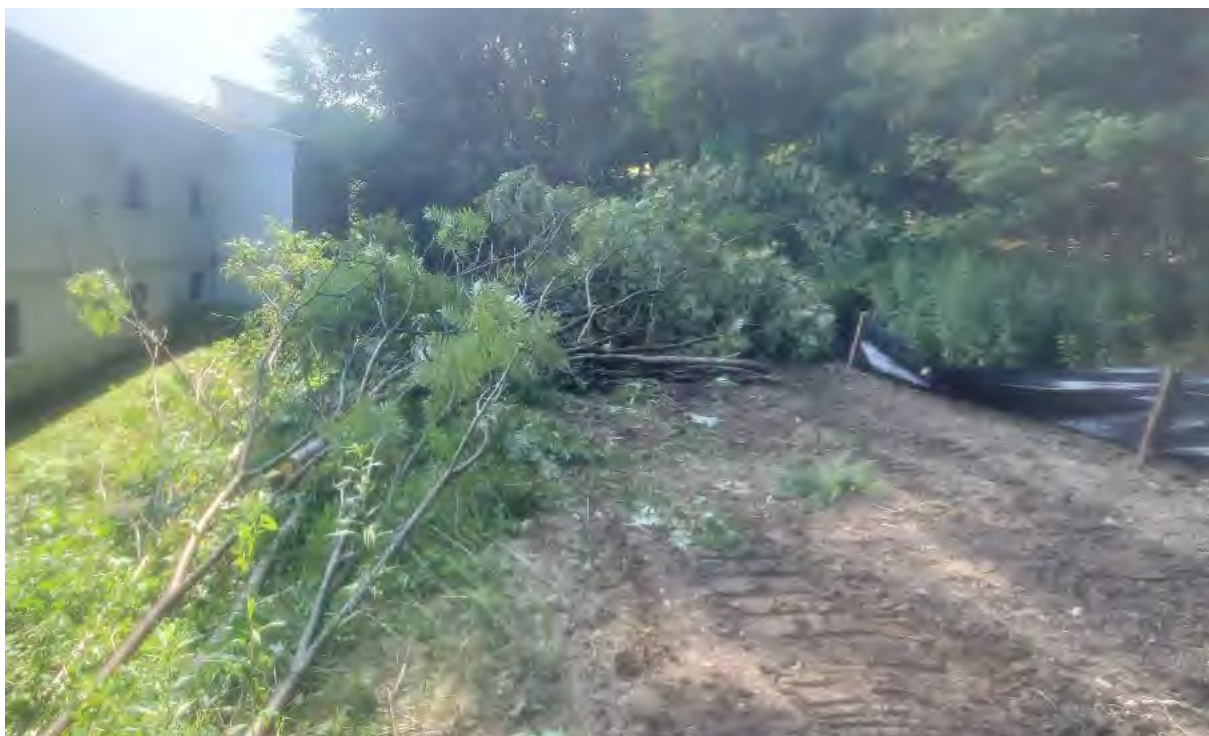
Photo 2: Cleared brush along access road, staged for chipping/mulching.
