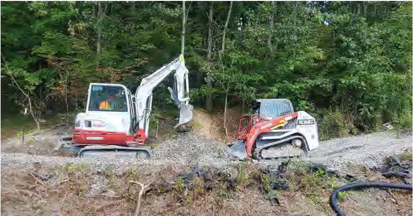
Photo 2: Using mini-excavator and skid steer to remove excess stone from temporary access road for placement within swale as stone cover
