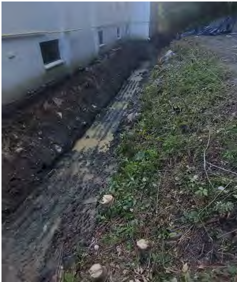
Photo 3: Swale excavation along north side of Building I, looking northwest
