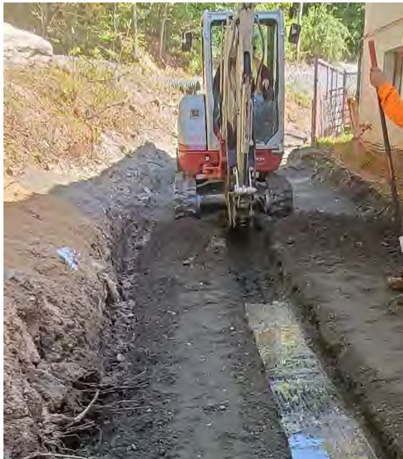
Photo 2: Mini-excavator digging swale grade and slope in preparation of GCL placement, looking east
