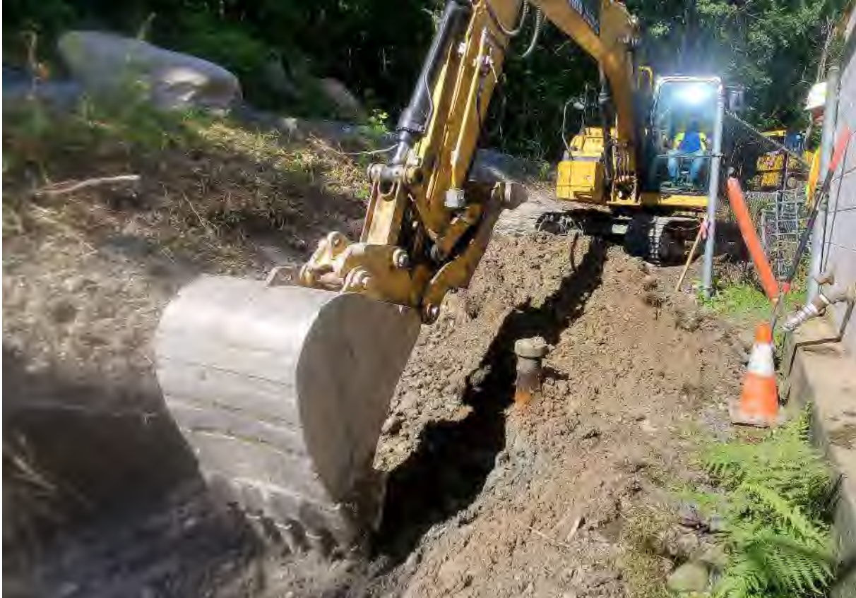
Photo 3: Swale excavation along northeast corner of Building I, water valve exposed
