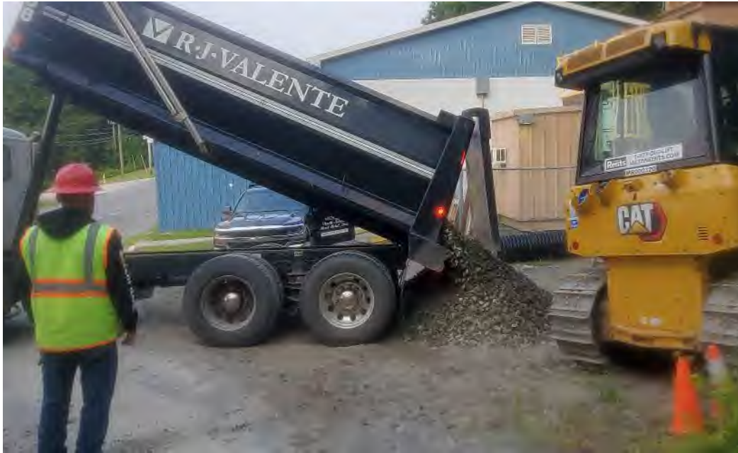
Photo 1: Dump truck unloading #3 crushed stone
