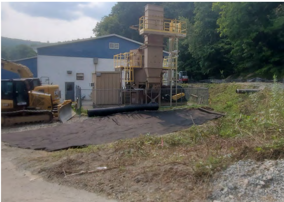
Photo 4: Geotextile fabric laid down to prep for stockpile containment area
