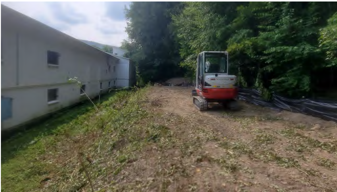
Photo 3: North side of building 1, vegetation cleared, prepped for excavation
