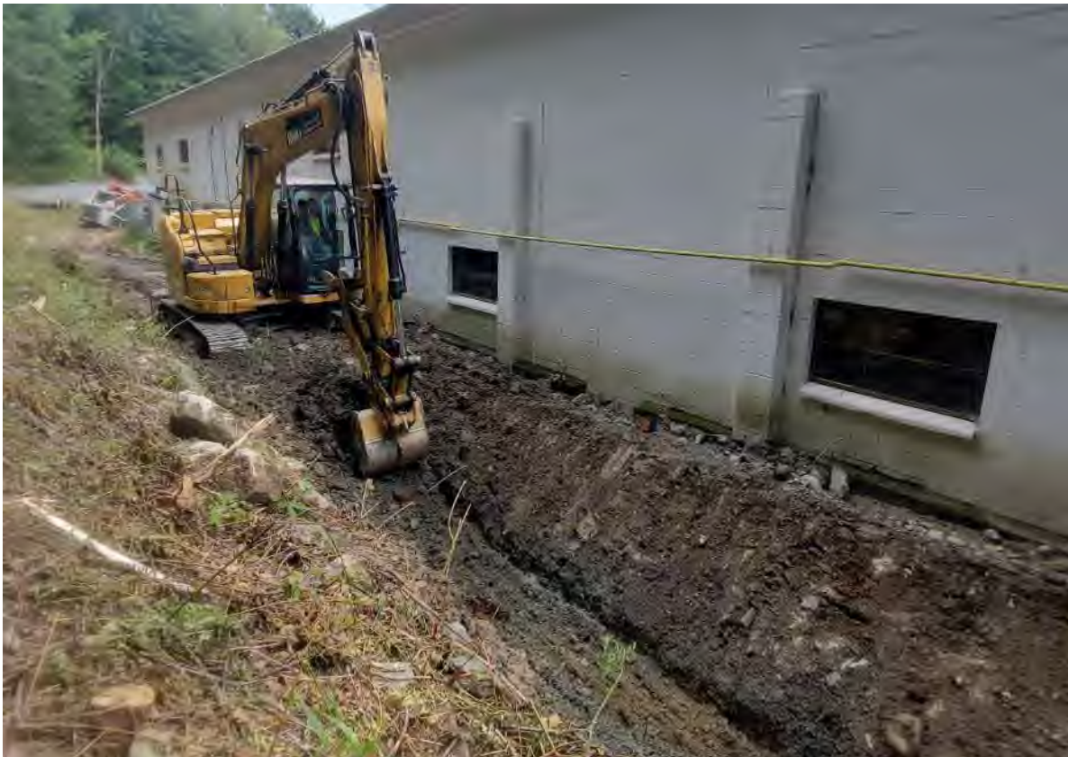
Photo 2: Excavating soils along the north side of Building I, looking southeast
