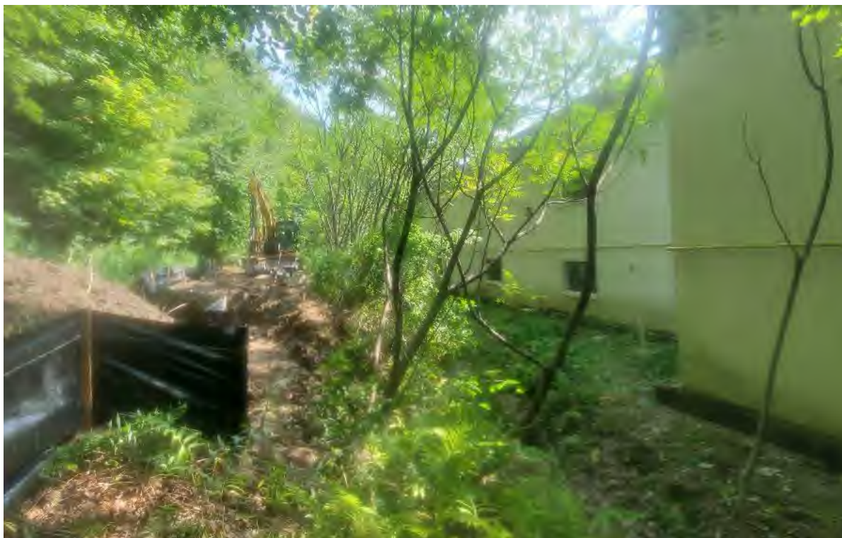
Photo 1: Access road clearing and silt fence installation at northwestern side of excavation limits
