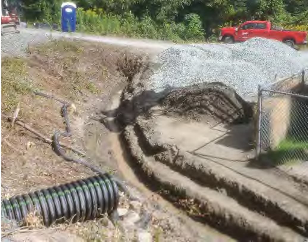
Photo 3: Eastern end of swale, backfill subgrade finished prior to GCL placement, looking east
