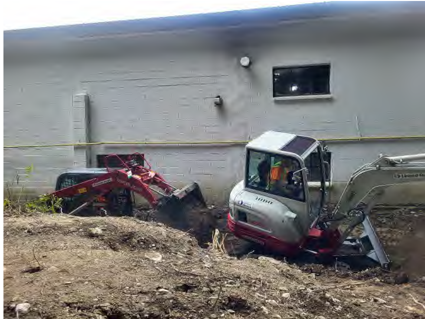
Photo 1: Skidsteer bringing backfill towards Mini-Excavator
