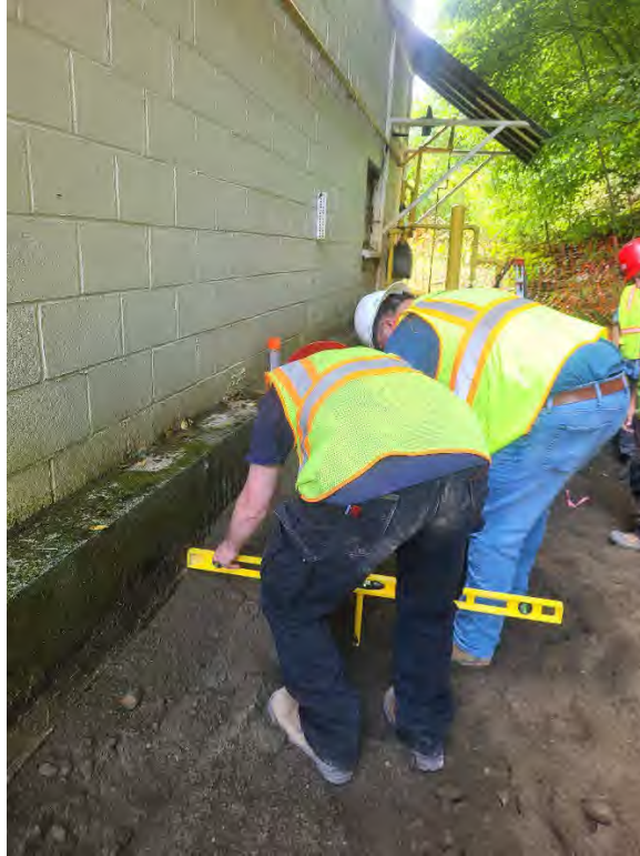
Photo 3: Measuring grade using tape measurer and level
