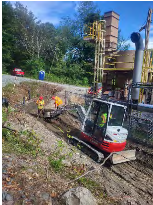
Photo 4: Digging out ramp made of backfill using rake, shovel, and Mini-Excavator
