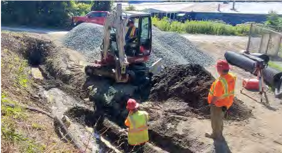
Photo 1: Using mini-excavator to grade swale at eastern end
