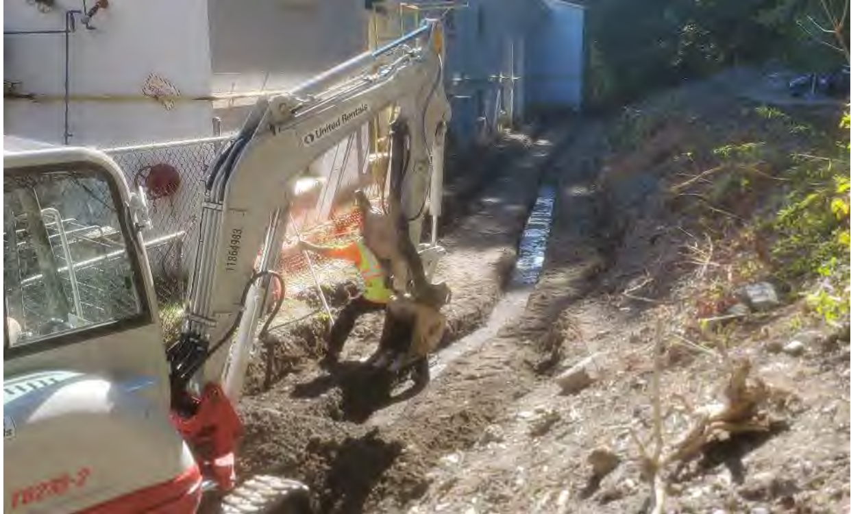
Photo 3: Mini-excavator digging swale grade and slope in ROB backfill, looking west
