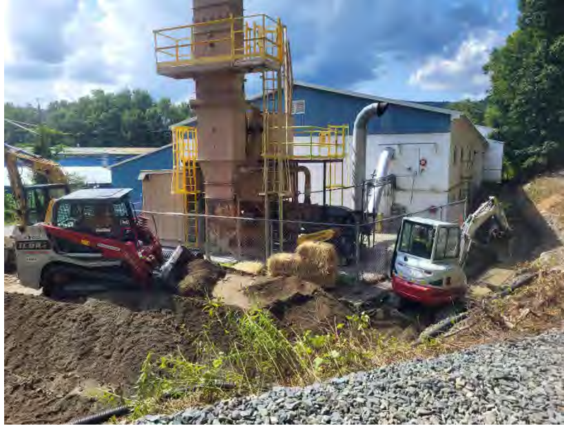
Photo 1: Skidsteer with bucket attachment brings ROB towards Mini-Excavator for backfilling
