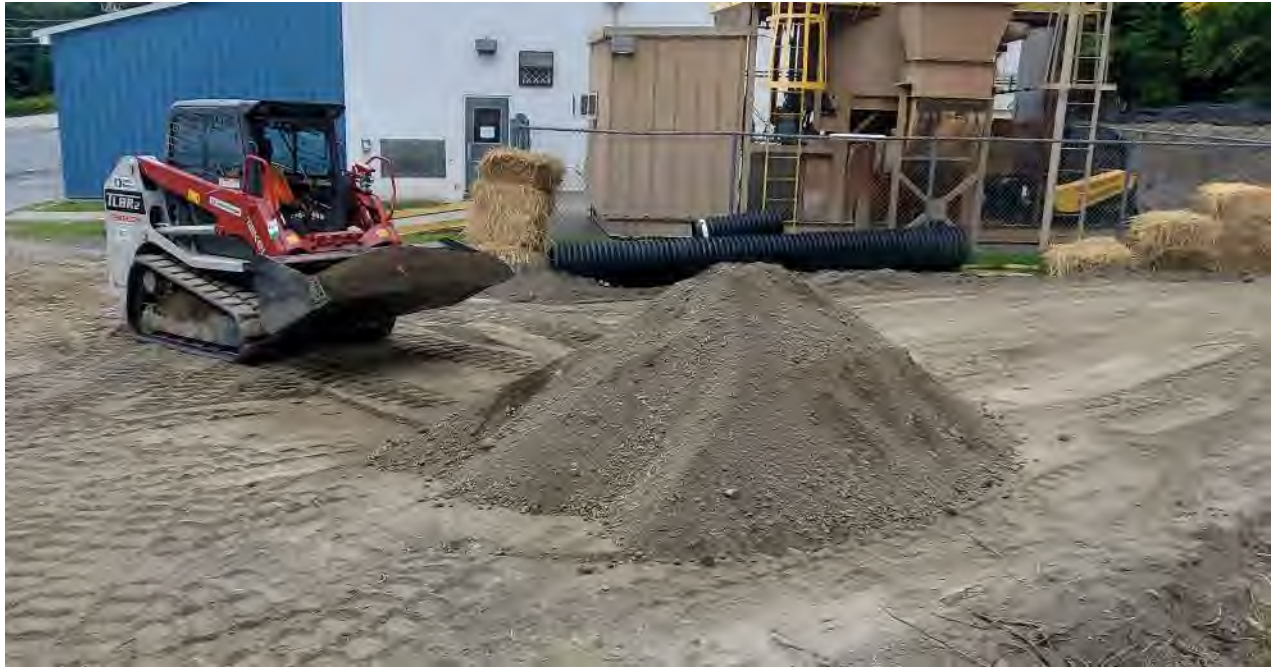
Photo 1: Skidsteer loading ROB backfill into bucket for placement into swale
