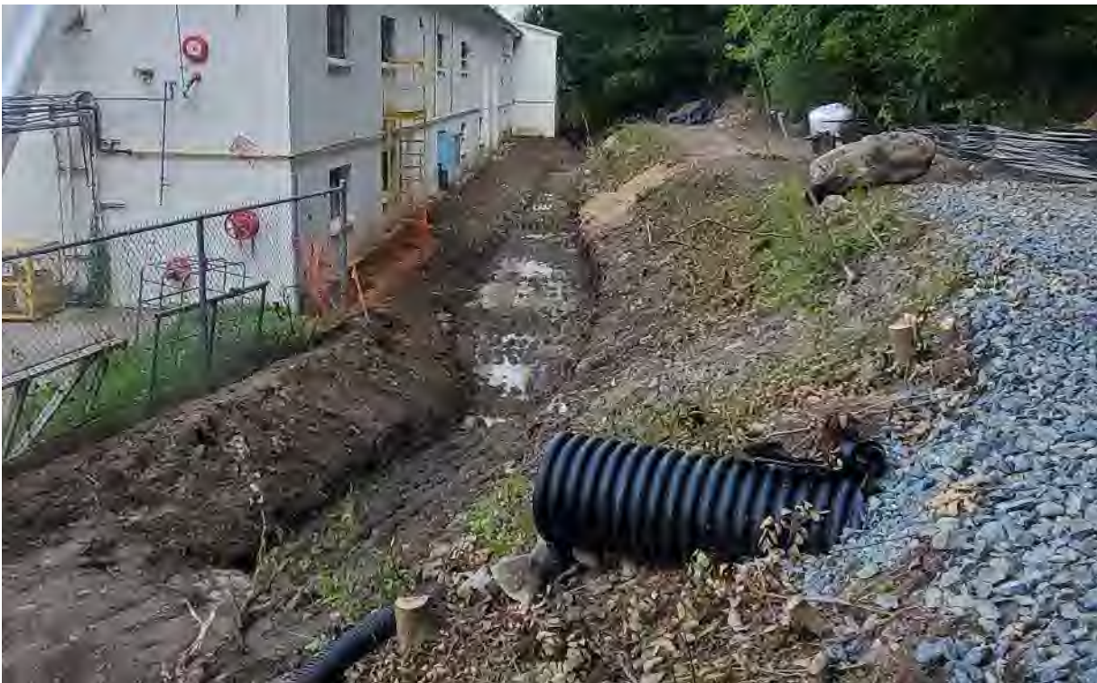
Photo 4: Completed excavation along northside of Building I, looking northwest
