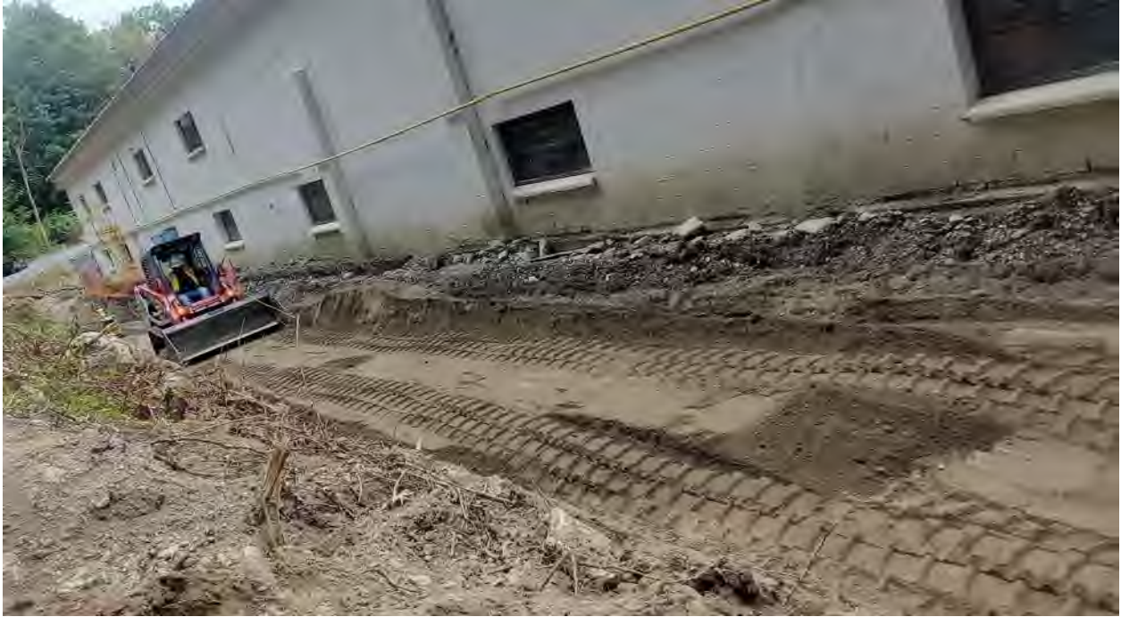
Photo 3: Skidsteer placing backfill and grading backfill surface
