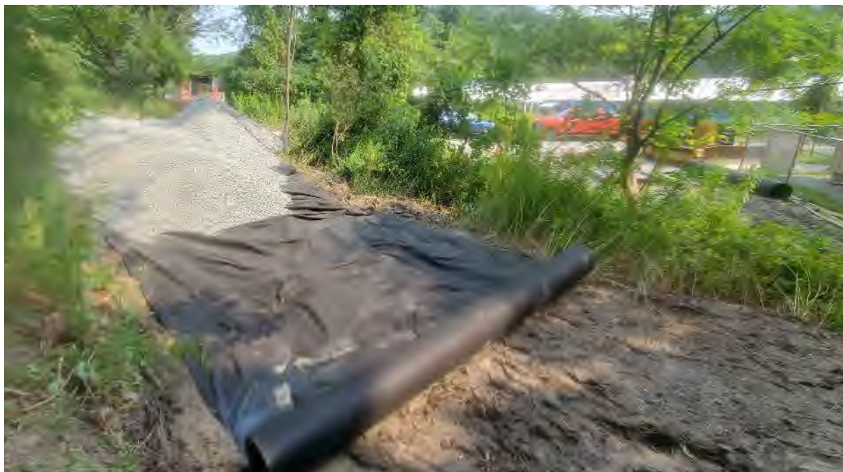
Photo 6: Geotextile fabric placed as separation layer on access road before placing #2 crushed stone
