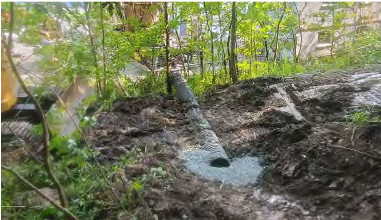
Photo 5: #2 crushed stone placement at HDPE Culvert inlet
