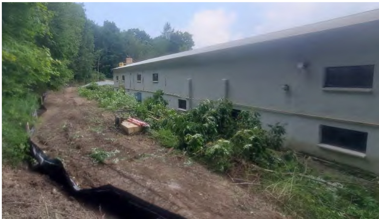
Photo 3: Access road cleared and grubbed, view looking east along north side of Building 1
