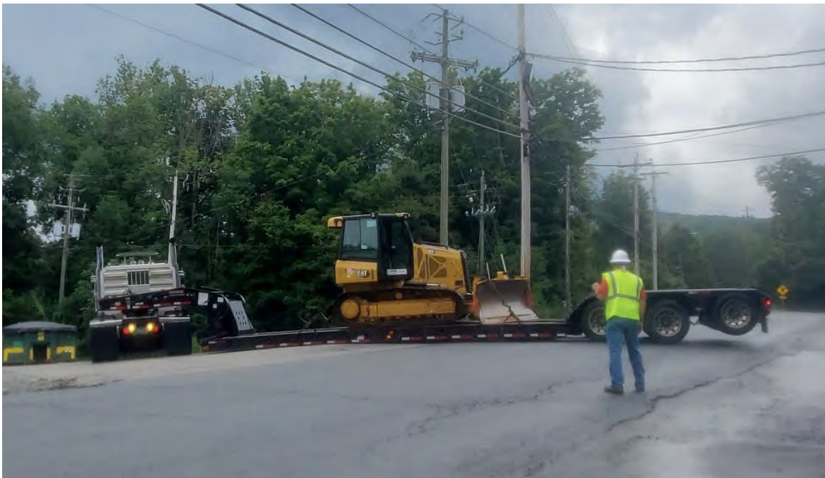
Photo 1: Clean Harbors spotting dozer delivery, unloading
