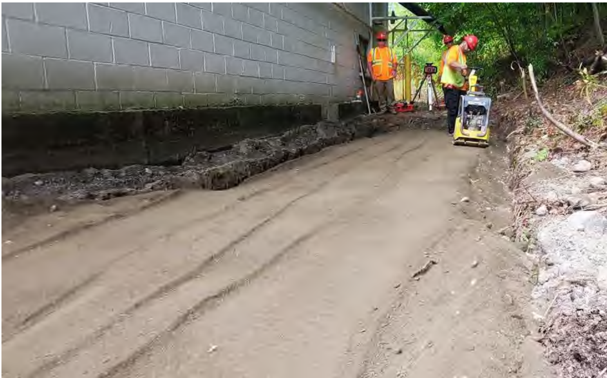
Photo 2: Using plate compactor to compact backfill surface
