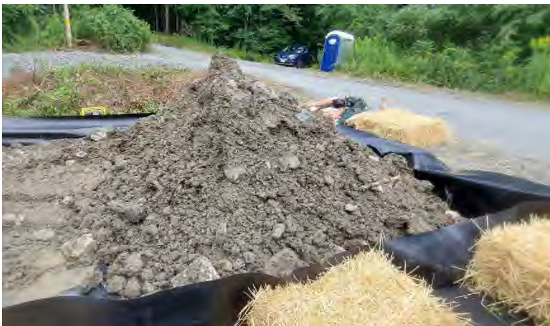
Photo 4: Stockpiled excavation soils in the containment area
