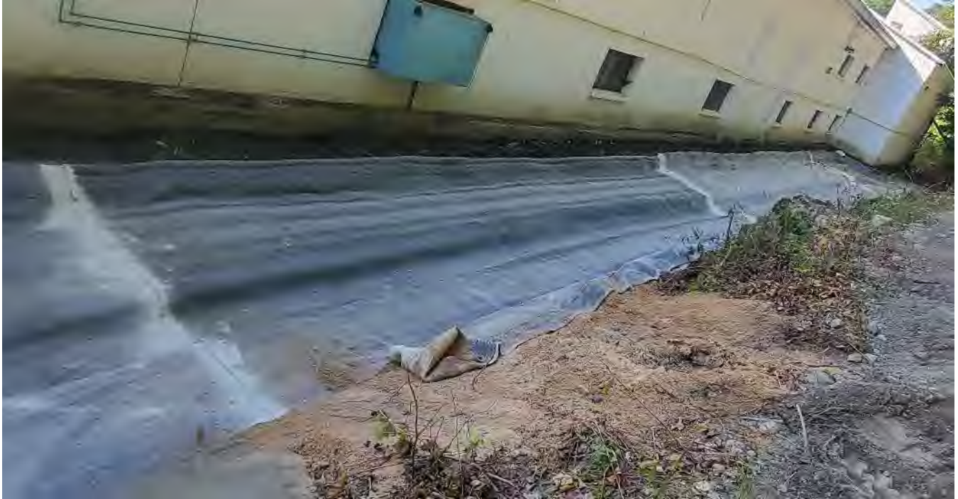
Photo 1: GCL placed in western half of swale, looking west
