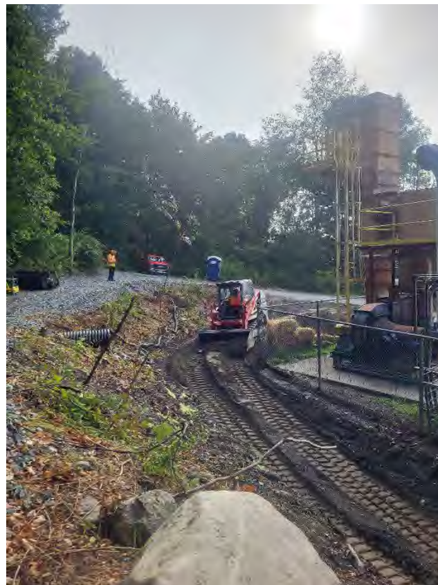
Photo 2: Ramp built with backfill along corner so that Skidsteer can easily bring backfill along swale
