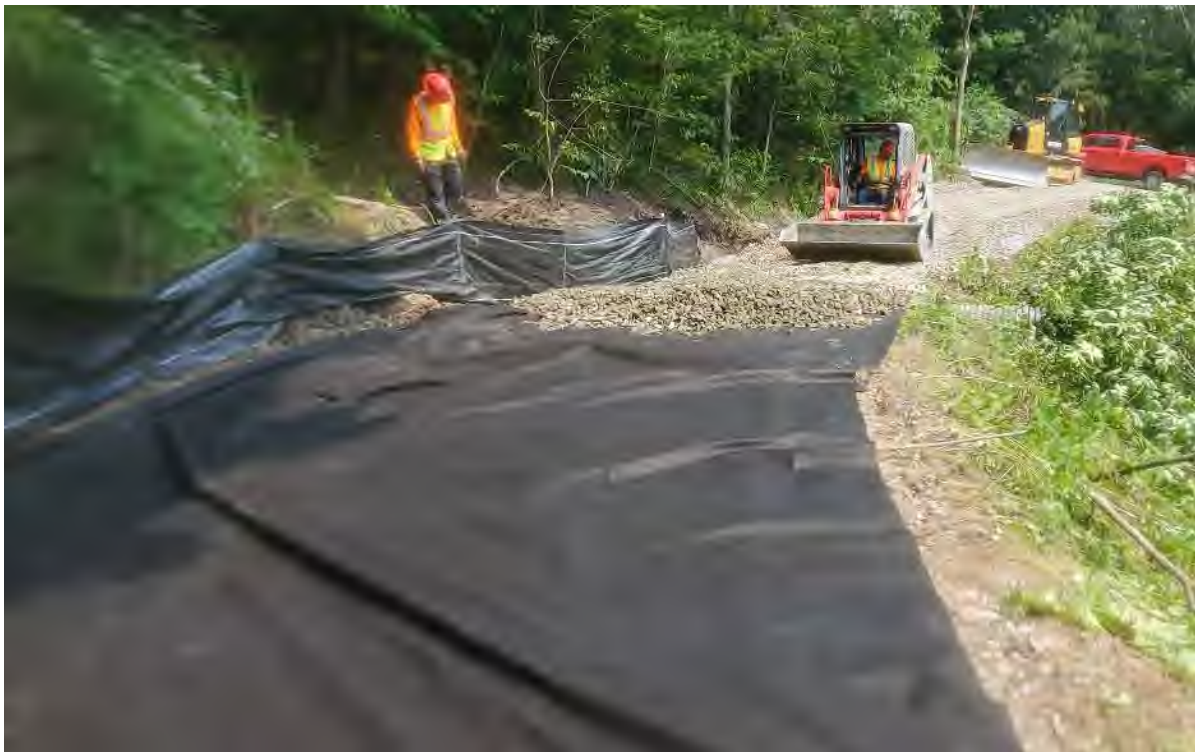
Photo 4: Skidsteer grading #3 stone over geotextile separation fabric along access road
