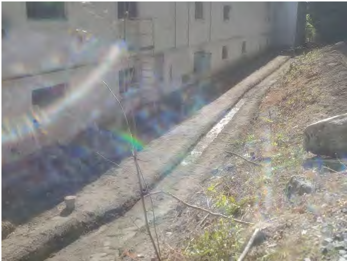
Photo 2: Western half of swale, backfill subgrade finished prior to GCL placement, looking west
