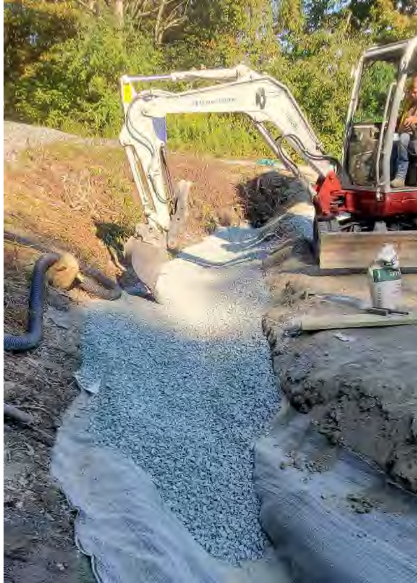
Photo 6: Placing stone cover over GCL in eastern end of swale, looking east
