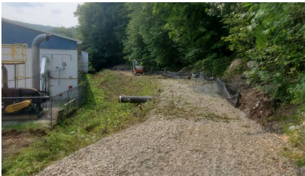
Photo 2: Access road established and cleared of vegetation, looking northwest
