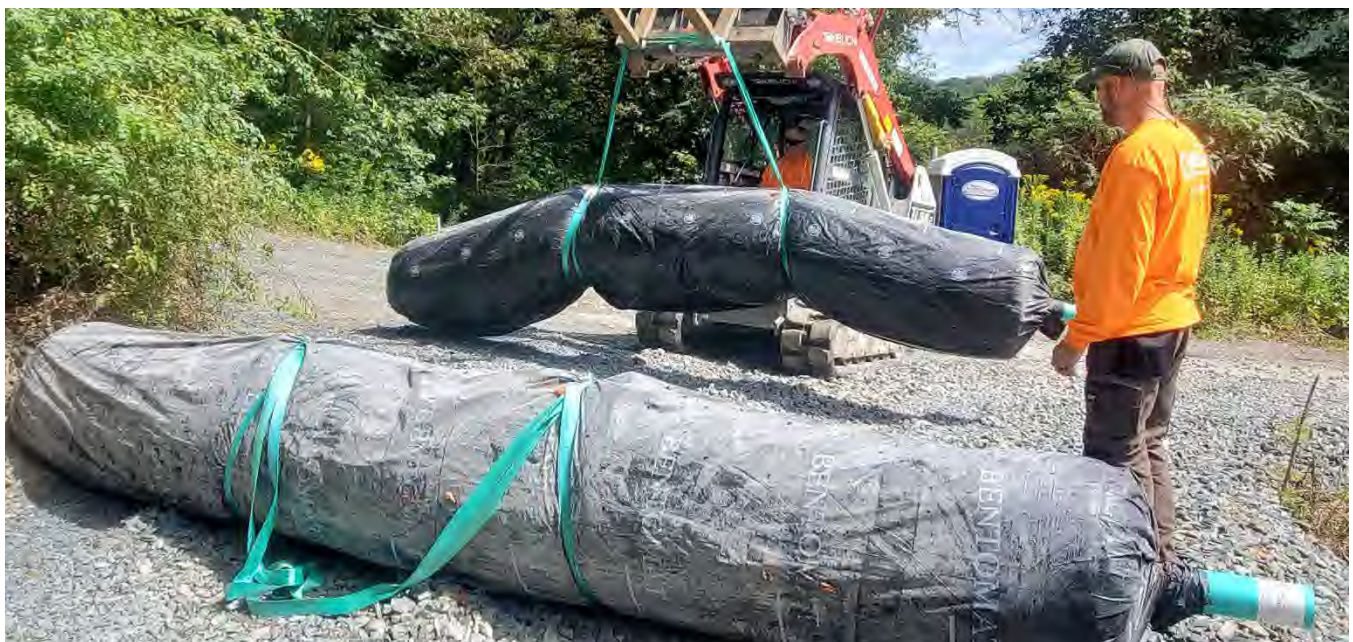
Photo 2: Moving and staging GCL rolls in preparation for placement
