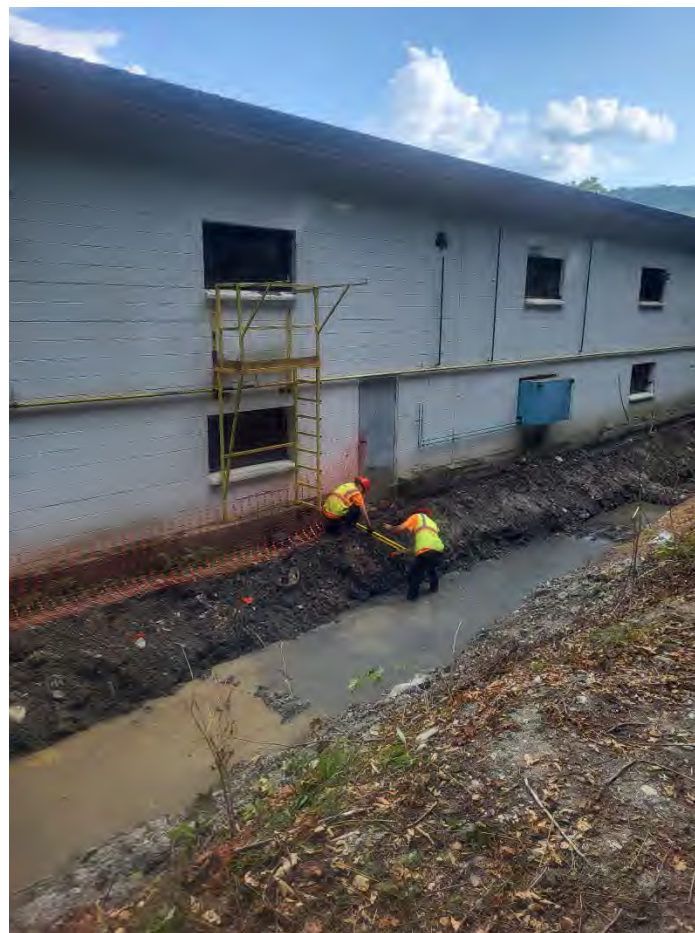
Photo 2: Using level to mark one foot below grade with orange spray can
