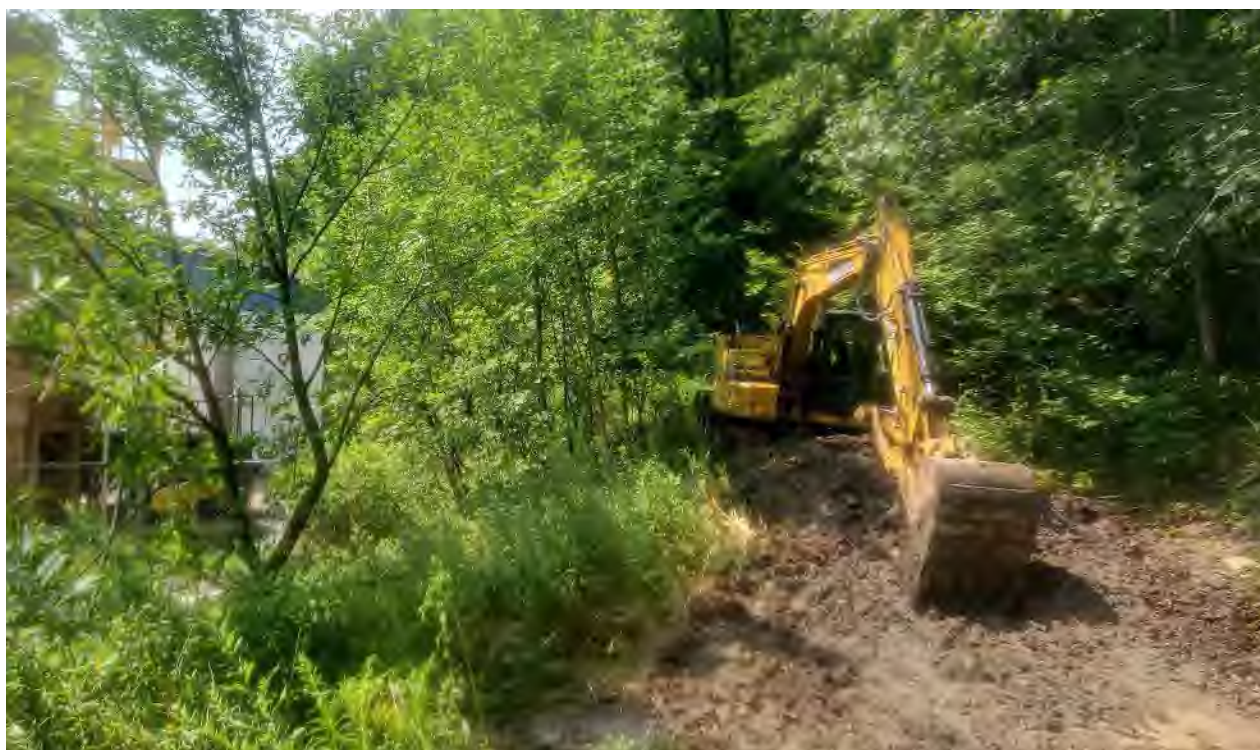
Photo 2: Excavator grading access road north of excavation area
