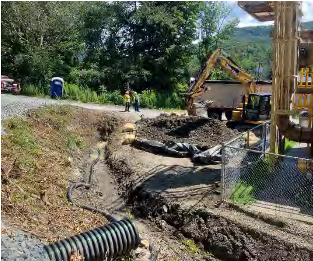
Photo 2: Eastern end of swale excavation completed
