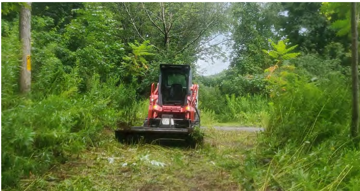
Photo 3: Skidsteer with Mower Attachment, attempted clearing access road
