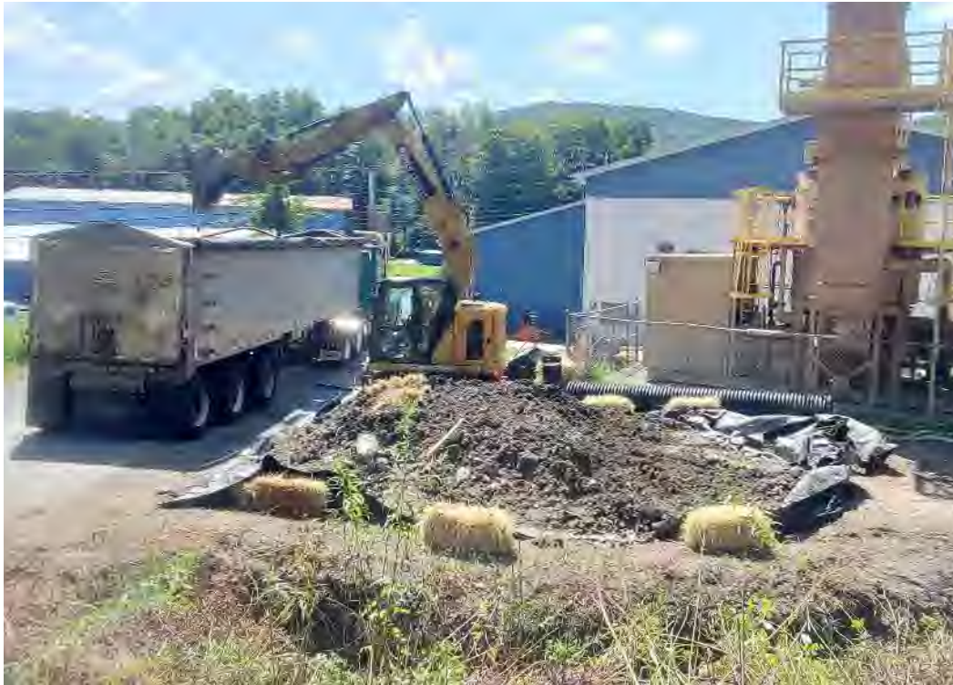
Photo 1: Excavator loading stockpiled soils into lined end-dump for hauling to disposal facility
