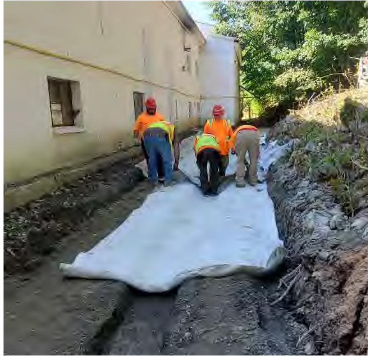
Photo 3: Unfolding GCL within swale and positioning for final placement, looking west
