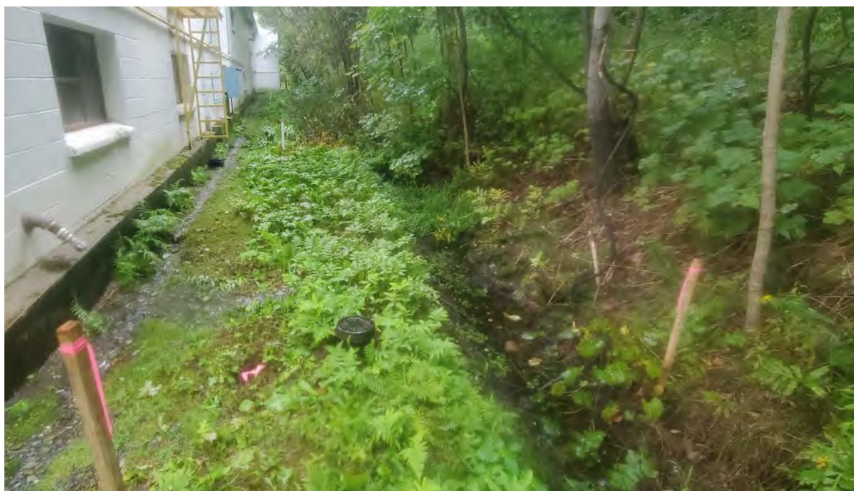
Photo 4: View of excavation limits along swale area, looking southwest
