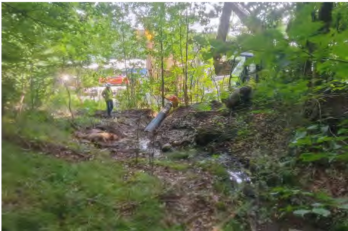
Photo 4: Placement of 15" dia. corrugated HDPE culvert under access road to allow for drainage
