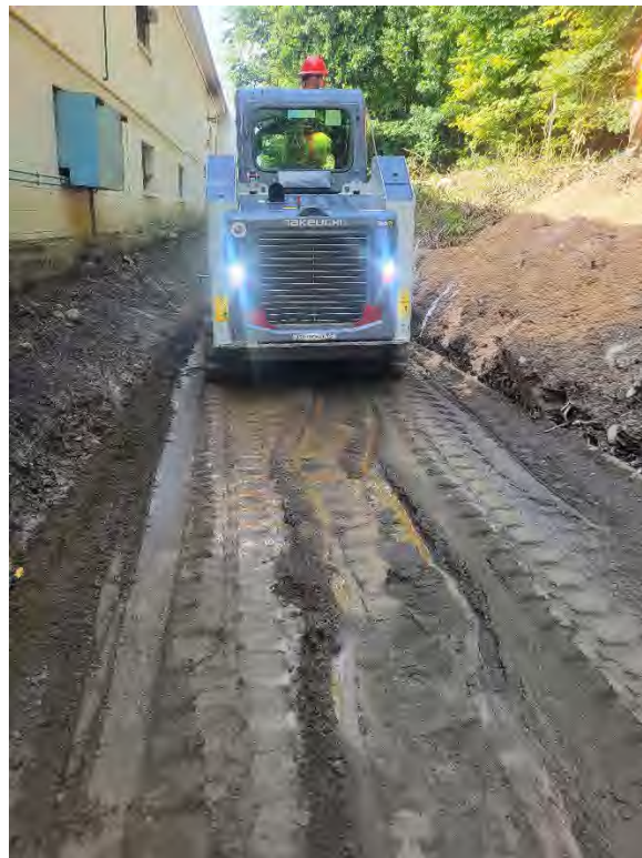
Photo 2: Visible water on top of backfill post using Compactor along center line
