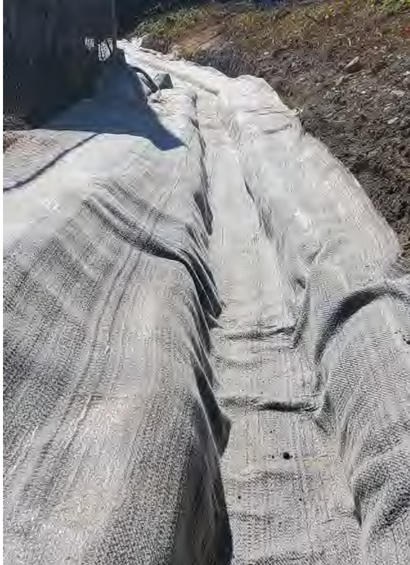
Photo 5: GCL placed in eastern end of swale, prior to cutting excess edges, view looking northwest
