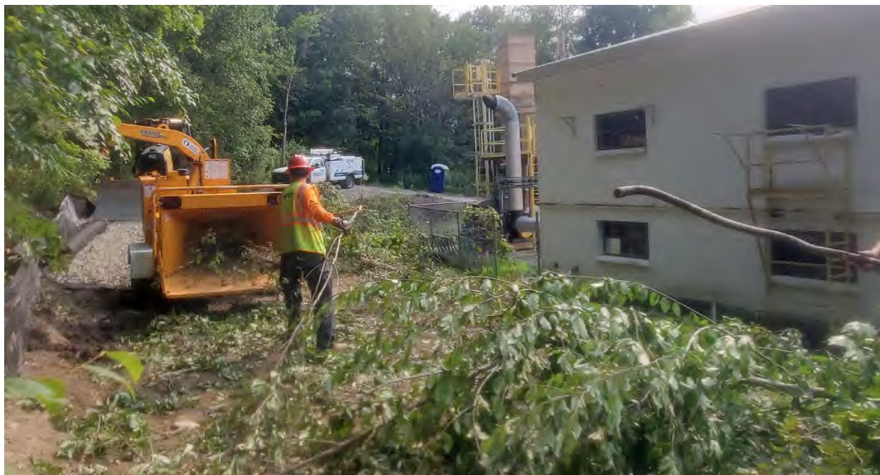
Photo 1: Crew using chipper to mulch cleared trees and vegetation
